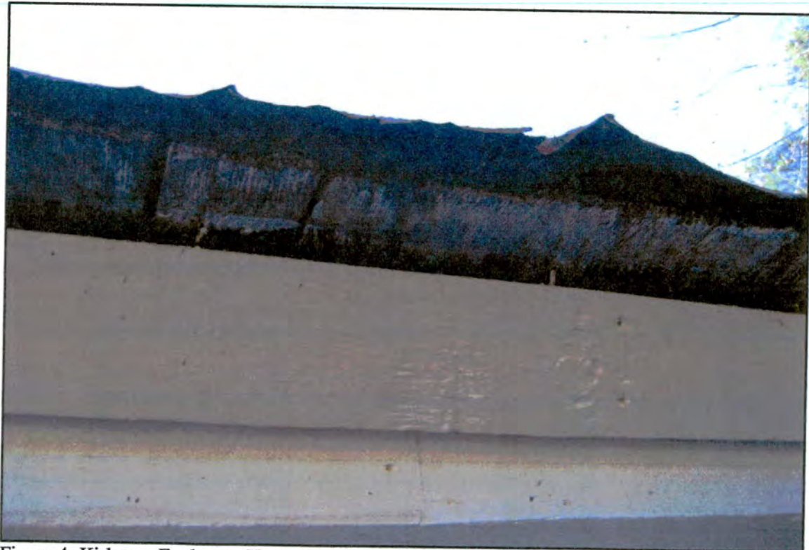
Figure 4: Kirkman-Fogleman House, detail showing wood shingles under pressed metal shingles
