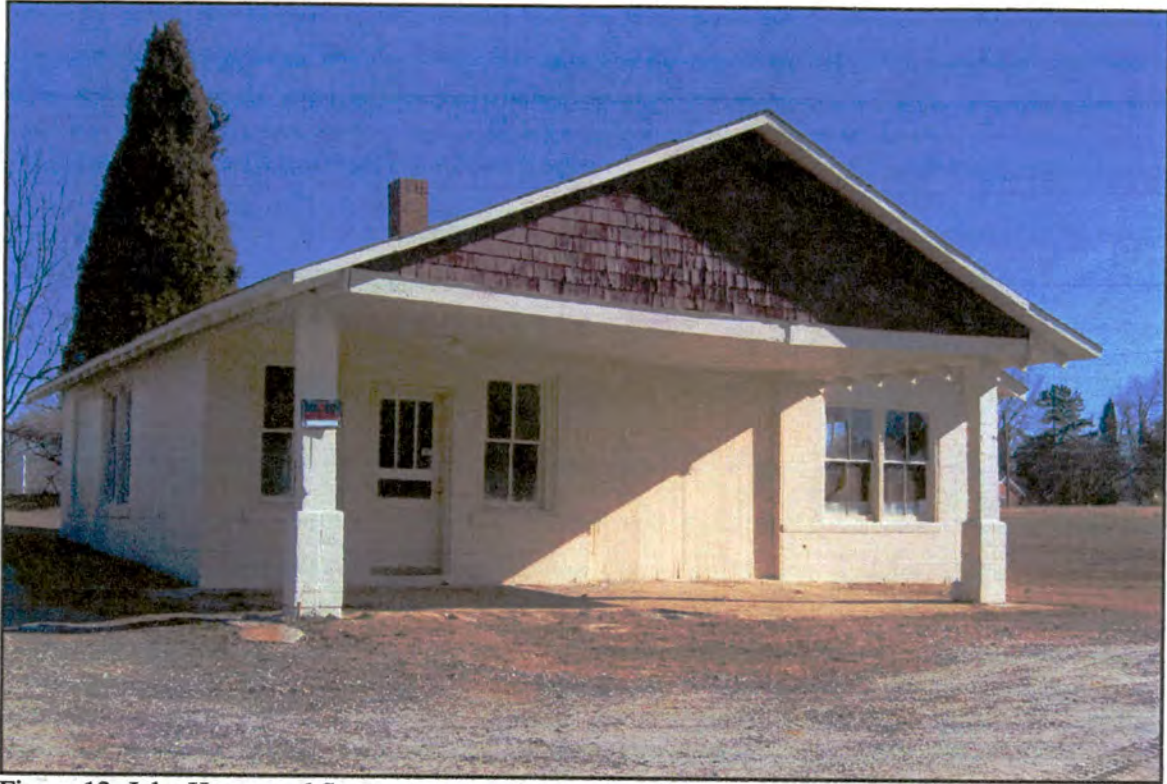
Figure 12: Jobe House and Store, store, southwest elevation
