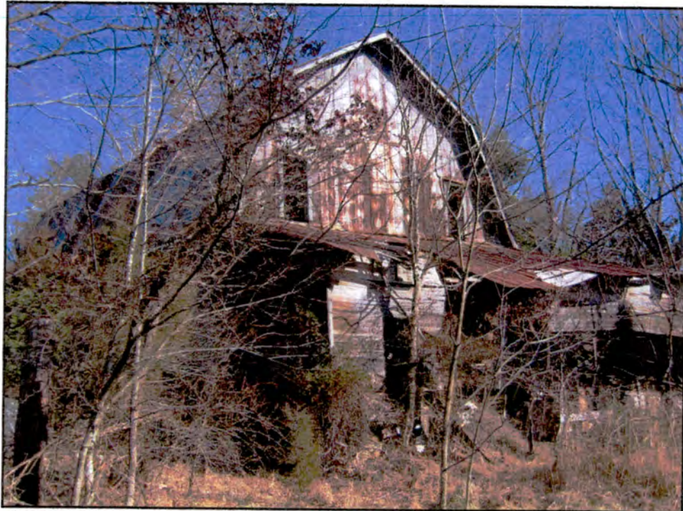
Figure 6: Kirkman-Fogleman House, gambrel-roof barn, south elevation
