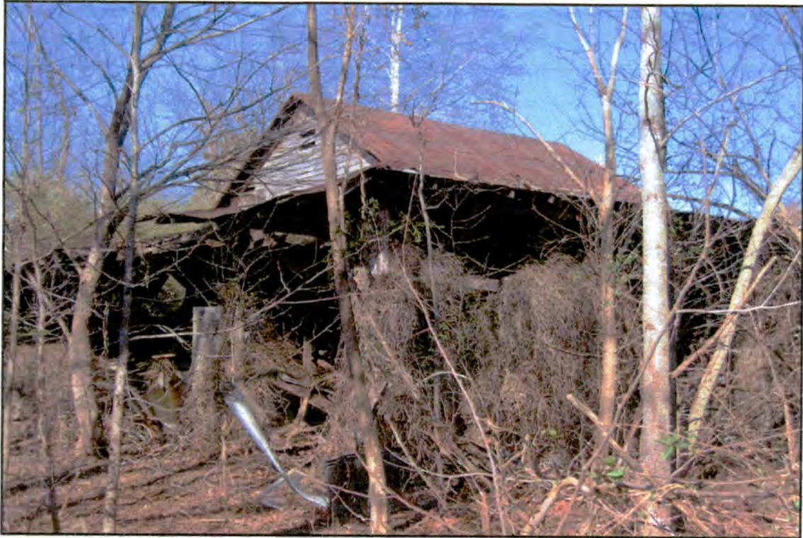
Figure 9: Kirkman-Fogleman House, barn, southeast corner
