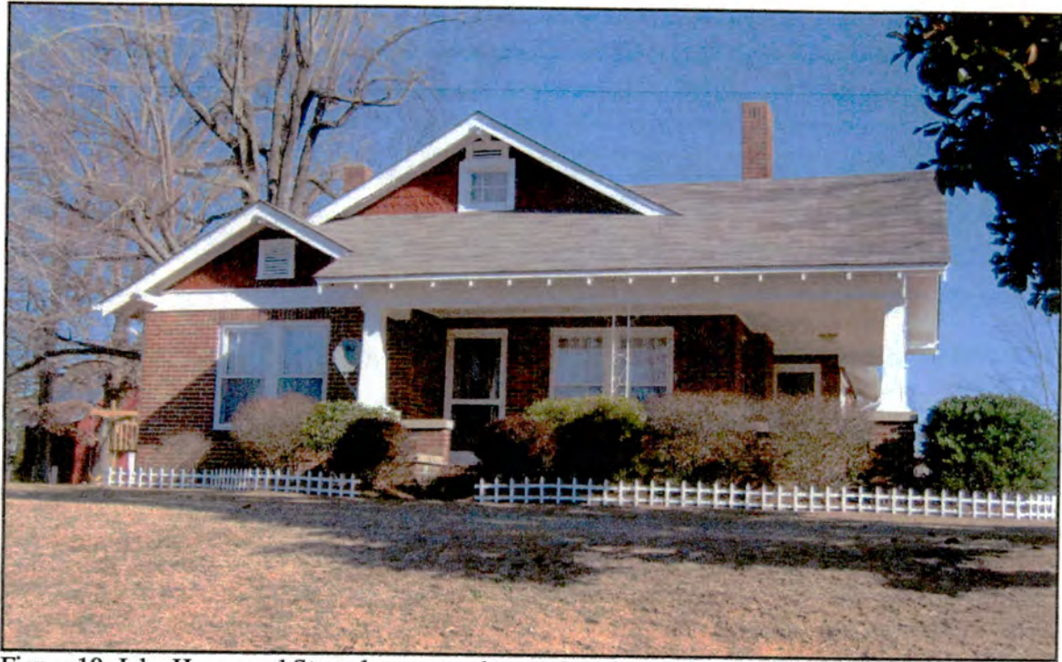
Figure 10: Jobe House and Store, house, southwest elevation
