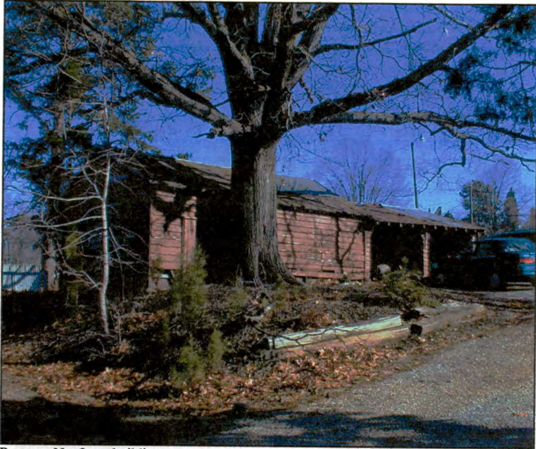
Property No. 3, outbuilding
