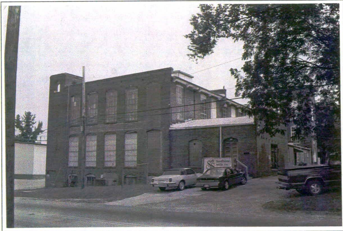
10. Sidney Cotton Mill: 1907 addition; pre-1931 stockroom to right; View A from SW.
