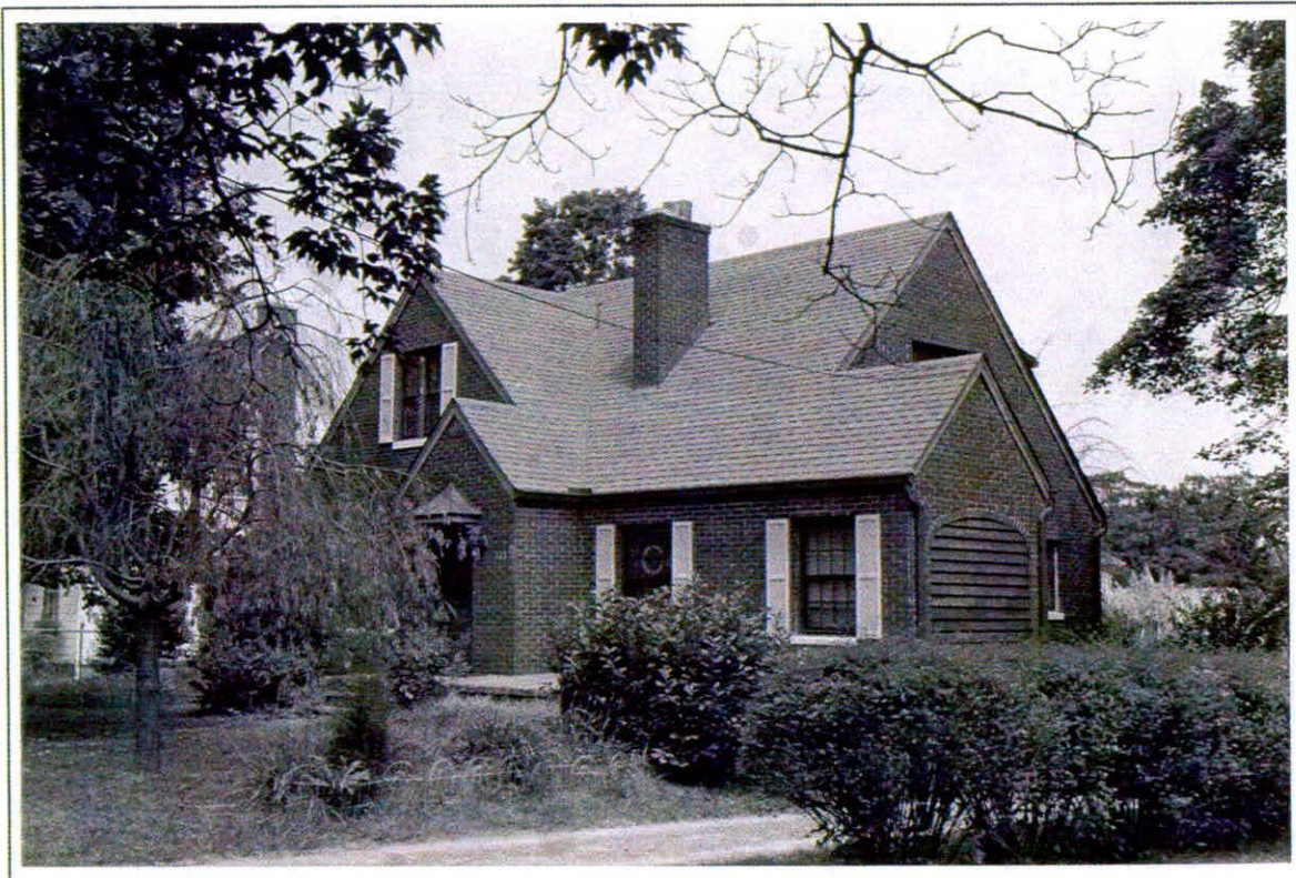
37. House, Tudor Revival, c.1931-43, N. Main St. H. D.
