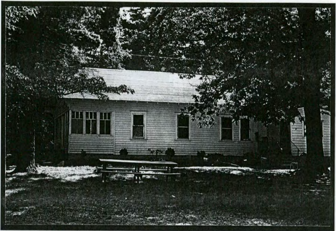
Hilgirt Court Shop
