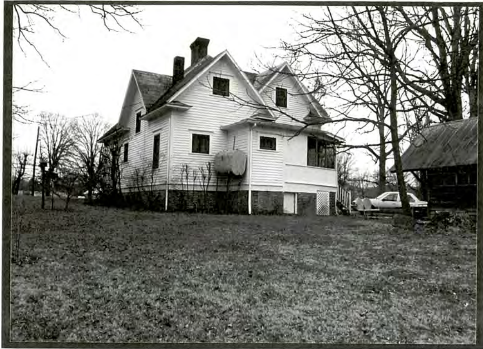
PLATE V.8 Cunningham-Poteat- Bagwell House (#9), west rear and north side elevations
