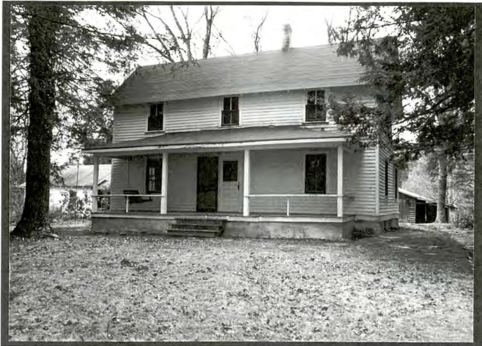
PLATE V.37 Liverett Farmhouse (#3), main house, northeast front and southwest side elevations
