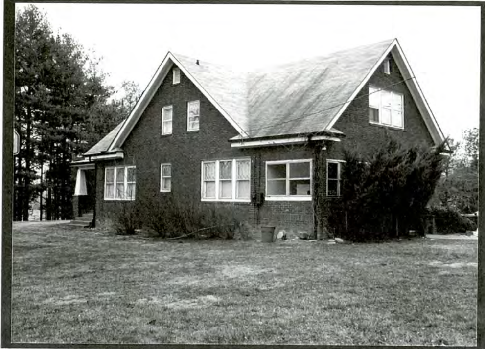
PLATE V.45 Bodenhammer House (#4), north side and west rear elevations
