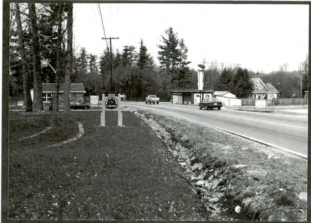
PLATE V.25 Mountain Home (#1), US 25 looking northeast towards junction with SR 1370
