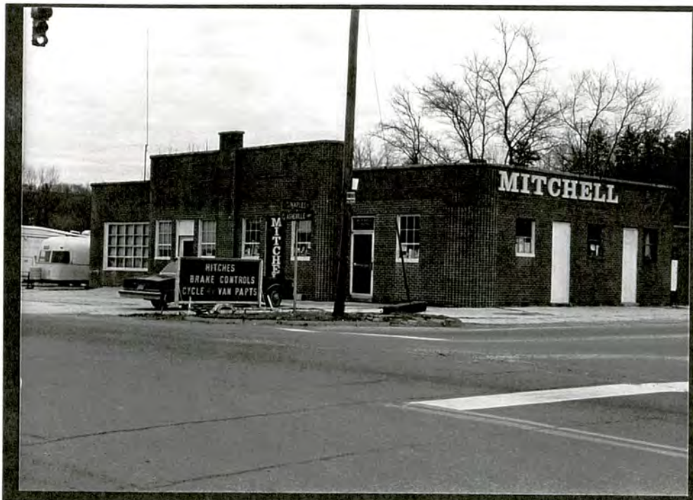
PLATE V.51 Mitchell Enterprises Building (#6), southwest front and southeast side elevations
