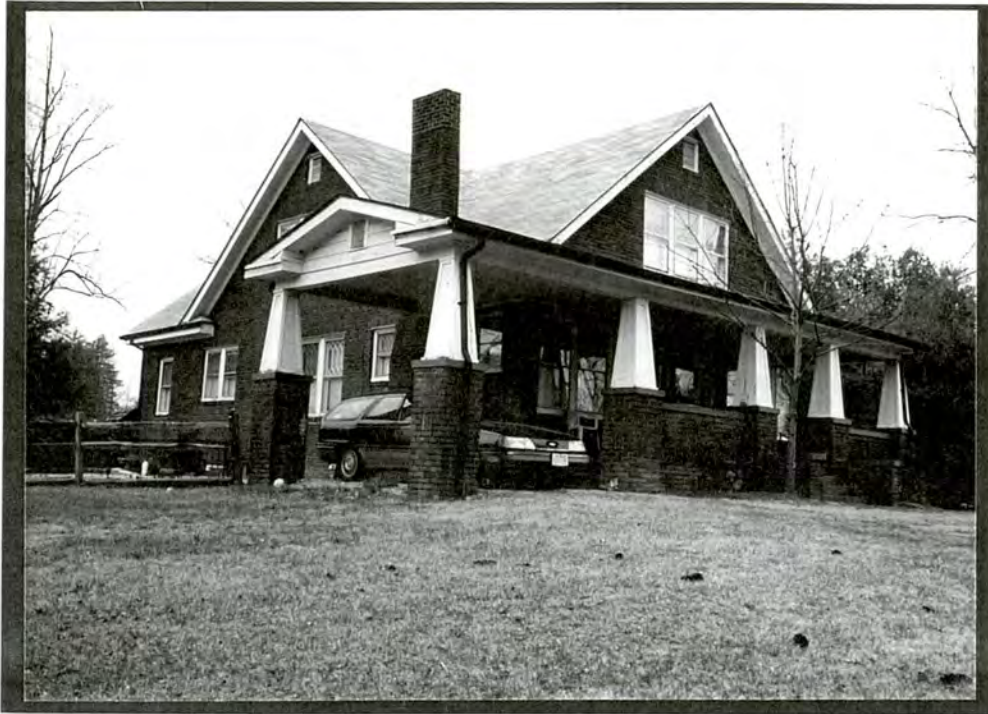
PLATE V.43 Bodenhammer House (#4), east front and south side elevations
