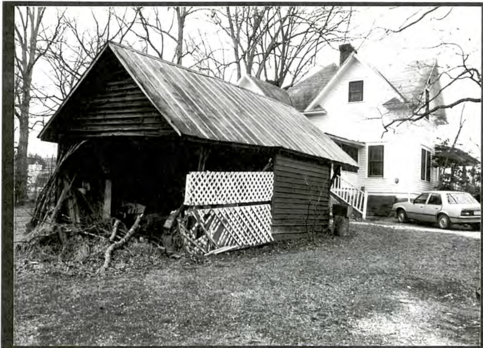
PLATE V.9 Cunningham-Poteat- Bagwell House (#9), shed to rear, facing northeast
