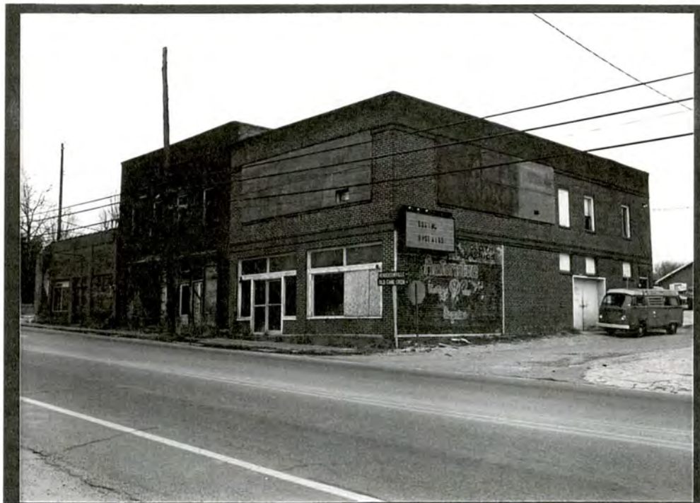
PLATE V.60 Fletcher Commercial District (#7), Early Commercial Buildings, [I] at right, [J] at left center, and [K] at far left, facing northeast
