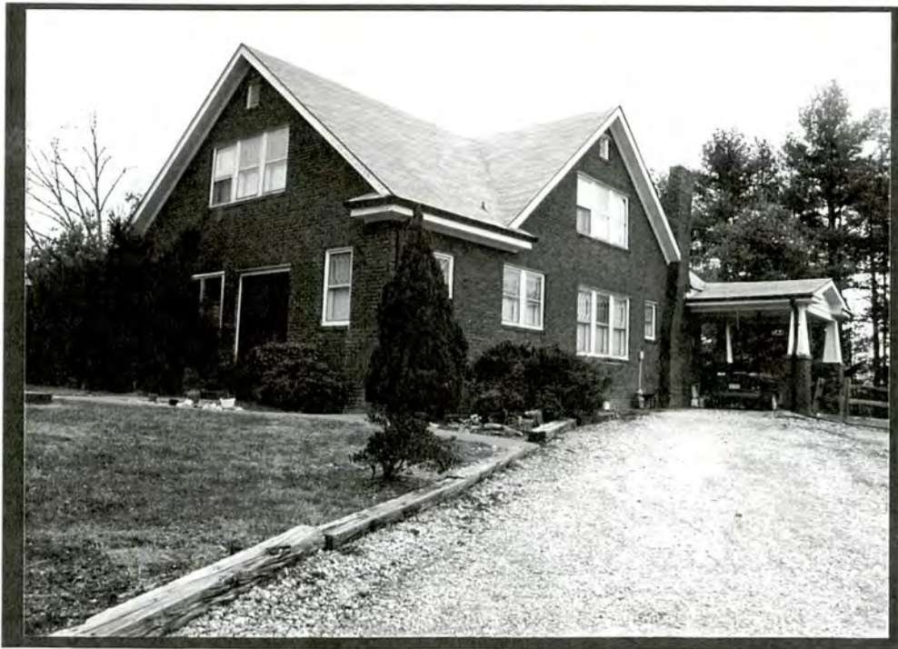
PLATE V.46 Bodenhammer House (#4), south side and west rear elevations
