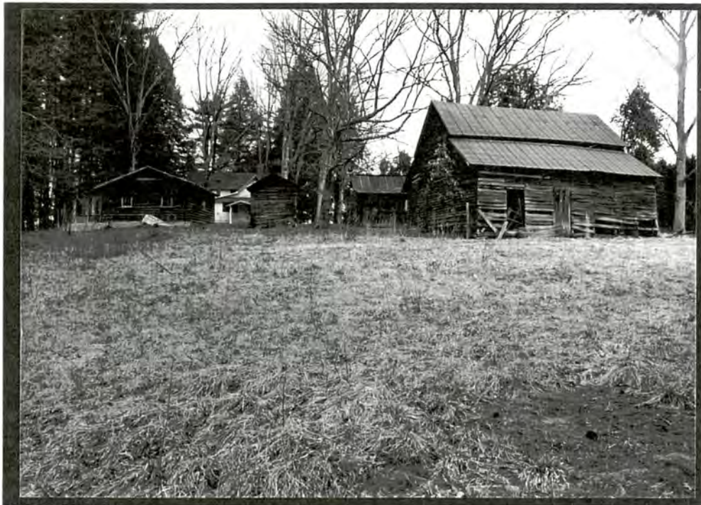
PLATE V.42 Liverett Farmhouse (#3), barn at right, crib at center right, shed at center left, garage at left, rear of main house in left background, facing northeast
