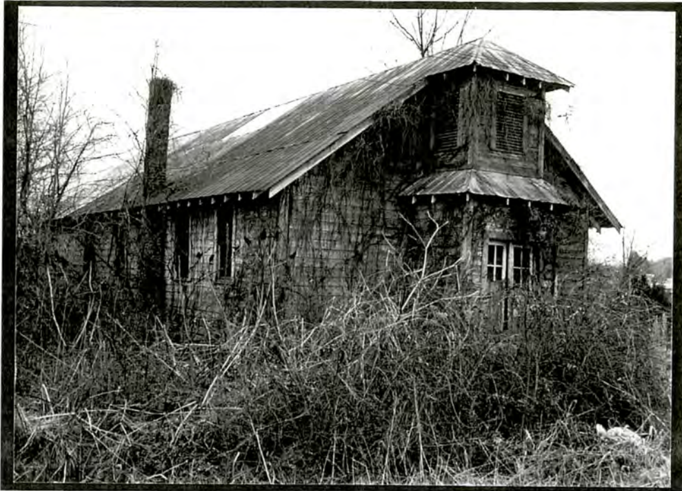
PLATE V.47 Former Naples Baptist Church (#5), east front and south side elevations
