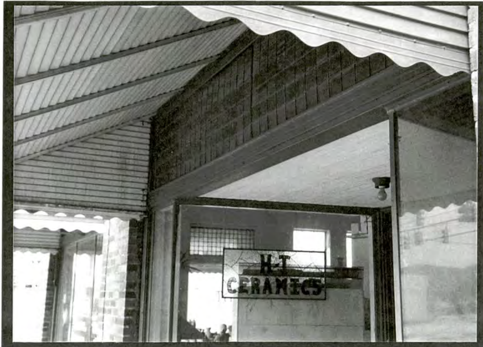
PLATE V.3 Former Youngblood General Store (#8), Luxfer glass transom, east front elevation
