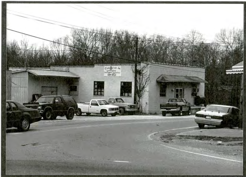
PLATE V.56 Fletcher Commercial District (#7), Circle F Electric Building [D], facing southwest
