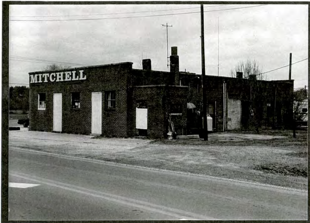
PLATE V.52 Mitchell Enterprises Building (#6), southeast side and northeast rear elevations
