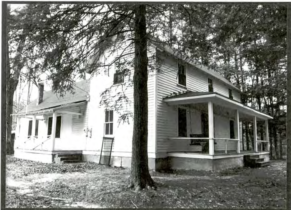
PLATE V.38 Liverett Farmhouse (#3), main house, northeast front and southeast side elevations
