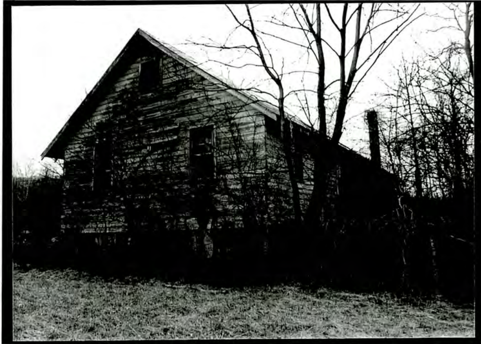
PLATE V.49 Former Naples Baptist Church (#5), west rear and south side elevations
