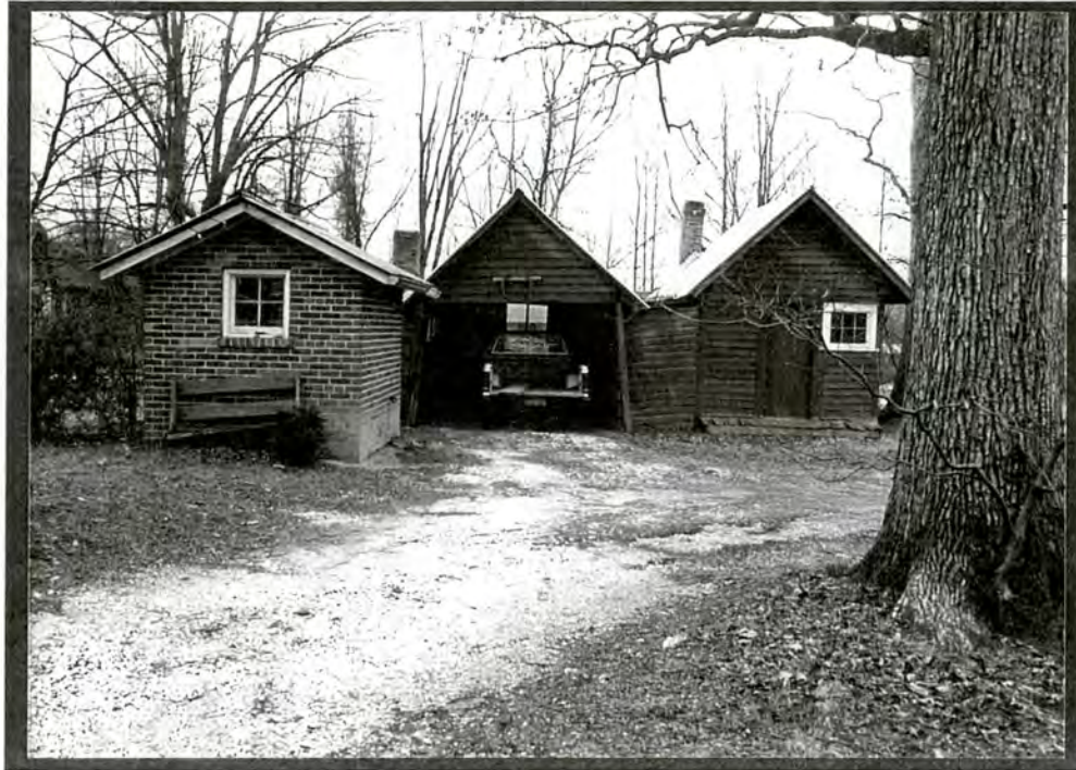
PLATE V.10 Cunningham-Poteat- Bagwell House (#9), outbuildings to south side, facing south
