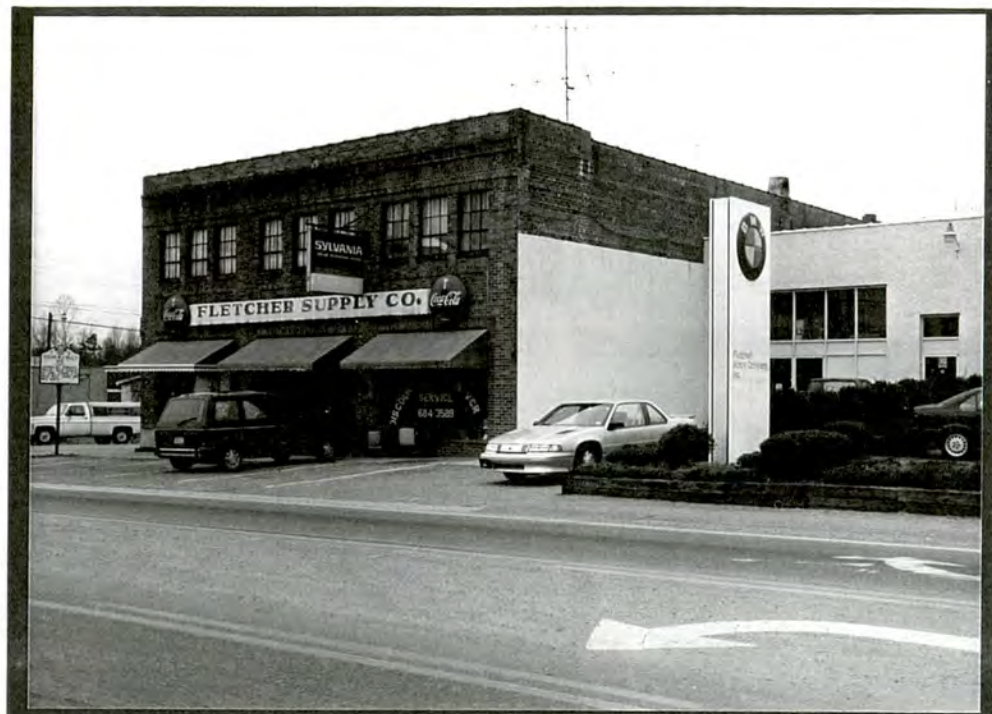
PLATE V.1 Former Youngblood General Store (#8), north side and east front elevations
