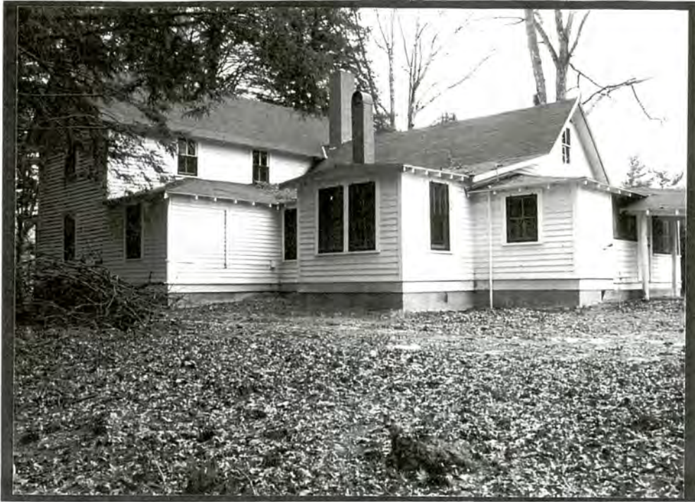
PLATE V.39 Liverett Farmhouse (#3), main house, southwest rear and northwest side elevations
