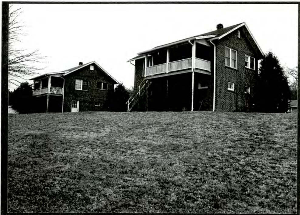
PLATE V.66 House and Duplexes (#10), duplexes B and C, south rear and east side elevations
