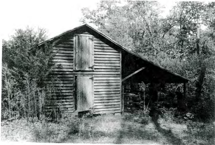
Lindley Nursery, Horse Stable (No. 89), Looking Northeast.
