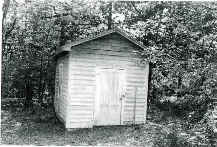
The Hill, Pump House (No. 53), Looking East.
