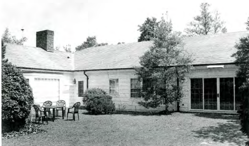
The Hill, Bird Song (No. 57), Rear (Southwest) Elevation and Terrace, Looking Northwest
