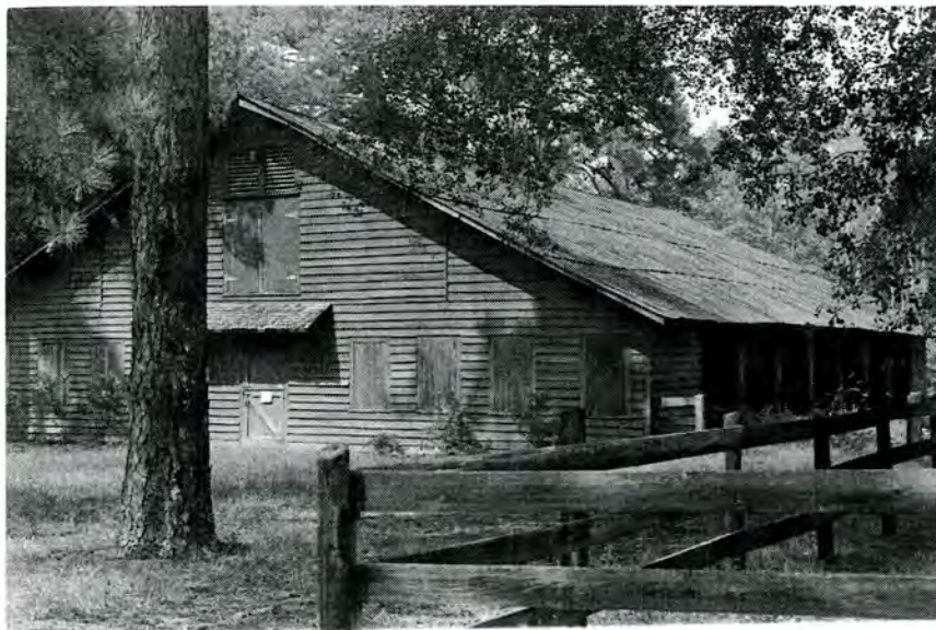
Entrance Compound, Polo Barn (No. 18), Front (Southwest) and Side (Southeast) Elevations, Looking Northeast.
