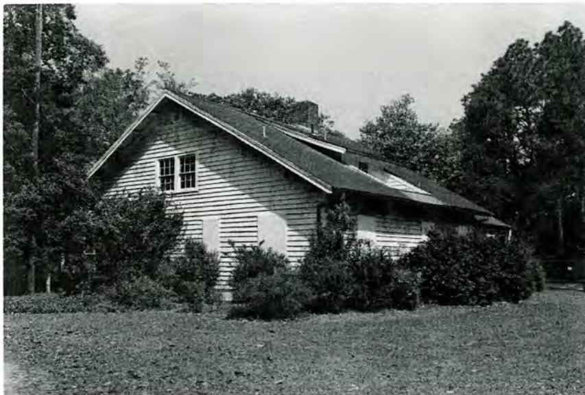
The Hill, Harriman Cottage (No. 46), Side (South) and Rear Elevations, Looking North.
