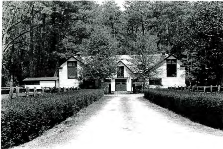
Entrance Compound, Riding Stable (No. 15), Stable and Entrance Drive, Looking Northeast.
