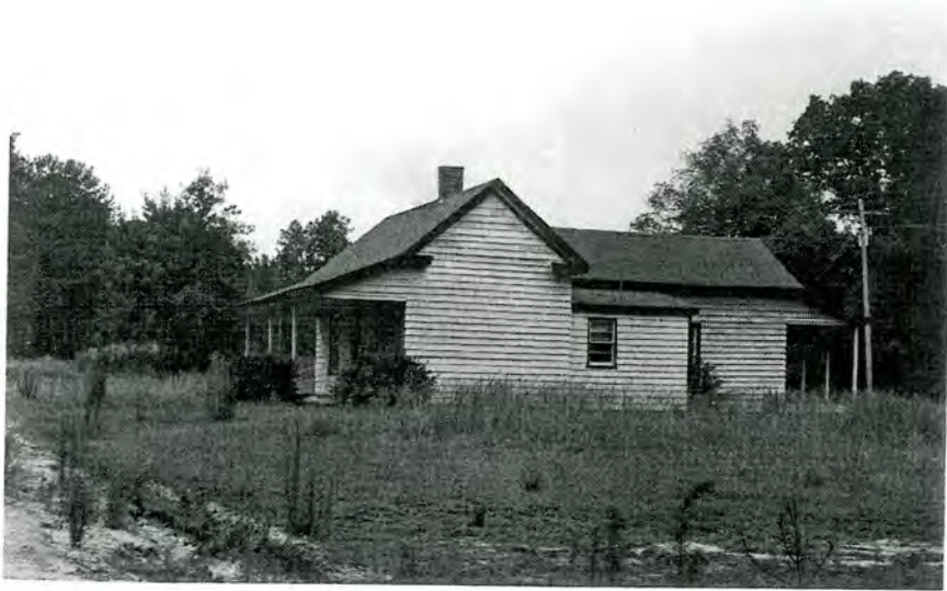
Lindley Nursery, Nursery Worker's House No. 4 (No. 85), Looking South.
