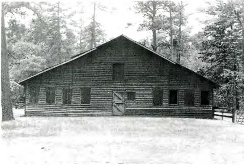
Plate 18. Polo Barn, Located within the Entrance Compound, Looking East.
