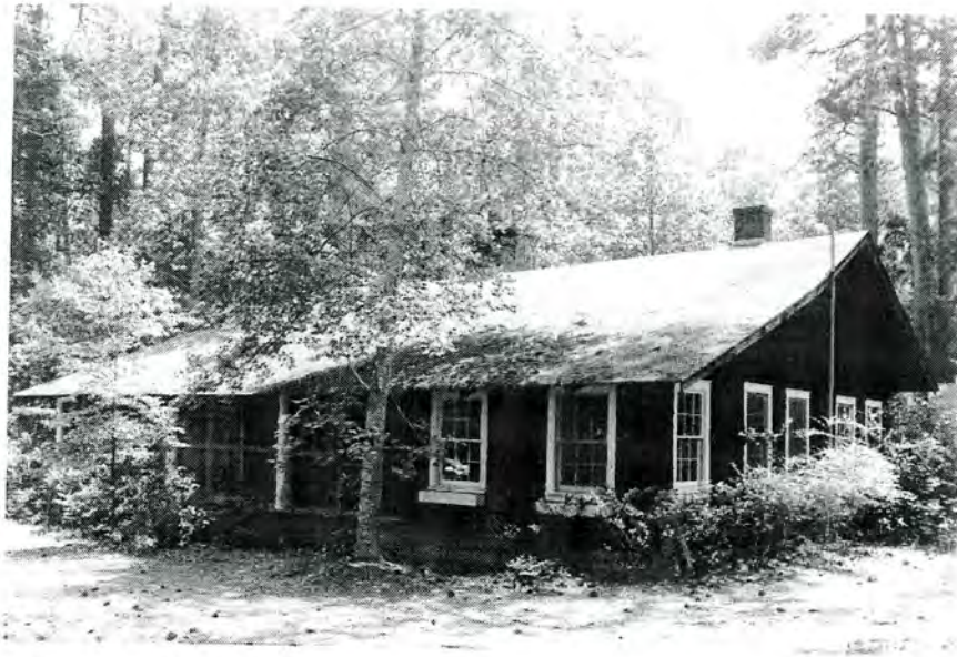
Shops Complex, Worker House No. 1 (No. 36), Facade and West Elevation, Looking South.
