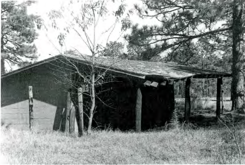
Pasture Stall (No. 64), Looking Northeast.
