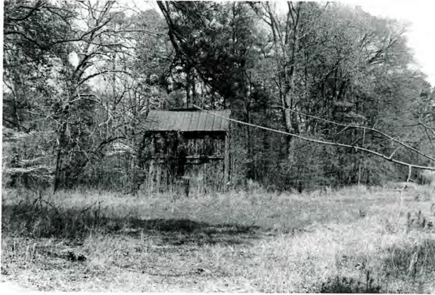
Dan Cameron Tenant Farm, Tobacco Barn (No. 106), Looking North.
