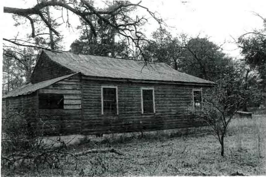
Townsend Tenant Farm, House No. 2 (No. 118), Facade (North Elevation), Looking Southeast.
