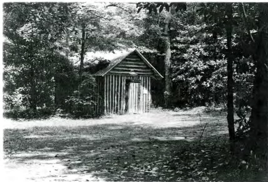
Entrance Compound, Pump House (No. 14), Looking East.
