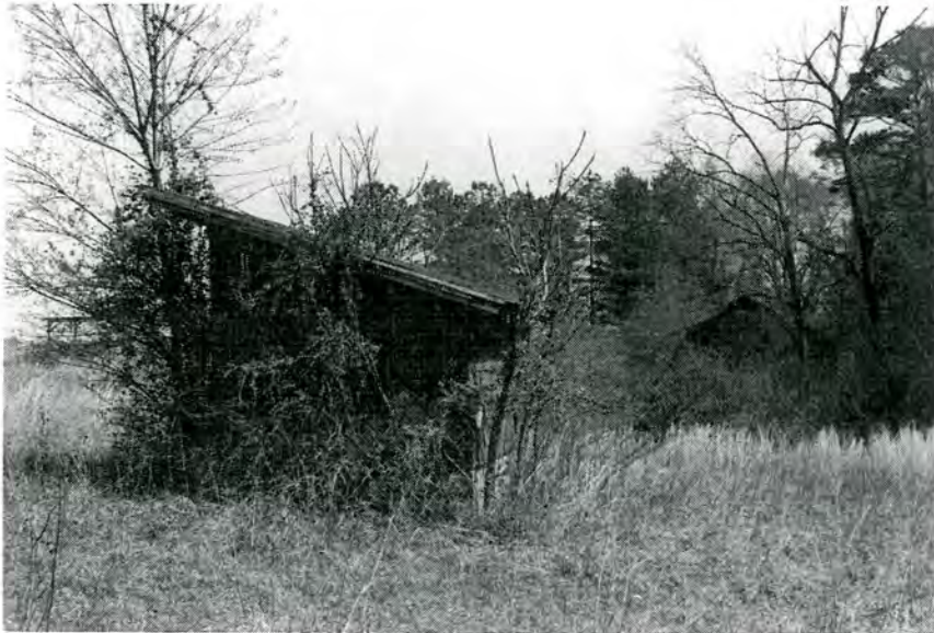
Clyde Williams Tenant Farm, Pump House (No. 100), Looking West.
