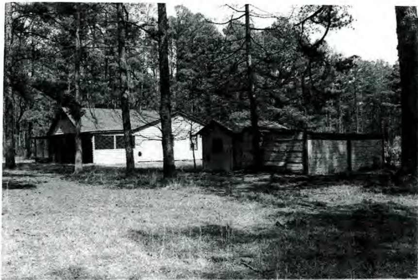
Townsend Tenant Farm, House No. 1 (No. 116) and Shed (No. 117), Looking Northeast.
