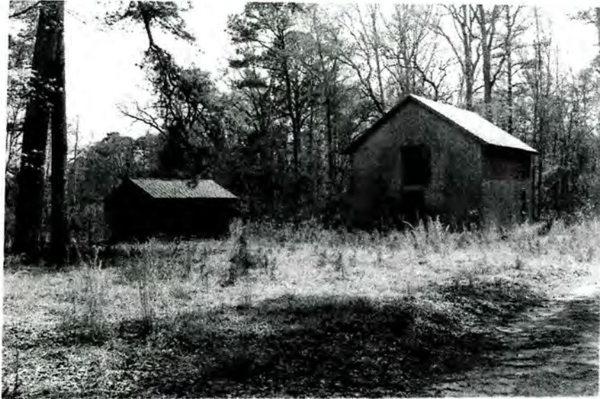
Townsend Tenant Farm, Pack House (No. 119) and Garage (No. 120), Looking Southeast.
