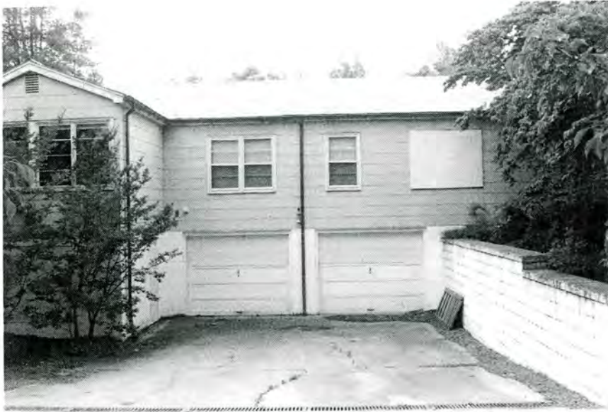
The Hill, Cherokee (No. 49), East Elevation and Basement Garage, Looking West.
