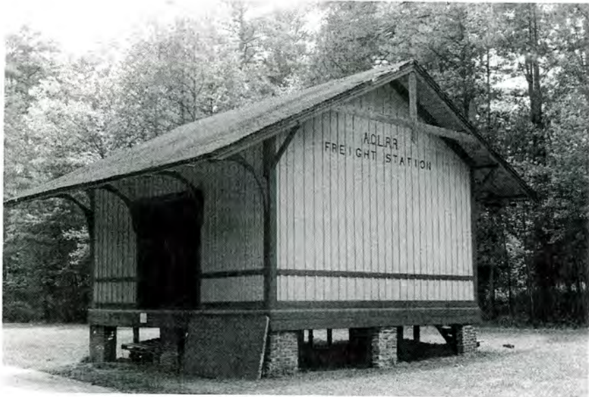
Entrance Compound, Freight Depot (No. 21), North and West Elevations, Looking Southeast.
