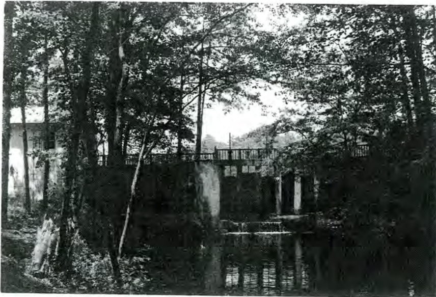
Overhills Lake, Dam and Gates (No. 22), Looking North along Muddy Creek.
