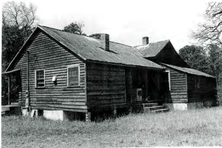
Townsend Tenant Farm, House No. 2 (No. 118), Rear Ell, Looking Northwest.
