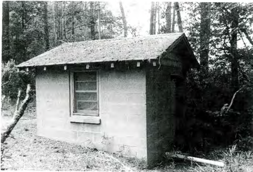
Overhills Lake, Pump House (No. 24), Looking North.
