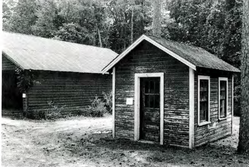
Shops Complex, Oil House (No. 30), Looking South (Shop Garage No. 1 in Background).
