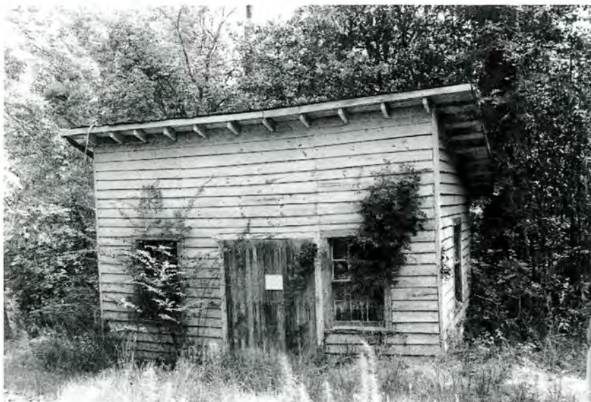
The Hill, Laundry (No. 45), Facade, Looking West.
