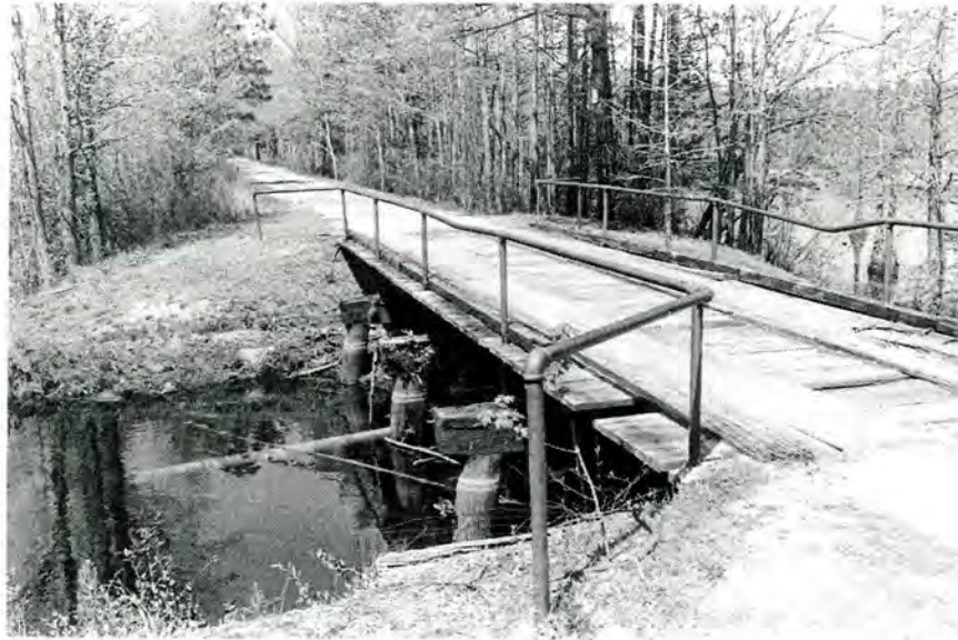
Overhills Lake, Railroad Bridge (No. 27), Looking Northeast Towards Overhills Lake.
