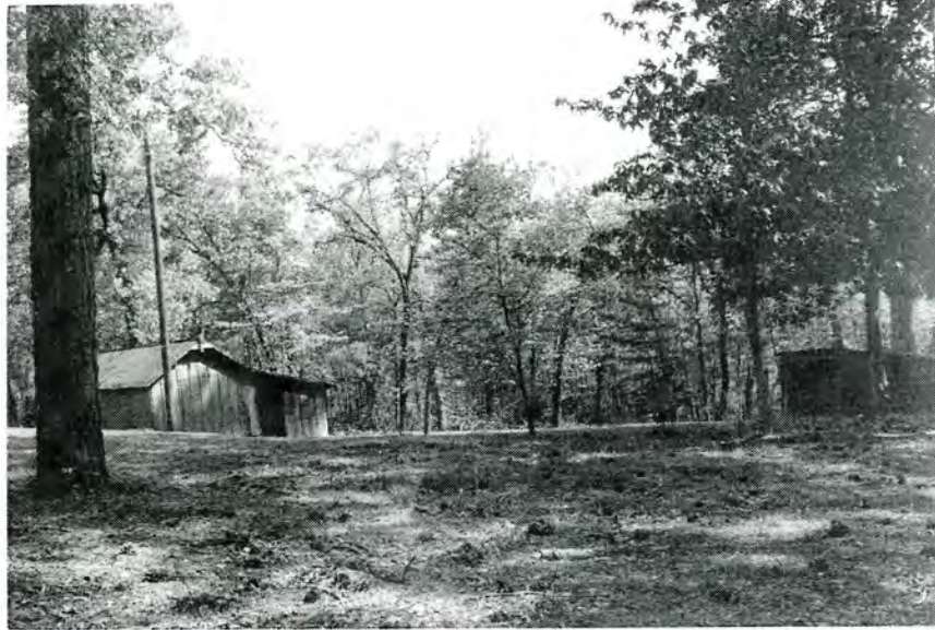
Hunt Stable Complex, Hunt Stable Residence No. 2, Garage (No. 7) and Hunt Stable Residence No. 2, Shed (No. 8), Looking East.
