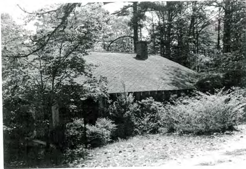
The Hill, White Servants' Quarters (No. 43), House and Setting, Looking Southeast.
