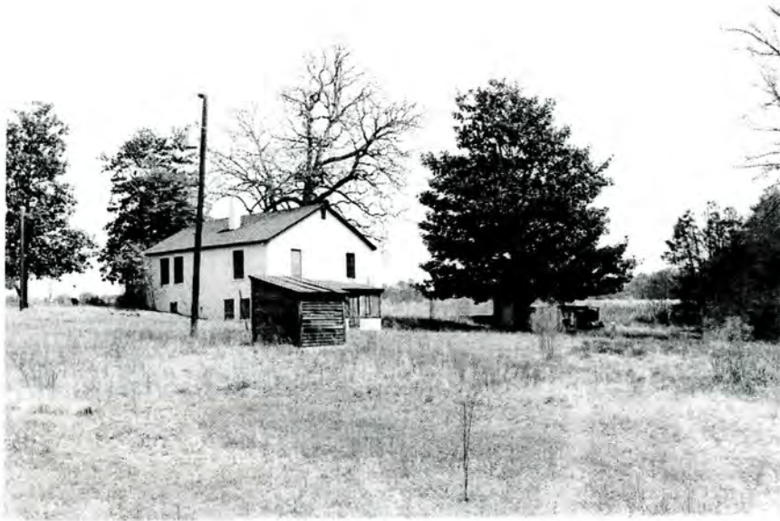
Dan Cameron Tenant Farm, Pump House No. 2 (No. 109), Looking Northeast.
