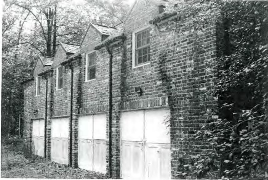
The Hill, Croatan Garage (No. 55), Front (East) Elevation, Looking South.
