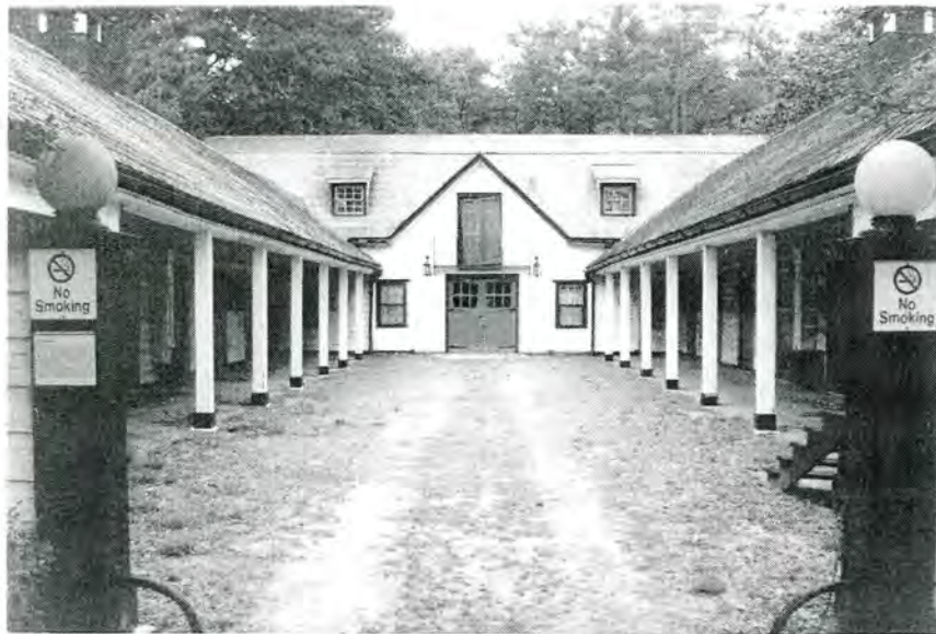
Entrance Compound, Riding Stable (No. 15), Looking Through Entrance into Forecourt.
