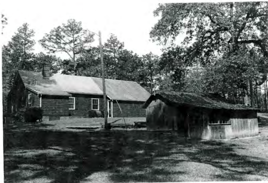
Hunt Stable Complex, Hunt Stable Residence No. 2 (No. 6) and Hunt Stable Residence No. 2, Garage (No. 7), Buildings and Setting, Looking Northwest.
