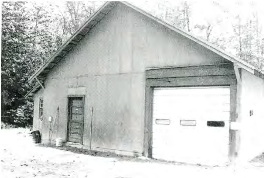
Shops Complex, Shop (No. 31), Looking West.
