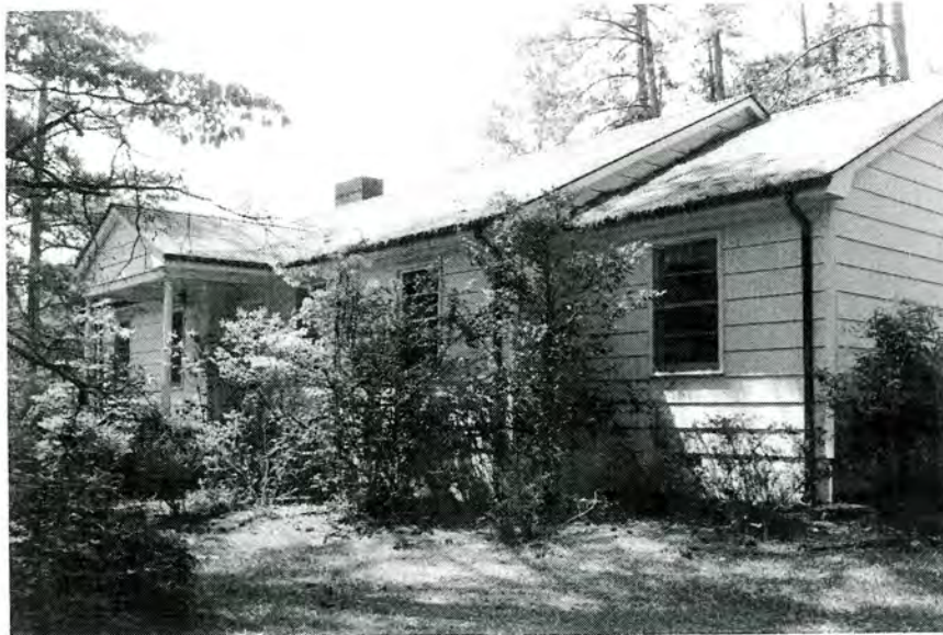
The Hill, Estate Manager's Residence (No. 50), House Facade (Northeast Elevation), Looking Southwest
