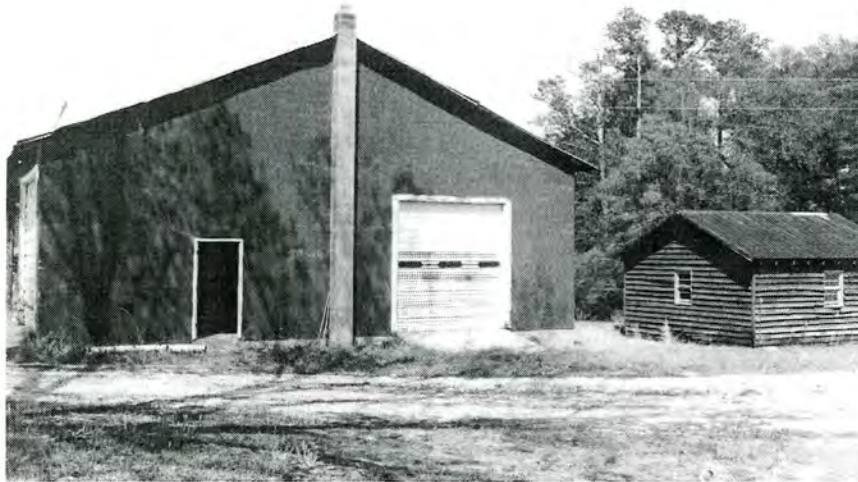
Lindley Nursery, Equipment Shed (No. 79) and Oil House (No. 80), Looking Northeast.
