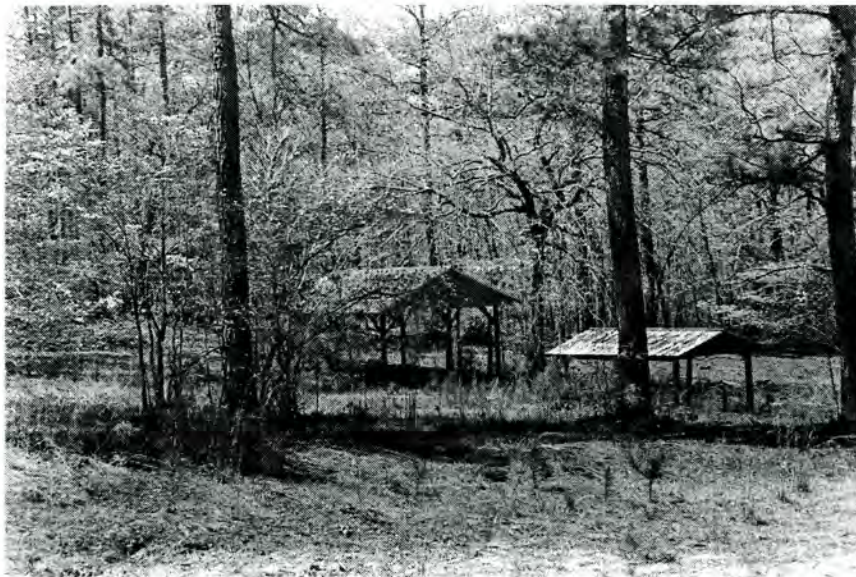
Shops Complex, Sheds (Nos. 140-141), Looking Northwest.
