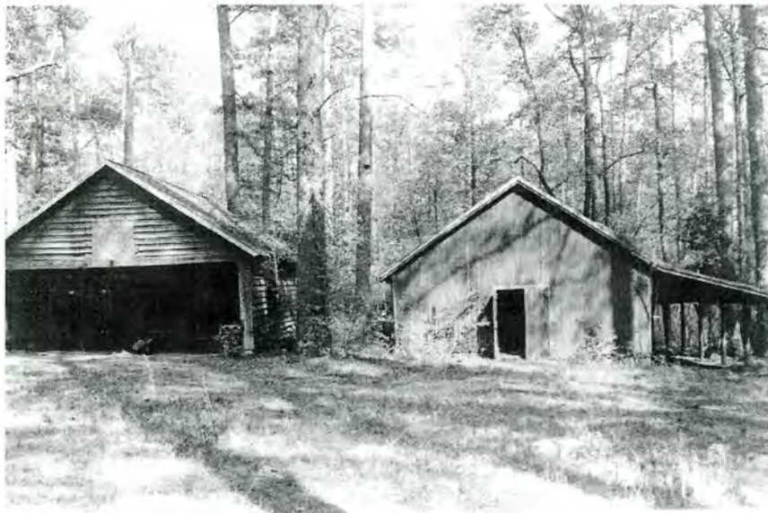
Lindley Nursery, Granary/Shop (No. 72) and Hay Barn (No. 73), Looking Southeast.
