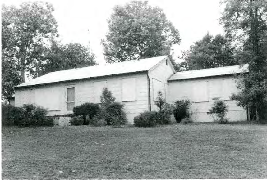
The Hill, Sycamore (No. 48), House and Setting, South Elevation, Looking North.
