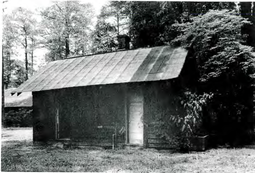
Shops Complex, Servant's House (No. 38), Facade, Looking North.
