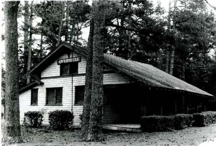
Entrance Compound, Overhills Passenger Station (No. 12), Front and Side (Northwest) Elevations, Looking Southeast.
