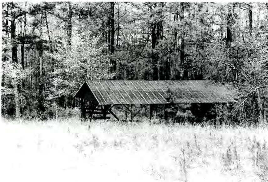
Shops Complex, Shed (No. 138), Looking North.
