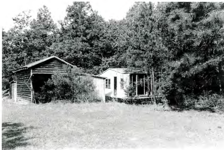
Hairfield Tenant Farm, Garage (No. 129) and Metal Storage Shed (No. 131), Looking West.
