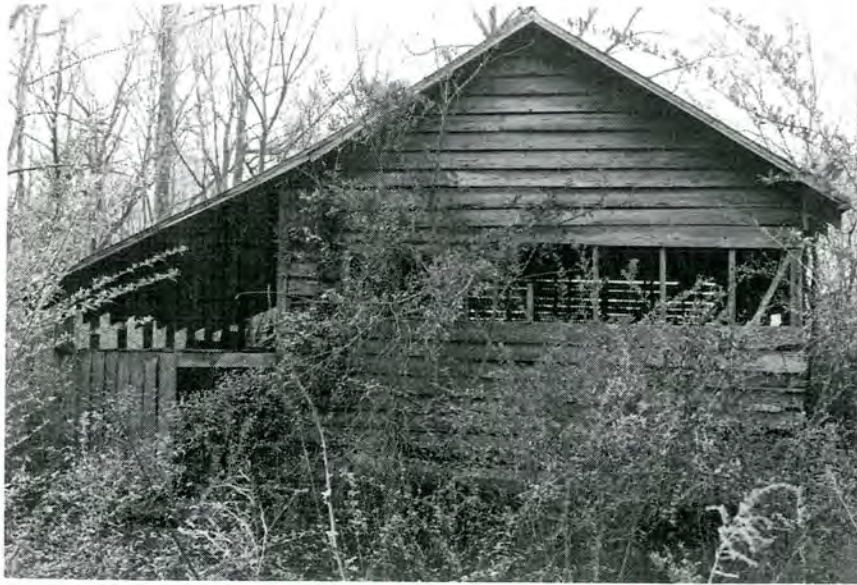
Clyde Williams Tenant Farm, Crib (No. 99), Looking South.
