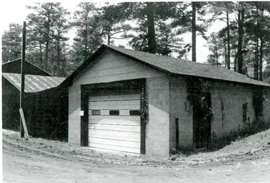
Shops Complex, Woodworking Shop (No. 35), Looking Northwest (Shop Garage No. 2 on Left).
