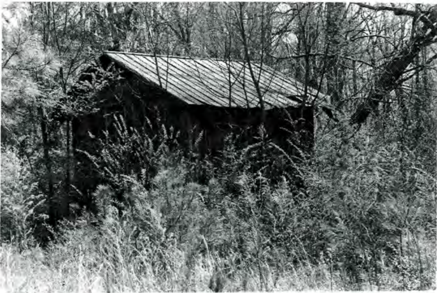
Clyde Williams Tenant Farm, Tobacco Barn No. 2 (No. 98), Looking Southeast.
