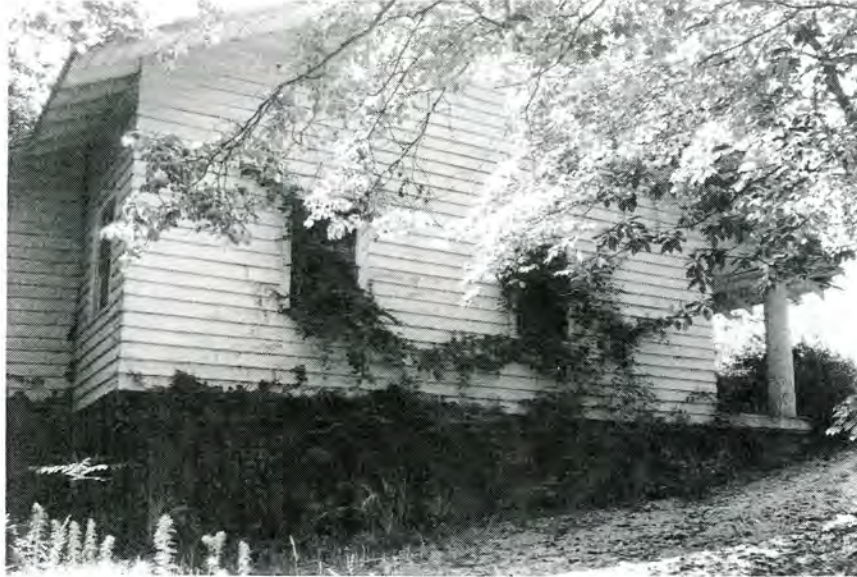
The Hill, Black Servants' Quarters (No. 44), Side (North) Elevation, Looking South.
