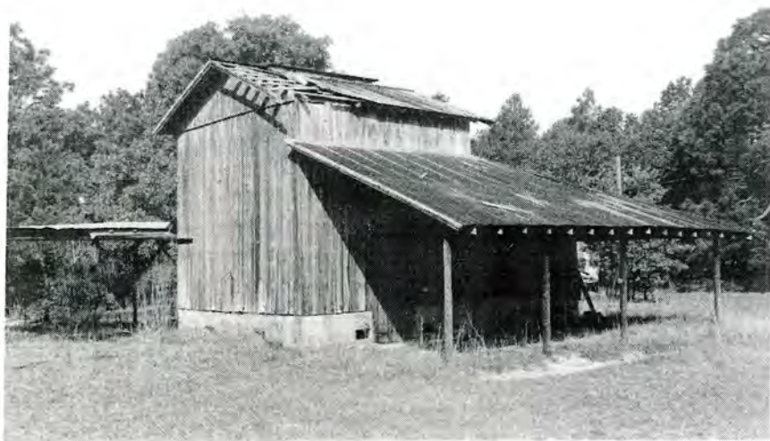
Hairfield Tenant Farm, Tobacco Barn (No. 127) and Sheds (No. 130), Looking Northwest.
