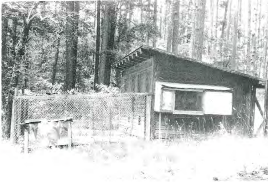
Shops Complex. Worker House No.2. Chicken House (No. 42), Looking South.
