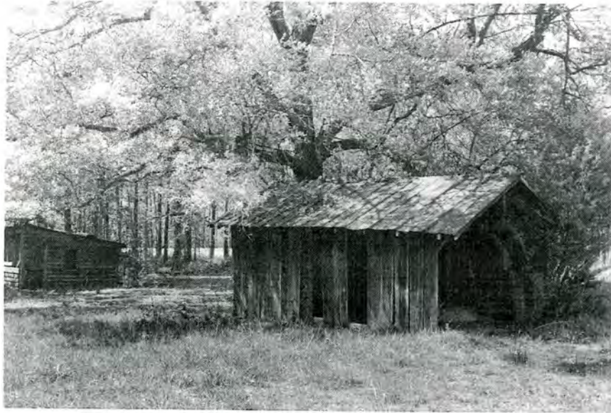
Lindley Nursery, Nursery Worker's House No. 4, Garage (No. 86) and Chicken House (No. 87), Looking Southwest.
