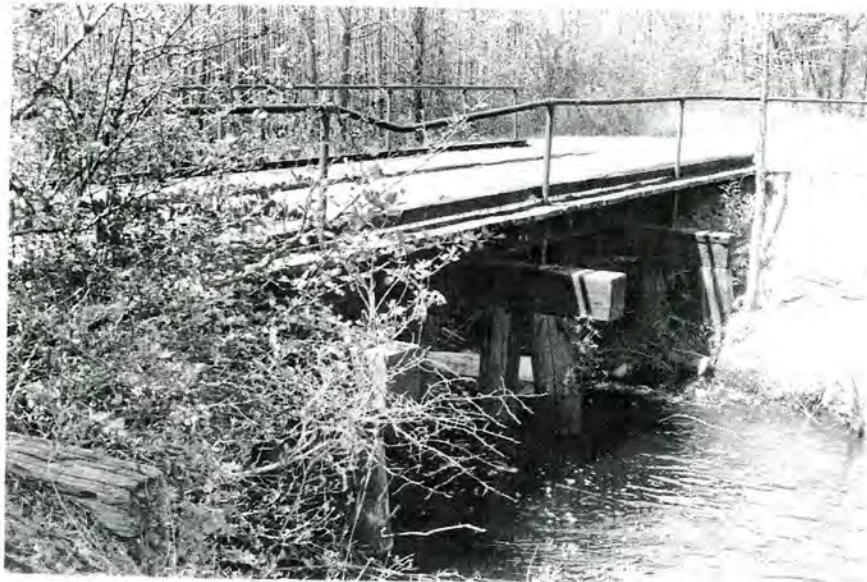
Overhills Lake, Railroad Bridge (No. 27), East Profile, Looking Northwest.
