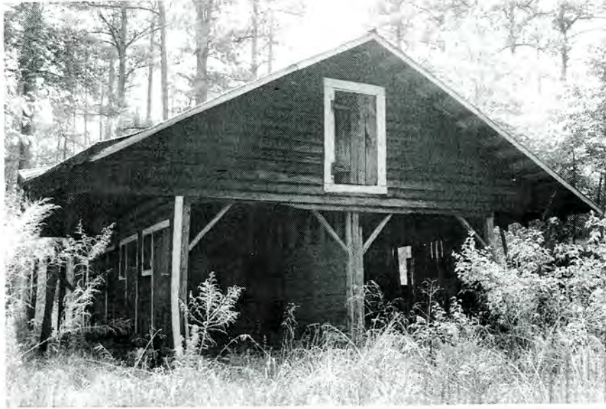
Shops Complex, Mule Barn (No. 40), Looking North.
