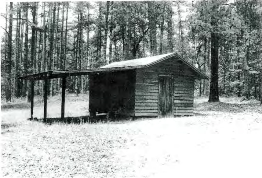
Shops Complex, Worker House No. 2, Wood Shed (No. 41), Looking Northwest.
