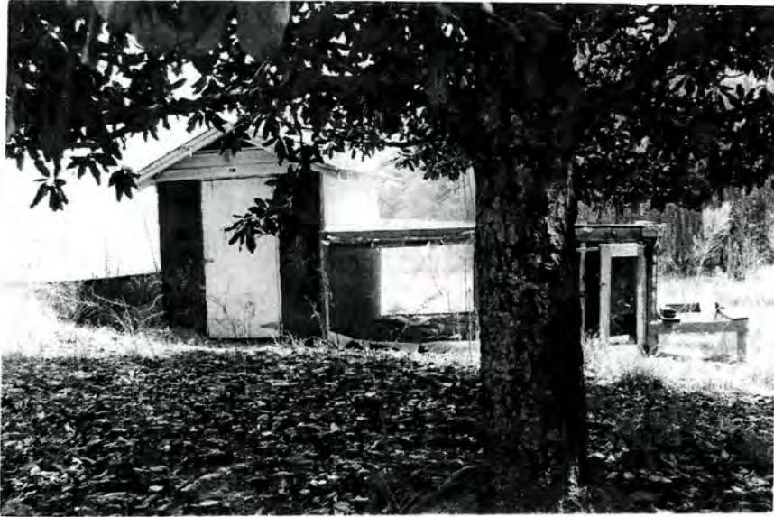
Dan Cameron Tenant Farm, Pump House No. 1 (No. 108), Looking East.
