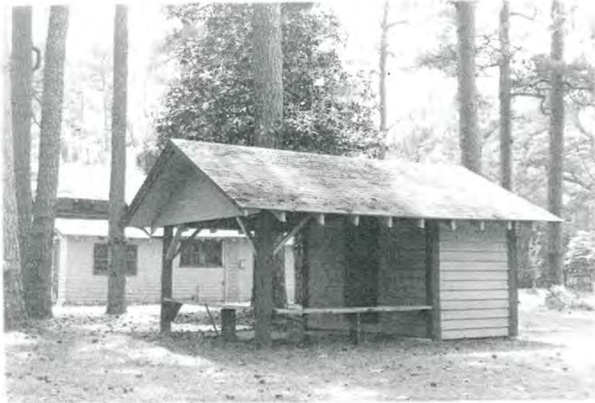
Entrance Compound, Storage Building (No. 13). Looking Northwest (Passenger Station in Background).
