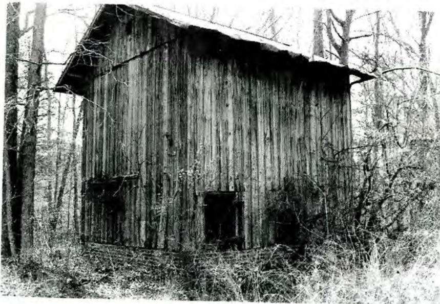
Townsend Tenant Farm, Tobacco Barn No. 2 (No. 124), Looking Southeast.
