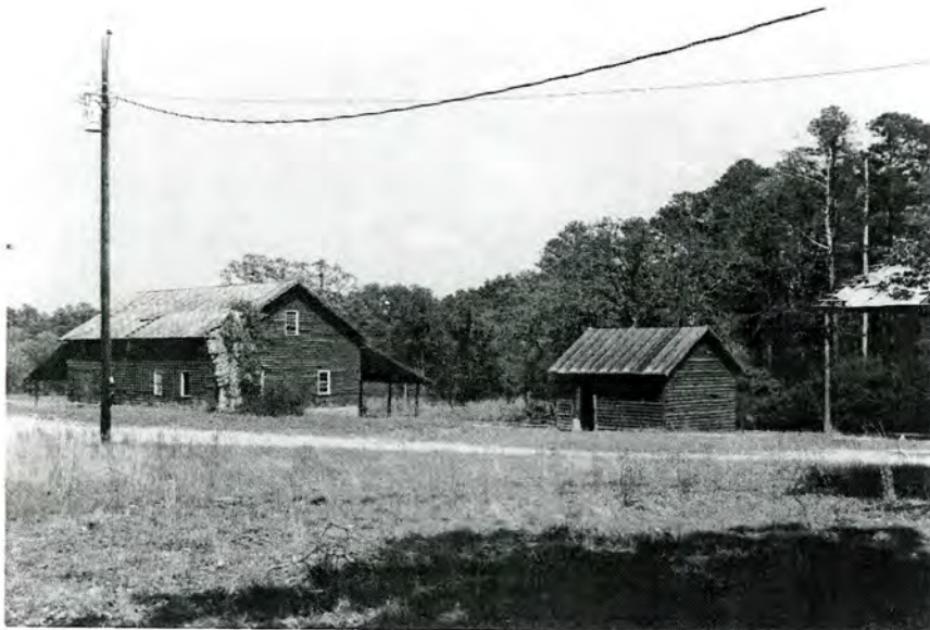
Lindley Nursery, Feed Barn (No. 81) and Garage/Stable (No. 84), Looking East.
