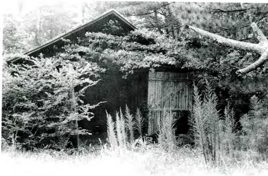
Lindley Nursery, Equipment Shed (No. 76), Looking West from Jumping Run Creek.
