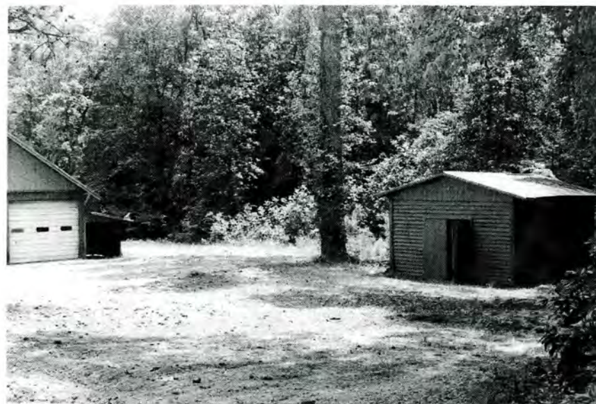
Shops Complex, Fuel Storage Shed (No. 29), Looking Southeast.
