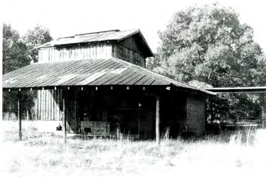
Hairfield Tenant Farm, Tobacco Barn (No. 127). Looking Southwest.
