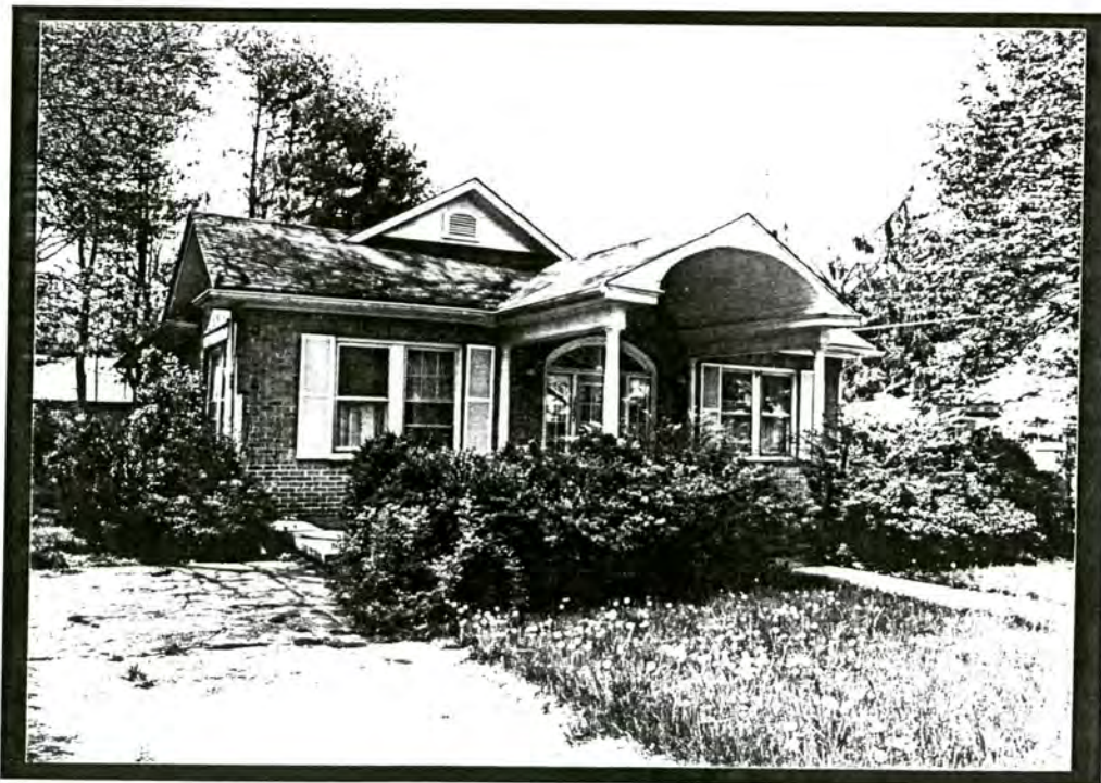
PLATE V.50 Druid Hills neighborhood northwest of APE, 1721 Haywood Road/NC 191
