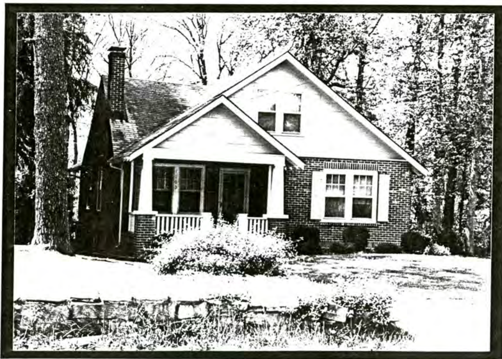
PLATE V.48 Druid Hills neighborhood northwest of APE, 1703 Haywood Road/NC 191
