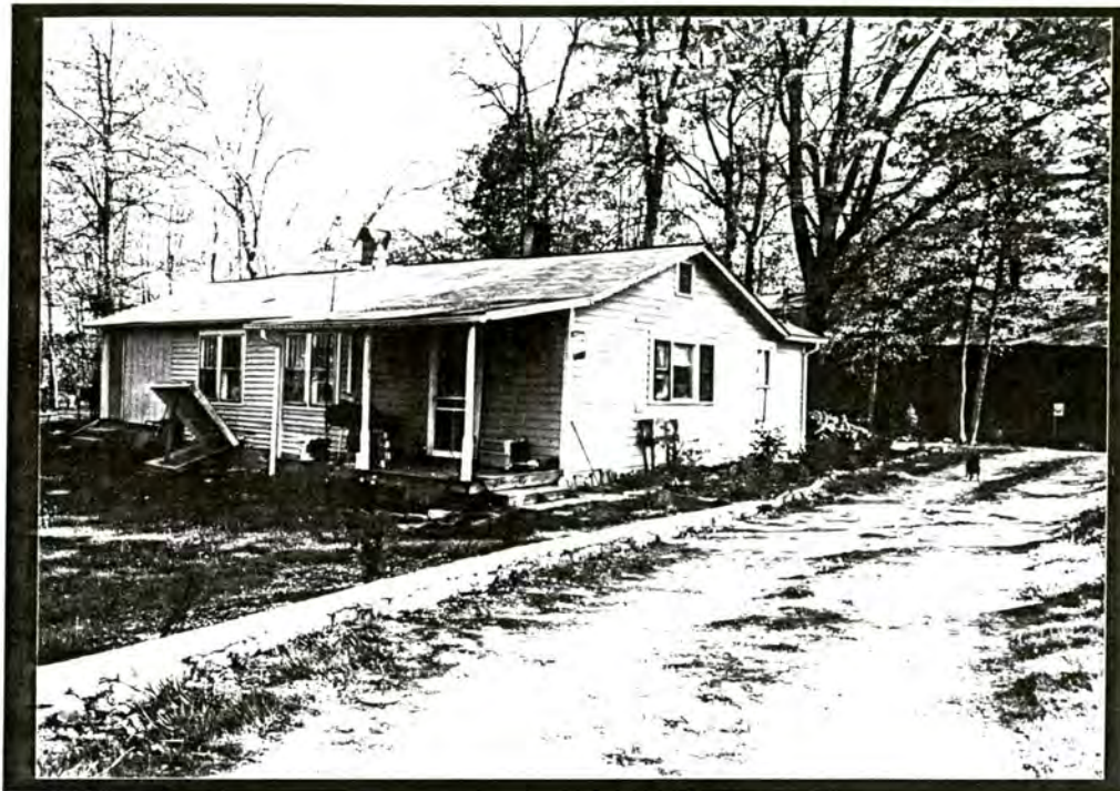
PLATE V.8 Sholtz-Cantrell Estate caretaker's house at left, equipment shed at right
