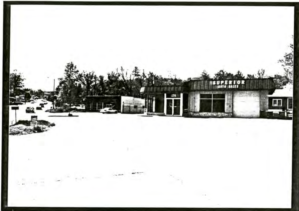
PLATE V.12 D r u i d H i l l s neighborhood, 1525 Asheville Highway/US 25 at right, 1521 Asheville Highway/US 25 at left center
