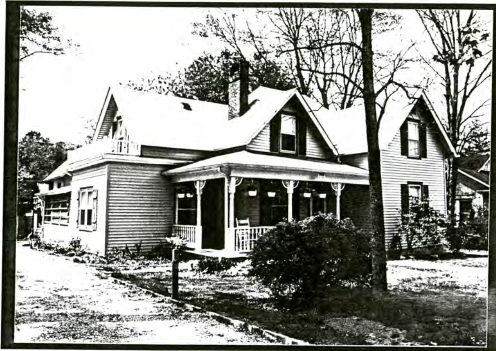
PLATE V.49 Druid Hills neighborhood northwest of APE, 1709 Haywood Road/NC 191
