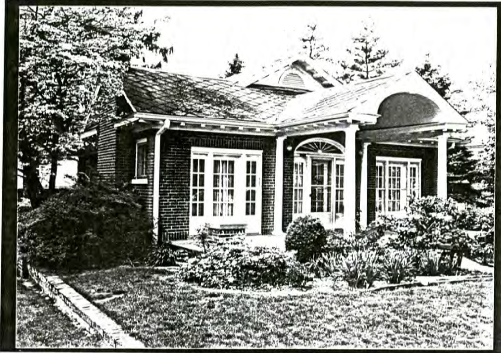
PLATE V.51 Druid Hills neighborhood northwest of APE, 1731 Haywood Road/NC 191
