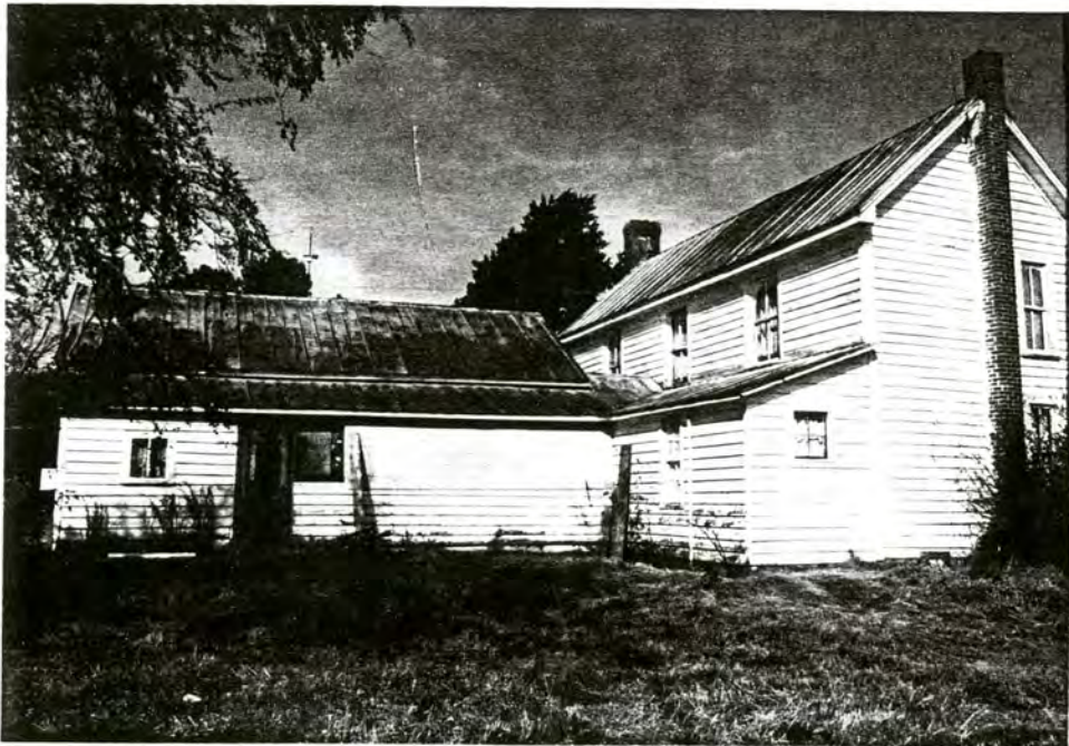
84. (B) Simmons Farm, S elevation, view to N
