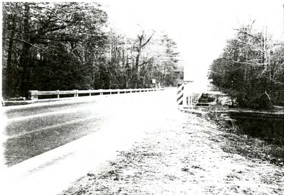
2. US 13/NC 42, just N of bridge over Ahoskie Creek in Ahoskie Swamp, view to SE
