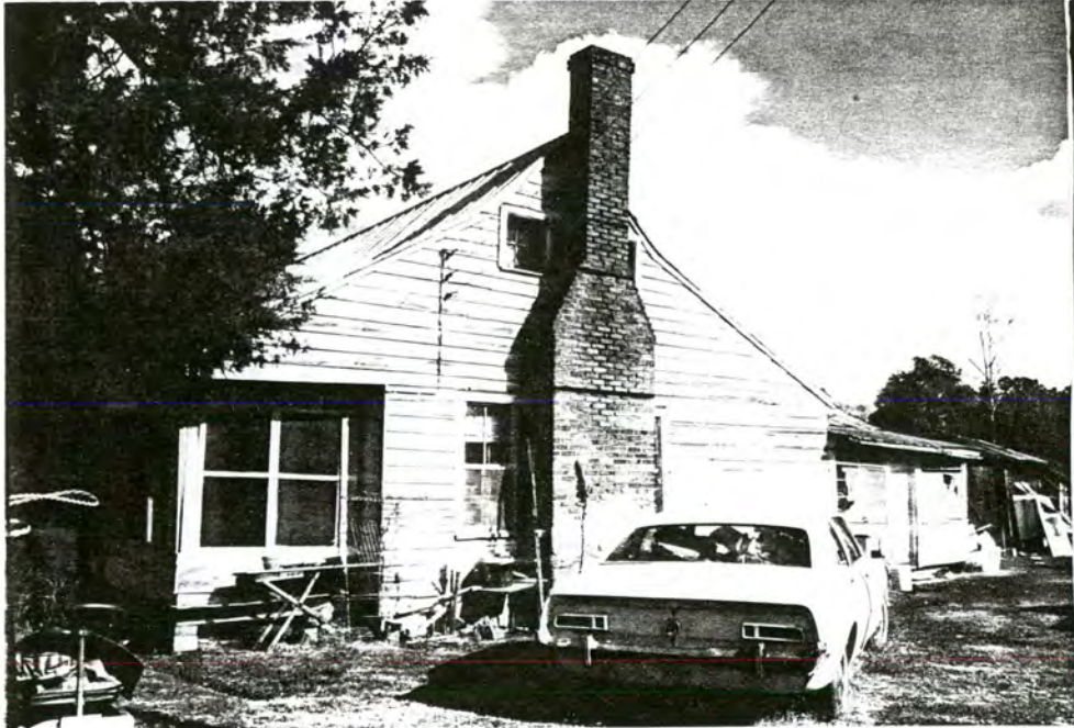
63. (A) House, S elevation, view to NE
