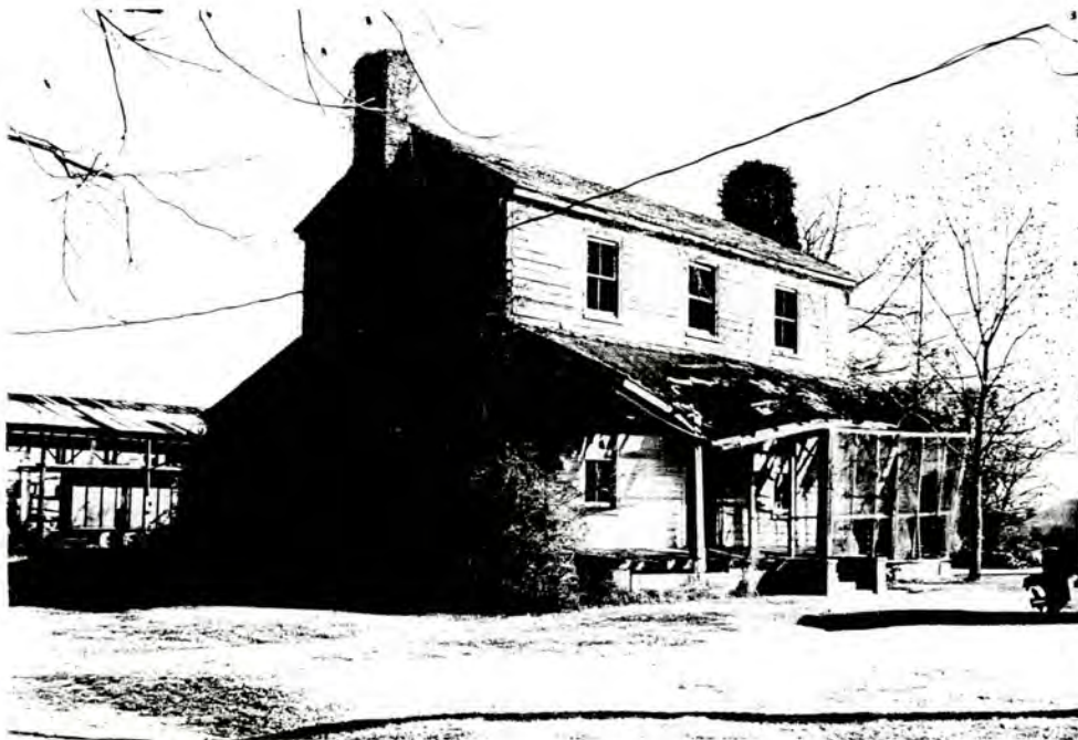
45. (A) Lawrence Askew House, overall view to NE
