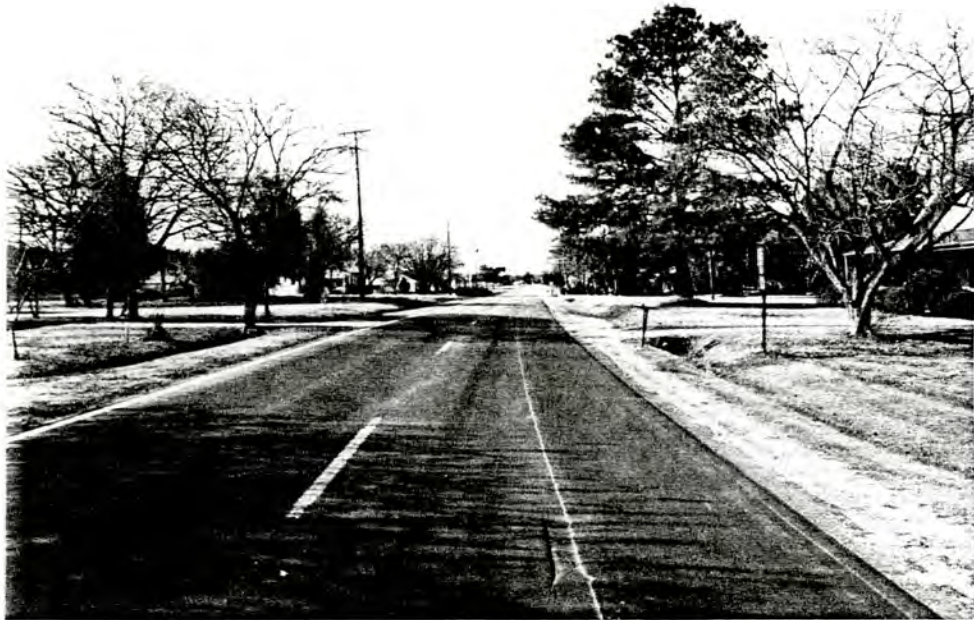
3. NC 561, 0.8 mi W of jct w/SR 1419, view to W
