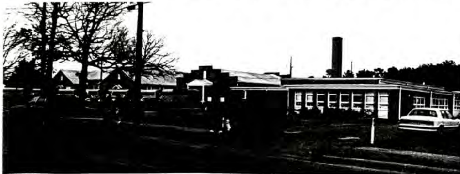
20. (A) Holloman Avenue Historic District, Robert L. Vann School, overall view to N
