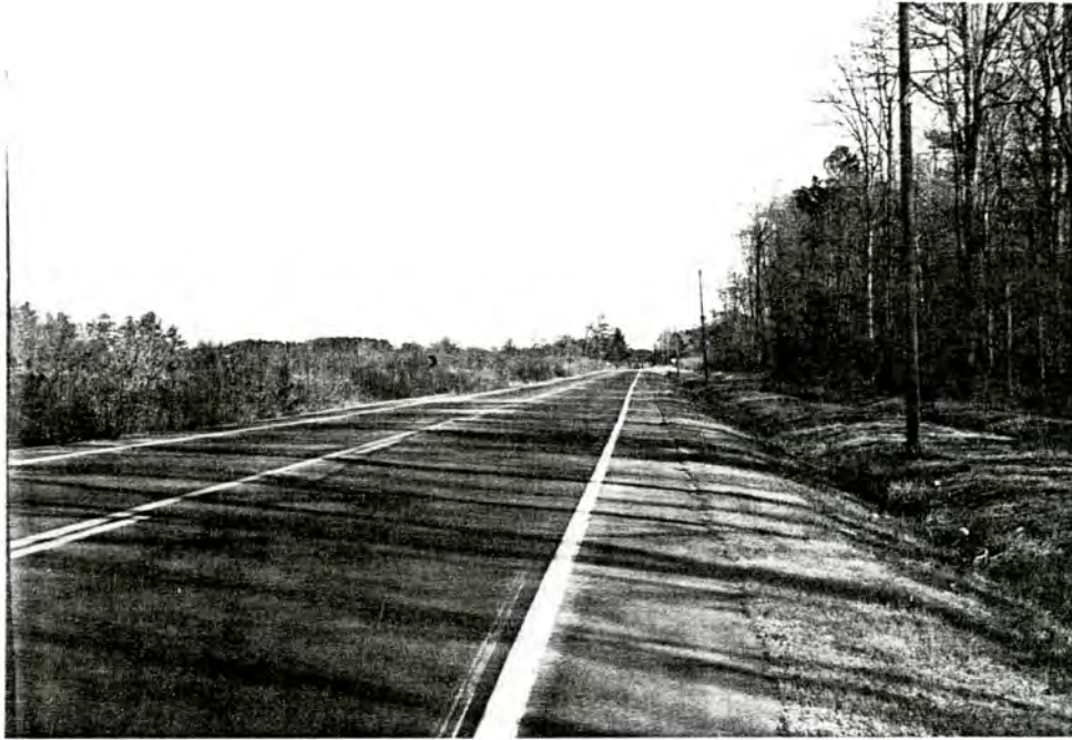
7. US 13, just N of jct w/SR 1132, view to NE
