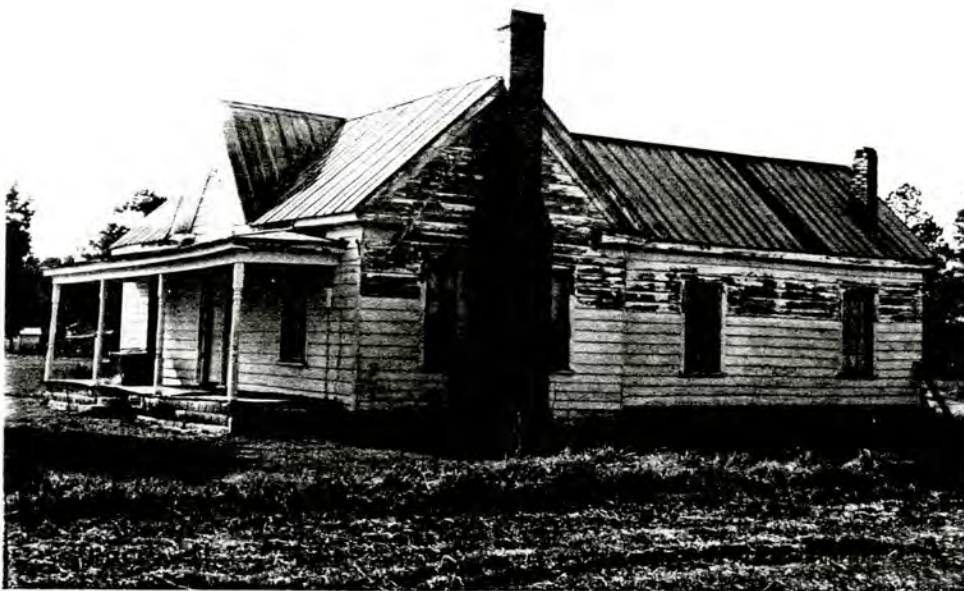
66. (B) House, N elevation, view to SW
