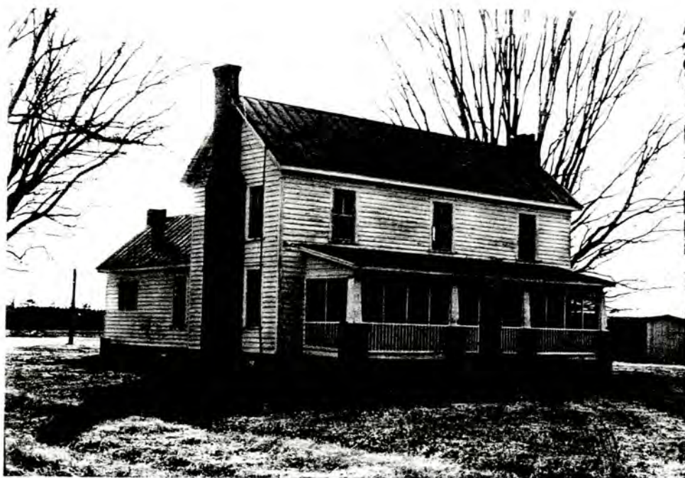
28. (B) William G. Livermon House and Outbuildings, overall view of house to SW
