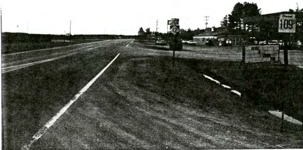
1. US 13, just S of jct w/NC 42, view to N
