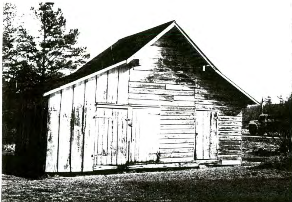
33. (C) Newsome-Hall House, smokehouse, view to NE
