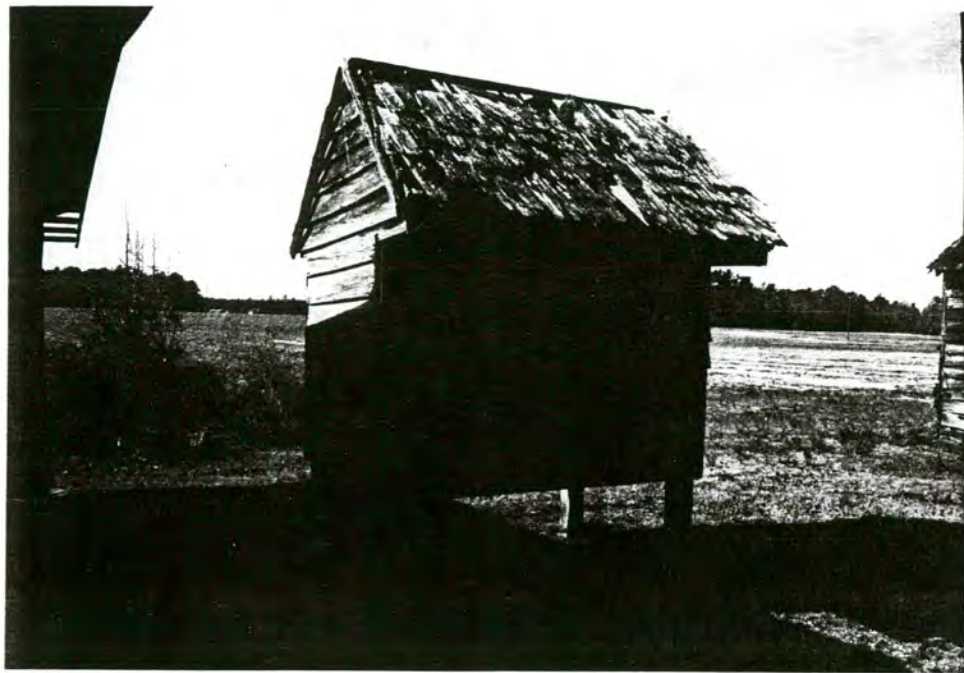
41. (D) William B. Weaver Farm, stilted dairy, view to W
