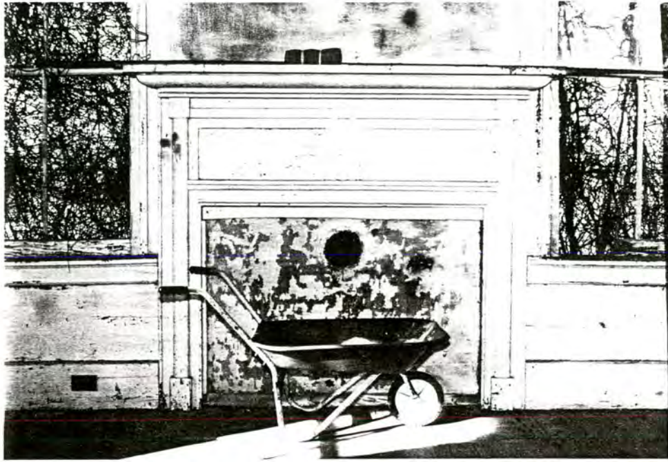
46. (B) Lawrence Askew House, parlor mantel, view to W
