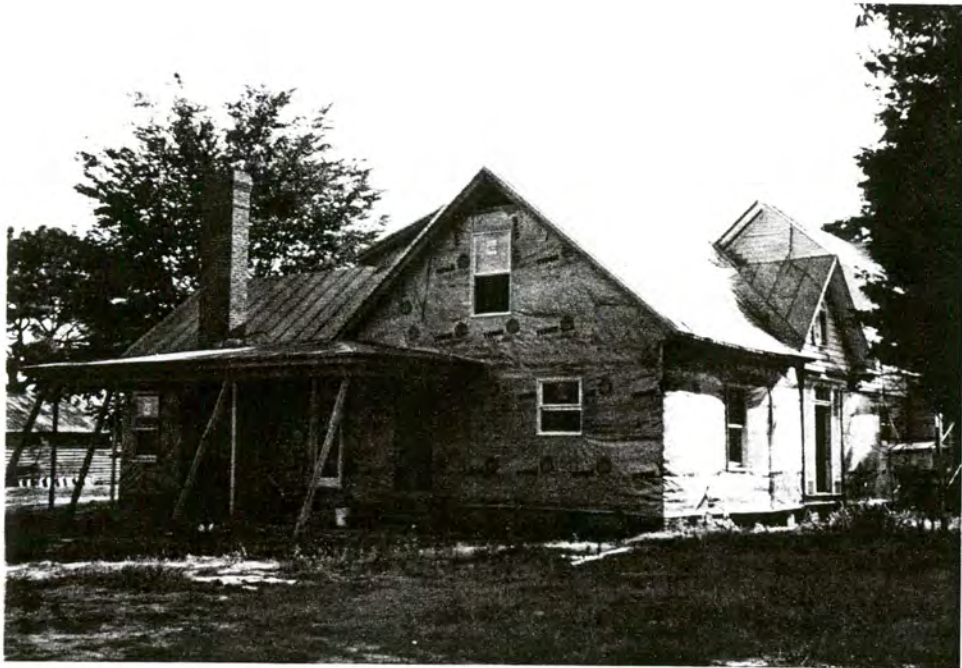
59. (B) James Lawrence Early House and Outbuildings, rear of house, view to southwest
