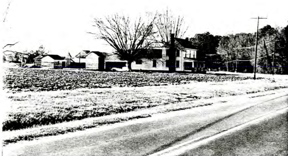
27. (A) William G. Livermon House and Outbuildings, overall view to SW
