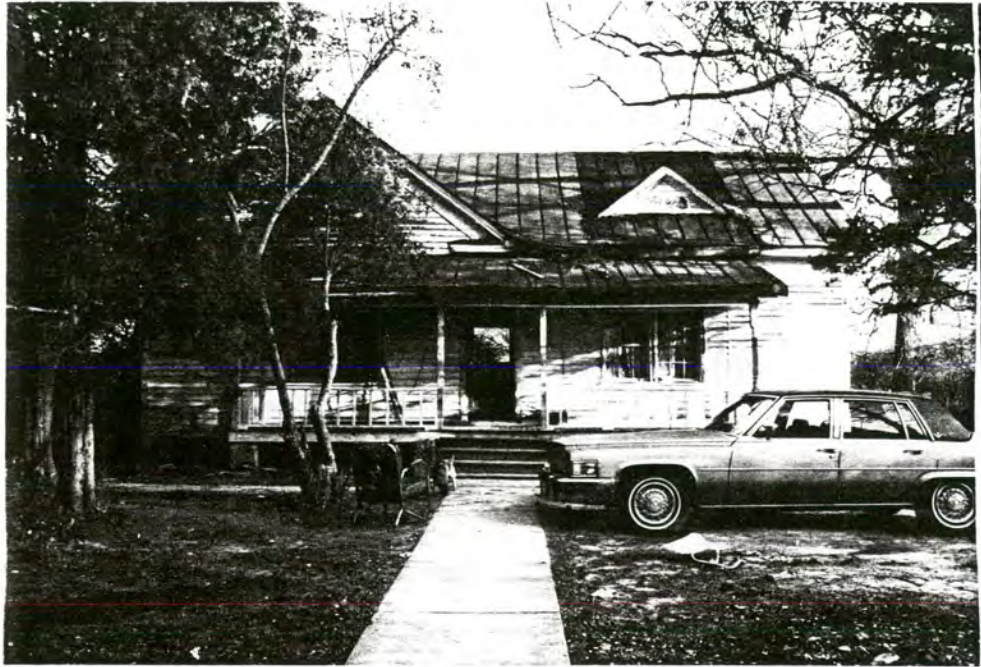
50. (A) Brantley's Grove School, facade, view to SE
