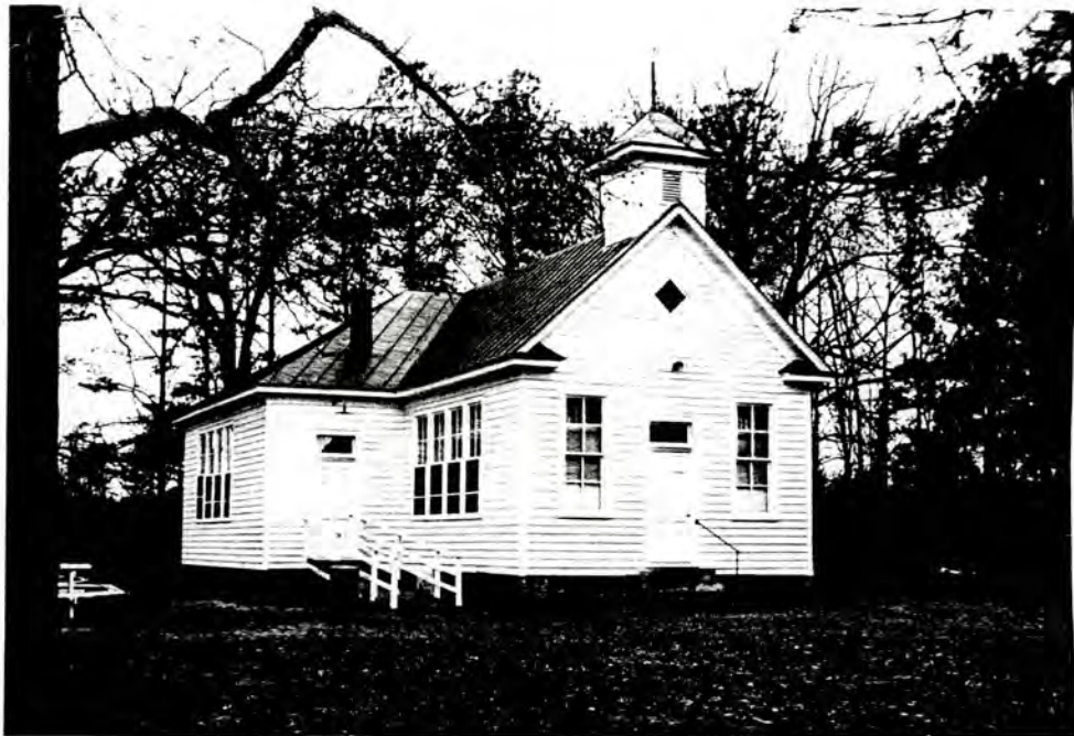
35. (A) Pleasant Plains School, overall view to NW
