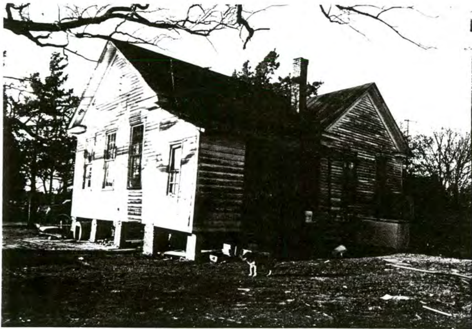
51. (B) Brantley's Grove School, rear, view to N
