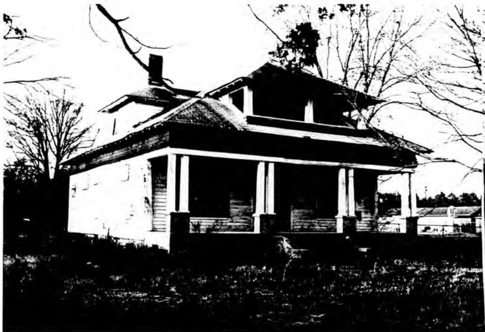
25. (A) Graham Holloman House, overall view to N
