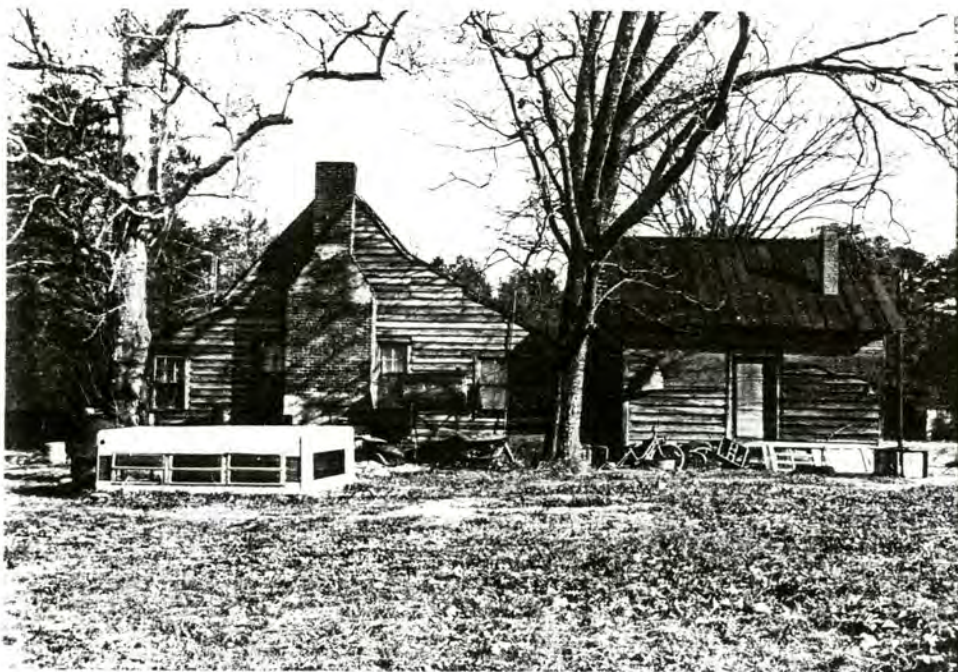
62. (B) Anthony Godwin House, S side, view to N
