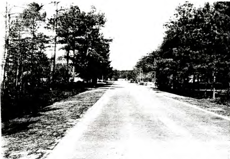
4. SR 1419, 1.5 mi N of jct w/NC 561, view to N
