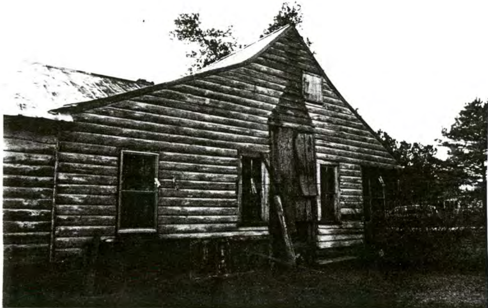
64. (B) House, N elevation, view to SW
