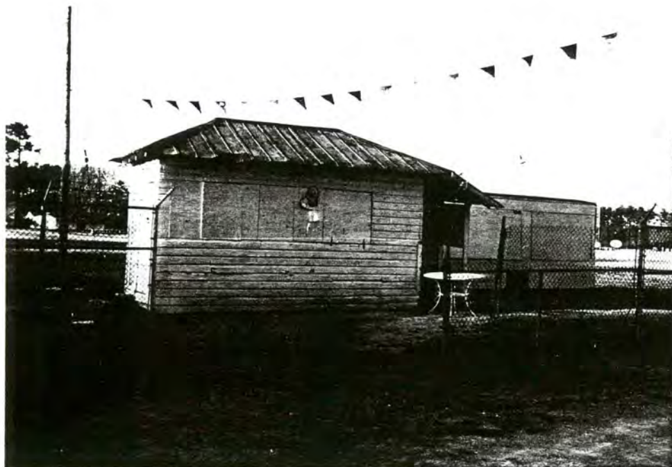
24. (E) Holloman Avenue Historic District, Atlantic District Fairground, ticket office, view to NW
