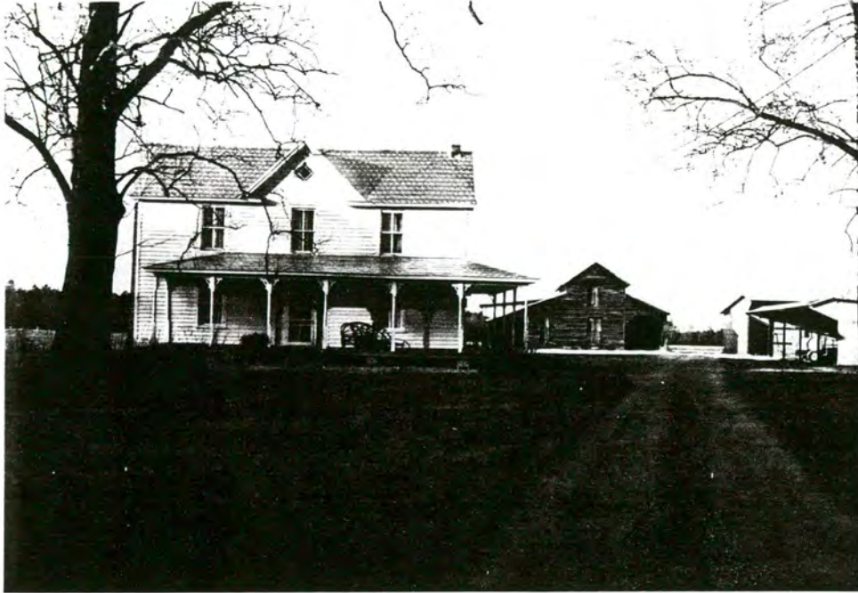
16. (A) Albert Hall Farm, overall view to N
