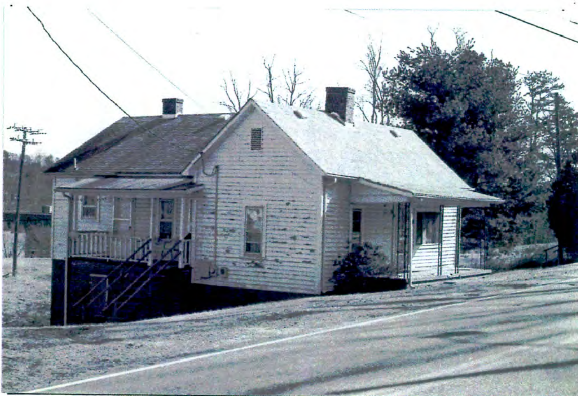
Illustration 15. Brookford Mills employee housing (typical), Brookford village.
