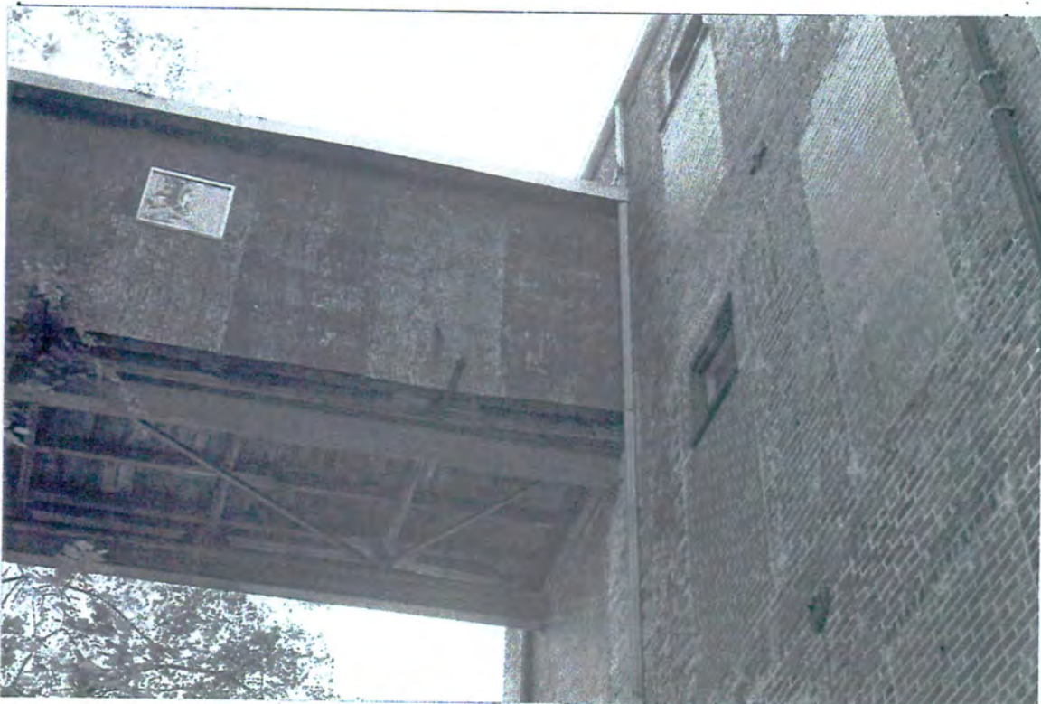
Illustration 29. Former Brookford Mills, fifth level loading ramp.
