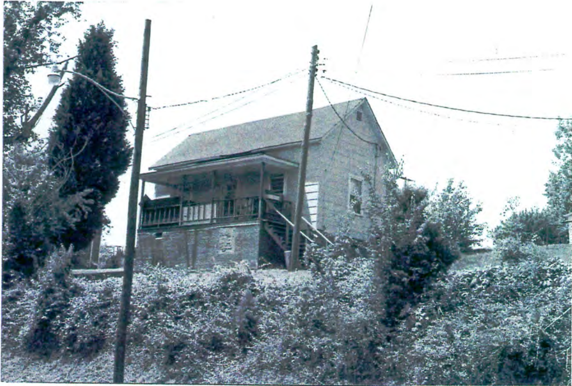
Illustration 16. Brookford Mills employee housing (typical), Brookford village.
