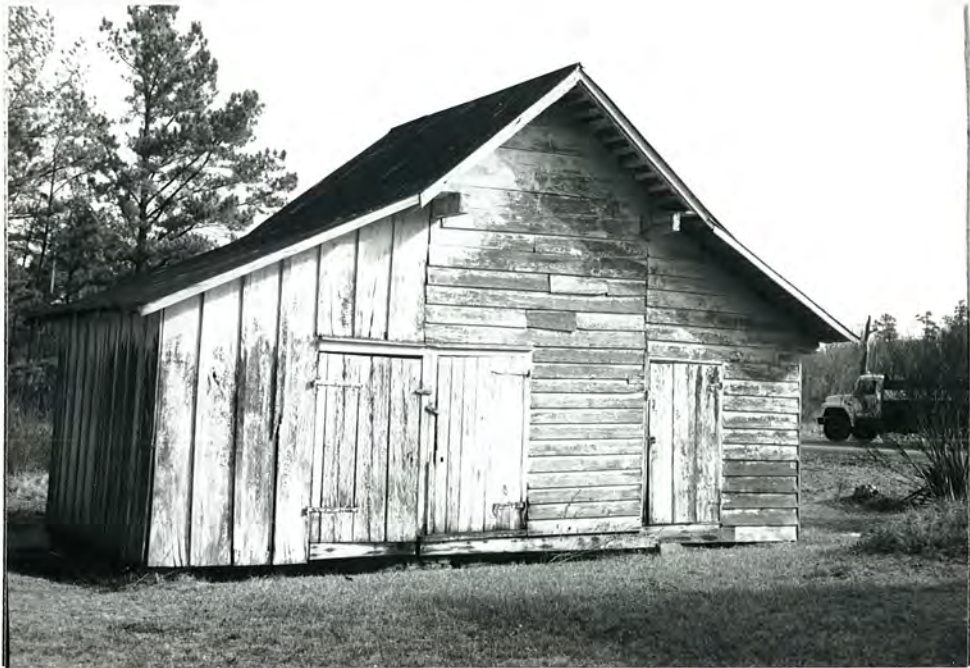
38. (C) Newsome-Hall House, smokehouse, view to NE
