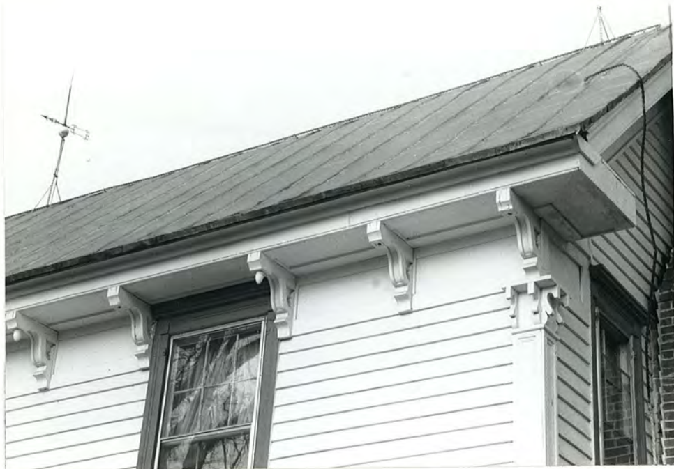
19. (B) Thomas Eley House, cornice, view to E
