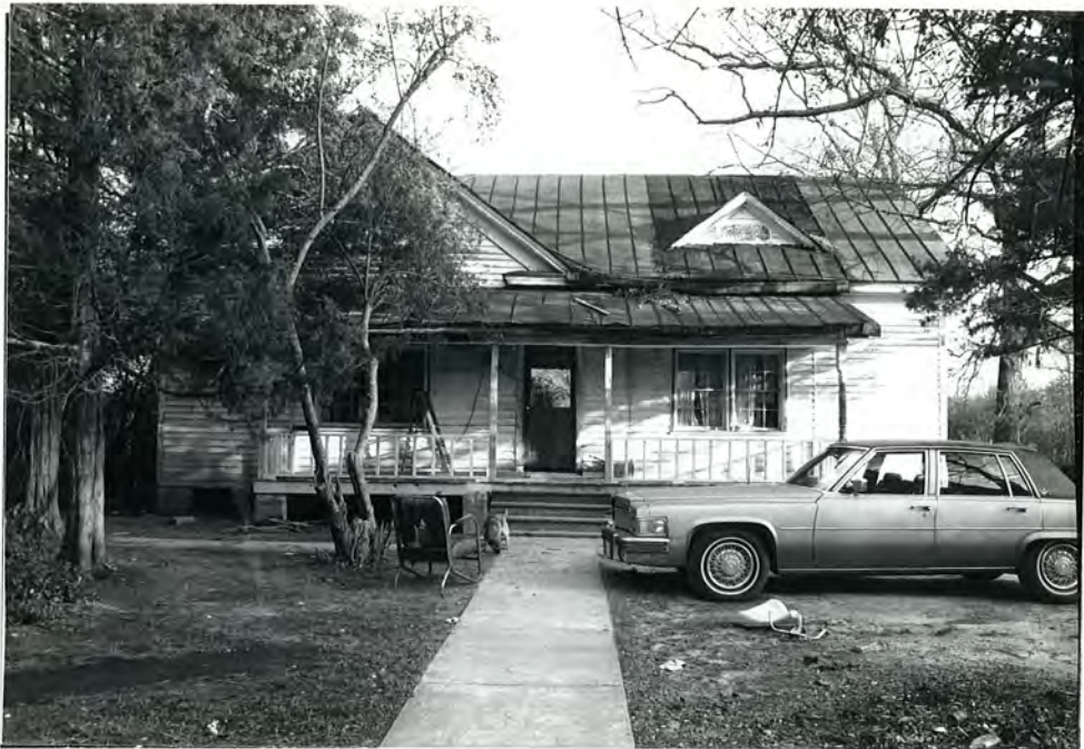
55. (A) Brantley's Grove School, facade, view to SE
