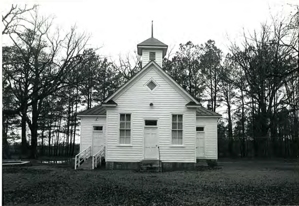
42. (C) Pleasant Plains School, facade, view to W
