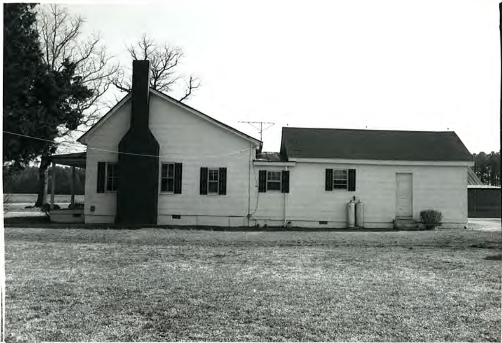
74. (B) House, NW elevation, view to SE
