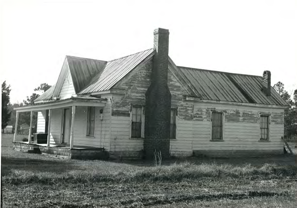
68. (B) House, N elevation, view to SW
