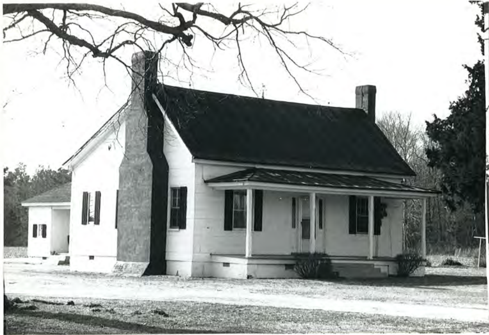
73. (A) House, overall view to W
