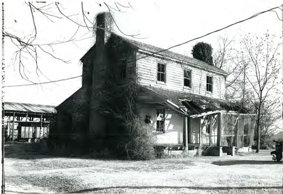
50. (A) Lawrence Askew House, overall view to NE
