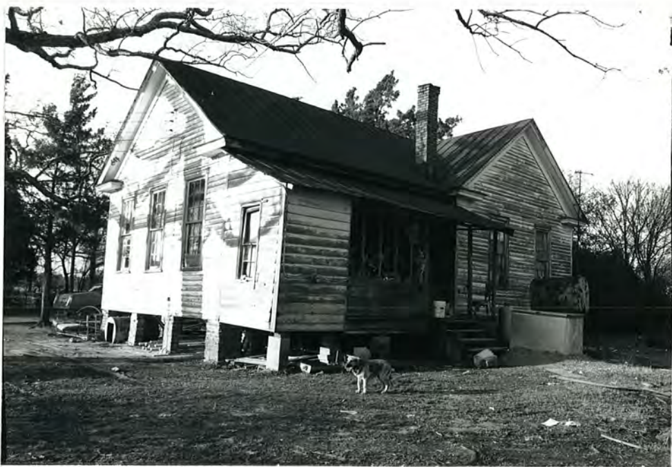
56. (B) Brantley's Grove School, rear, view to N
