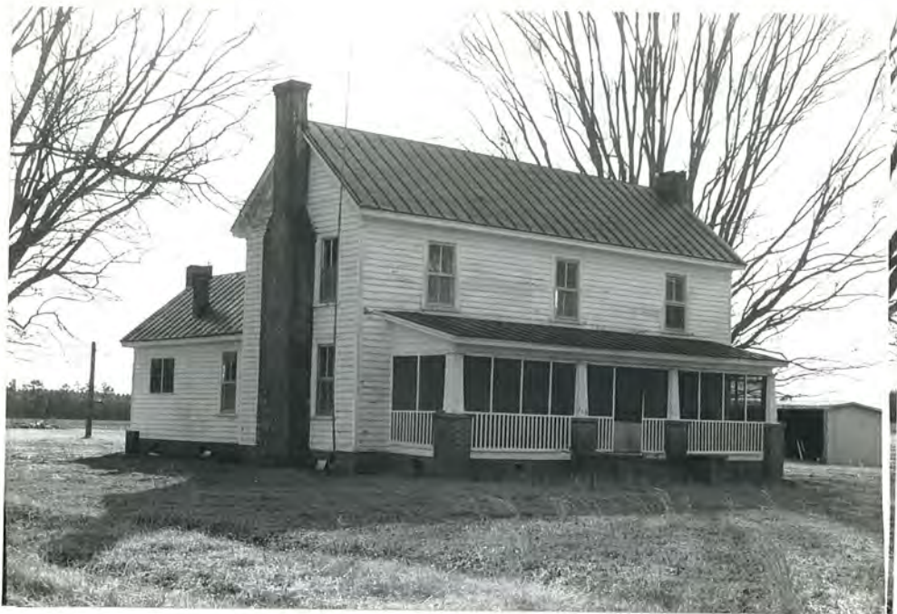
33. (B) William G. Livermon House and Outbuildings, overall view of house to SW
