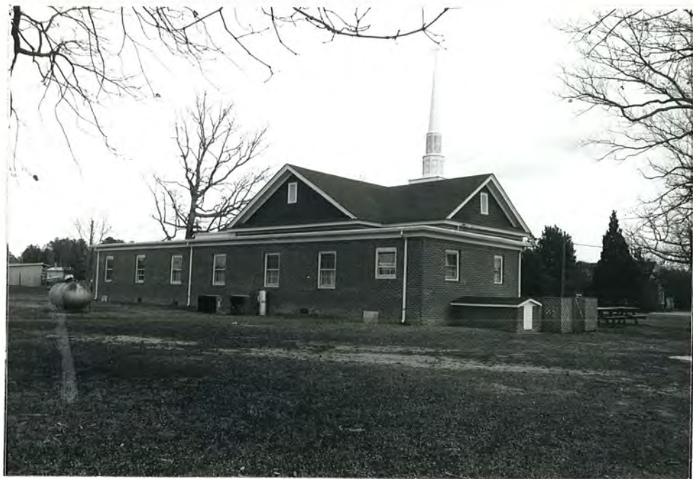
54. (B) Brantley's Grove Baptist Church, rear view to E
