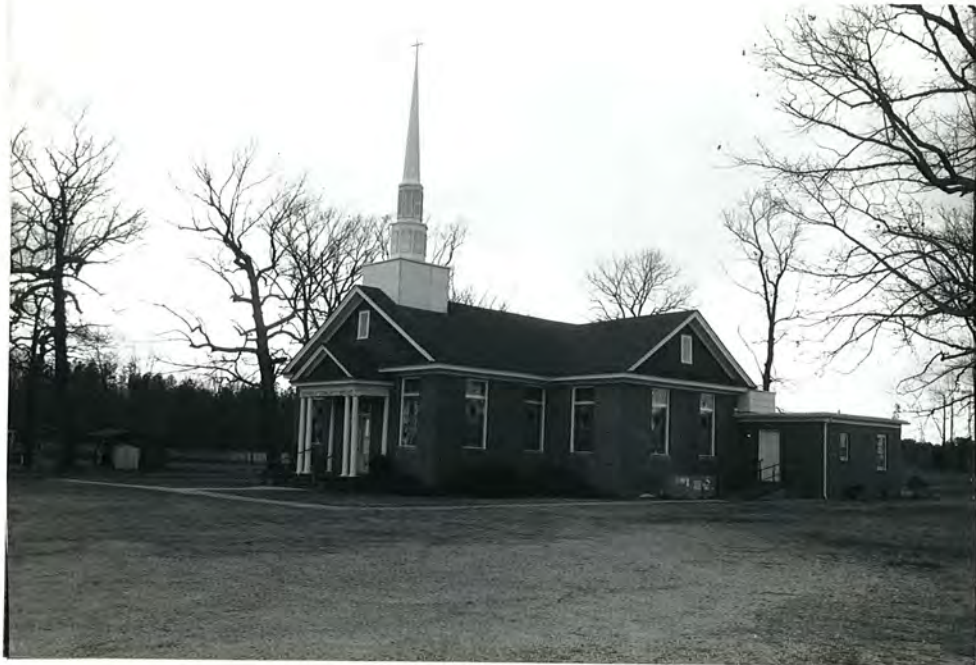
53. (A) Brantley's Grove Baptist Church, overall view to W
