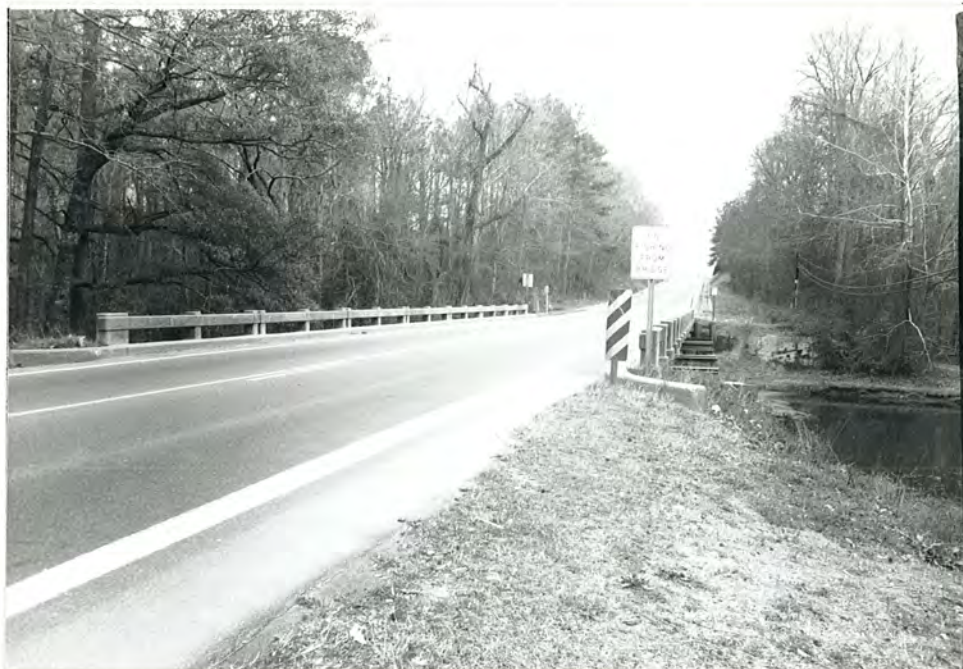
2. US 13/NC 42, just N of bridge over Ahoskie Creek in Ahoskie Swamp, view to SE
