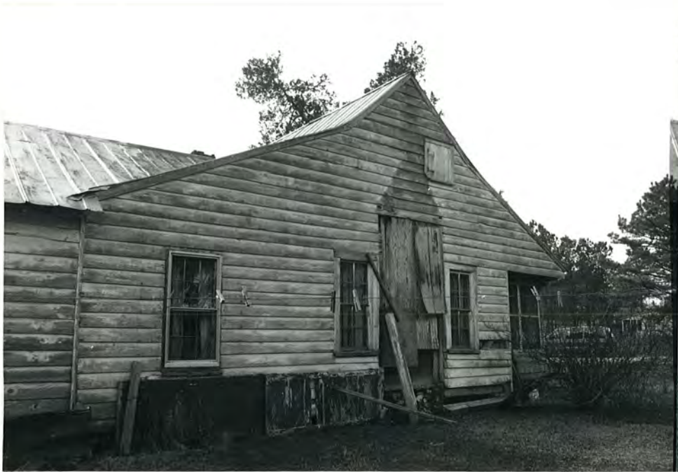
66. (B) House, N elevation, view to SW
