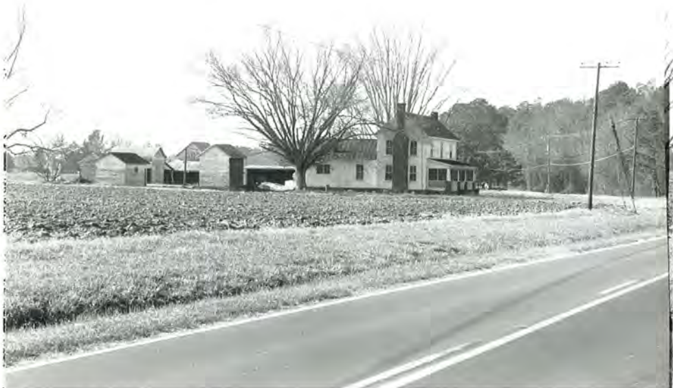
32. (A) William G. Livermon House and Outbuildings, overall view to SW
