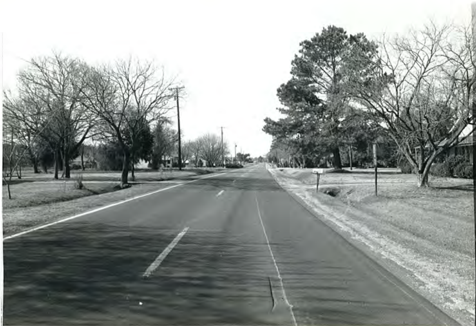
3. NC 561, 0.8 mi W of jct w/SR 1419, view to W
