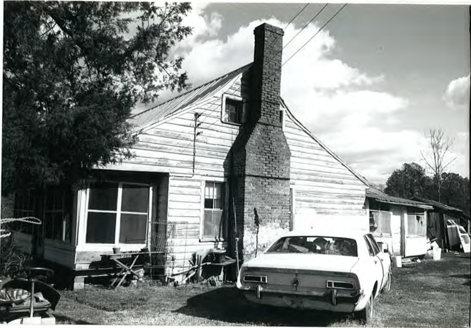
65. (A) House, S elevation, view to NE
