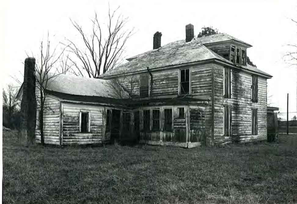
82. (B) John Whidby Newsome House, rear, view to NE
