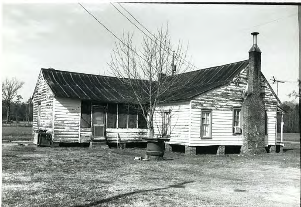
76. (B) House, rear, view to N
