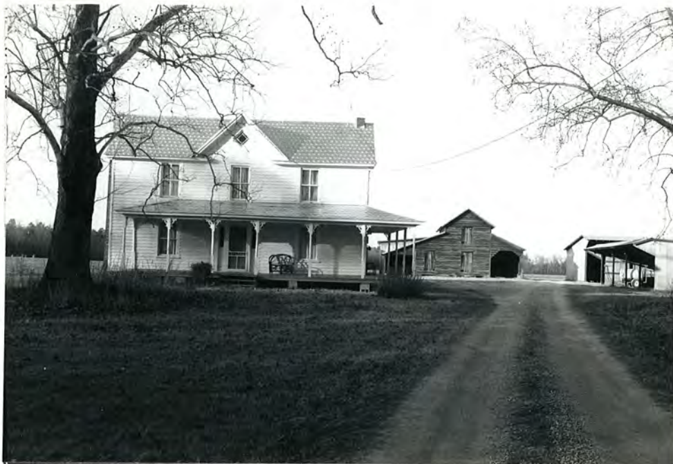
21. (A) Albert Hall Farm, overall view to N
