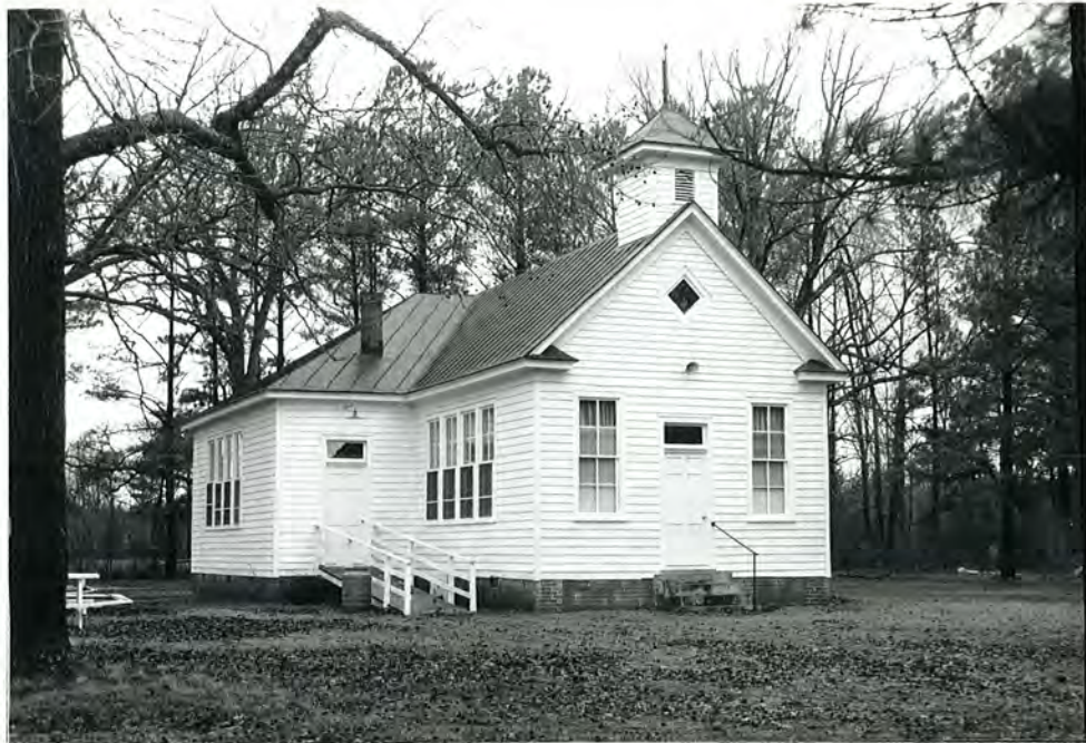
40. (A) Pleasant Plains School, overall view to NW
