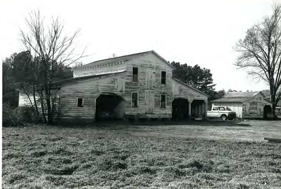
77. (C) House, outbuildings, view to W
