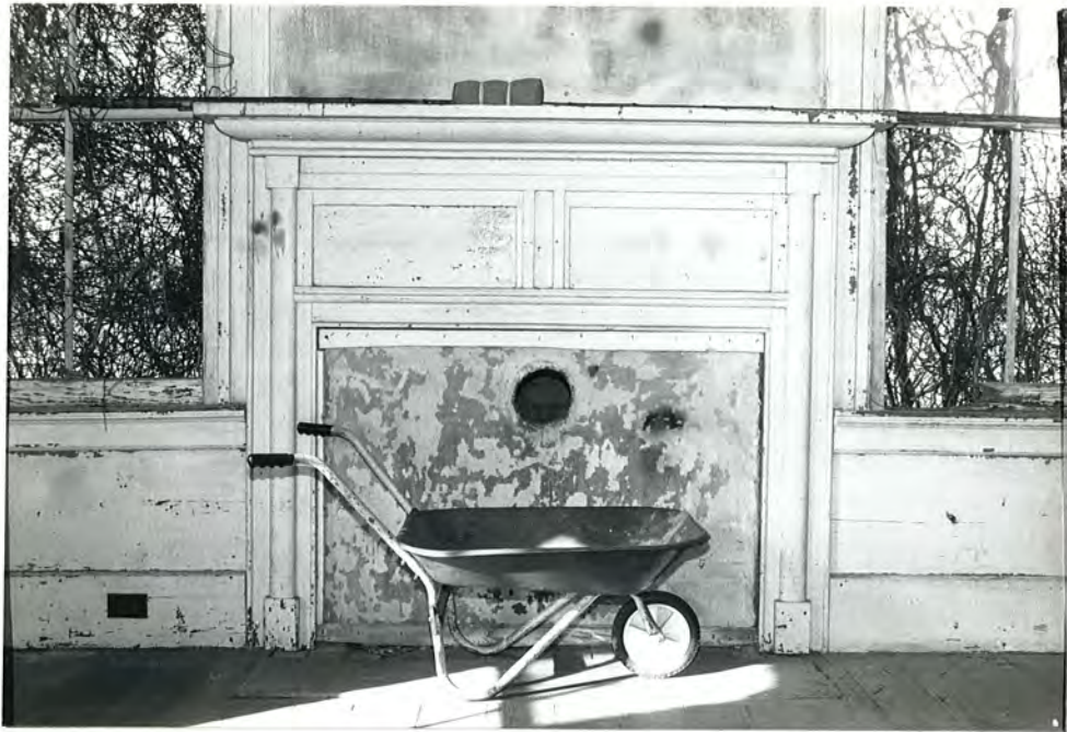
51. (B) Lawrence Askew House, parlor mantel, view to W
