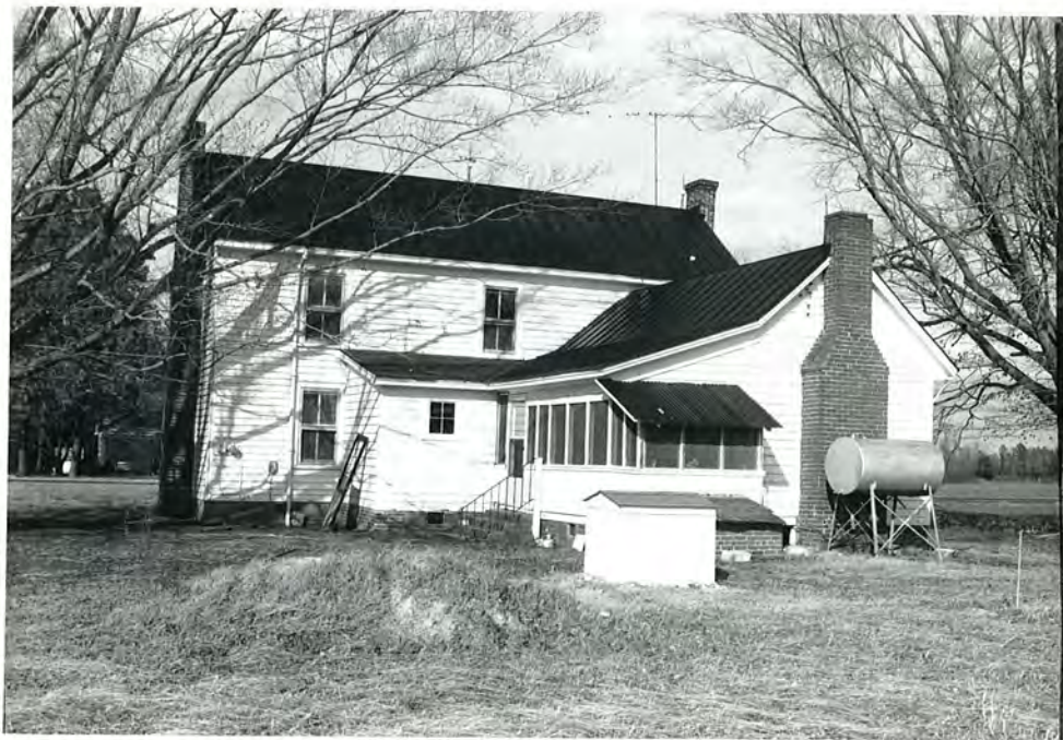
34. (C) William G. Livermon House and Outbuildings, rear view to N
