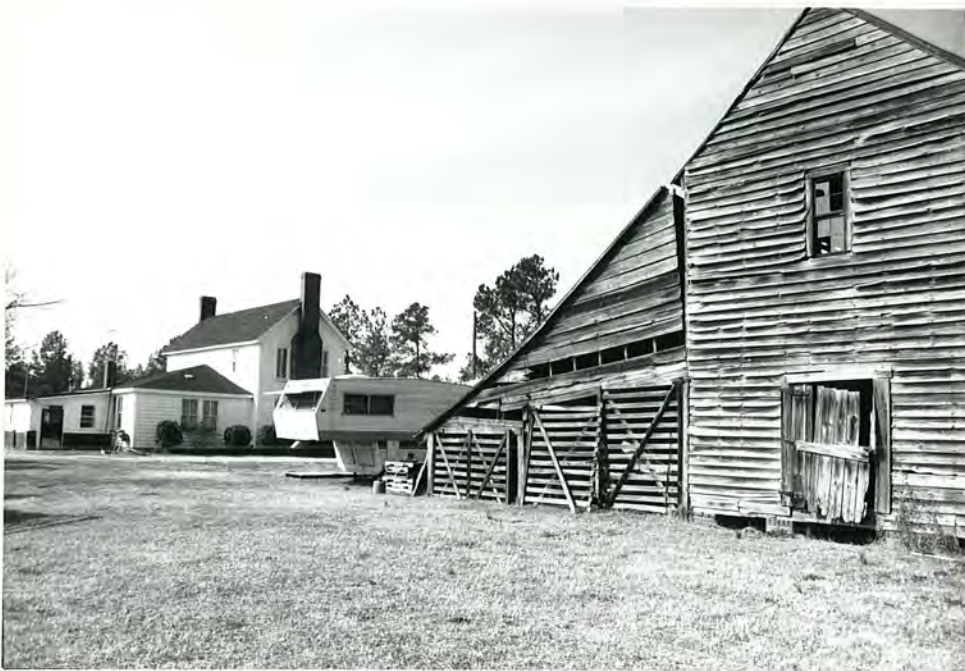
70. (B) House, barn and house, view to W
