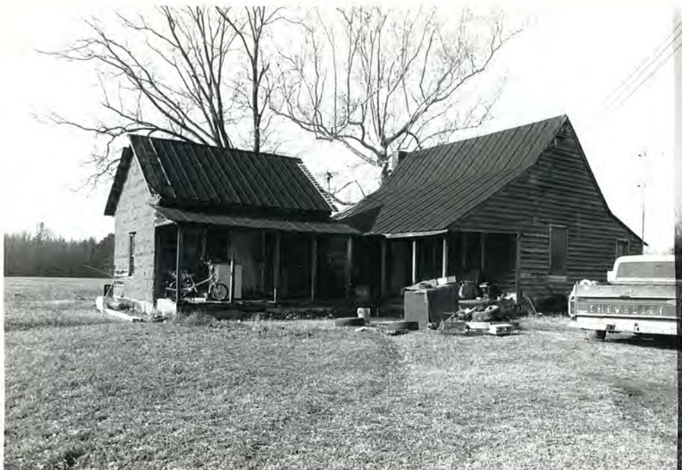
63. (A) Anthony Godwin House, overall view to SW
