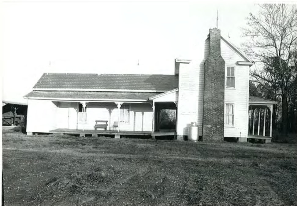
22. (B) Albert Hall Farm, W elevation, view to E
