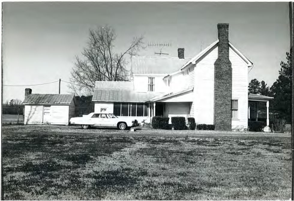
44. (B) William B. Weaver Farm, SE elevation, view to NW
