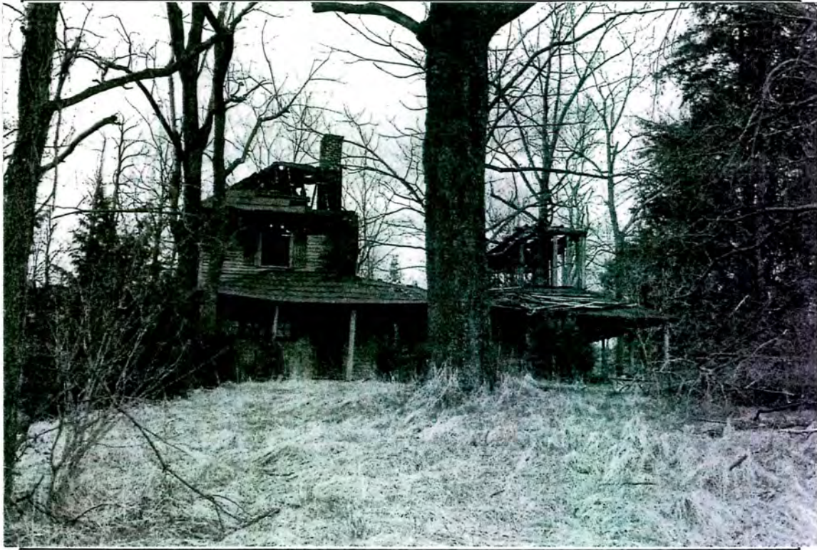
7. Williamson House. Located in southeast quadrant of I-26/US 25 interchange, Henderson County.
