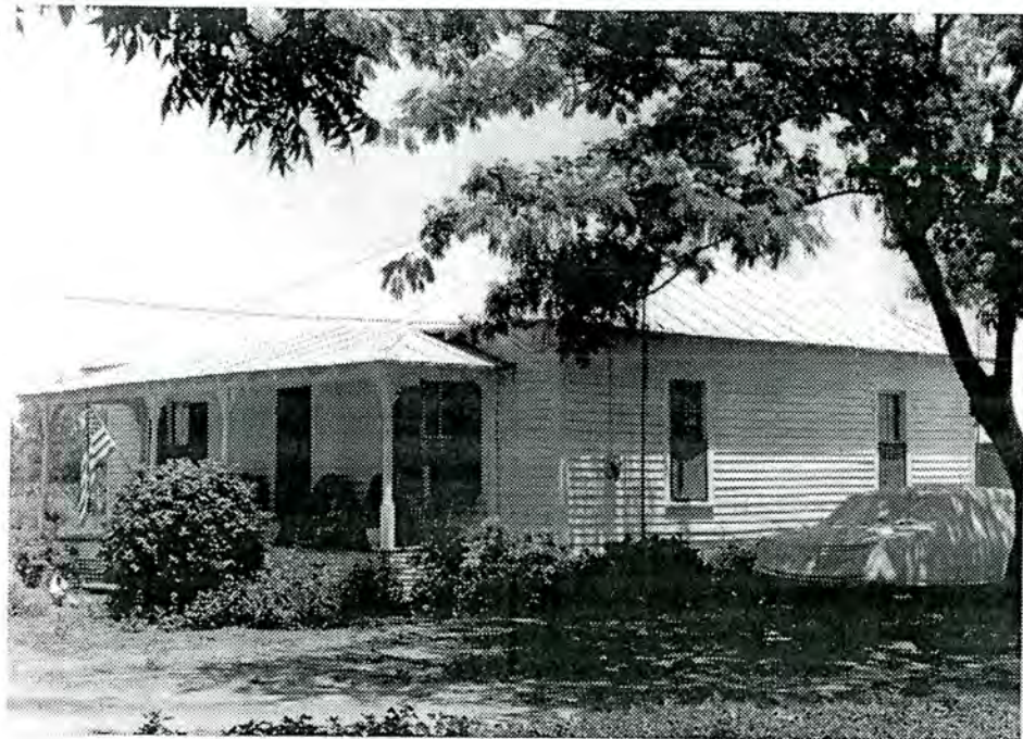
Figure V.73 Noah Small, Sr. House: overall front view
