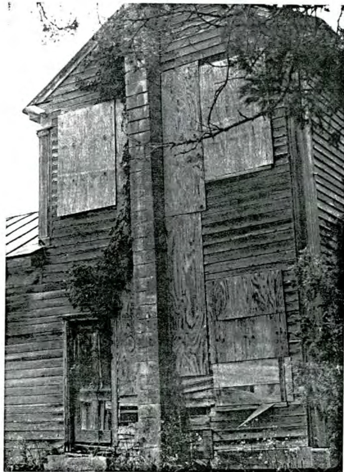
Figure IV.24 Wylie T. Moseley House: east gable end
