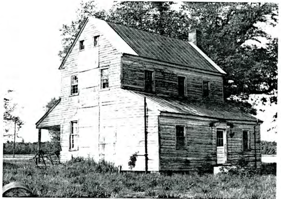
Figure IV.33 A. Moore House: overall view from rear
