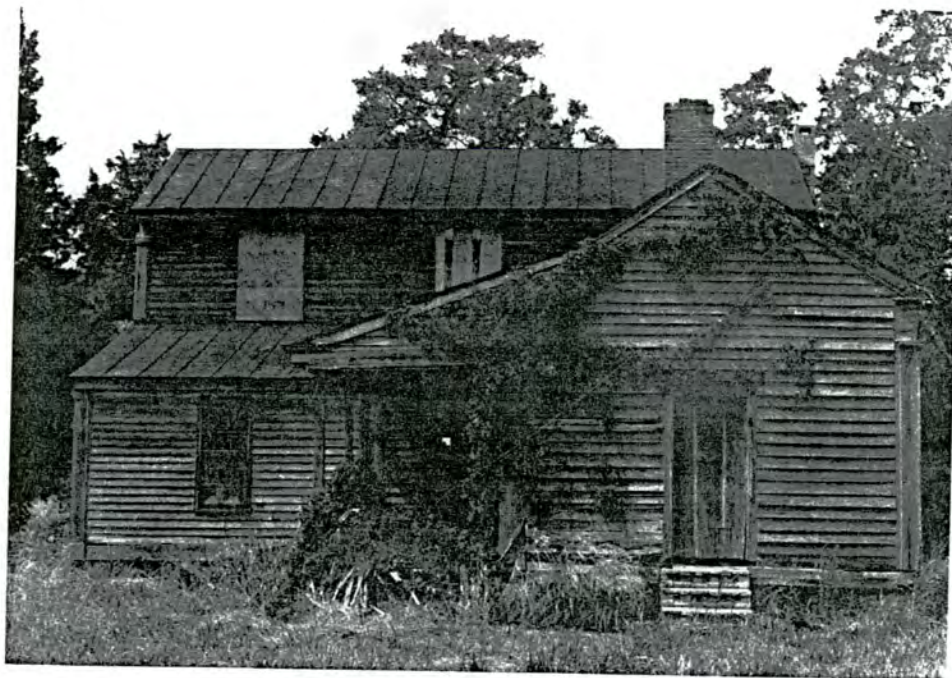
Figure IV.26 Wylie T. Moseley House: hall view toward front door
