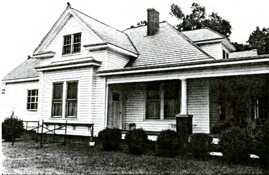
Plate 19. Frank Watt House, North Elevation, Looking South.
