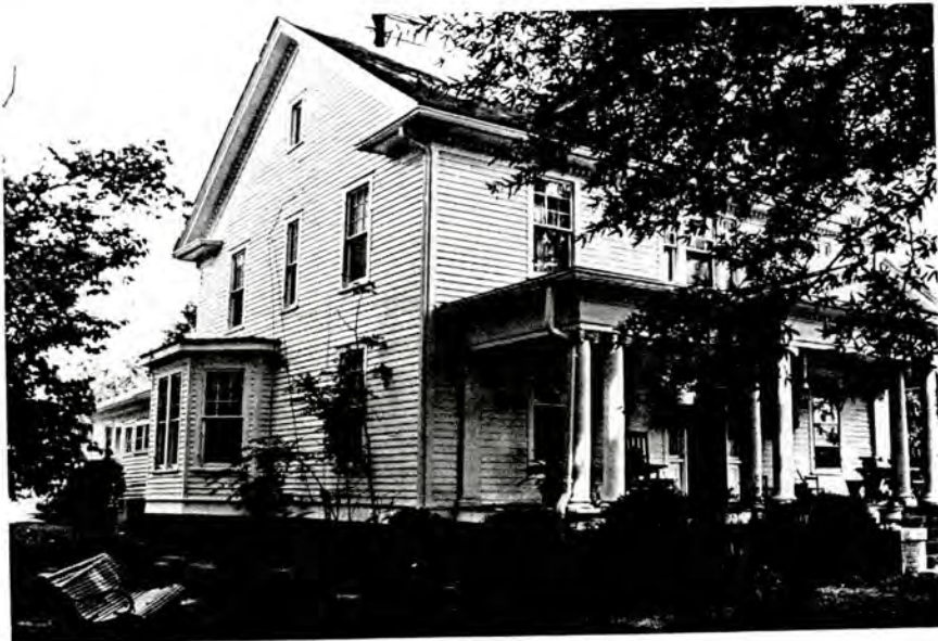
Plate 8. McDowell House, Main Facade and North Elevation, Looking Southeast.
