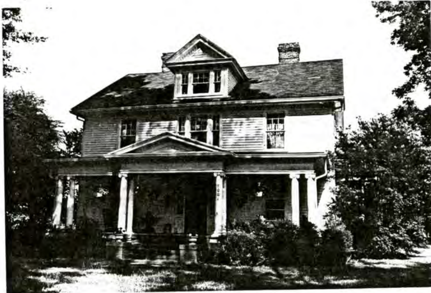
Plate 6. McDowell House, Main Facade, Looking East.
