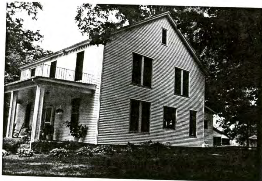
Plate 45. J. B. Watt House, North Elevation, Looking South.
