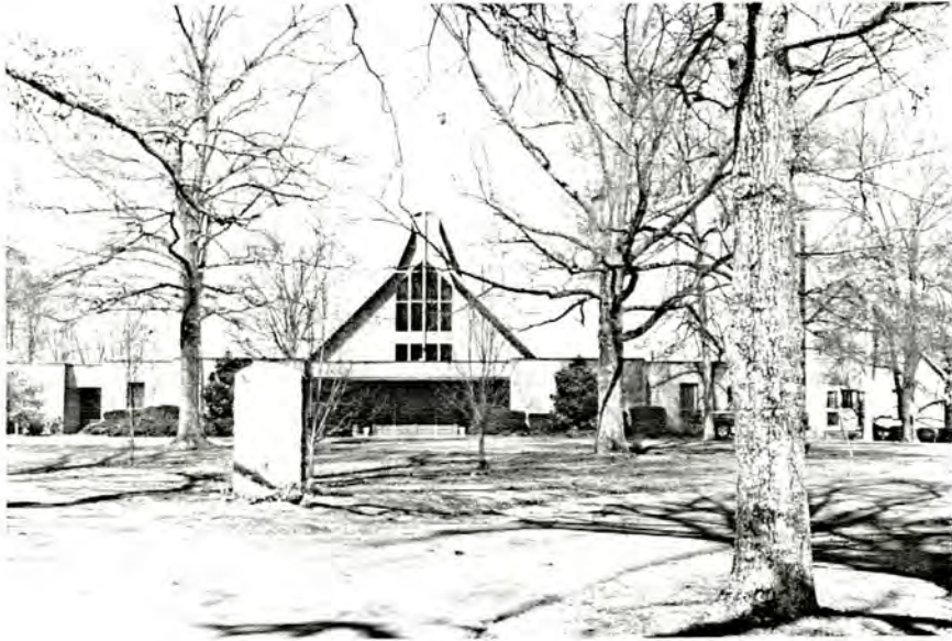
Plate 32. Pleasant Hill Presbyterian Church, Looking North.
