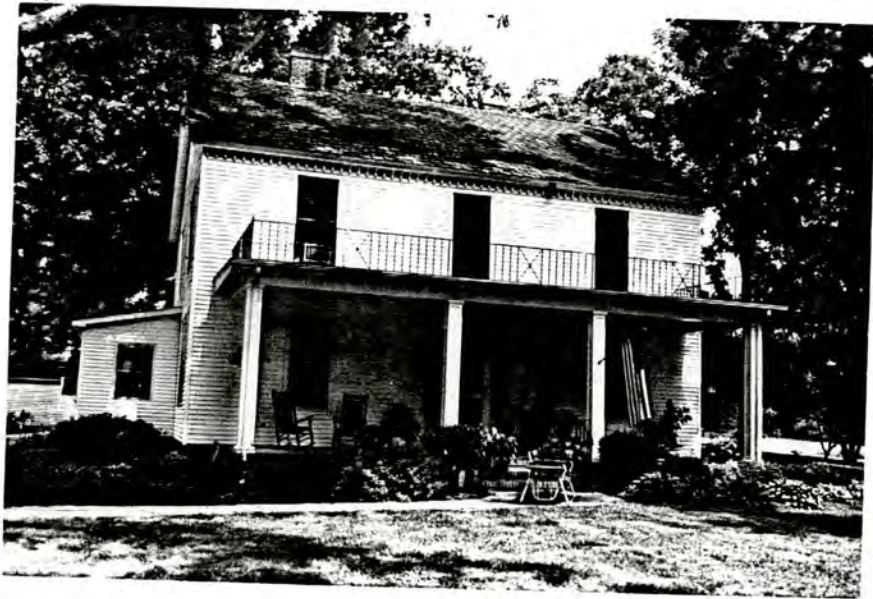
Plate 43. J. B. Watt House, Main Facade, Looking West.
