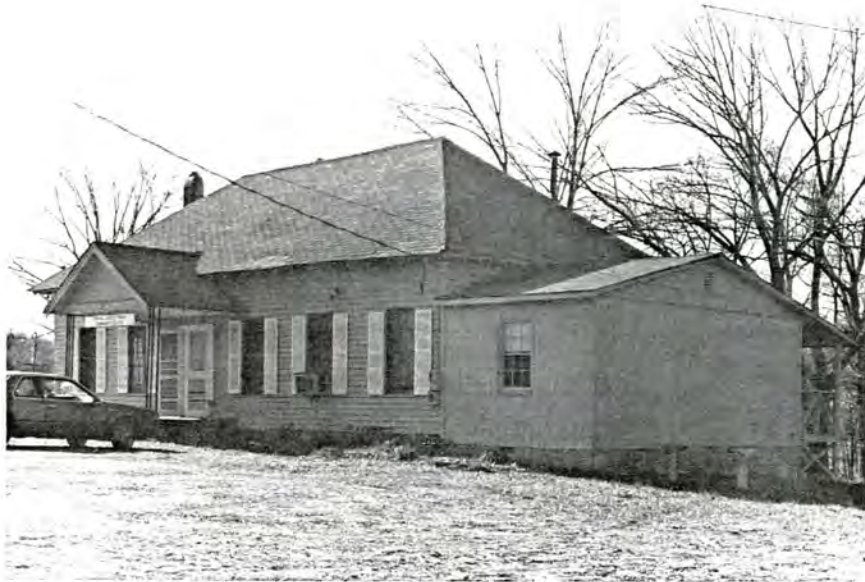
Plate 39. (Former) Steele Creek School, Facade and North Elevation, Looking Southwest.
