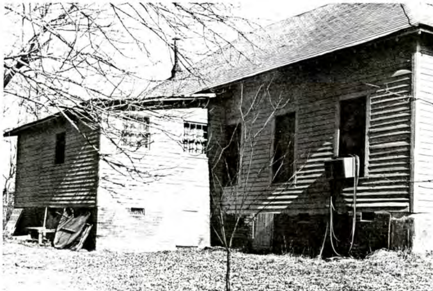
Plate 40. (Former) Steele Creek School, Rear Elevation, Looking Northeast.
