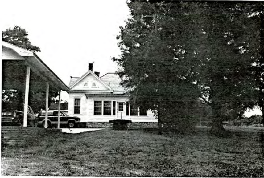
Plate 20. Frank Watt House, Rear Elevation, Looking West.
