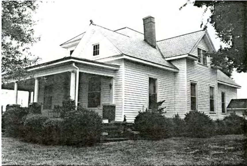
Plate 18. Frank Watt House, Main Facade and South Elevation, Looking Northeast.
