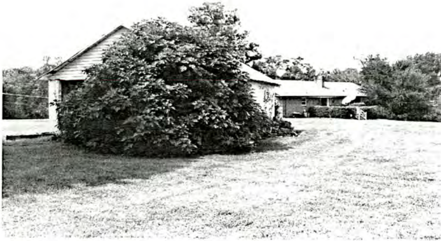
Plate 15. McDowell House Property, Auto Garage, Looking North.
