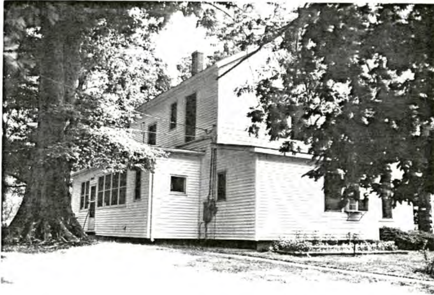
Plate 46. J. B. Watt House, Rear Elevation, Looking North.
