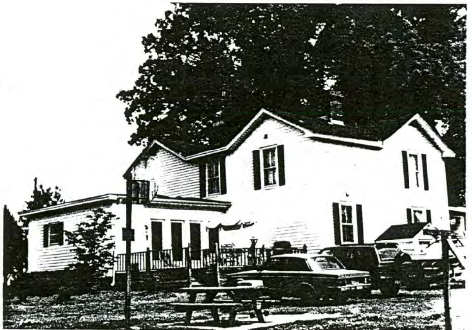
Fig. VIII.42 Hartsfield-Taylor House Rear view
