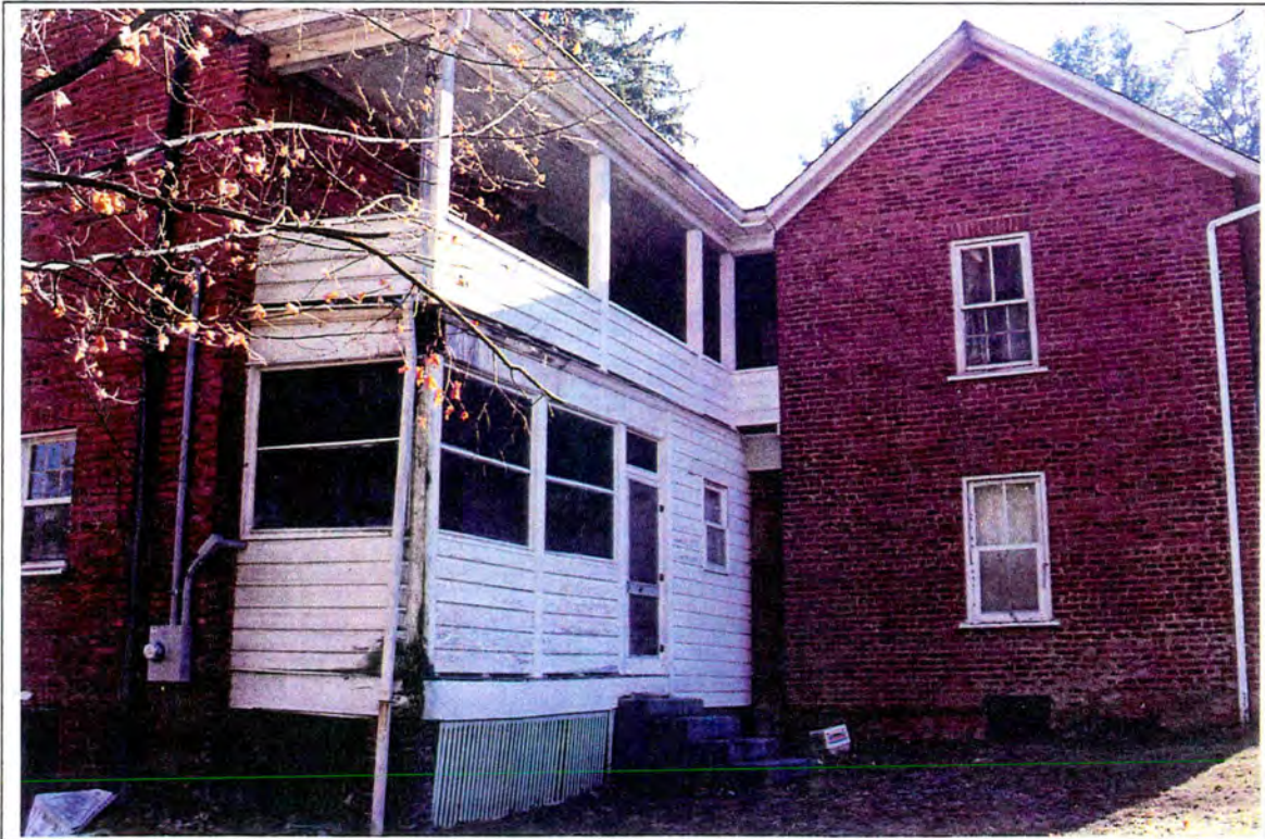
MILLER-FRANCIS HOUSE (HW 81), rear
