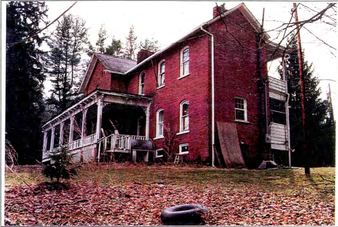
MILLER-FRANCIS HOUSE (HW 81), view from northeast
