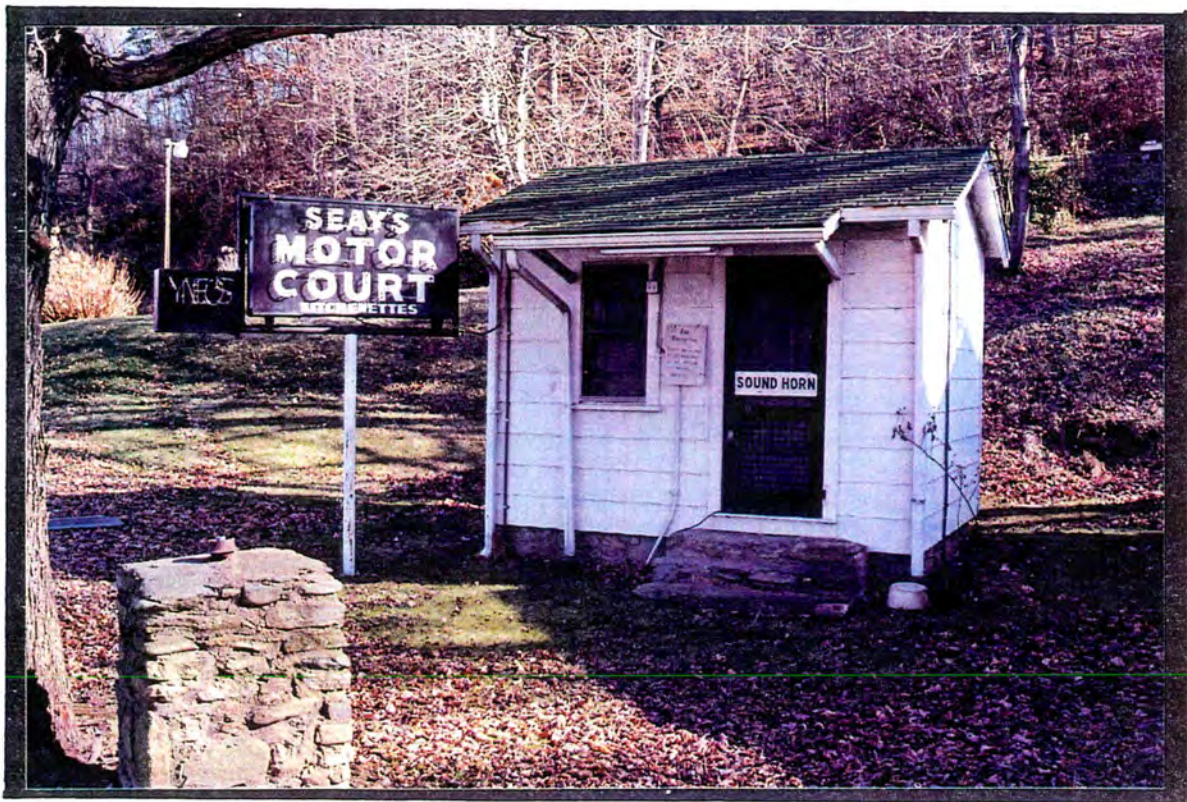
Property #6--Seay's Motor Court, office.
