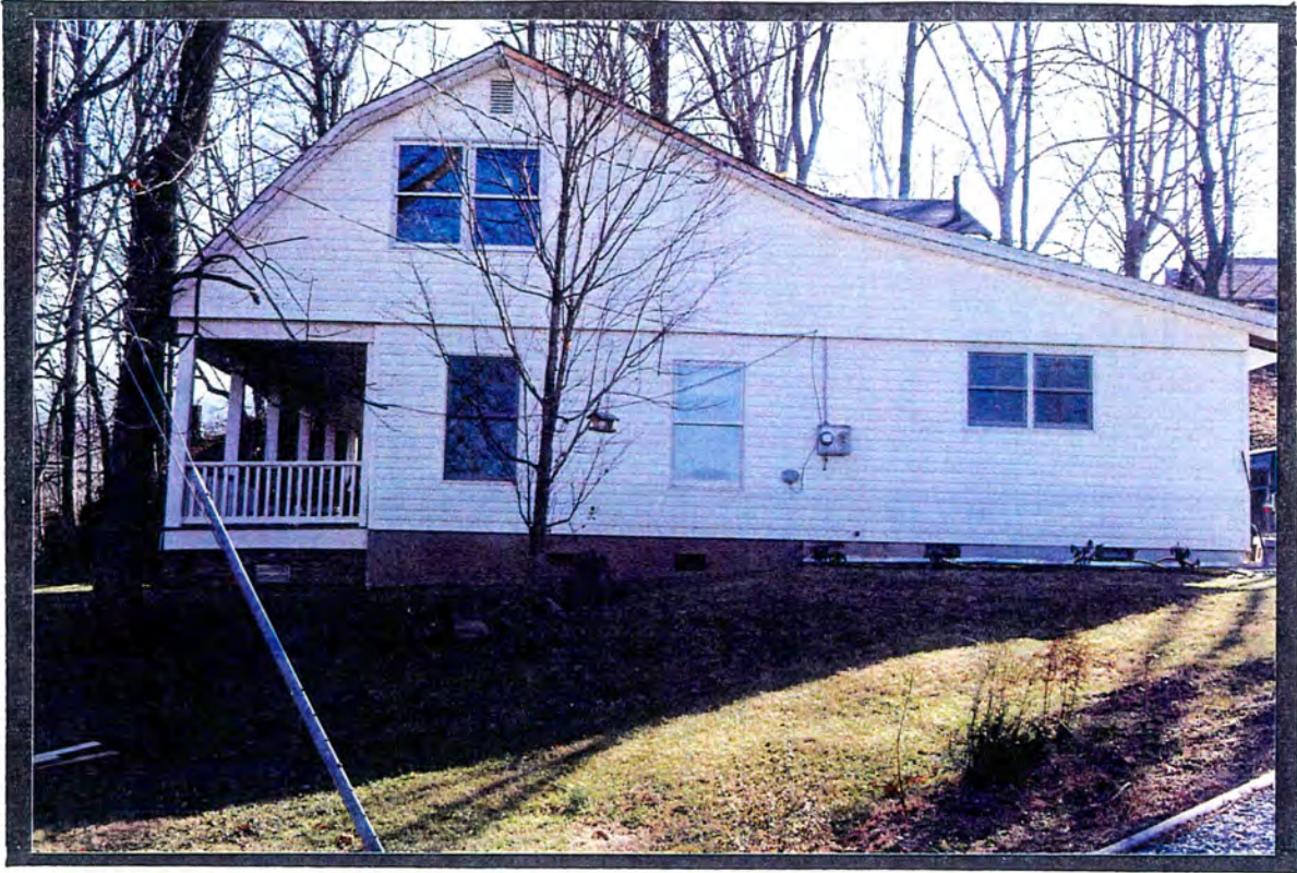
Property #9--Welch-Byers House, side elevation.
