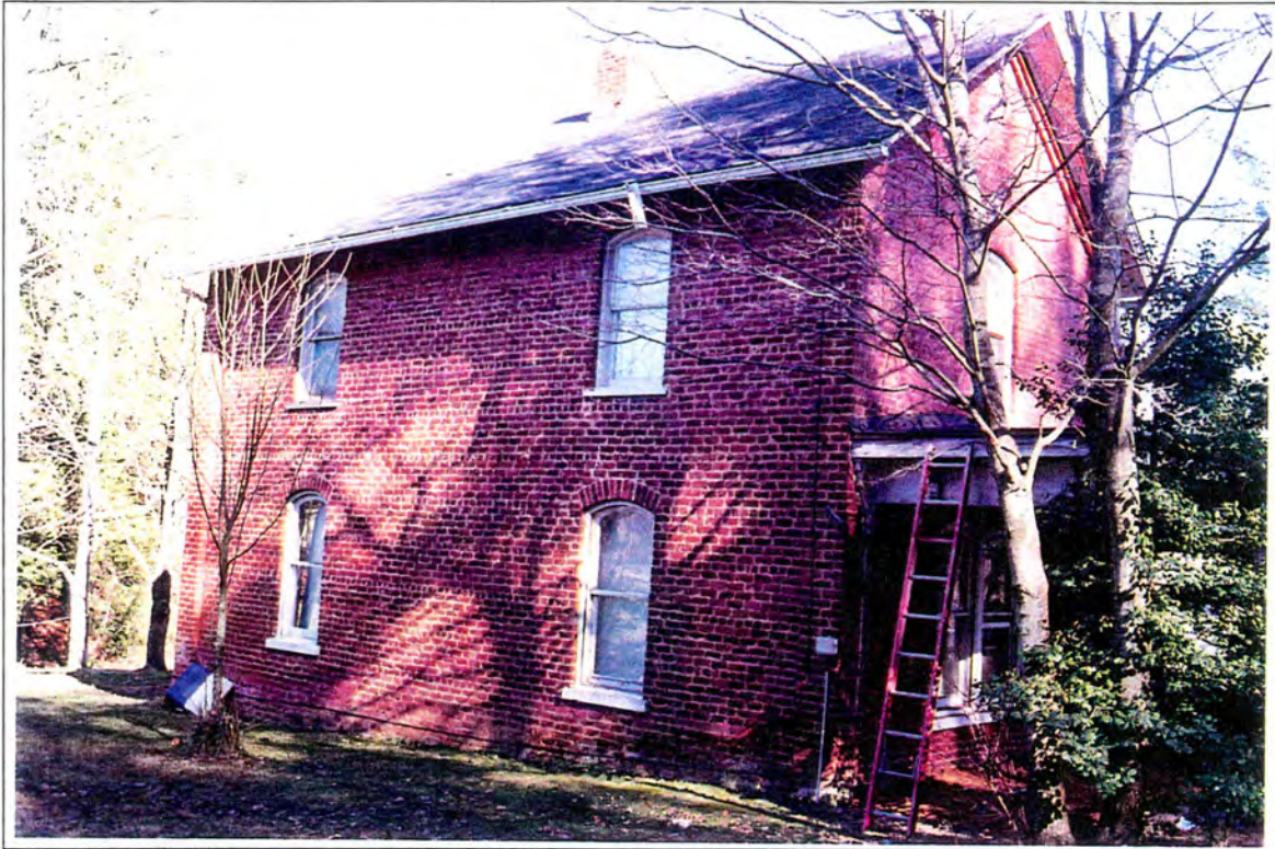
MILLER-FRANCIS HOUSE (HW 81), west side elevation
