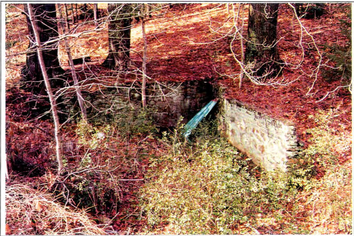
MILLER-FRANCIS HOUSE (HW 81), foundations at the back of the property
