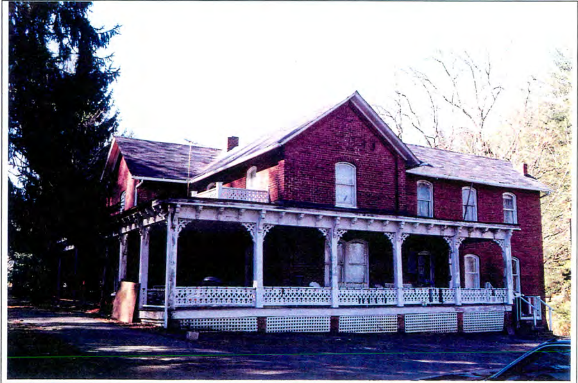
MILLER-FRANCIS HOUSE (HW 81), east side elevation
