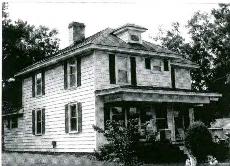
Fig. IV-13 Mt. Shiloh Baptist Church District: Rev. Alonzo Dudley House, Kennedy St. Dorcias Oden House, Scott St.
