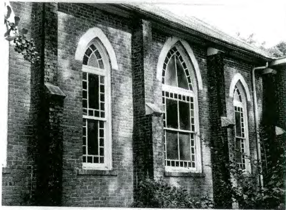
Fig. III-5 Jones Chapel AME Zion Church: front door; side windows
