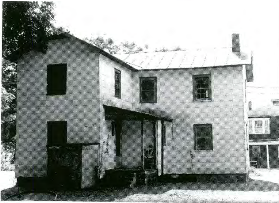
Fig. IV-22 Andrews House, 1202 Old Cherry Point Road: views
