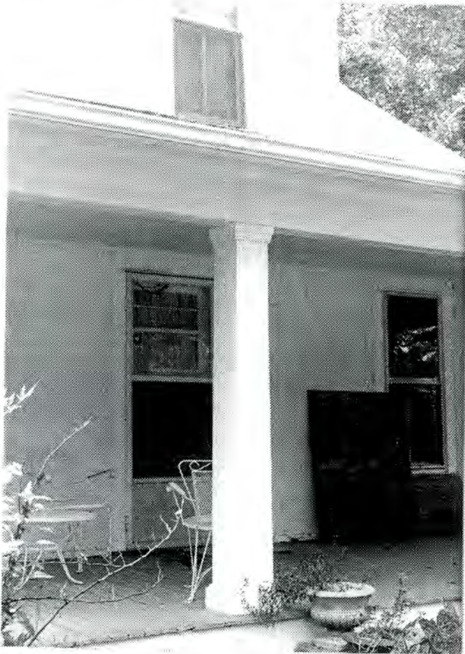
Fig. IV-26 House, 302 Green Springs Road: views
