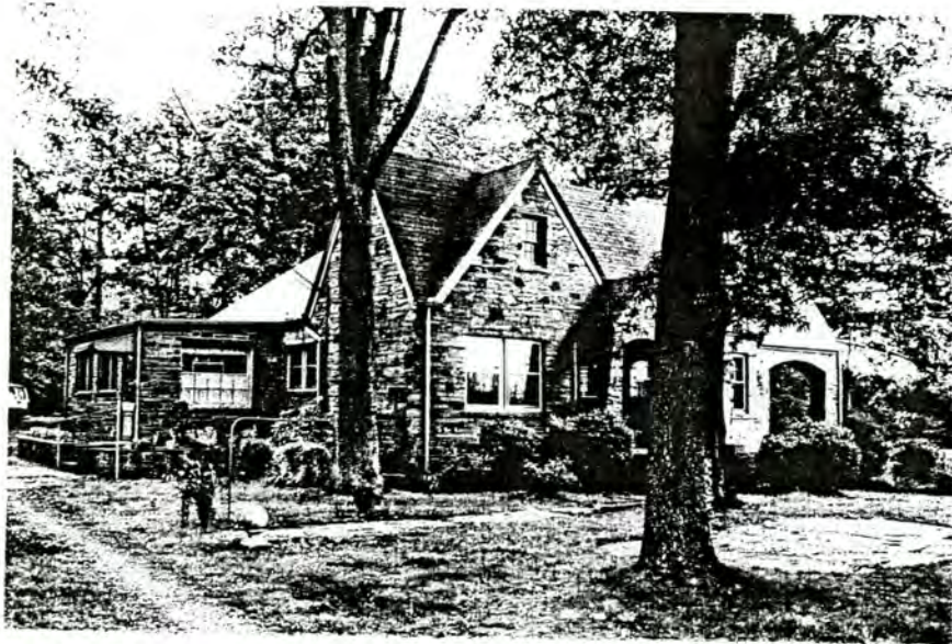
Plate 8. Herman Wagoner House, Facade and North Elevation, Looking Northeast.
