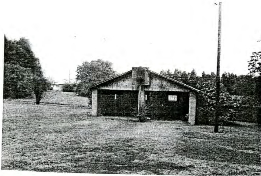
Plate 4. Barringer-Lanning House, Garage, Looking Northeast.
