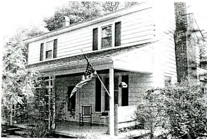
Plate 53. Lyerly Log House, Front Elevation, Looking South.
