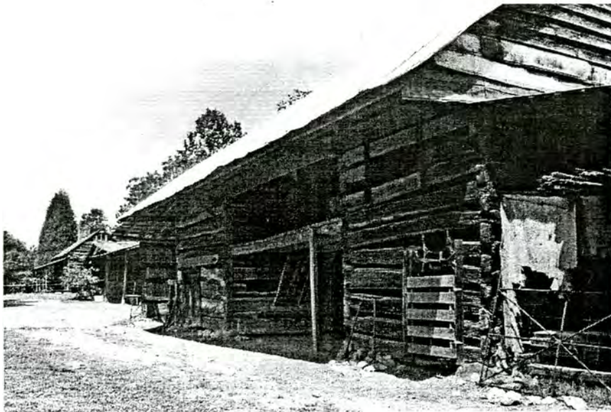
Plate 79. Walton Log Barn, Looking West.
