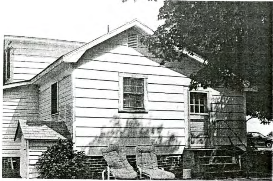
Plate 87. Lyerly-Huffman House, Rear Ell, Looking North.
