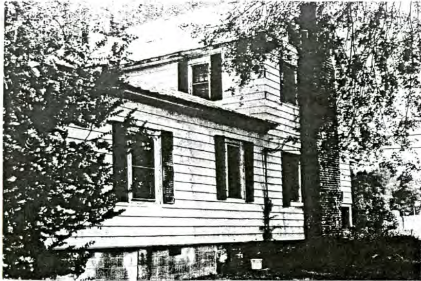
Plate 26. Pickler House, East Elevation and Rear ell, Looking Northwest.
