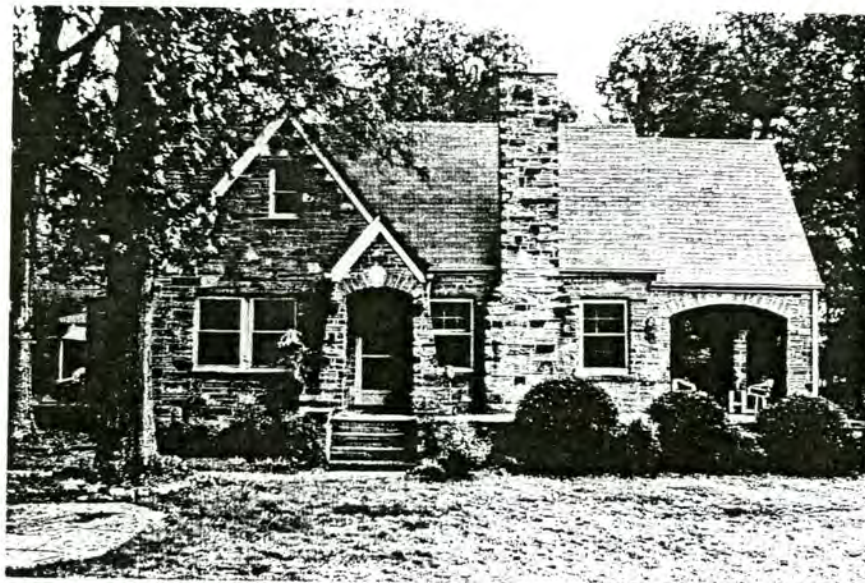
Plate 6. Herman Wagoner House, Facade, Looking Northeast.
