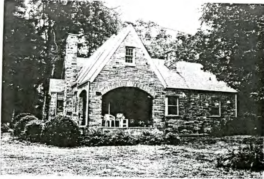
Plate 7. Herman Wagoner House, South Elevation, Looking North.
