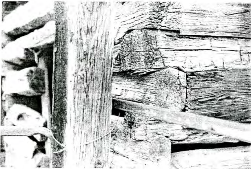
Plate 37. Notching Detail, Earnhardt Log Barn.
