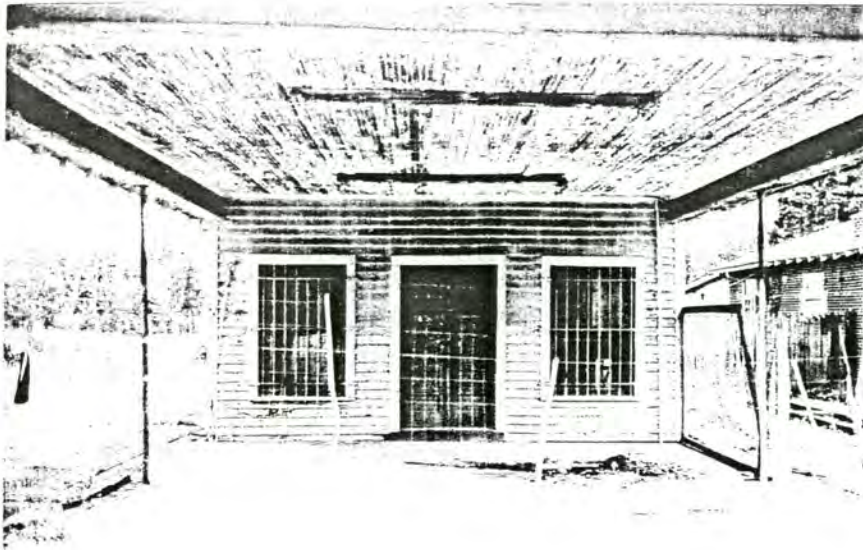
Plate 21. Helderman Gas Station, Facade, Looking Northeast.
