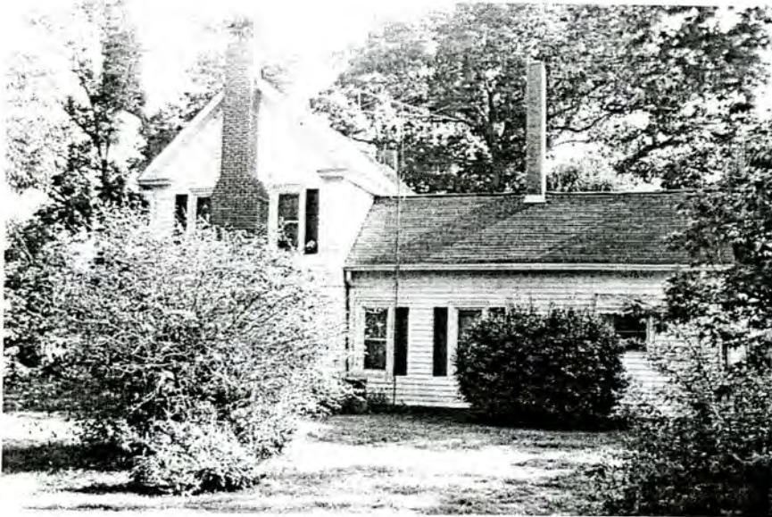
Plate 108. Rufus Eller Farm, North Elevation of House, Looking South.
