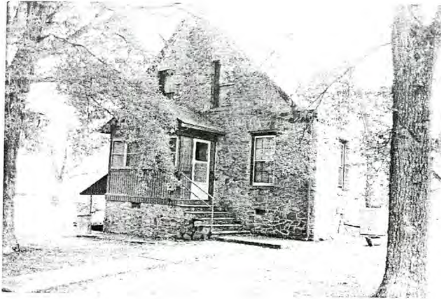
Plate 3. Barringer-Lanning House, Rear (North) and West Elevations, Looking South.
