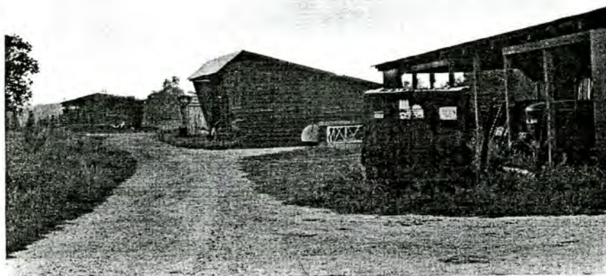
Plate 93. Lyerly-Huffman House, Modern Farm Buildings South of Farmyard, Looking South.
