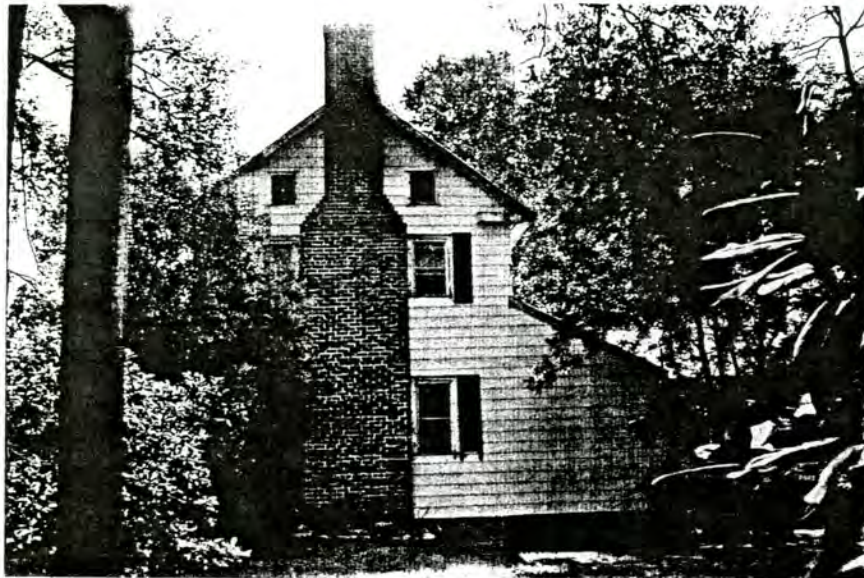
Plate 27. Pickler House, West Elevation, Looking East.
