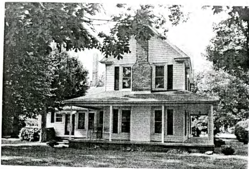
Plate 109. Rufus Eller Farm, South Elevation of House, Looking North.
