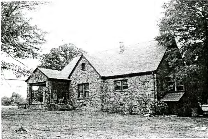
Plate 2. Barringer-Lanning House, South Elevation, Looking Southwest.
