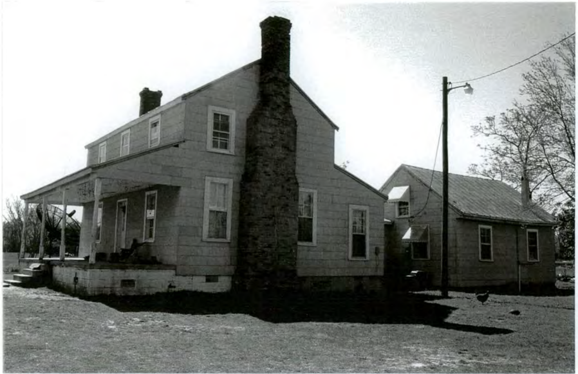
PLATE 17 Munfred Brewer House (#17) - Main house, north front and west side elevations
