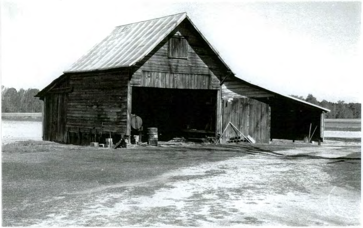
PLATE 5 Fields-Sugg House (#9) - Tobacco barn/shed, north front and east side elevations
