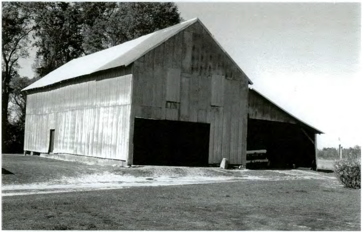
PLATE 11 Fields-Sugg House (#9) - Barn, north front and east side elevations
