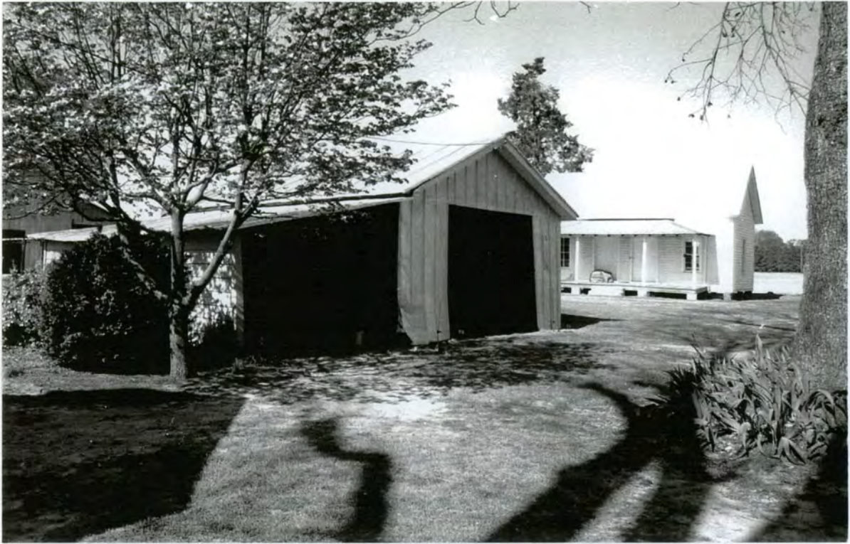
PLATE 8 Fields-Sugg House (#9) - Garage, north front and east side elevations; servant's dwelling to far right
