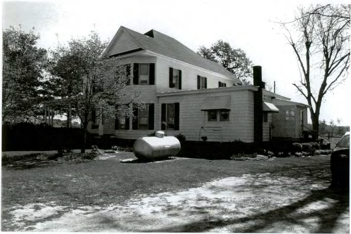
PLATE 4 Fields-Sugg House (#9) - Main house, south rear and west side elevations
