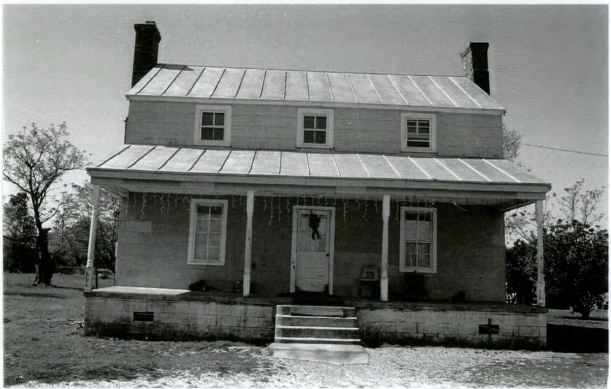
PLATE 18 Munfred Brewer House (#17) - Main house, north front elevation
