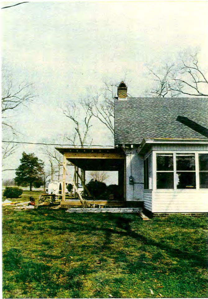
Figure 8 James M. Parrott House, Reconstruction of W porch
