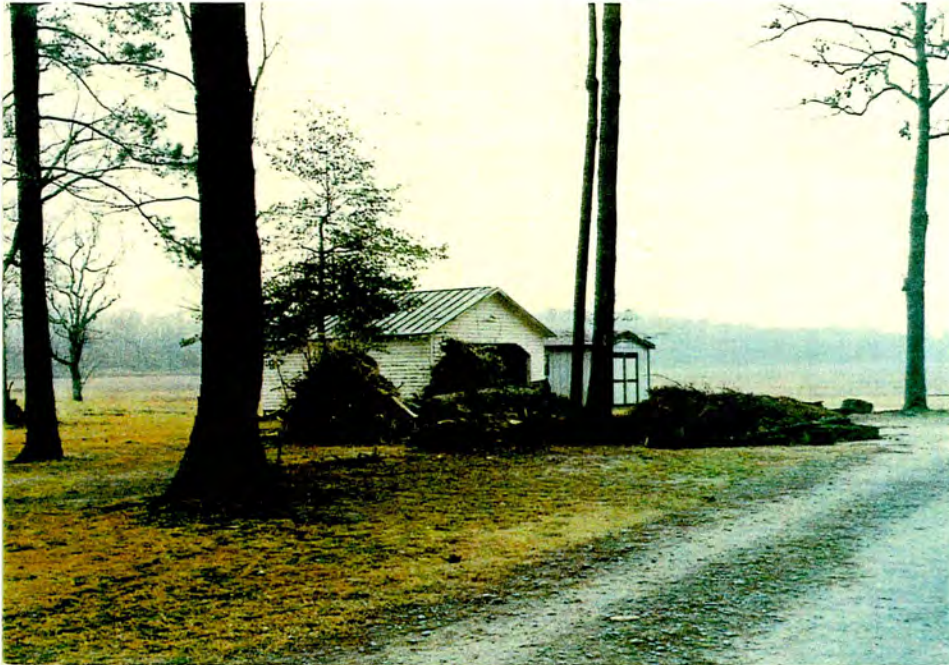
Figure 28 Sutton Farmhouse, E Elevation of garage
