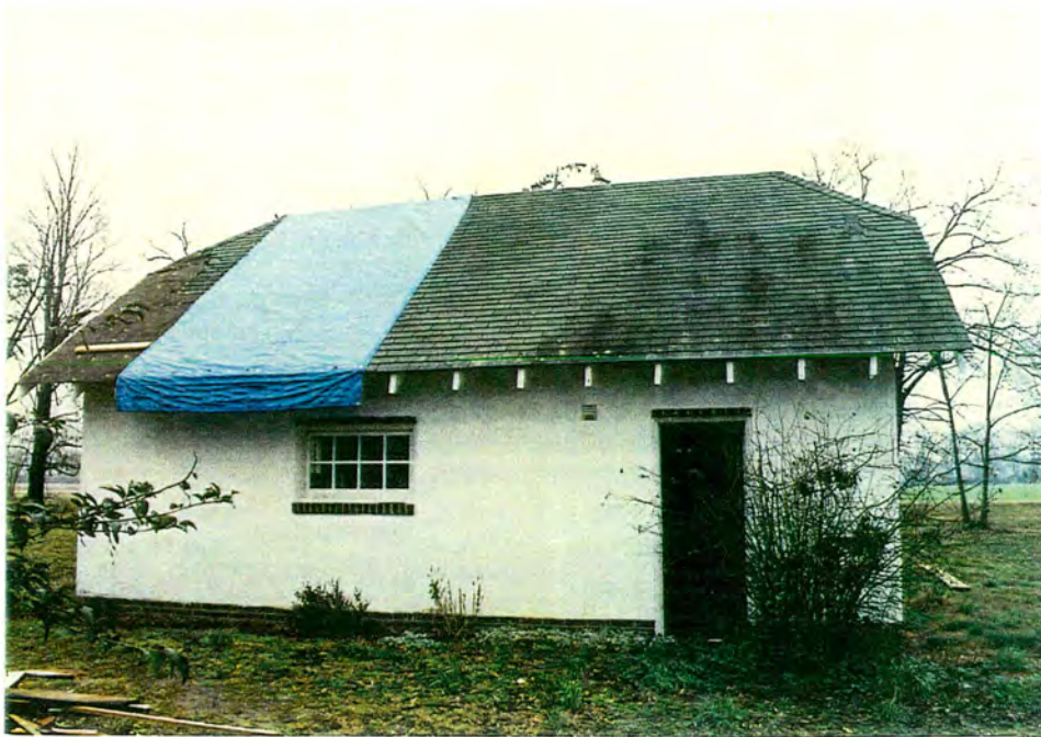
Figure 13 James M. Parrott House, W Elevation of garage
