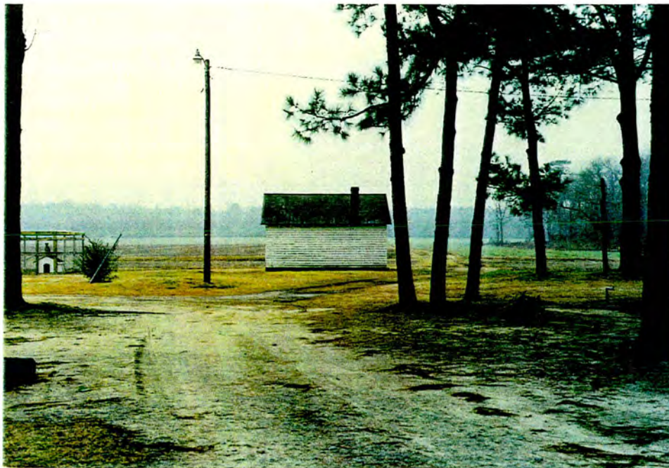
Figure 29 Sutton Farmhouse, E Elevation of storage shed
