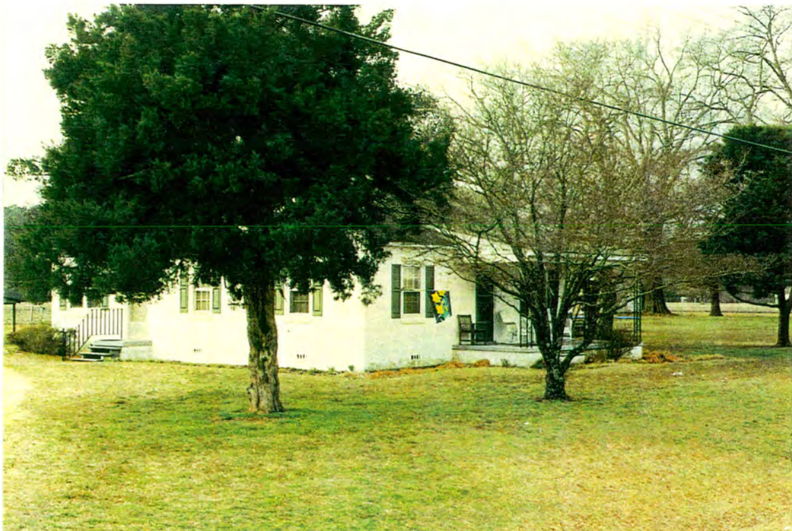
Figure 33 Property #3, House associated with Falling Creek Farms, Inc
