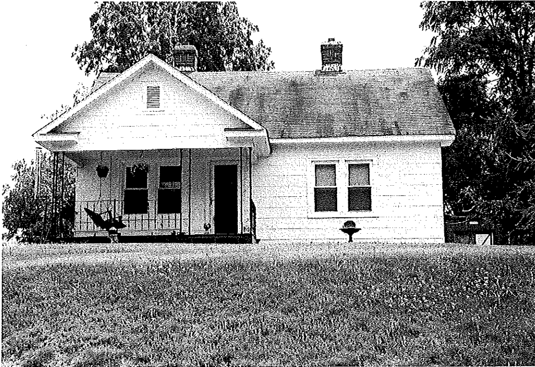
Property 49. House, 1938, 4024 Thomasville Road (NC 109), Forsyth County
