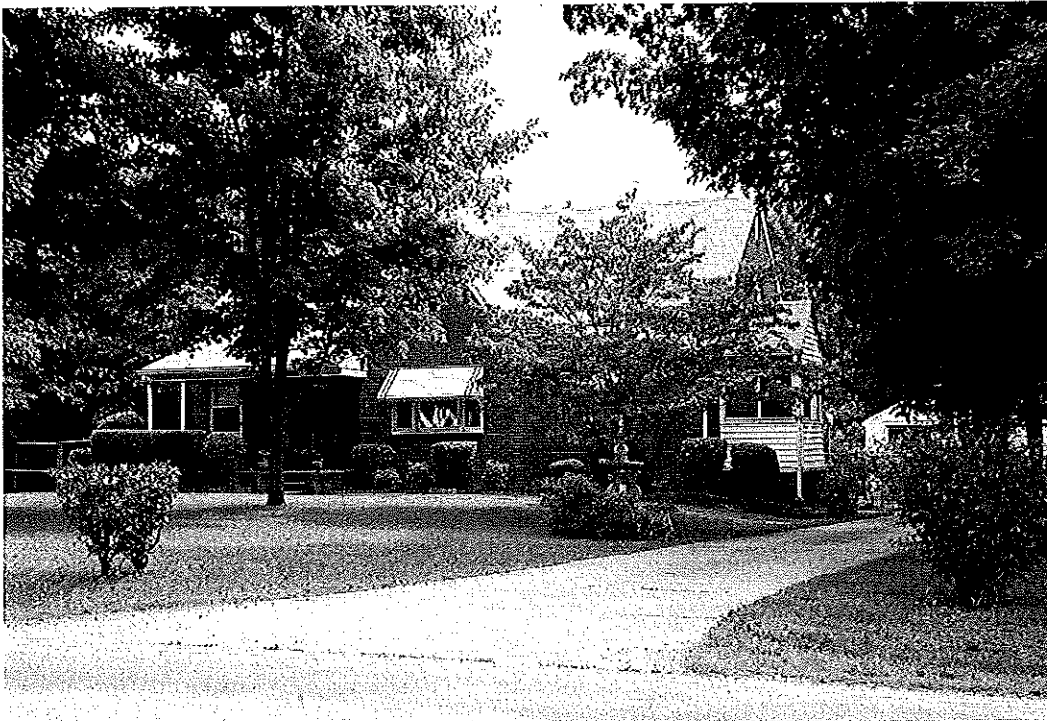
Property 16. House, 1951, 3511 Thomasville Road (NC 109), Forsyth County
