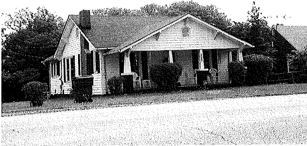
Property 15. House, 1931, 3503 Thomasville Road (NC 109), Forsyth County
