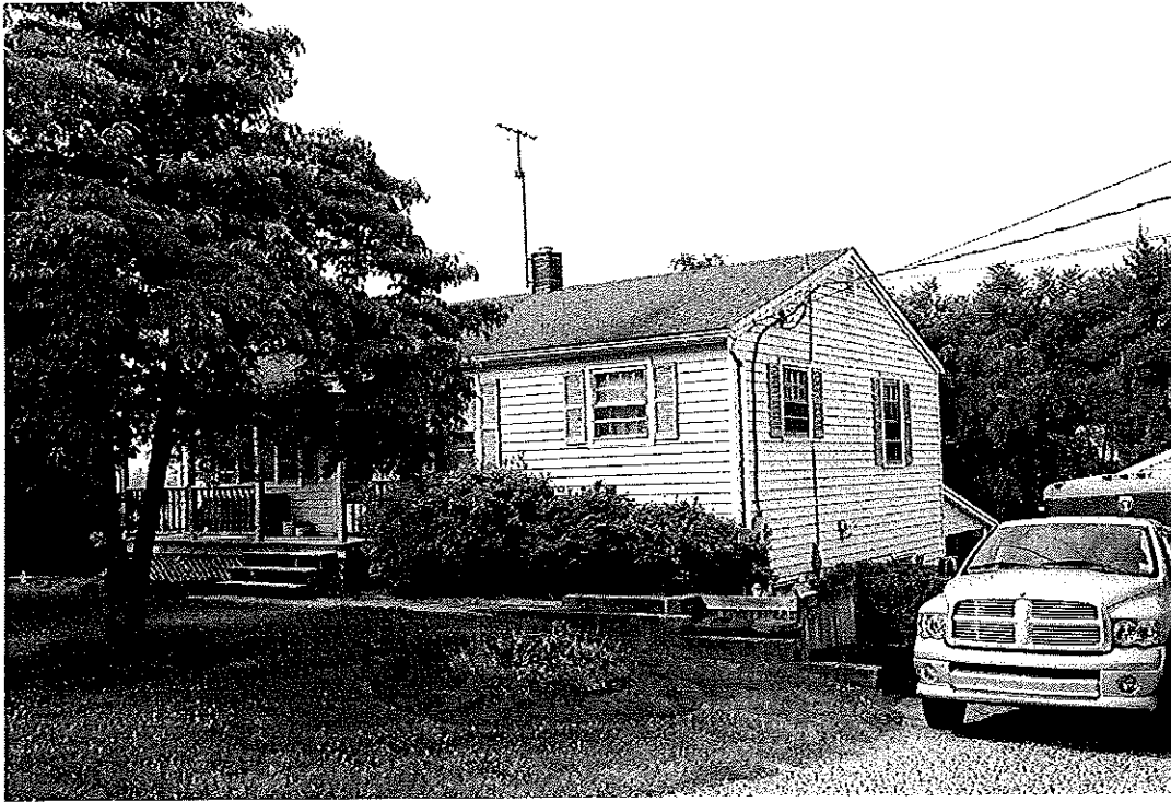
Property 33. House, 1956, 3634 Thomasville Road (NC 109), Forsyth County
