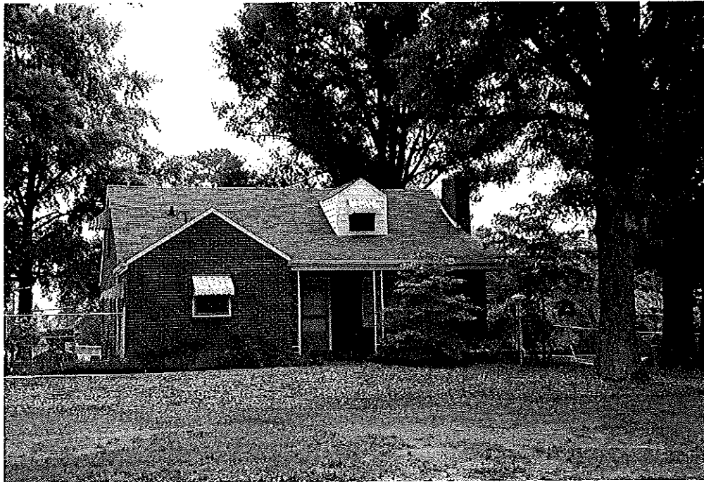
Property 17. House, 1953, 3531 Thomasville Road (NC 109), Forsyth County
