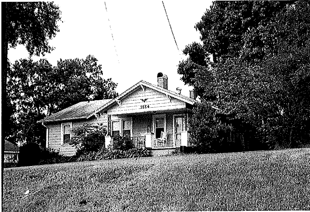
Property 29. House, 1930, 3554 Thomasville Road (NC 109), Forsyth County
