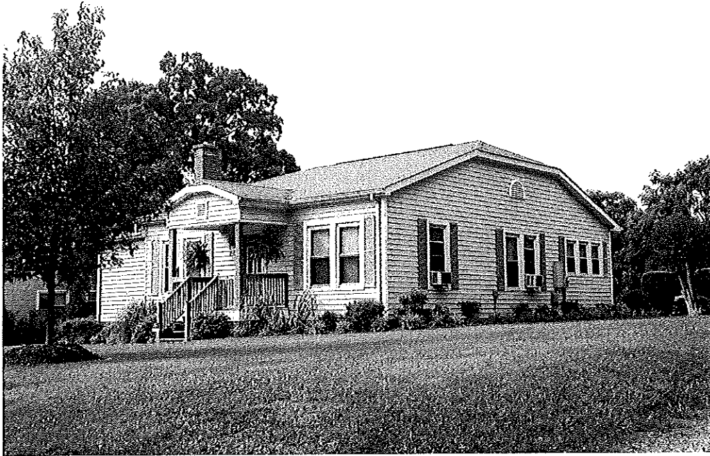
Property 27. House, 1928, 3540 Thomasville Road (NC 109), Forsyth County
