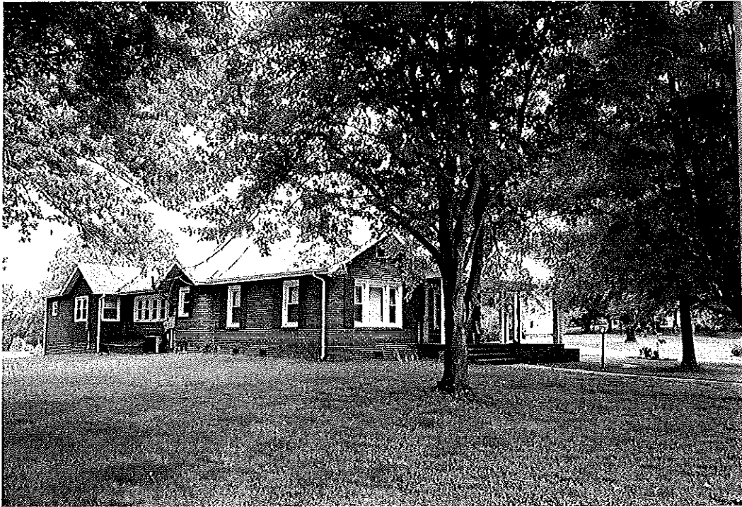
Property 57. House, 1925, 4313 Thomasville Road (NC 109), Forsyth County
