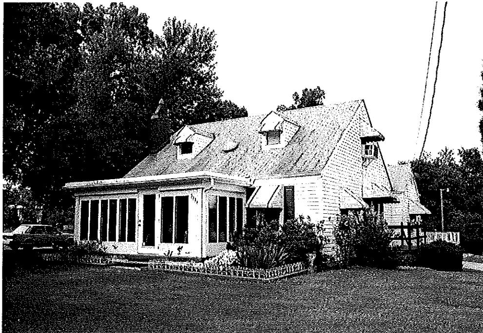
Property 26. House, 1938, 3506 Thomasville Road (NC 109), Forsyth County
