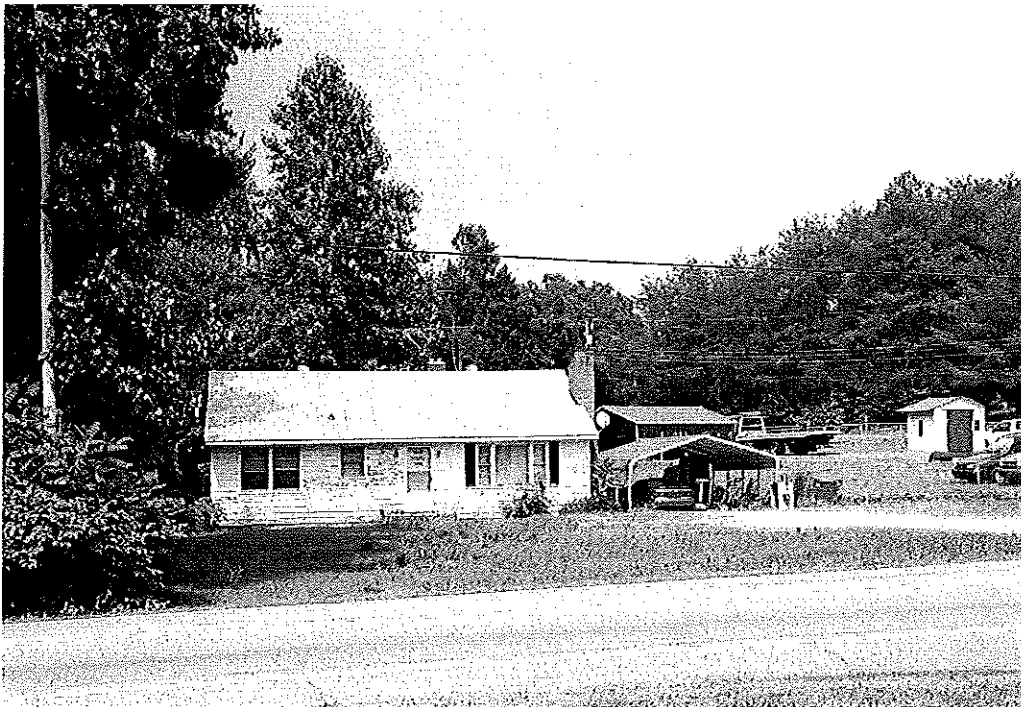
Property 66. House, 1955, 4391 Thomasville Road (NC 109), Forsyth County
