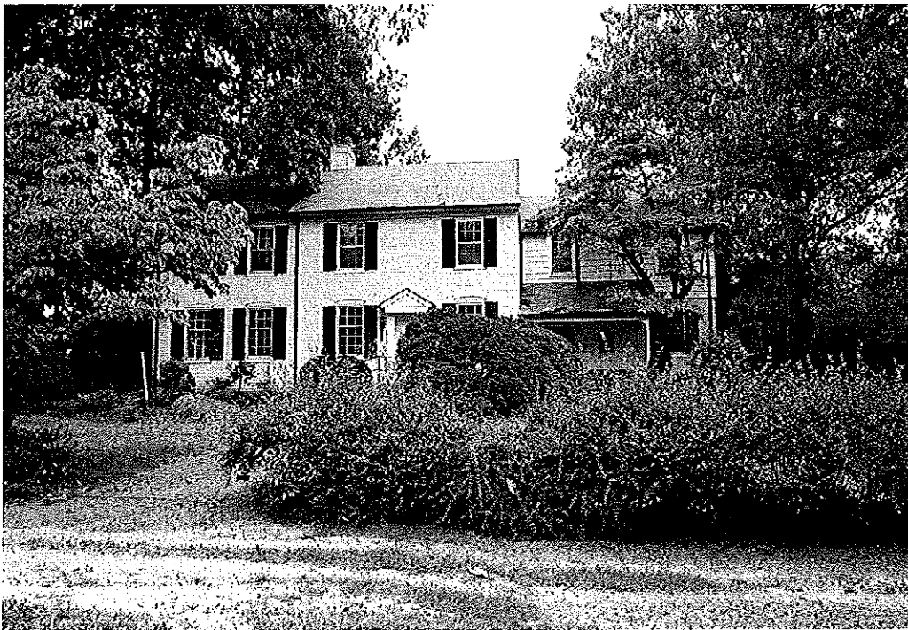
Property 86. Gray Swain House, 1952, 4175 Thomasville Road (NC 109), Forsyth County
