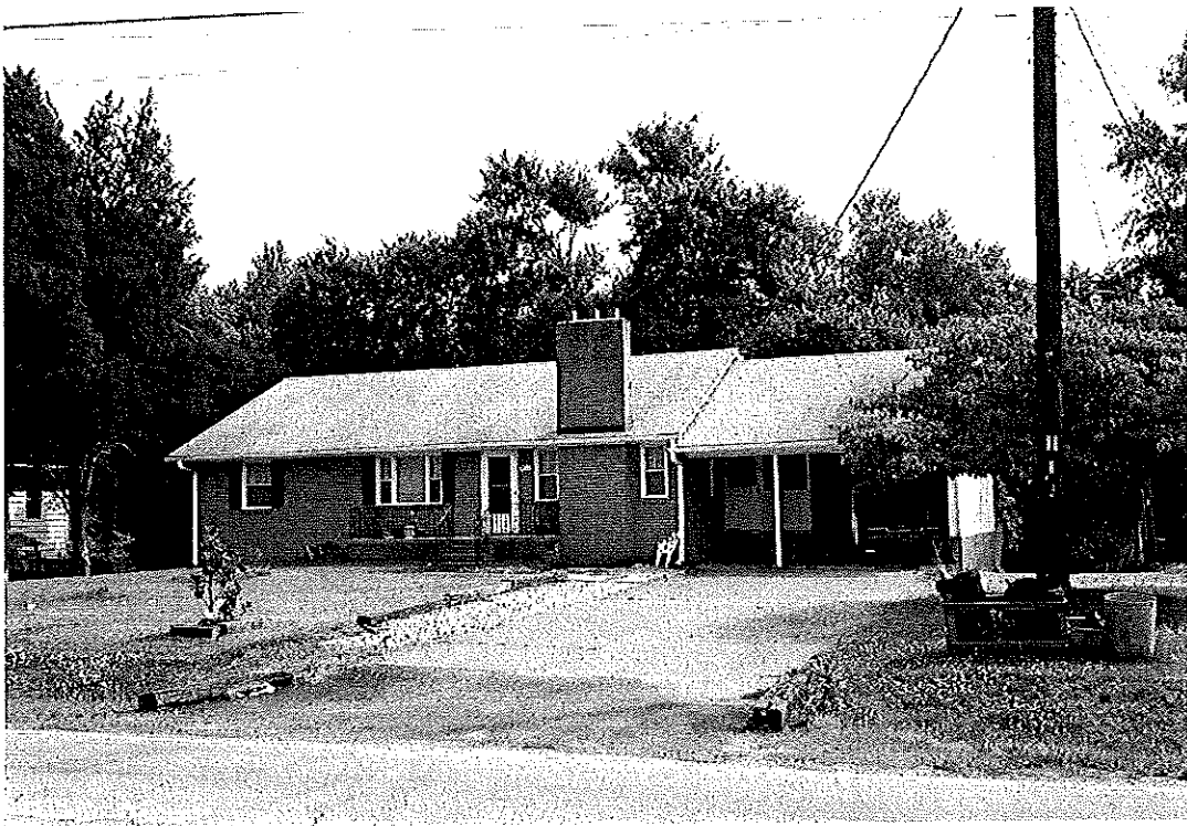
Property 32. House, 1958, 3633 Thomasville Road (NC 109), Forsyth County
