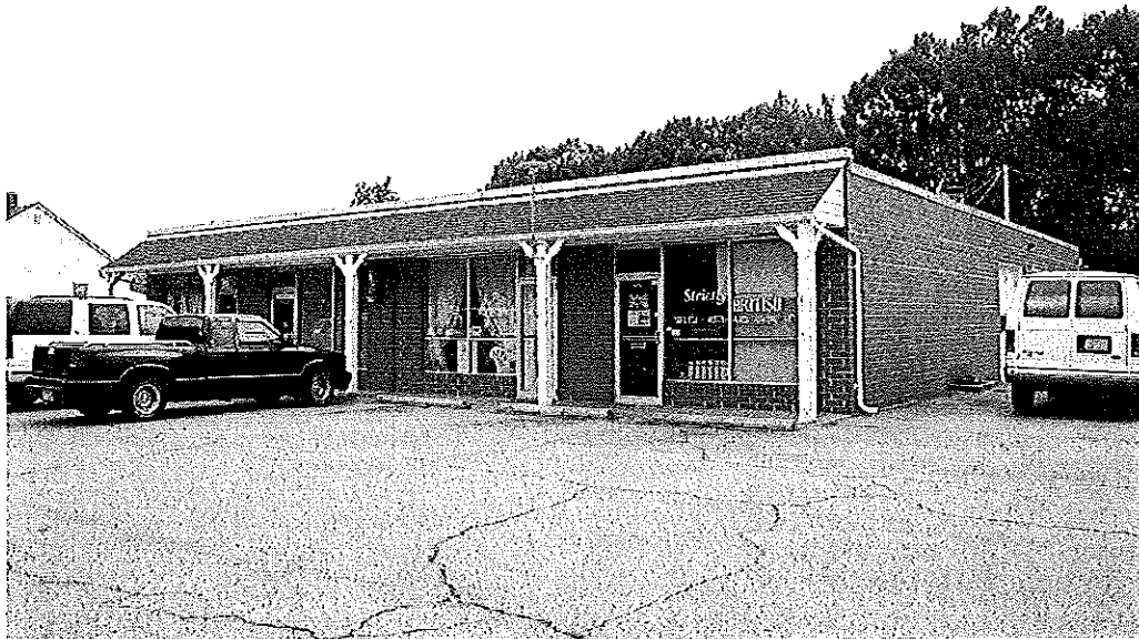
Property 64. Commercial Building, circa 1970, 4352-54-56-58 Thomasville Road (NC 109), Forsyth County
