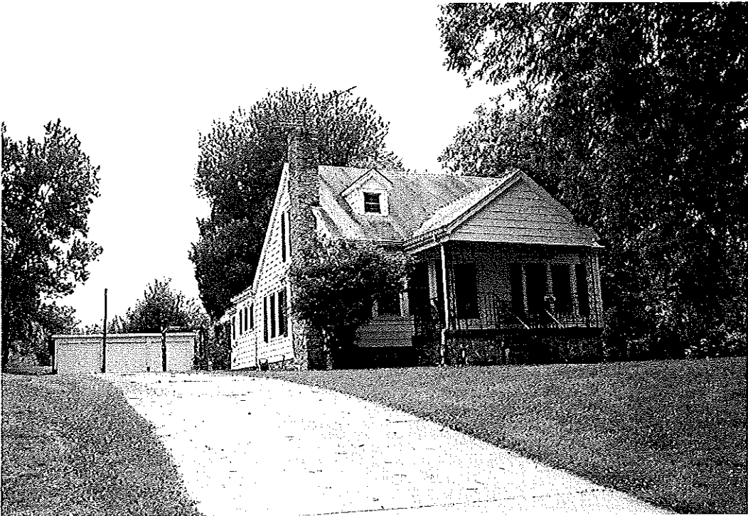
Property 48. House, 1938, 4018 Thomasville Road (NC 109), Forsyth County
