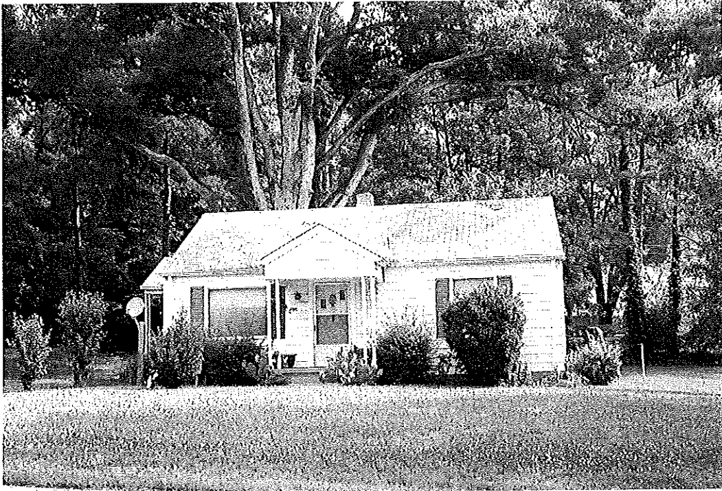
Property 36. House, 1950, 3725 Thomasville Road (NC 109), Forsyth County
