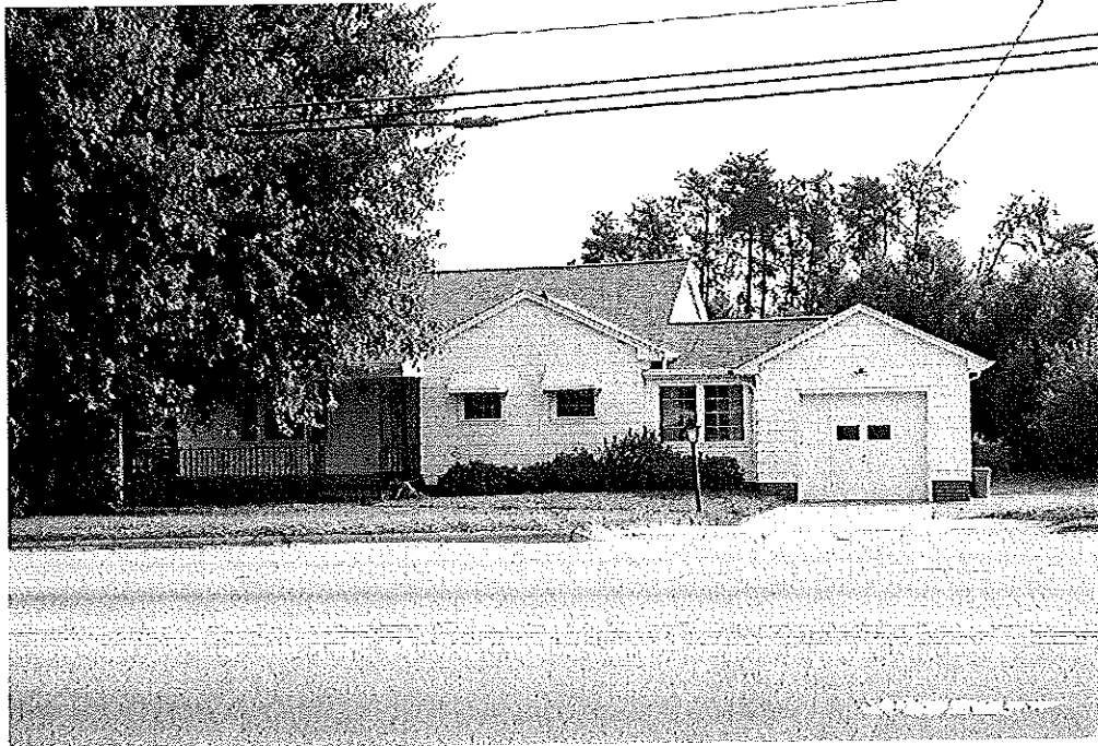
Property 1. House, 1953, 3207 Thomasville Road (NC 109), Forsyth County
