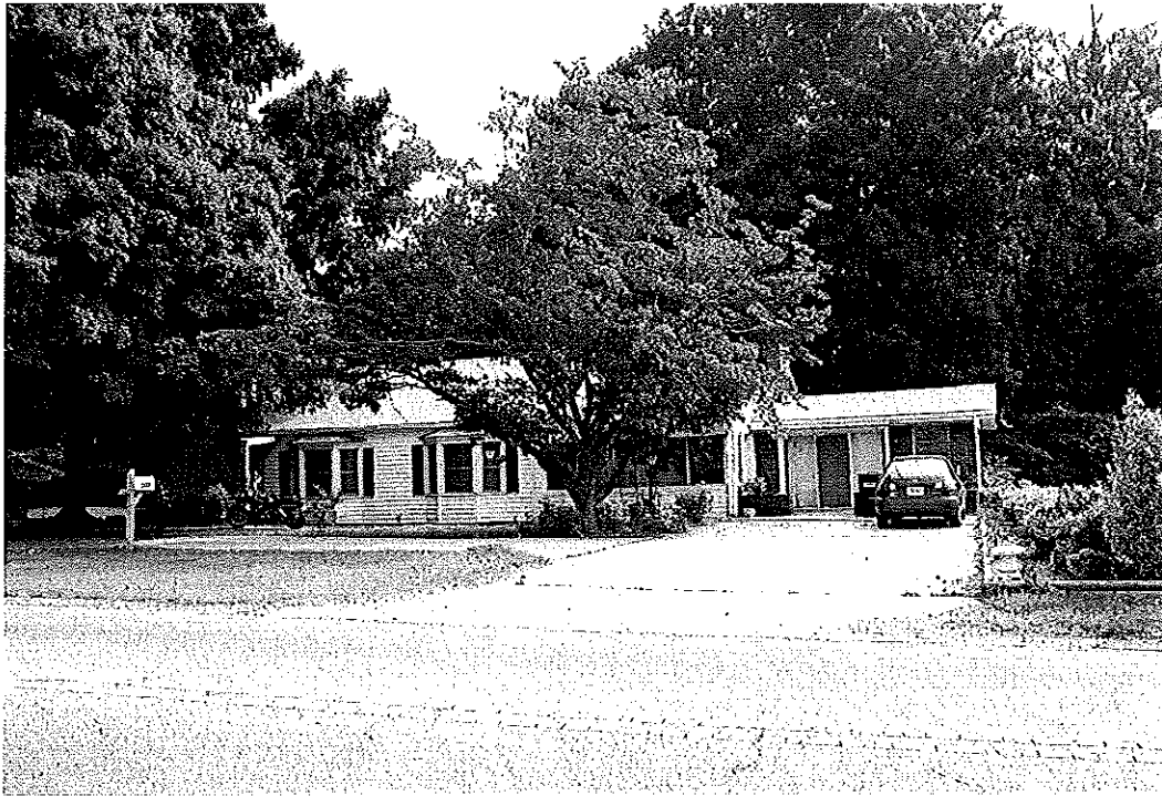
Property 21. House, 1948, 3583 Thomasville Road (NC 109), Forsyth County
