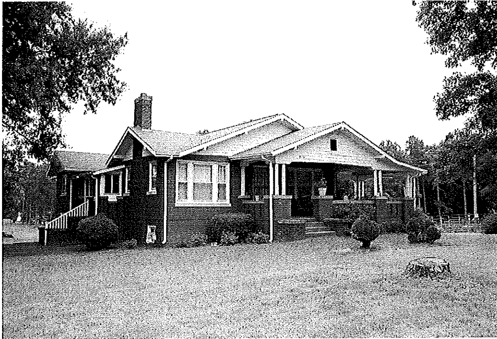
Hine House, North and East Elevations
