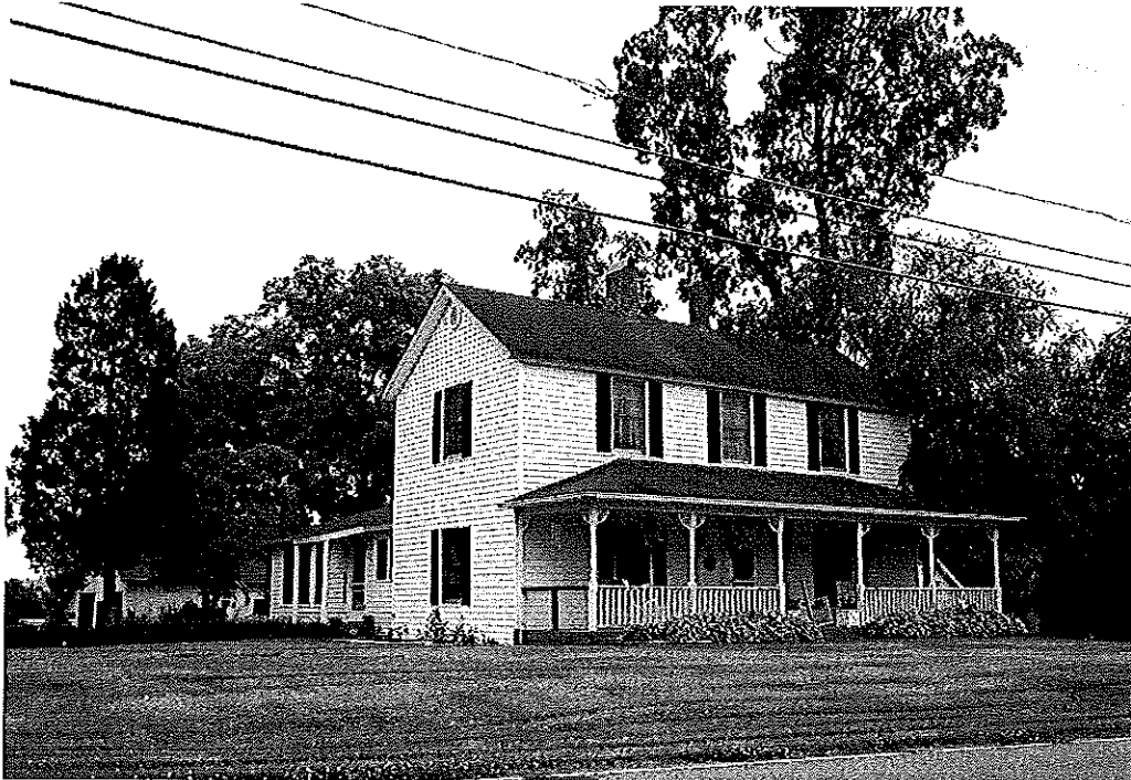
Property 52. House, 1896, 2535 Union Cross Road, Forsyth County
