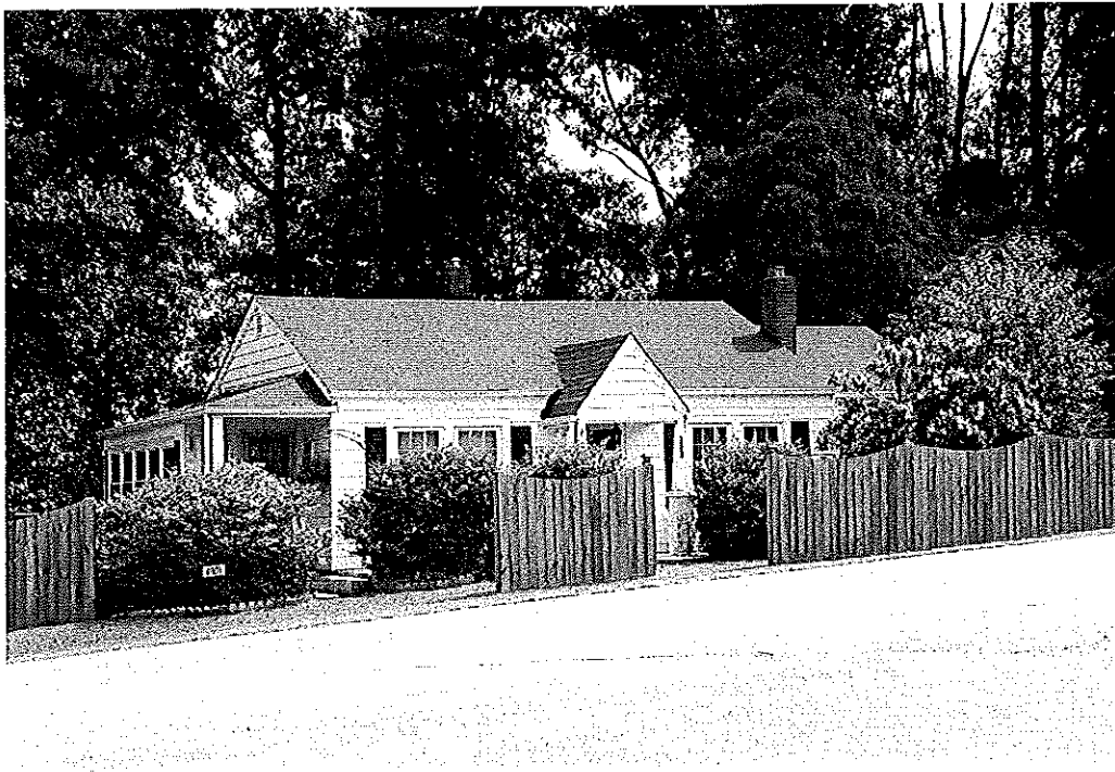
Property 38. House, 1932, 4001 Thomasville Road (NC 109), Forsyth County
