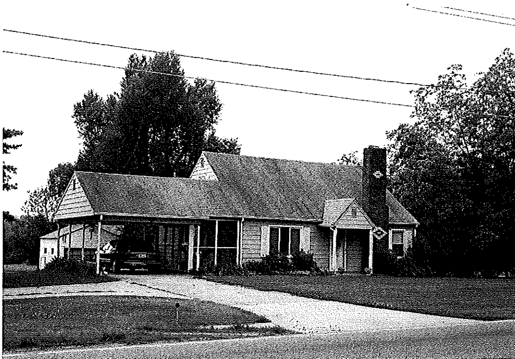
Property 60. House, 1938, 4310 Thomasville Road (NC 109), Forsyth County
