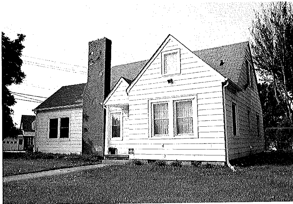
Property 2. House, 1948, 3210 Thomasville Road (NC 109), Forsyth County
