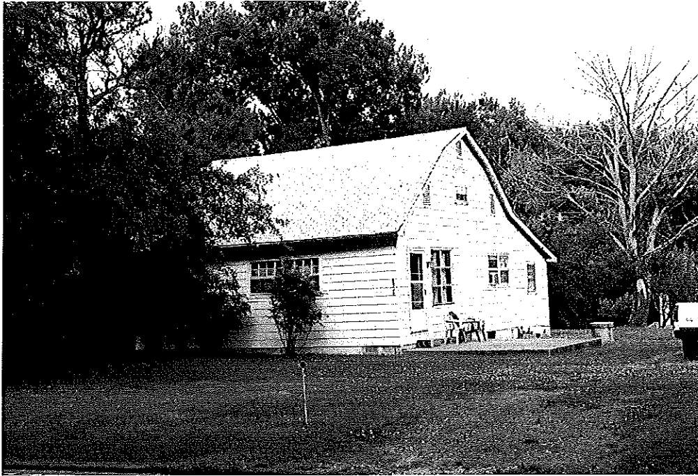
Property 73. Barn/House, circa 1920, 6904 Thomasville Road (NC 109), Davidson County
