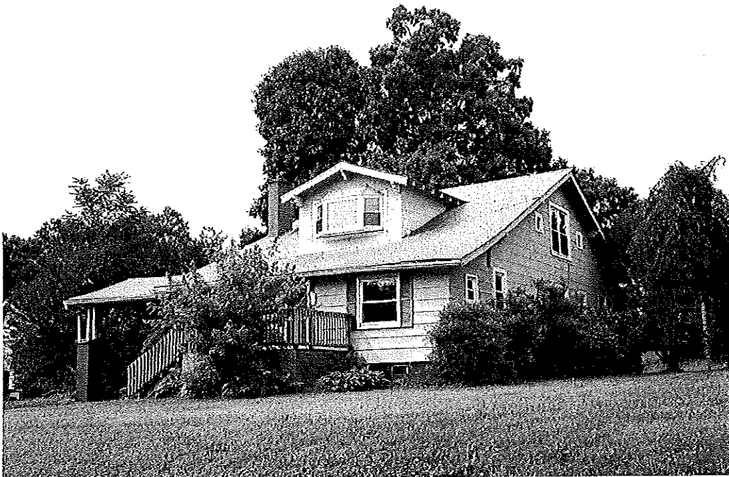
Property 28. House, 1926, 3548 Thomasville Road (NC 109), Forsyth County
