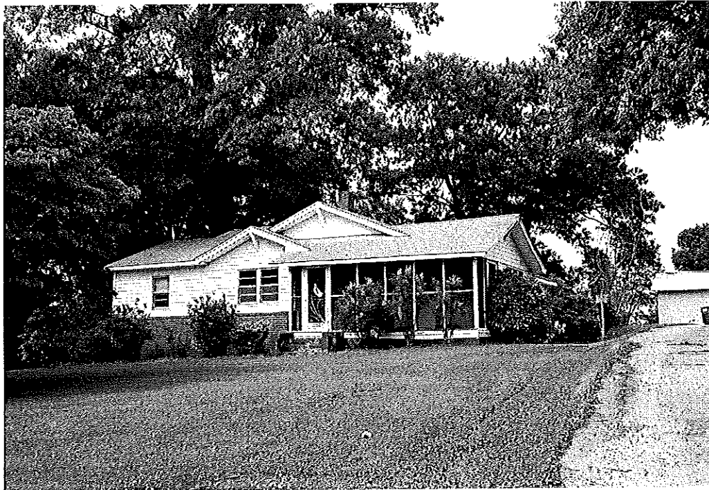
Property 30. House, 1925, 3562 Thomasville Road (NC 109), Forsyth County
