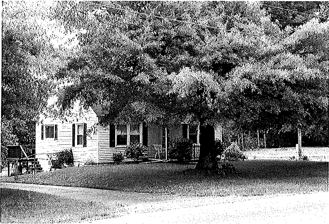
Property 61. House, 1948, 4306 Thomasville Road (NC 109), Forsyth County
