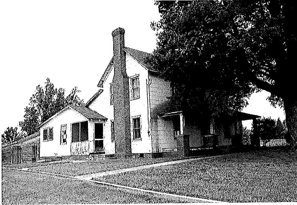
Property 109. House, circa 1900, west side Thomasville Road (NC 109) approximately 750 feet south of its intersection with Jesse Green Road (SR 1753), Davidson County
