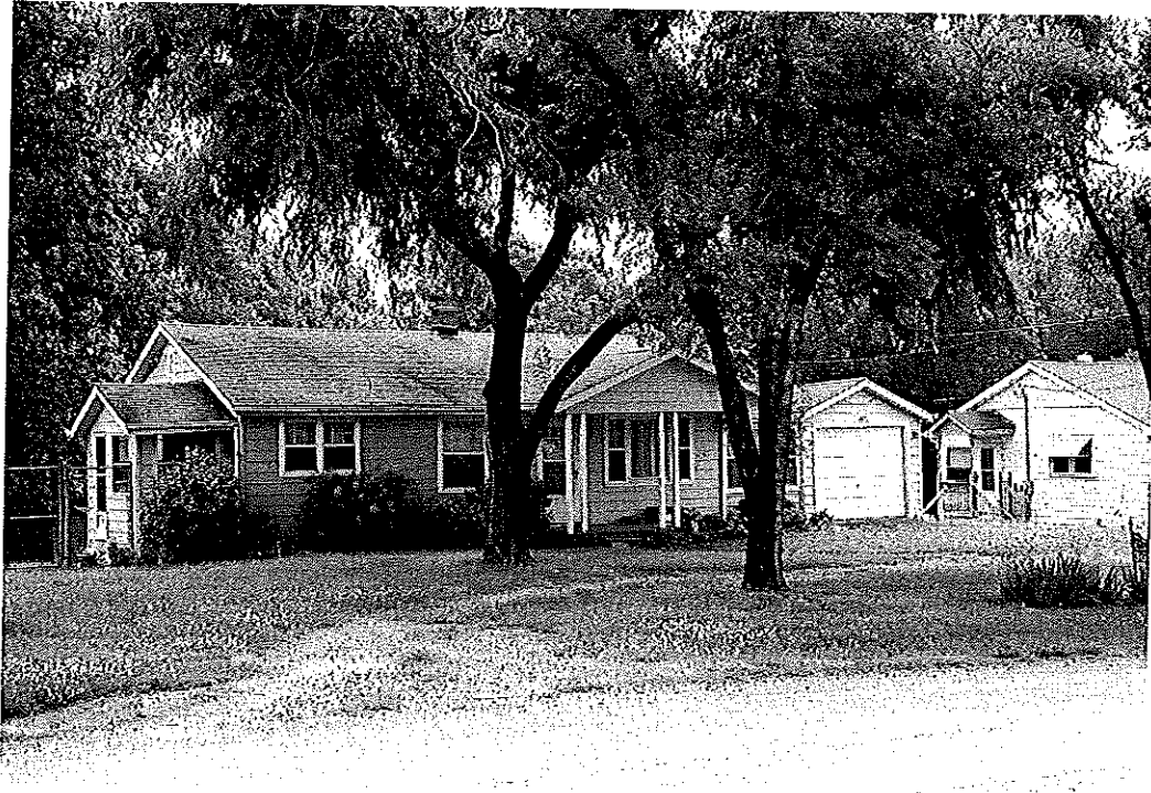
Property 23. House, 1950, 3621 Thomasville Road (NC 109), Forsyth County
