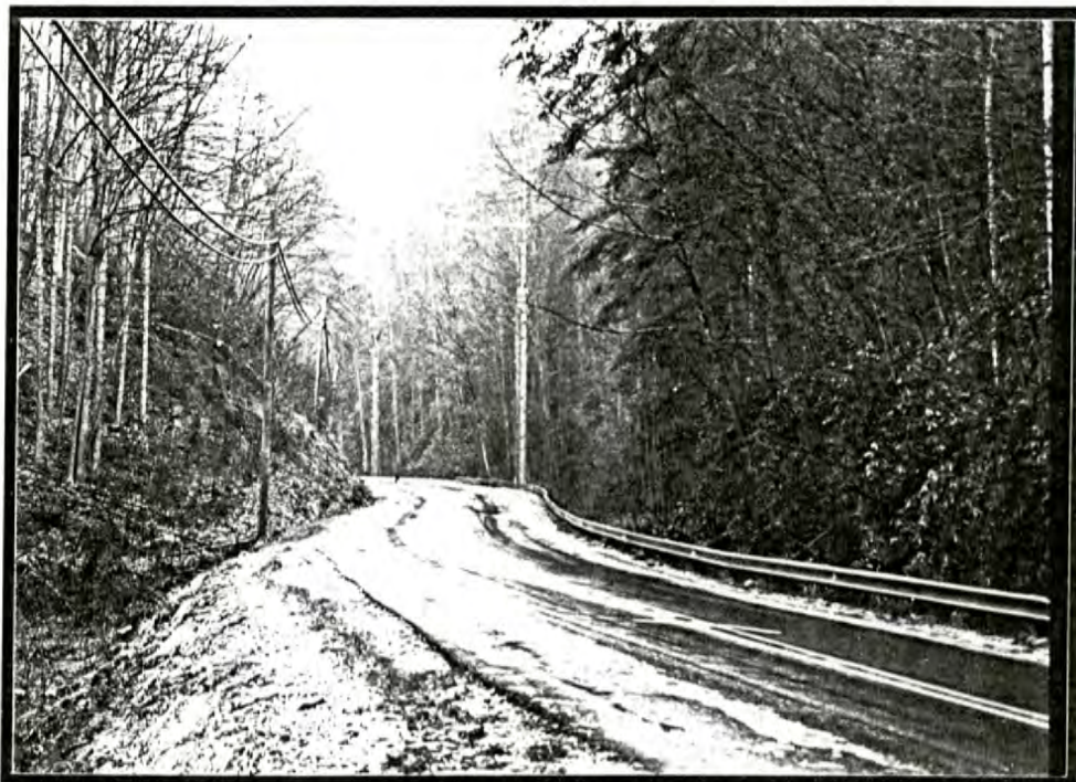
Plate VI.2 US 221 ALONG HICKORY BOTTOM BRANCH NORTH OF TURKEY COVE, FACING NORTH
