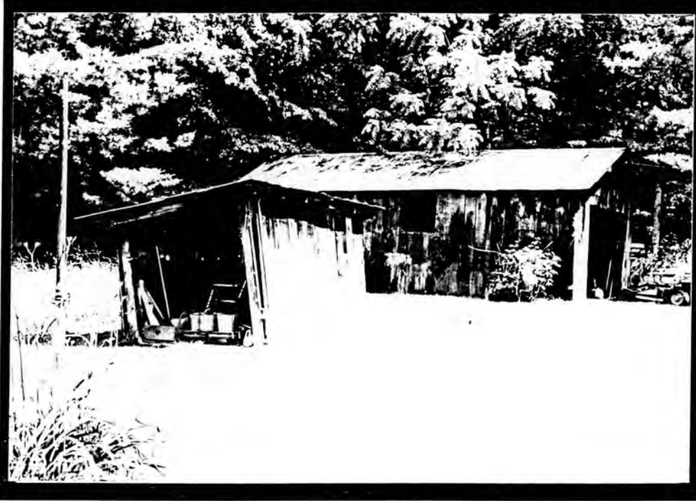
Plate IX.45 SOUTH AND WEST ELEVATIONS OF SHED AND GARAGE TO REAR OF CONNELLY-PHILLIPS HOUSE (#25)
