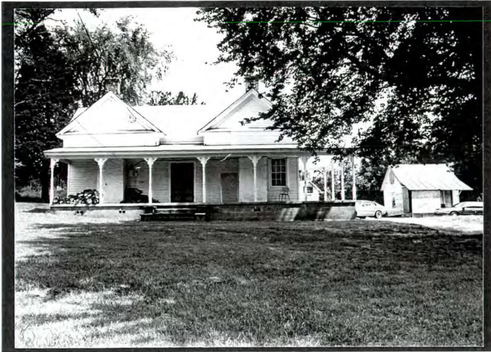
PLATE VI.36 House (#72) - south front elevation of house at right, outbuilding at right, shed visible behind porch at right center
