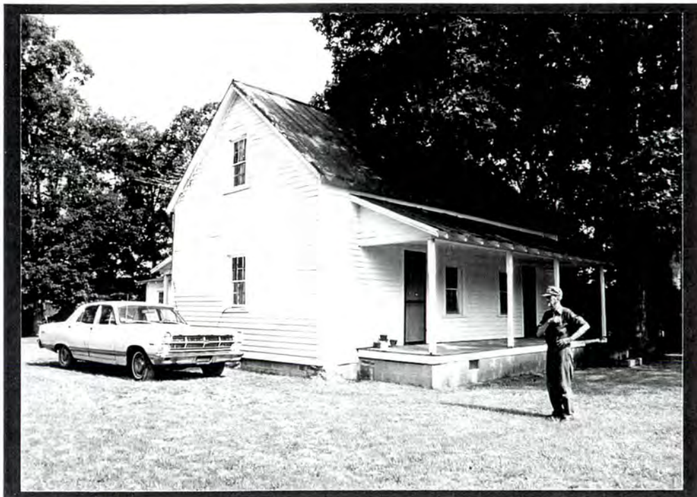
PLATE V.2 House (#82), east front and south side elevations
