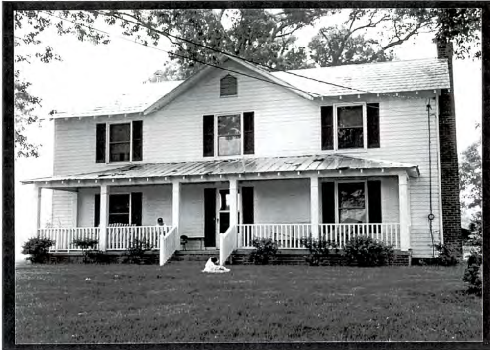
PLATE VI.59 Walker-Long-Shotwell Farmstead (#56) - southeast front and northeast side elevations
