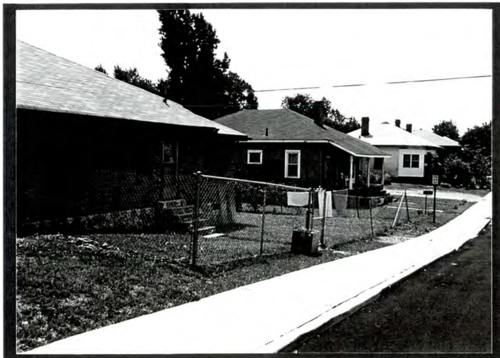
PLATE VI.50 Baker-Ca-Vel Mill Village and Mill (#31) - east side of Sunset Street, facing southeast from Kerr Drive
