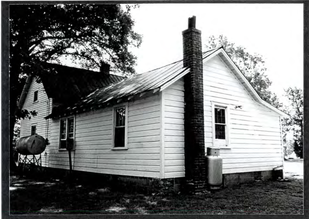
PLATE VI.69 House (#82) - west rear and north side elevations
