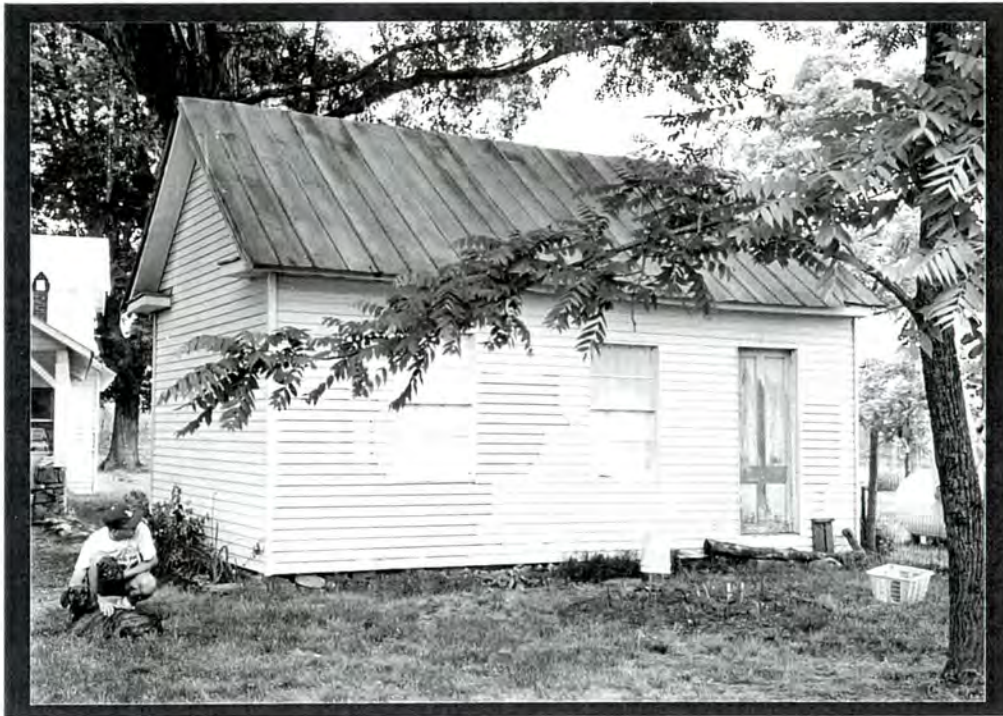
PLATE VI.61 Former dining room and kitchen to west of Walker-Long-Shotwell farmhouse (#56)
