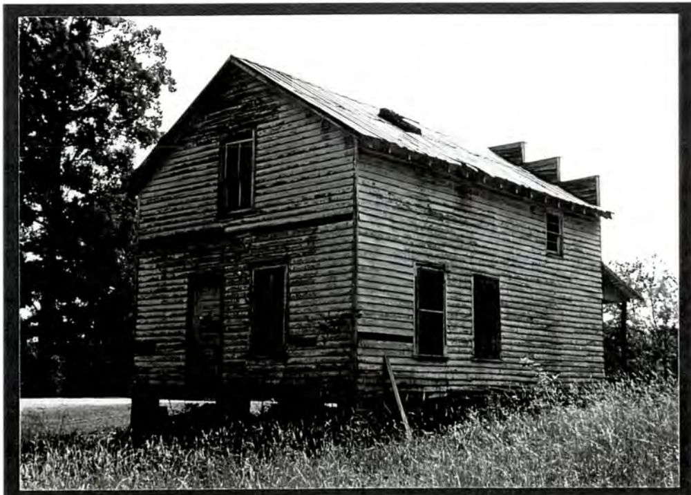
PLATE VI.71 Woody-Jones Store (#92) - south side and west rear elevations
