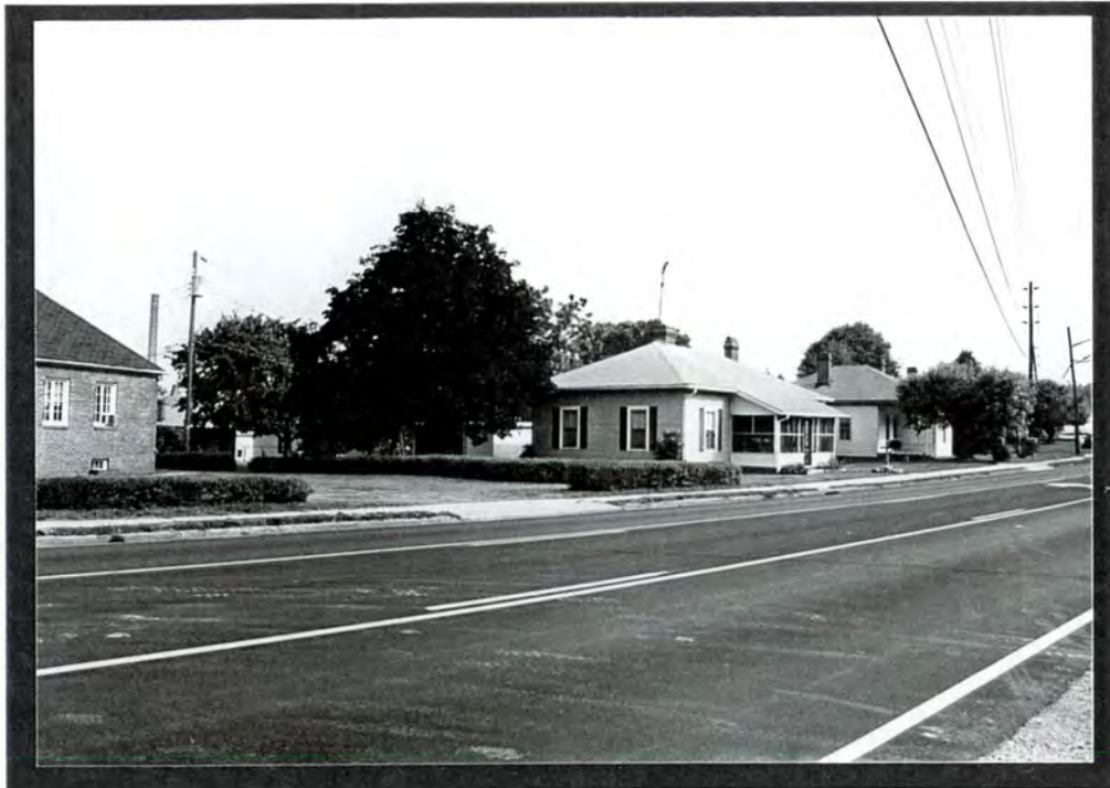
PLATE VI.44 Baker-Ca-Vel Mill Village and Mill (#31) - east front and south side elevations of Type Three house at 1707 North Main Street
