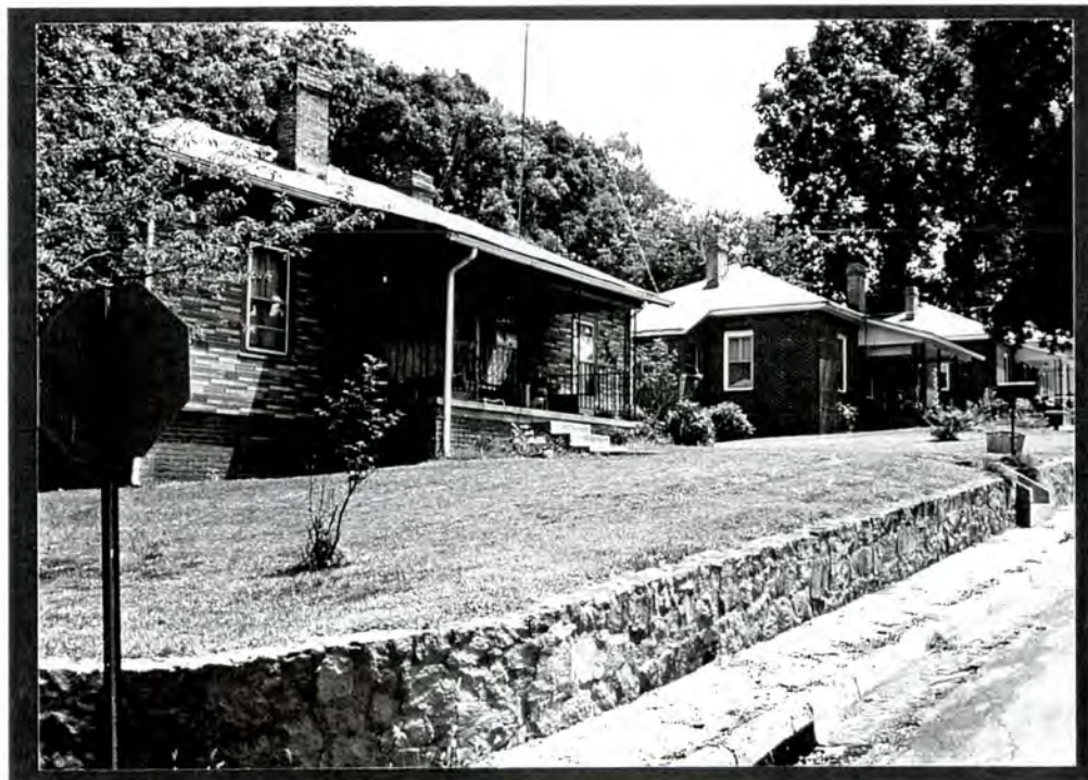
PLATE VI.48 Baker-Ca-Vel Mill Village and Mill (#31) - north side of 200 block of Hicks Circle, facing northeast from bend in street
