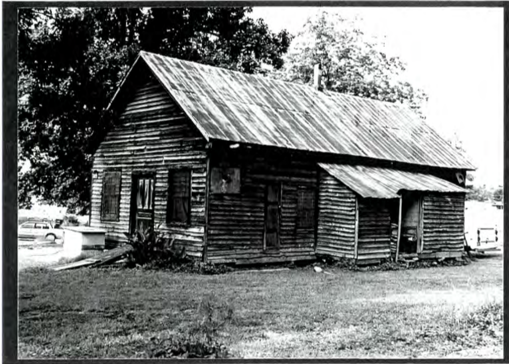
PLATE VI.56 House (#47) - west and south elevations
