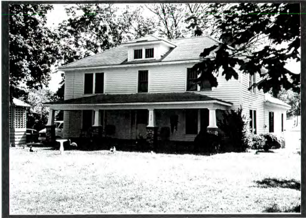
PLATE VI.38 Walker Sisters House (#30) - west front and south side elevations
