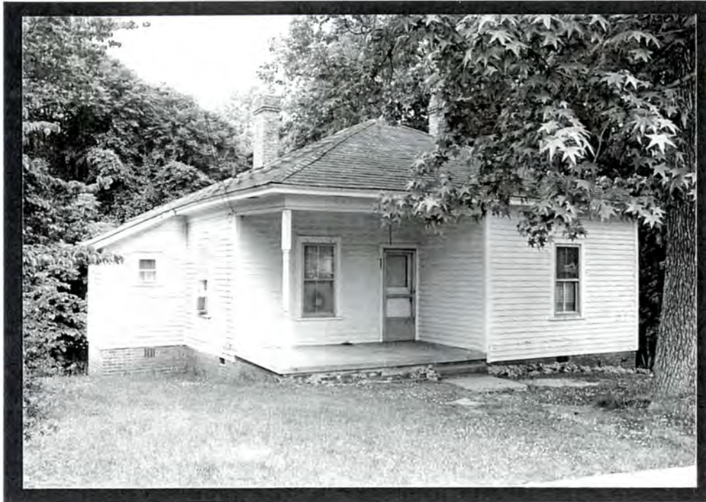
PLATE VI.42 Baker-Ca-Vel Mill Village and Mill (#31) - east front and south side elevations of Type One house at 1817 Hicks Circle
