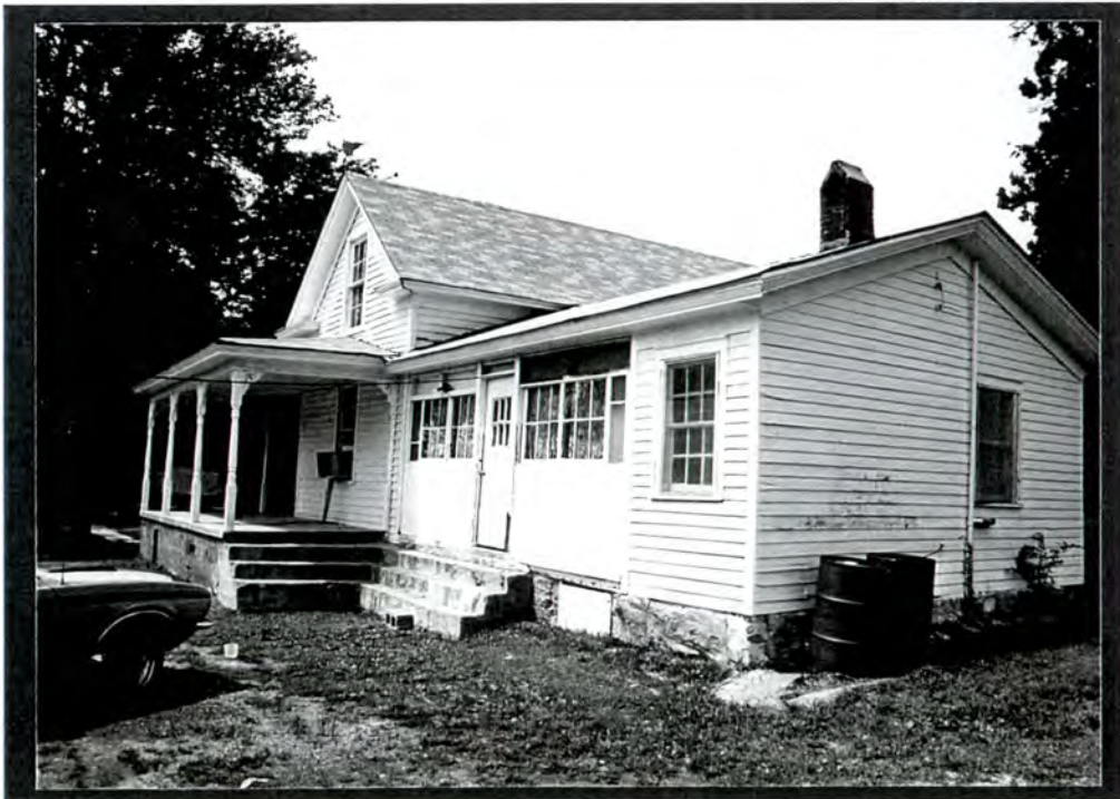
PLATE VI.35 House (#72) - east side and north rear elevations
