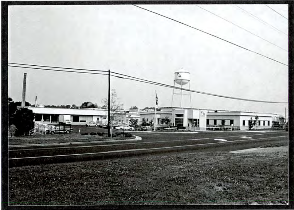
PLATE VI.41 Baker-Ca-Vel Mill Village and Mill (#31) - south and east elevations of Ca-Vel Mill, 1803 North Main Street
