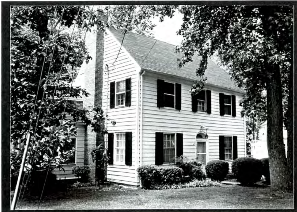
PLATE VI.16 Ca-Vel Executive Village Historic District (#32-#40) - 1869 Executive Lane (#35), east front and south side elevations
