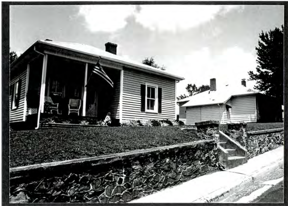
PLATE VI.49 Baker-Ca-Vel Mill Village and Mill (#31) - west side of 1800 block of Hicks Circle, facing northwest from Kerr Drive
