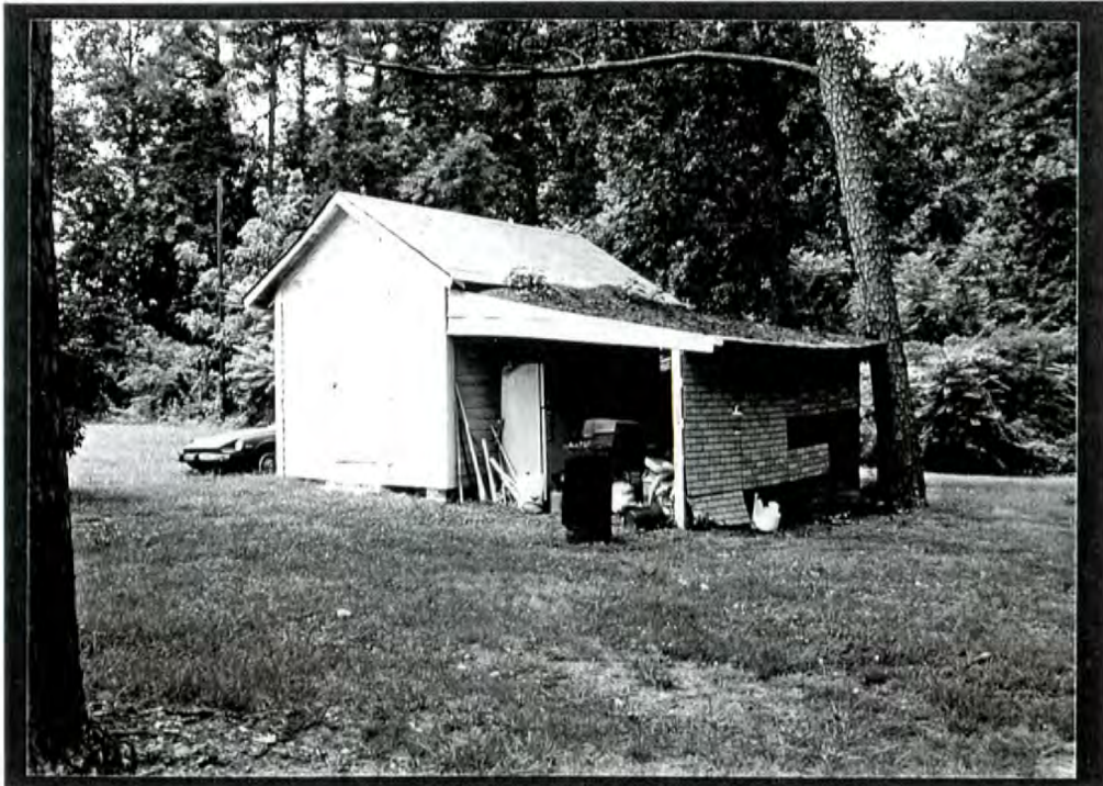
PLATE VI.10 Will Walker House (#29), shed to rear of west elevation
