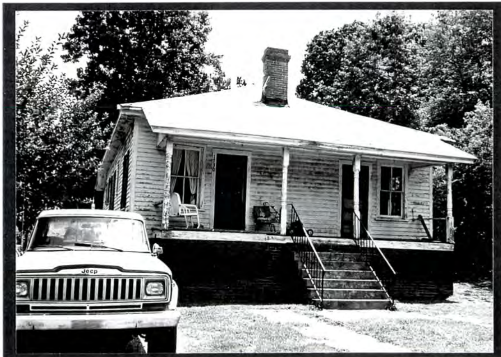
PLATE VI.43 Baker-Ca-Vel Mill Village and Mill (#31) - west front and north side elevations of Type Two house at 1128- 1130 Turner Street
