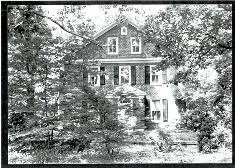
PLATE VI.24 Main house of the John H. Merritt Homeplace (#84), east front elevation
