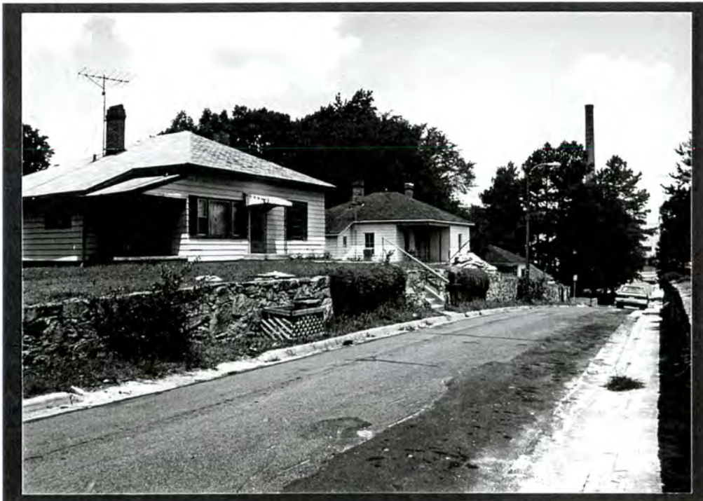
PLATE VI.52 Baker-Ca-Vel Mill Village and Mill (#31) - west side of Wall Street, facing northwest towards Kerr Drive
