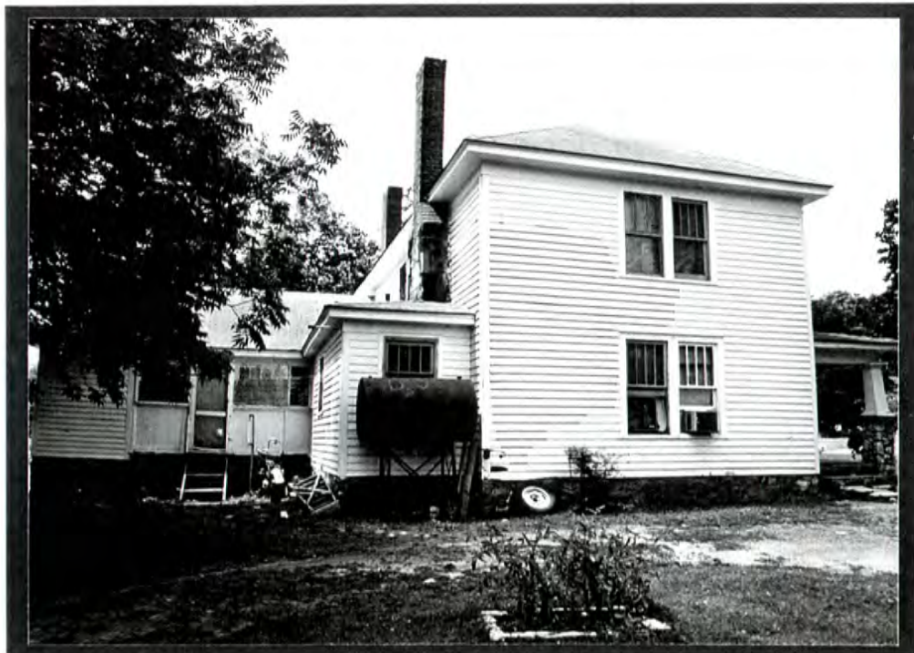
PLATE VI.39 Walker Sisters House (#30) - north side and east rear elevations
