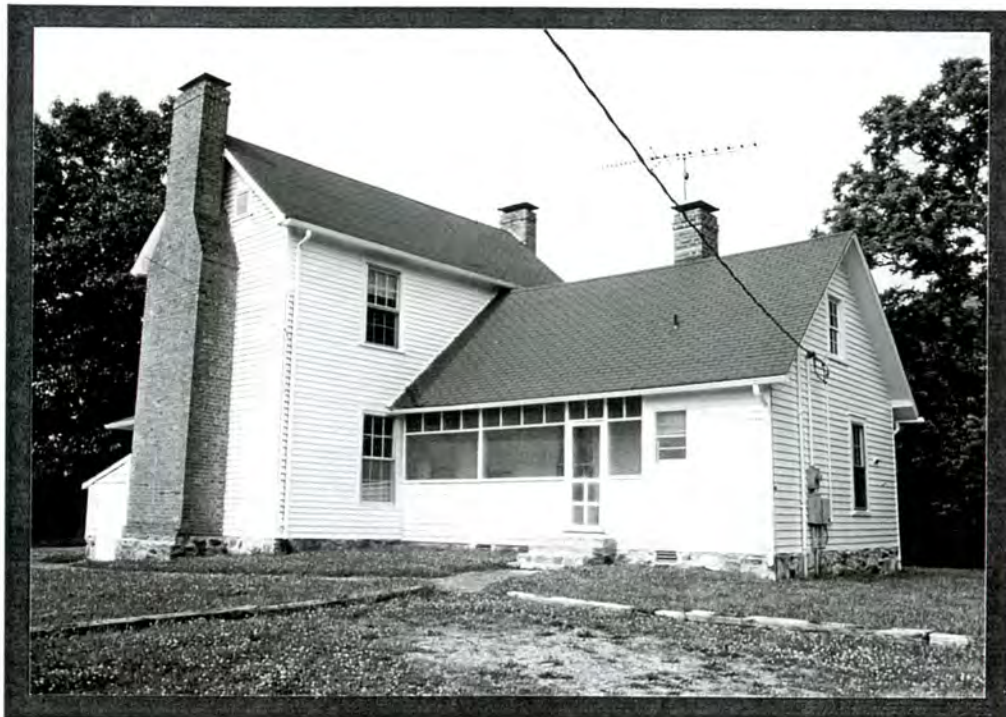
PLATE VI.2 Holloway-Jones-Day House (#86), east side and north rear elevations
