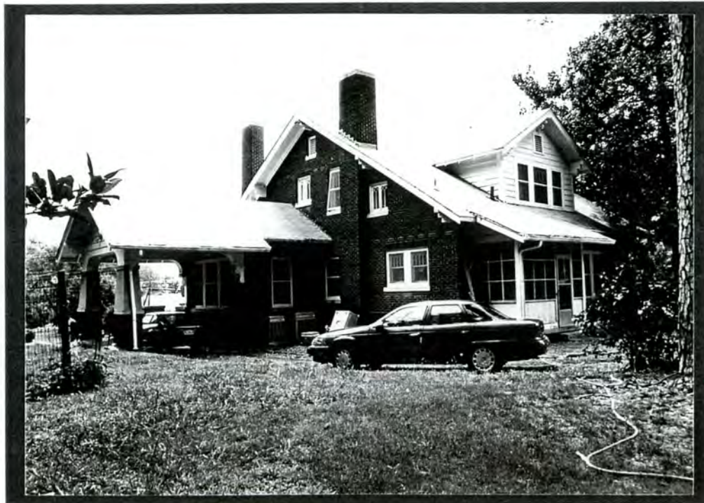
PLATE VI.8 Will Walker House (#29), west rear and north side elevations
