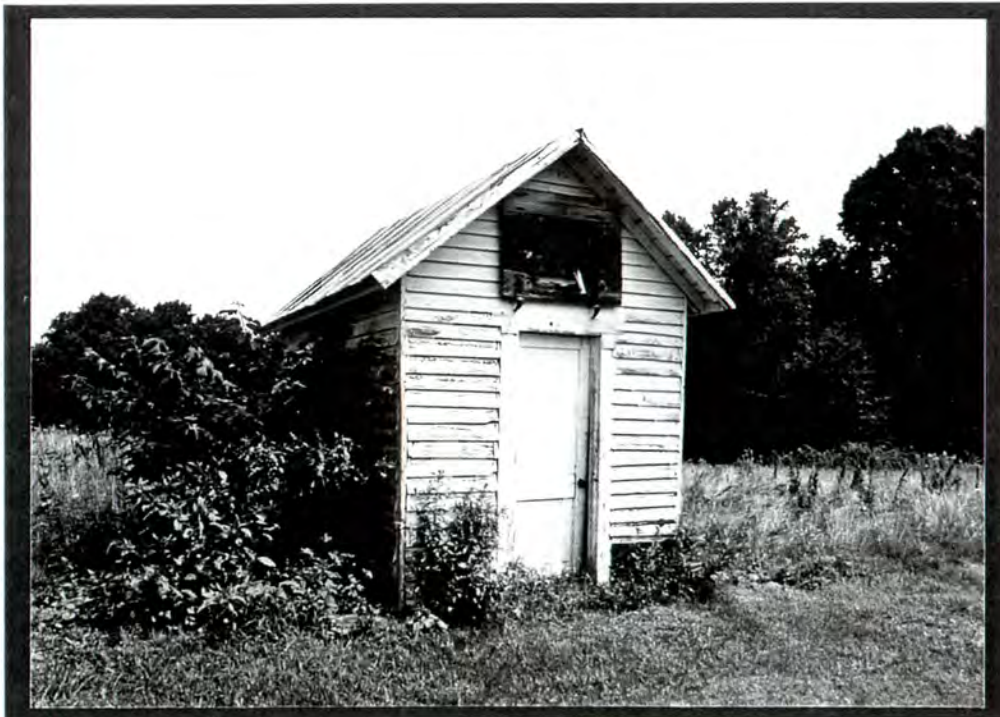
PLATE VI.37 House (#72) - south front elevation of shed
