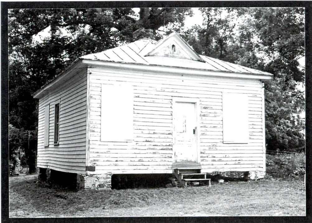
PLATE VI.31 Doctor's Office of the John H. Merritt Homeplace (#84), west front and north side elevation
