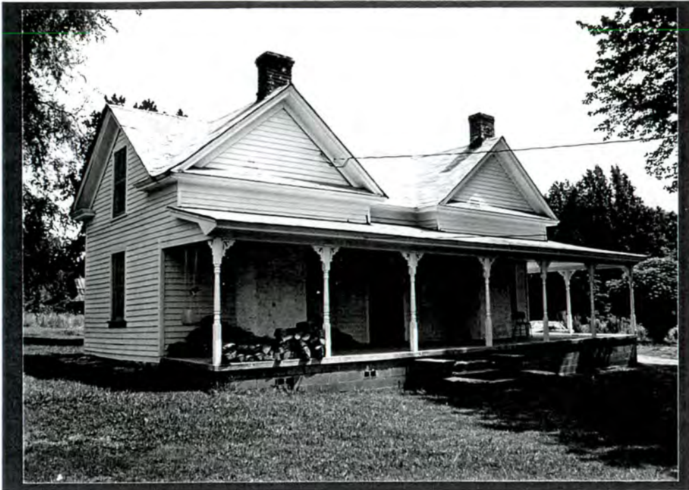
PLATE VI.34 House (#72) - south front and west side elevations
