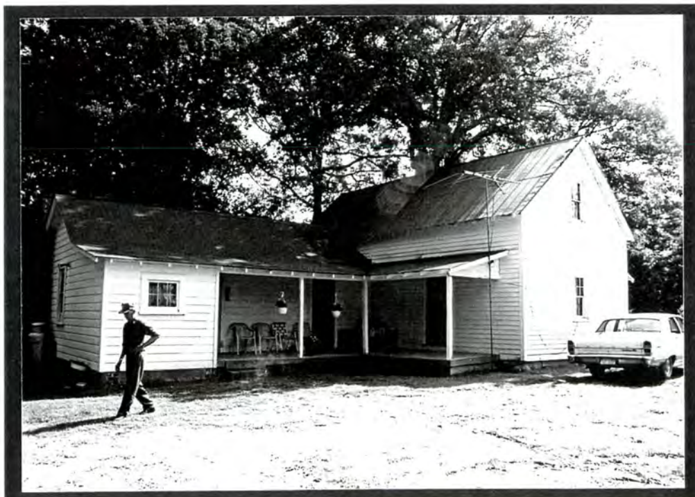
PLATE VI.68 House (#82) - south side and west rear elevations
