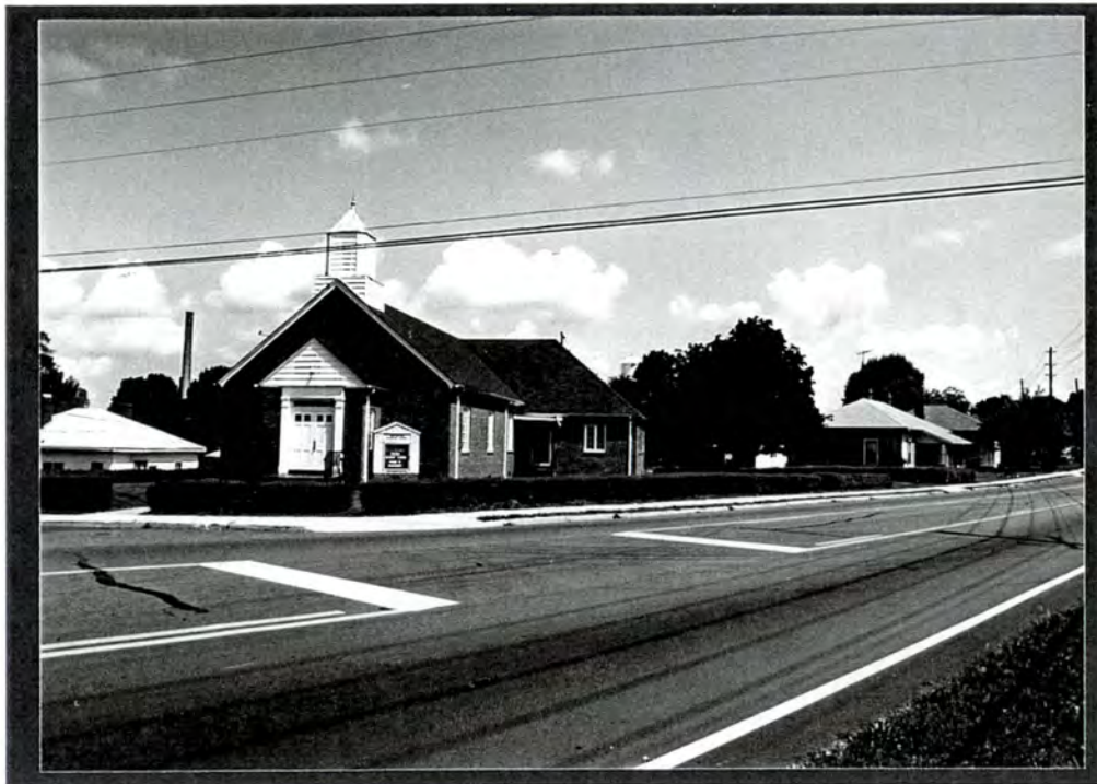
PLATE VI.45 Baker-Ca-Vel Mill Village and Mill (#31) - west side of North Main Street facing north from Edgewood Street
