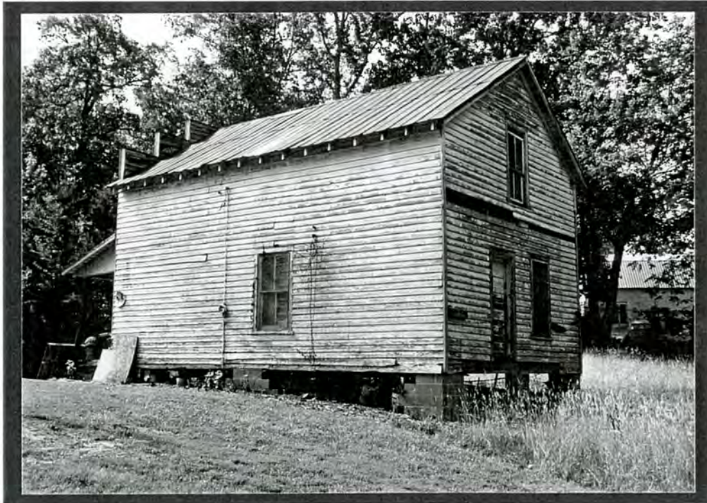
PLATE VI.72 Woody-Jones Store (#92) - west rear and north side elevations
