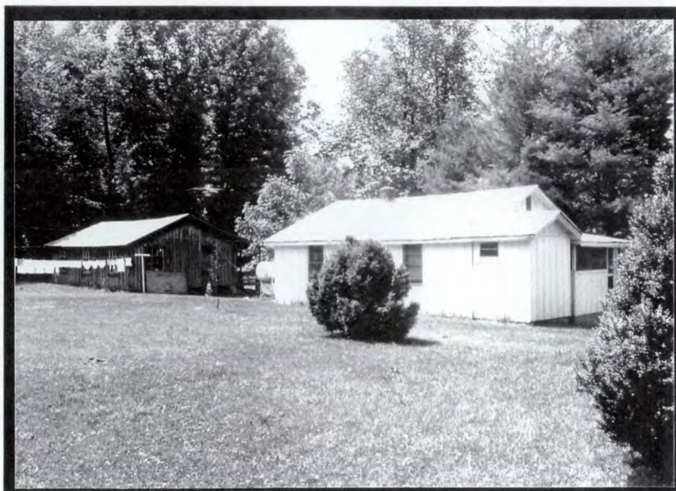
Plate IX.44 NORTH AND WEST ELEVATIONS OF WORKERS' HOUSES TO SOUTHEAST OF CONNELLY-PHILLIPS HOUSE (#25)
