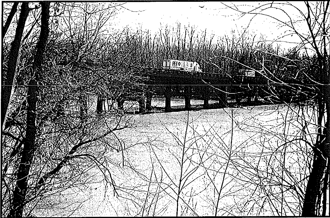
Plate 35. Looking southeast toward upstream elevation of I-85 bridge over the Yadkin.
