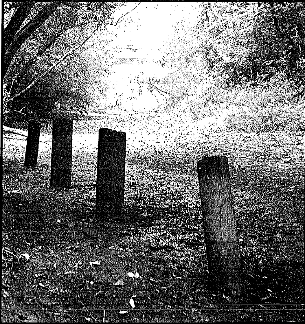
Plate 36. August 2004 photo of pole remnants alleged to represent ferry landing (view northwest with I-85 bridge in background). Note how outside poles lean in towards inner pair.
