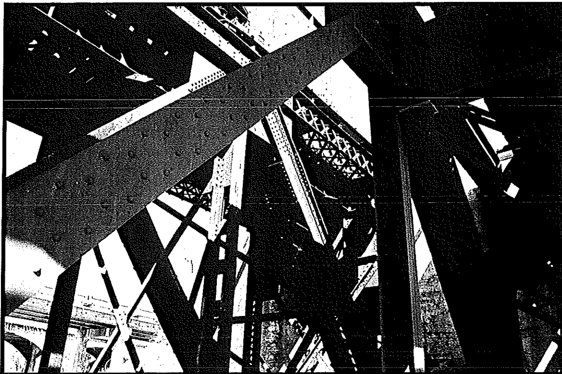
Plate 31. North Carolina Railroad Bridge No. 2 (1919) at left; Bridge No. 1 (1907) at right.
