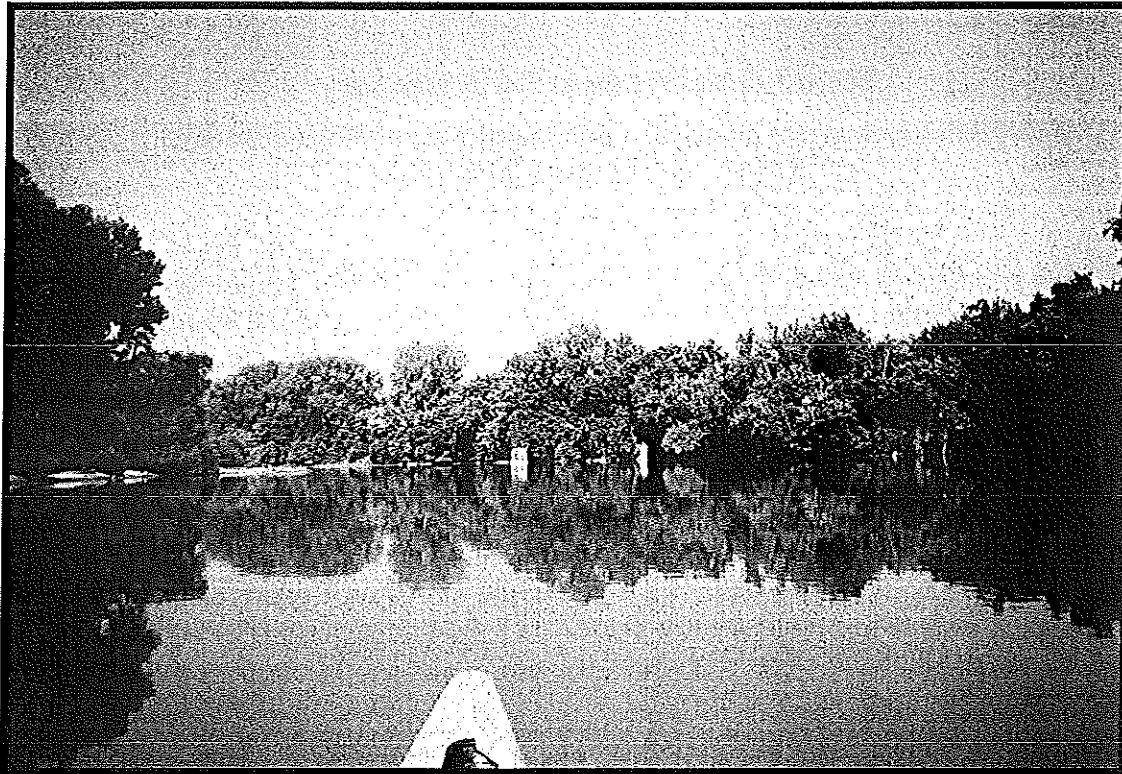
Plate 14. Looking upriver at piers of Beard's Bridge/Piedmont Toll Bridge.
