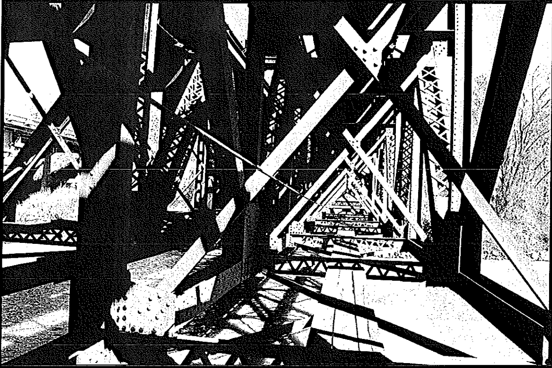
Plate 28. North Carolina Railroad Bridge No. 1 (1907) at right; Bridge No. 2 (1919) at left.
