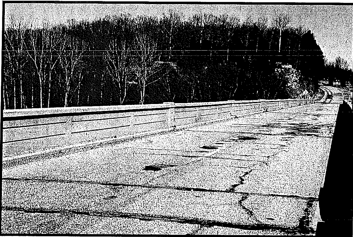
Plate 21. Looking northwest at parapet wall of Wilcox Bridge. York Hill in Davidson County in background.
