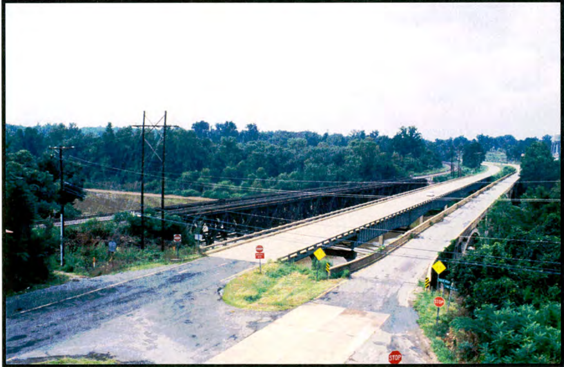
Plate 2. Highway and Railroad Bridges Over the Yadkin River. View South from York Hill in August 2004.
