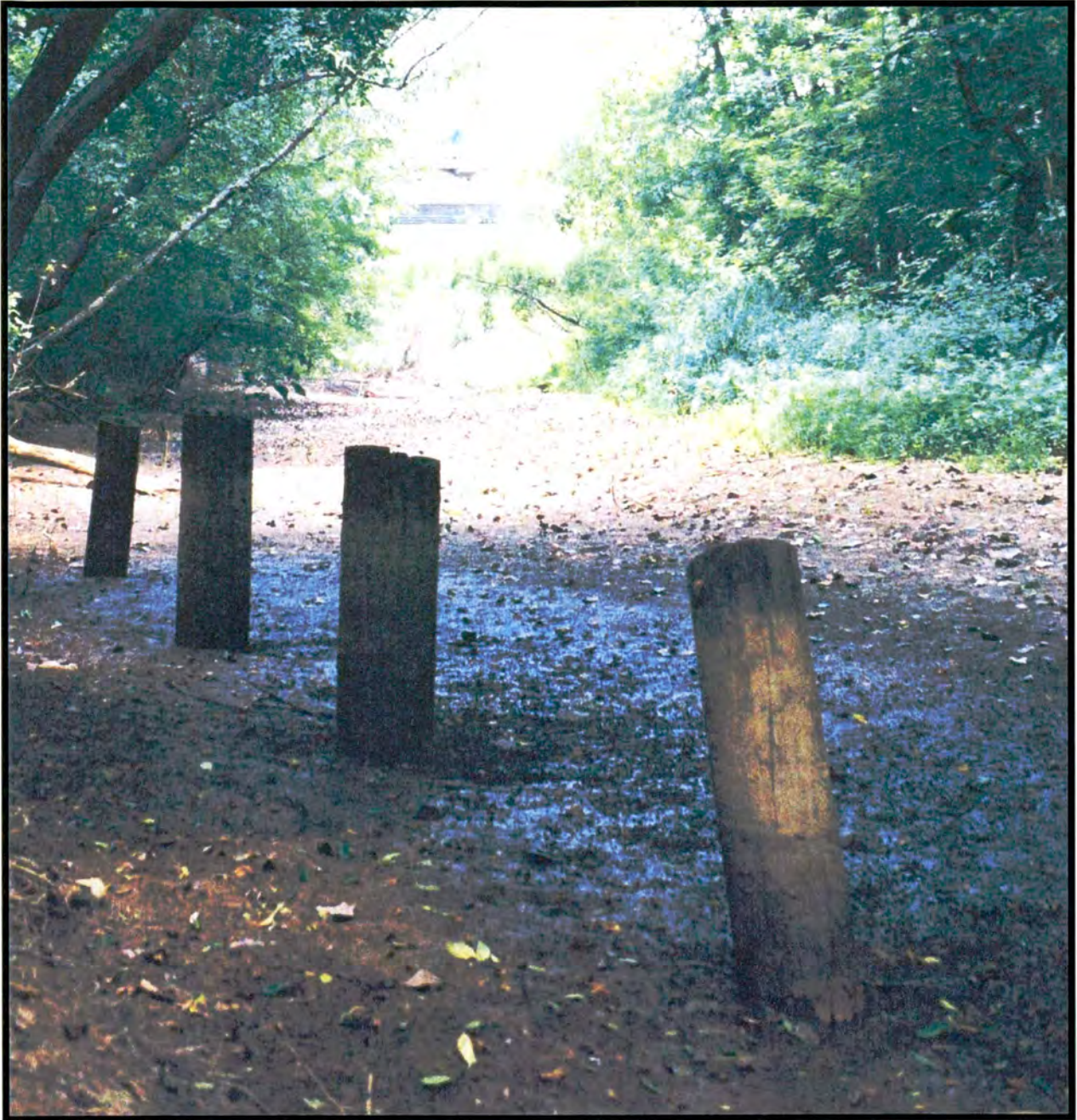
Plate 5. August 2004 Photo of Pole Remnants Alleged to Represent Ferry Landing (I-85 Bridge in Background). Note how outside poles lean in towards inner pair.
