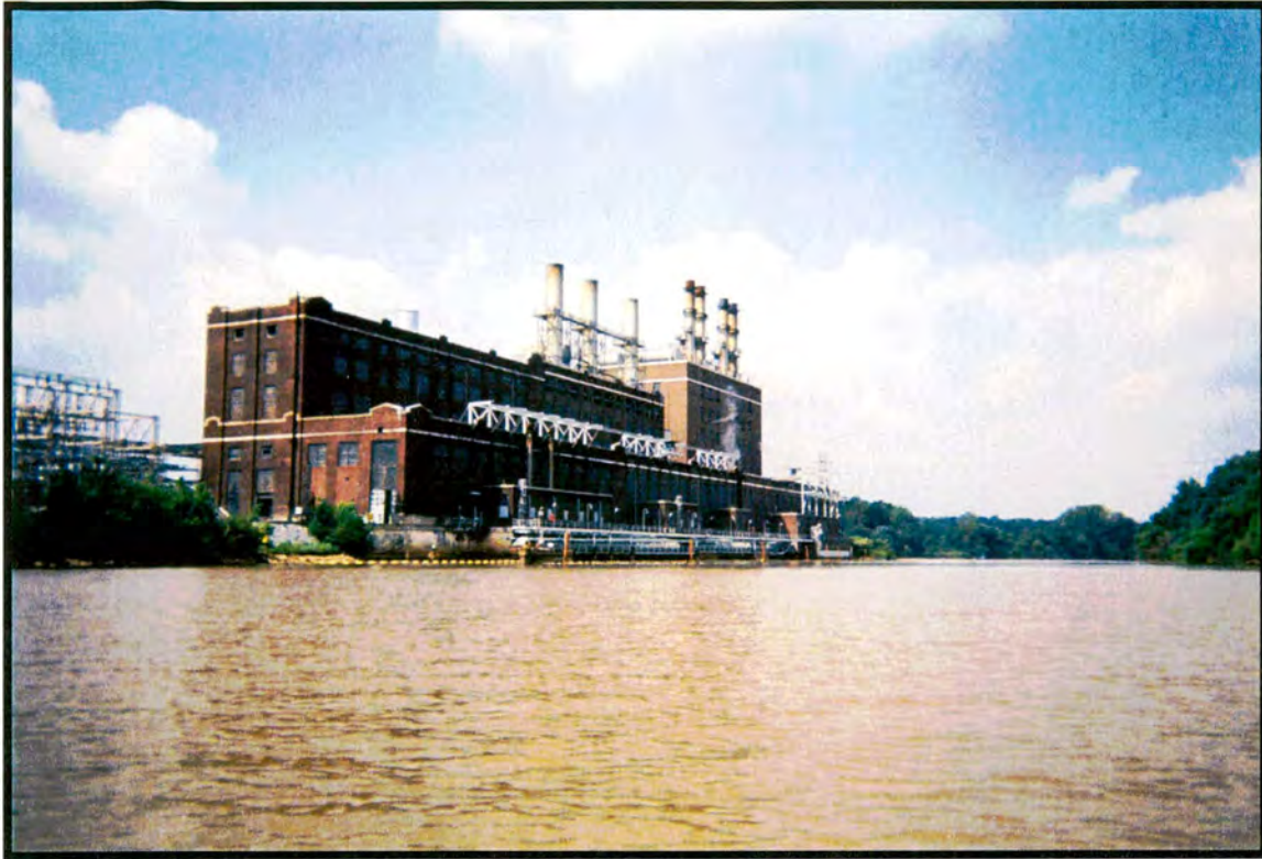
Plate 1. Buck Steam Plant on South Bank of Yadkin River. View west in August 2004.
