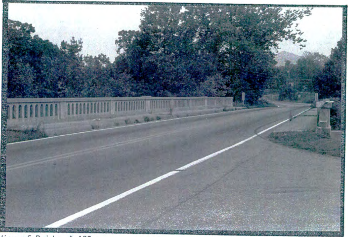
View of Bridge # 183
