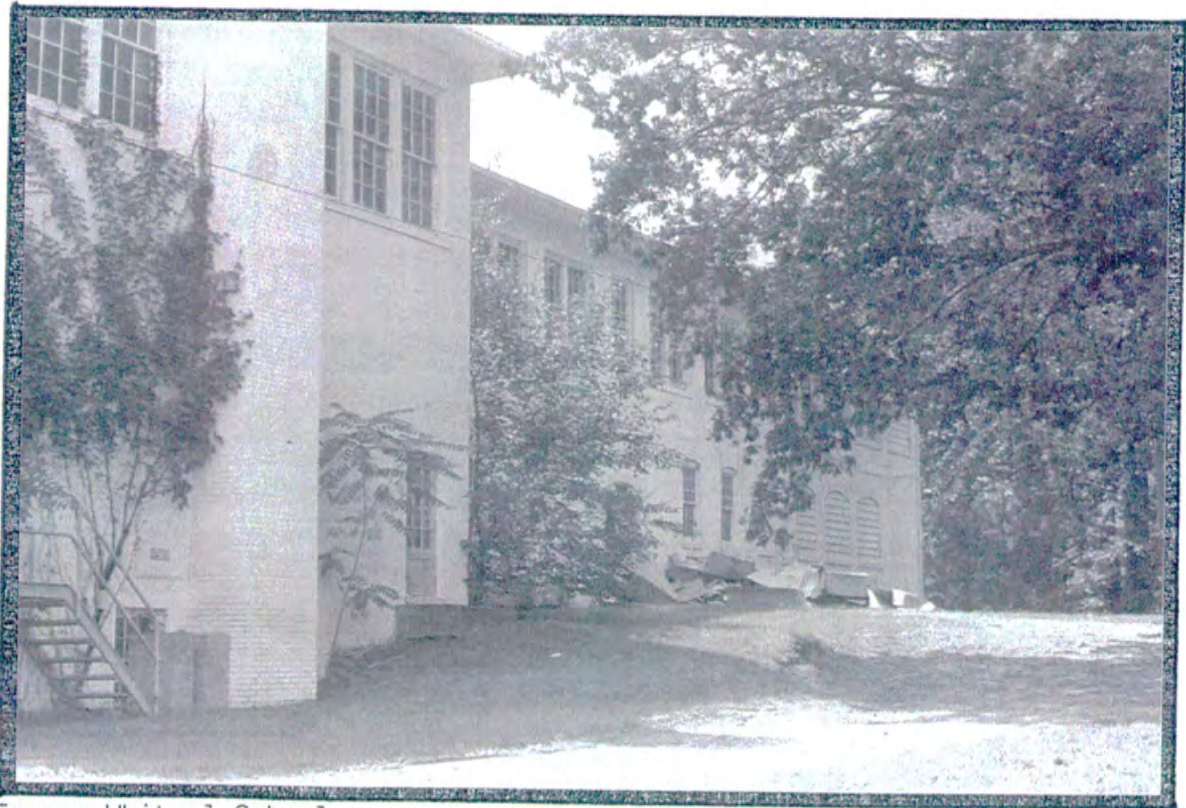
Former Whitnel School Rear Elevation
