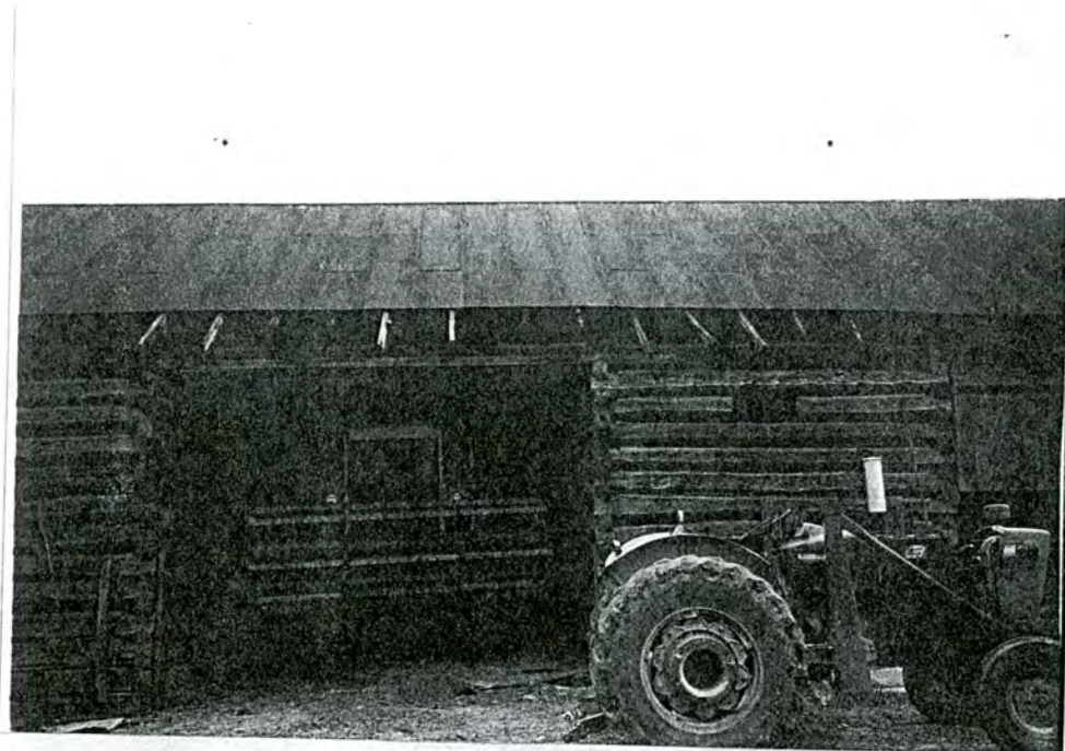
detail of roof support above entrance; notches for former joists are visible
