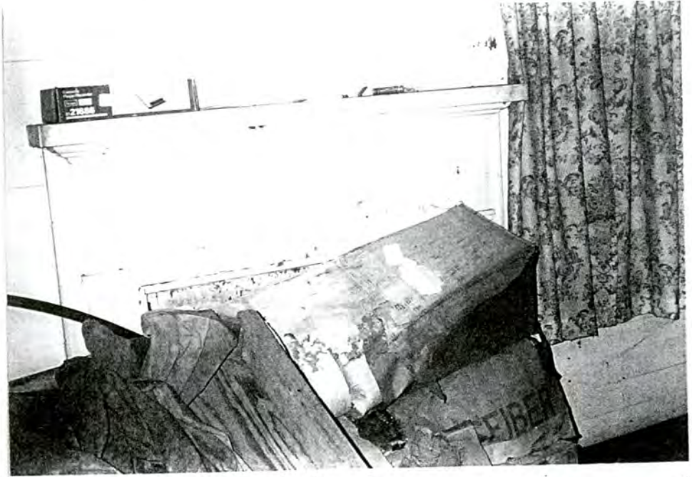
Mantel at front chimney (SE)
