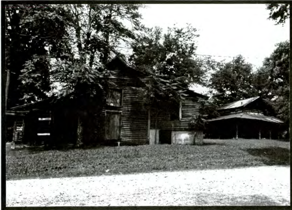
Plate VII.21 Packhouse and Tobacco Barn at Gaddis Hunt Farmstead, 3906 Guess Road (#8) Tobacco Barn at
