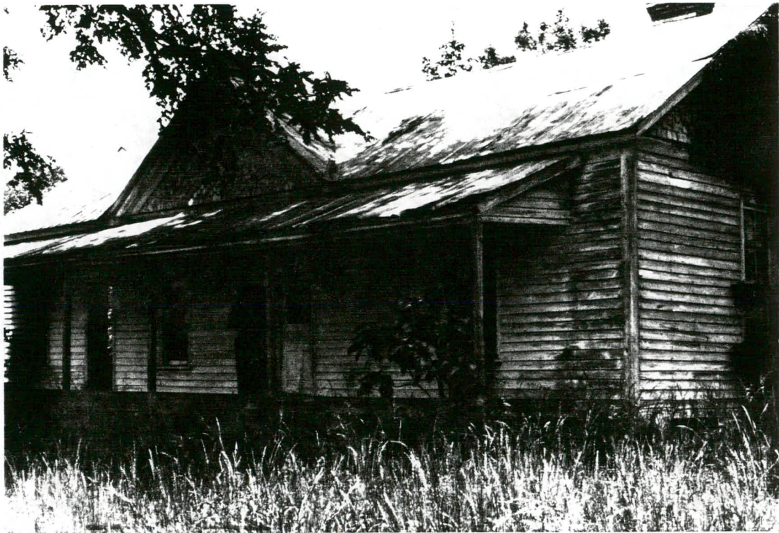
Figure 7: House/Hay barn on Pony Farm Road. View looking southwest.
