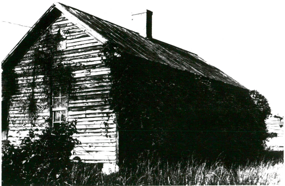
Figure 2b: House. View looking northeast.
