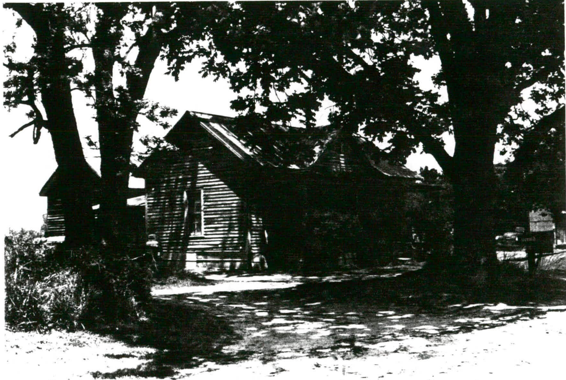
Figure 9: Cole Road House. View looking northwest.
