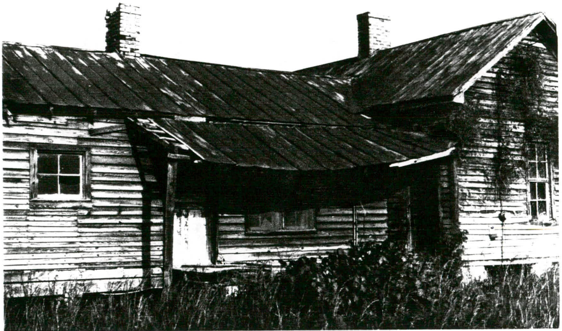
Figure 2a: House. View looking southeast.
