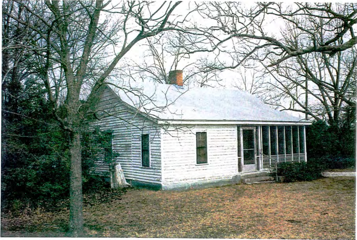
Head Farmhouse -- Three-quarter view from southwest.
