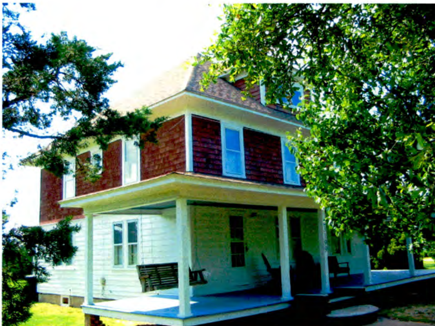
Plate 6. Rodanthe Historic District, Levine Midgett House, Facade and Side (South) Elevation, Looking Northwest.
