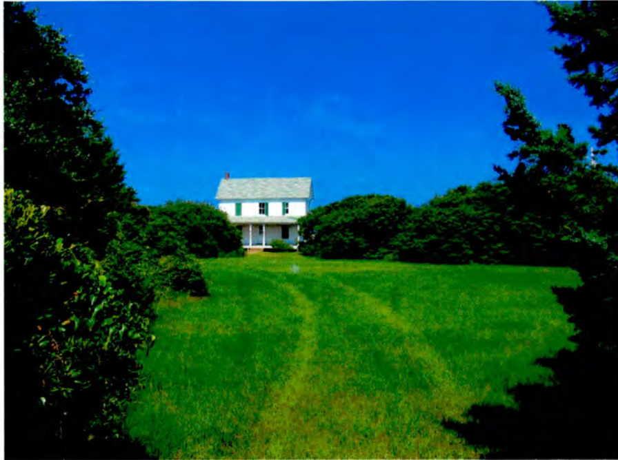
Plate 13. Rodanthe Historic District, Payne House, House and Setting, Looking East.
