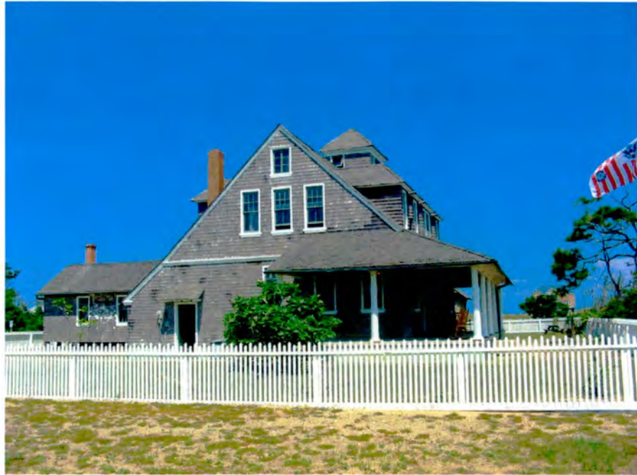
Plate 1. Rodanthe Historic District, Chicamacomico Lifesaving Station, 1911 Building, Side (West) Elevation, Looking East.
