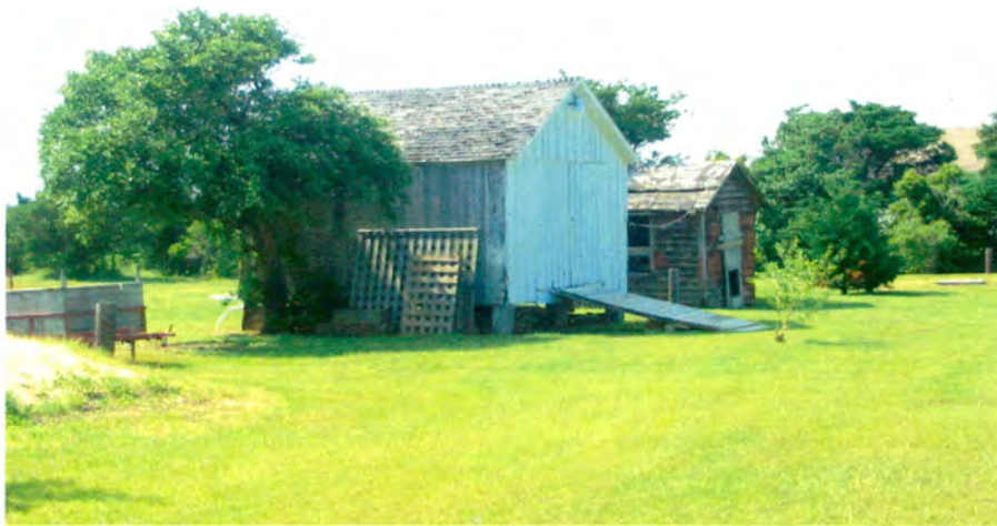
Plate 8. Rodanthe Historic District, Levine Midgett House, Boat House and Shed Behind House, Looking North.
