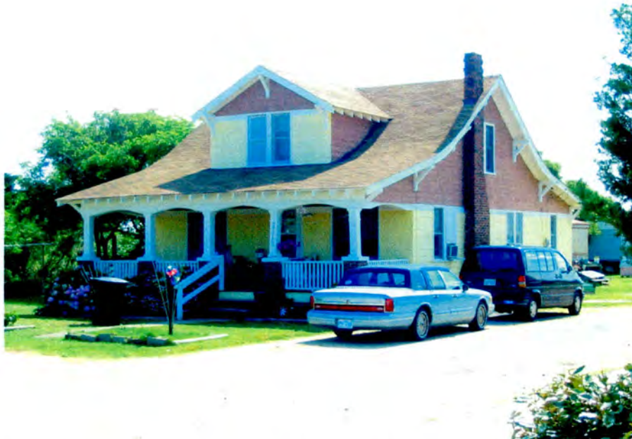
Plate 18. Rodanthe Historic District, Midgett Bungalow, Facade and Side (North) Elevation, Looking Southwest.
