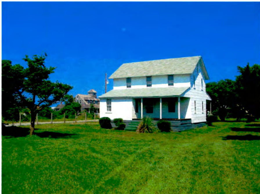
Plate 10. Rodanthe Historic District, Midgett House, Facade and Side (South) Elevation, Looking East.
