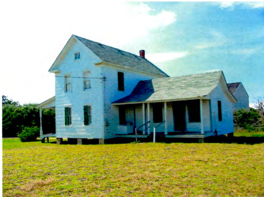
Plate 14. Rodanthe Historic District, Payne House, Side (South) Elevation, Rear (East) Elevation, and Rear Ell, Looking Northwest.
