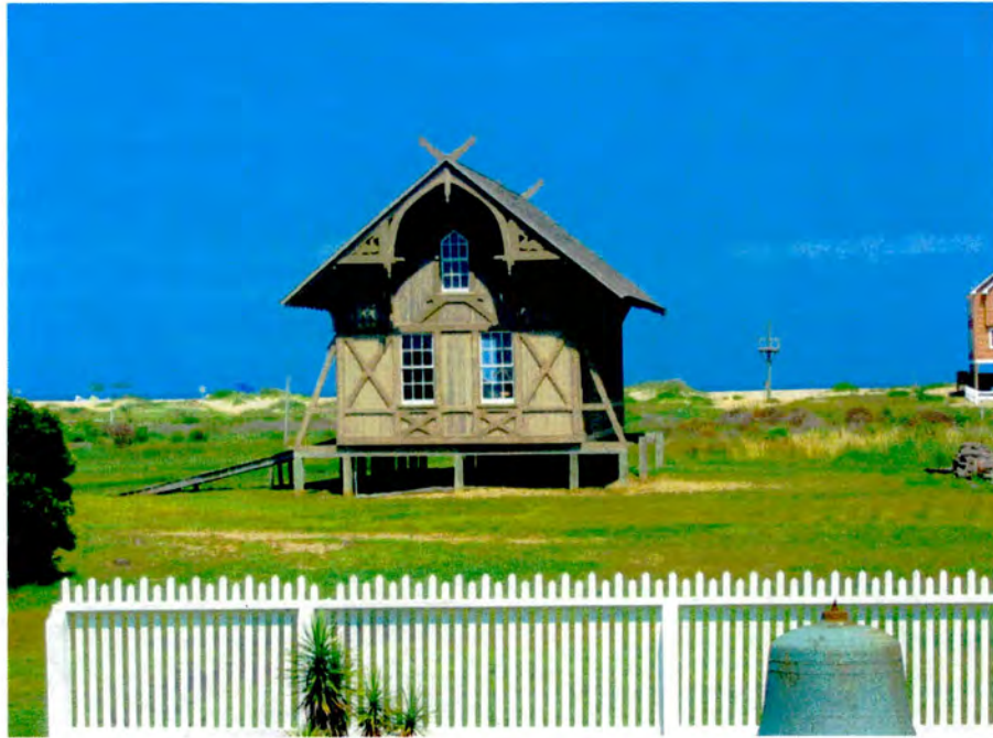
Plate 3. Rodanthe Historic District, Chicamacomico Lifesaving Station, 1874 Station (Now Boat House), Looking East.
