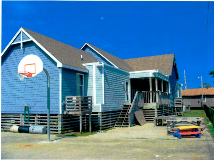
Plate 21. (Former) Rodanthe School, Side (South) and Rear (West) Elevations, Looking East.
