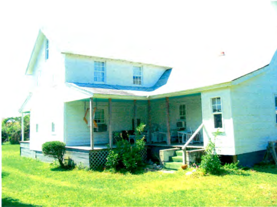
Plate 11. Rodanthe Historic District, Midgett House, Rear (East) Elevation and Rear Ell, Looking Northwest.
