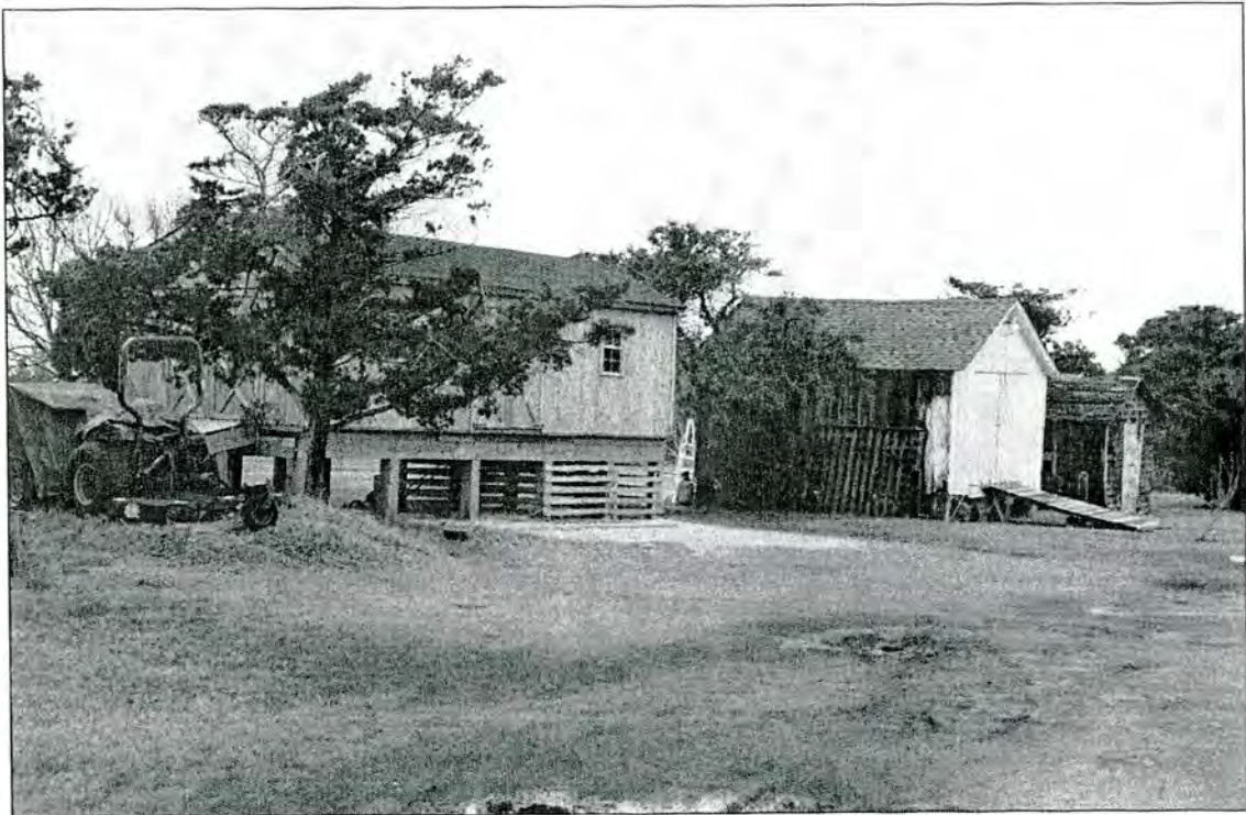
Plate 8: Looking northwest at shed and boathouse at right and elevated noncontributing outbuilding at left
