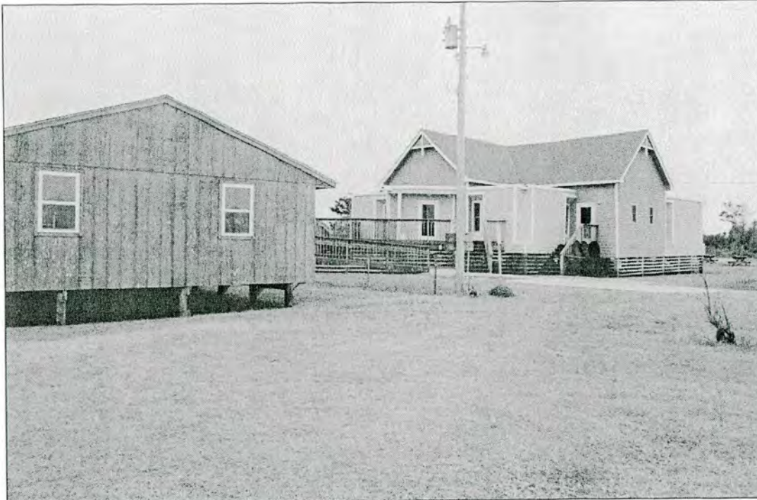
Plate 16: Former Rodanthe School – looking northwest; modern store on NC 12 in foreground
