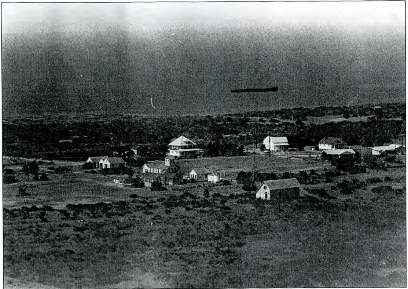
Plate 5: Looking northwest in Rodanthe in the 1960s at the Chicamacomico Lifesaving Station complex in the foreground and, across NC 12, the pyramidal-roofed Levene W Midgett House at the center and the Edward Midgett House at the far right; the house between the Midgett and Meekins houses was replaced in 1970 by a convenience store and gas station (source: OBHC)
