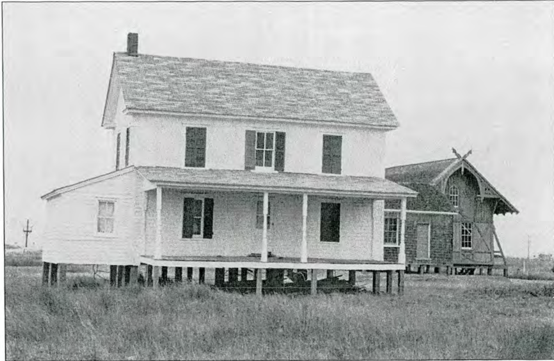
Plate 25: Cornelius P. Midgett House in 2006, looking southeast with 1874 lifesaving station at right
