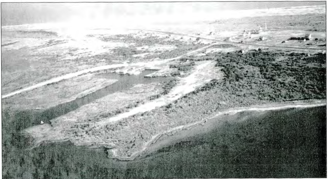
Plate 3: Looking east at Rodanthe in 1950s with sound at bottom, fish house and cruciform harbor at left, and lifesaving station and houses at right; proposed district extends linearly from harbor edge past lifesaving station to the ocean (source: NCDAH)
