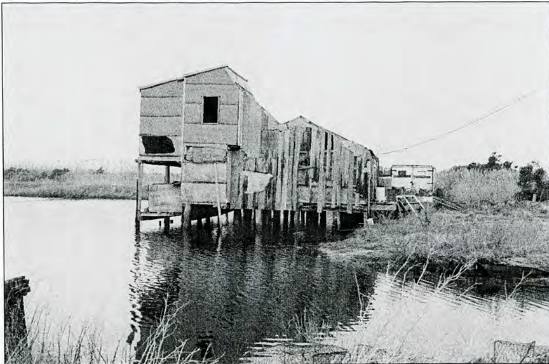
Plate 9: J. Frank Meekins Fishhouse – looking north
