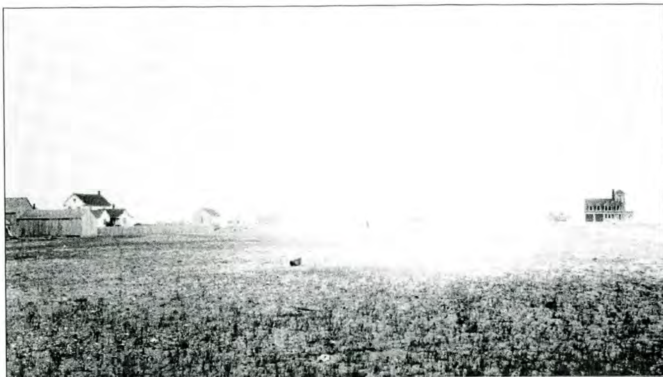
Plate 1: Rodanthe, September 6, 1926 – looking north at Cornelius P. Midgett House on original site at left, John Allen Midgett House at center left, and Chicamacomico Lifesaving Station at right (source: NCDAH)
