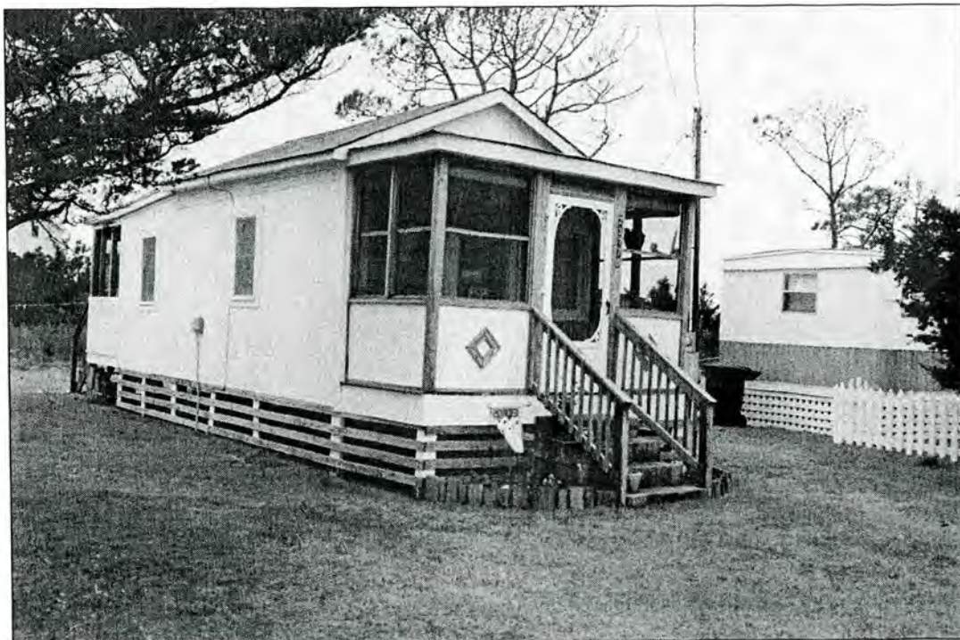
Plate 37: Looking northwest at Nora E. Herbert House with modern trailer on same lot at right
