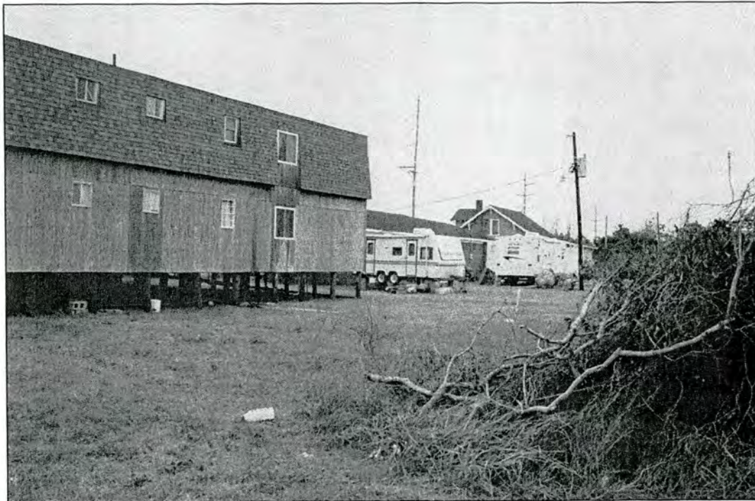
Plate 36: Looking southeast from Rodanthe School at Joseph Midgett House at right, ranchhouse behind recreational vehicle at center, and store at left
