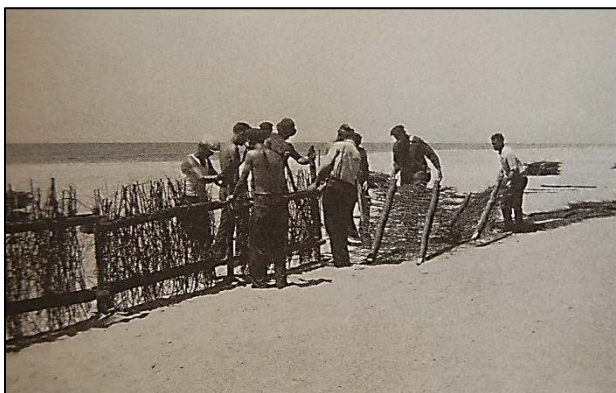
Sand fence under construction by Civilian Conservation Corps on Hatteras Island in 1936, at left, and completed fence, at right (source: Senter, “Live Dunes and Ghost Forests” and National Park Service, at left, and Dolan and Lins, “Outer Banks of North Carolina” and National Park Service, at right)
