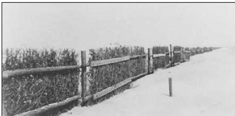
Sand fence under construction by Civilian Conservation Corps on Hatteras Island in 1936, at left, and completed fence, at right (source: Senter, “Live Dunes and Ghost Forests” and National Park Service, at left, and Dolan and Lins, “Outer Banks of North Carolina” and National Park Service, at right)
