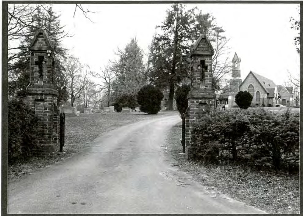
PLATE V.7 Calvary Episcopal Church (#1), lych gates and church, facing northeast
