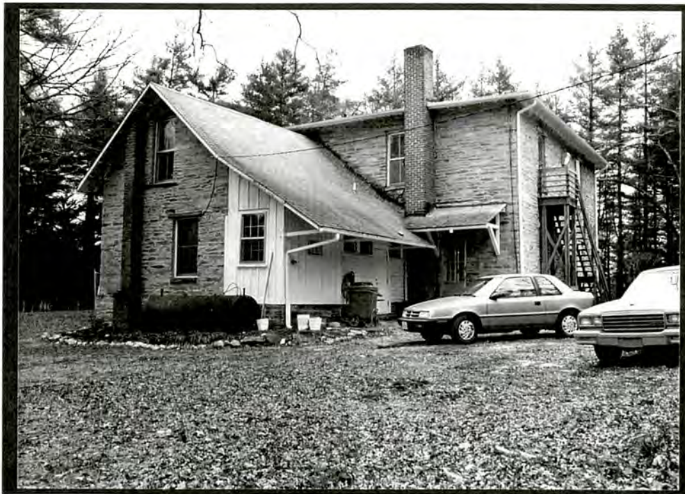
PLATE V.13 Calvary Episcopal Church (#1), former rectory, west rear and south side elevations
