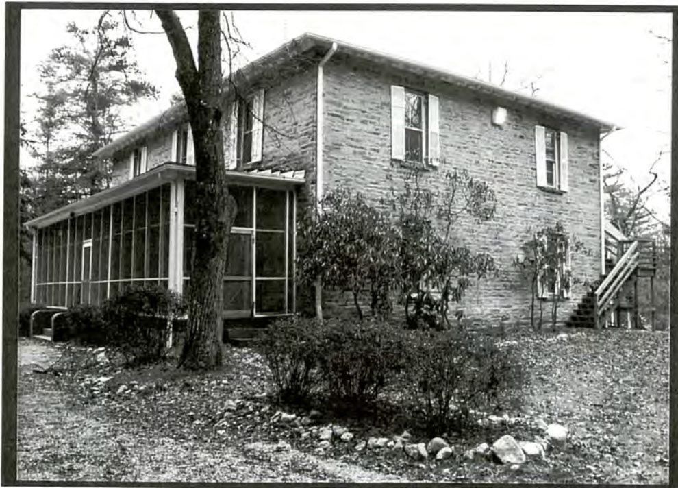
PLATE V.11 Calvary Episcopal Church (#1), former rectory, east front and north side elevations
