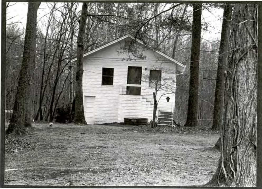
PLATE V.34 Oak Park Historic District (#2), house at 22A Graceland Place west front elevation
