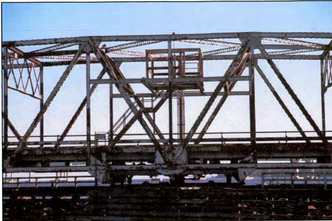
Figure 24: Truss bridge, stair and former frame of operator's house
