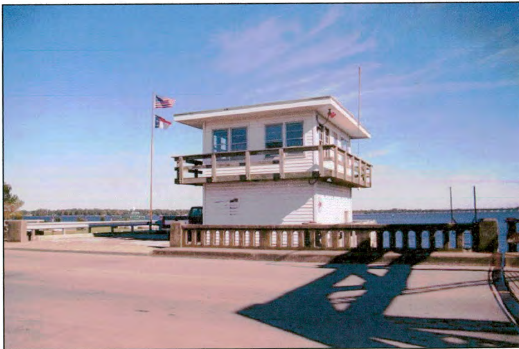
Figure 21: 1988 moved operator's house, west and south elevations (1988 parking deck adjacent)
