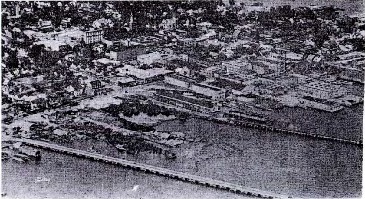
Figure 39: Trent River Bridge at George Street (foreground) ca. 1940. This bridge, west of the railroad trestle bridge, had undergone major repairs ca. 1930. Image taken from The City of New Bern, NC, Extends a Hearty Welcome to All (brochure, probably written by Gertrude Carraway). North Carolina Collection, J. Y. Joyner Library, East Carolina University, Greenville, NC.
