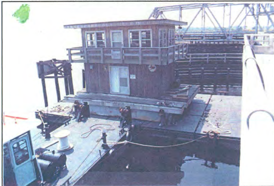
Figure 23: Bridge Operator's House moved by barge from Carteret County at new site on Cunningham Bridge, 1988 (Bridge Maintenance Records, NCDOT).
