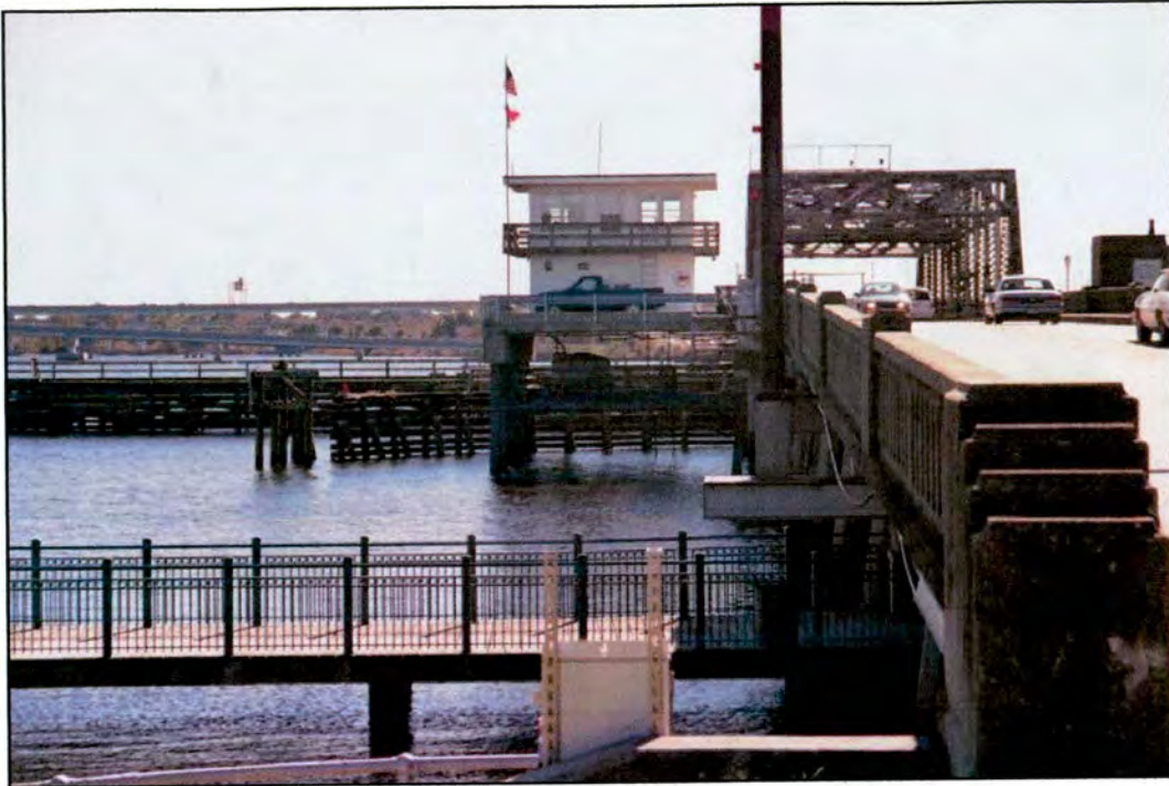
Figure 14: Alfred A. Cunningham Bridge, viewpoint from bridge's east side, looking south (walkway under bridge constructed ca. 1997 for Union Point Park)
