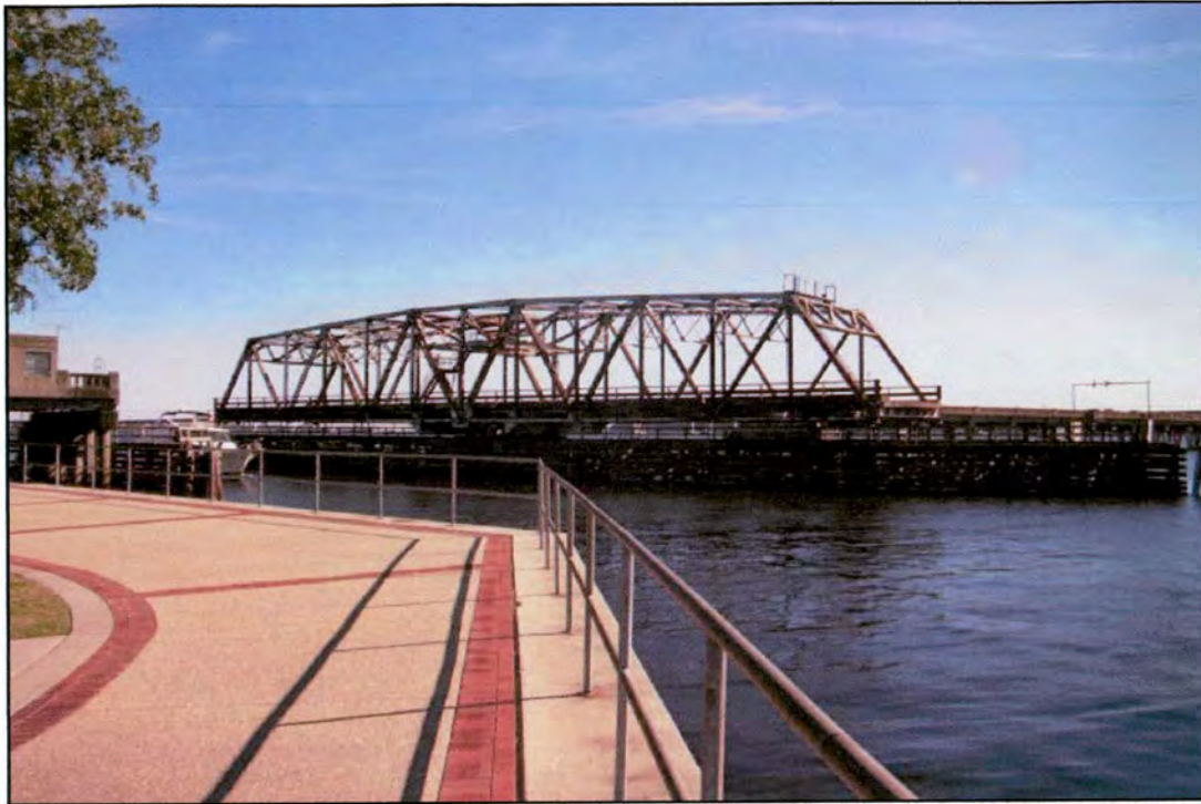
Figure 26: Alfred A. Cunningham Bridge, west elevation, swing span in operation. Photograph taken from Convention Center promenade.
