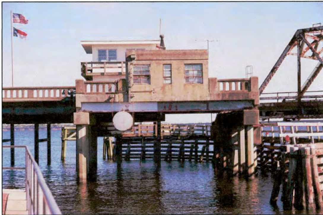
Figure 17: 1955 bridge tender house, west elevation
