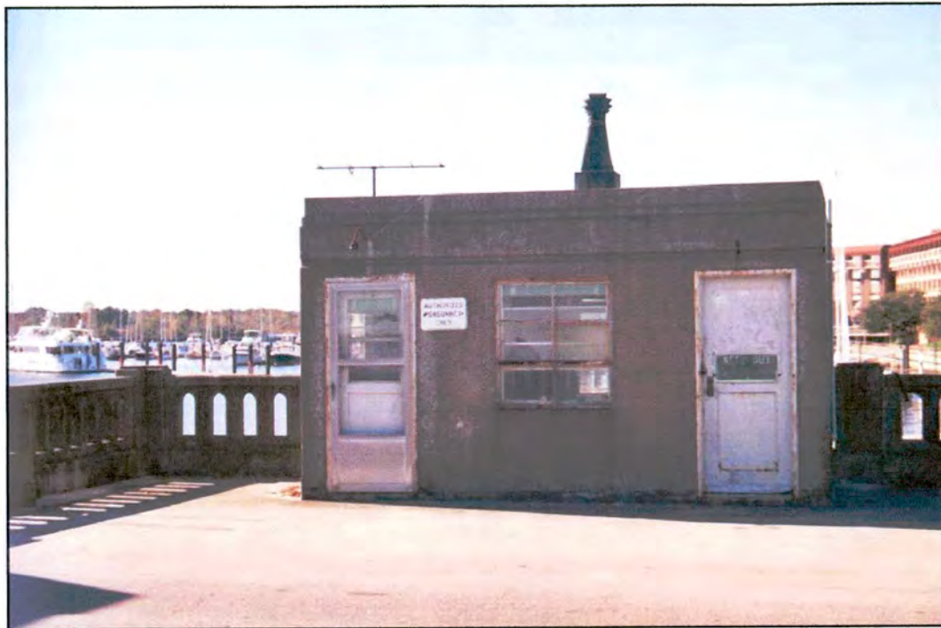
Figure 18: Bridge tender's house, east elevation
