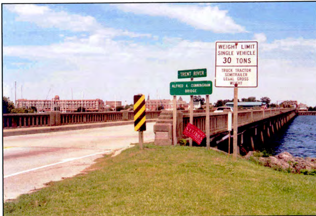
Figure 13: South Approach, Alfred A. Cunningham Bridge, looking towards north bank of Trent River waterfront
