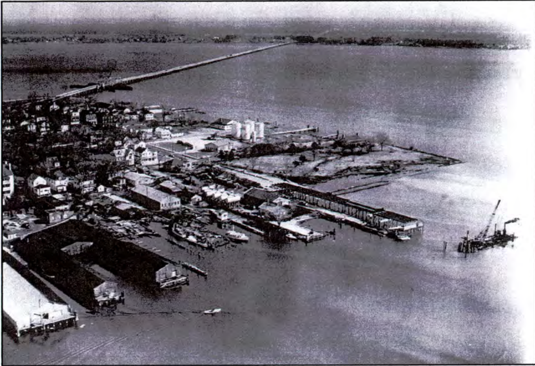
Figure 33: Aerial photograph of Alfred A. Cunningham Bridge under construction, ca. 1954. Kellenberger Room, Craven County Public Library, New Bern, NC
