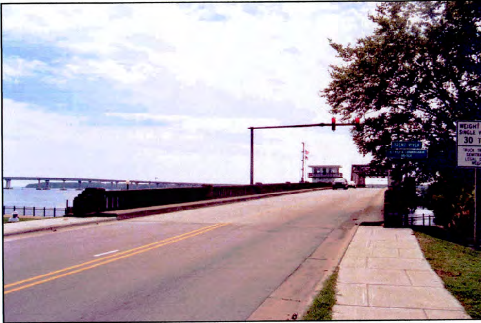
Figure 12: North Approach, Alfred A. Cunningham Bridge
