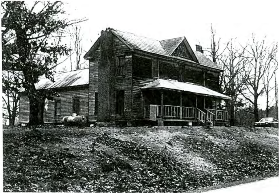
2-A. Thomas A. Ausley House, overall view to E
