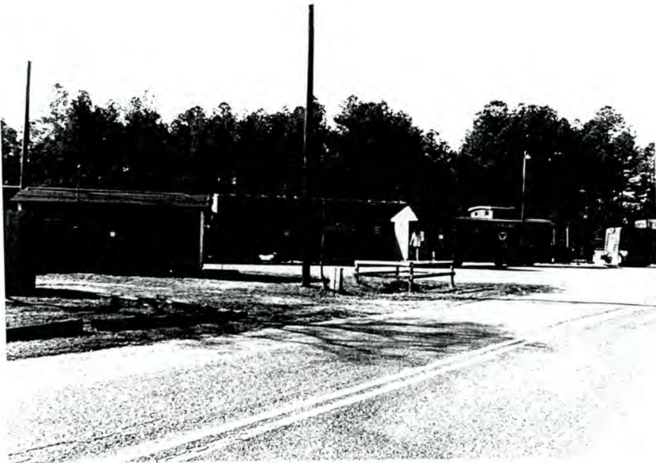
70-A. North Carolina Railroad Museum, view to W
