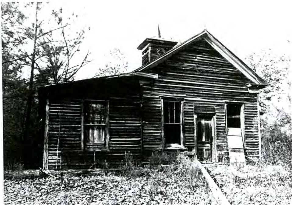
17-D. Lawrence School, E elevation, view to W
