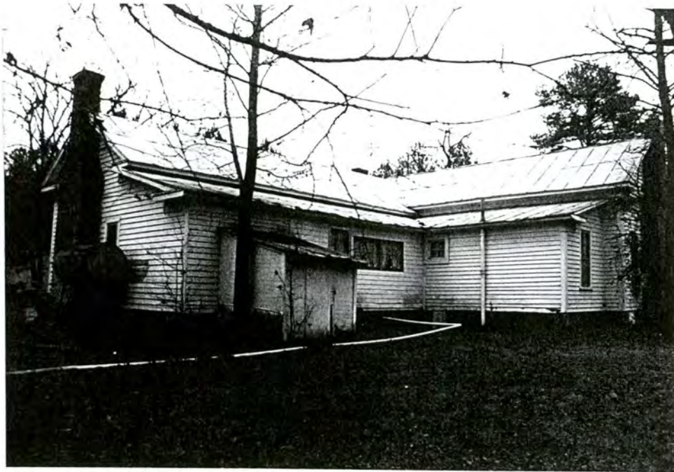
18-B. Marks-Harrington House, rear view to SE
