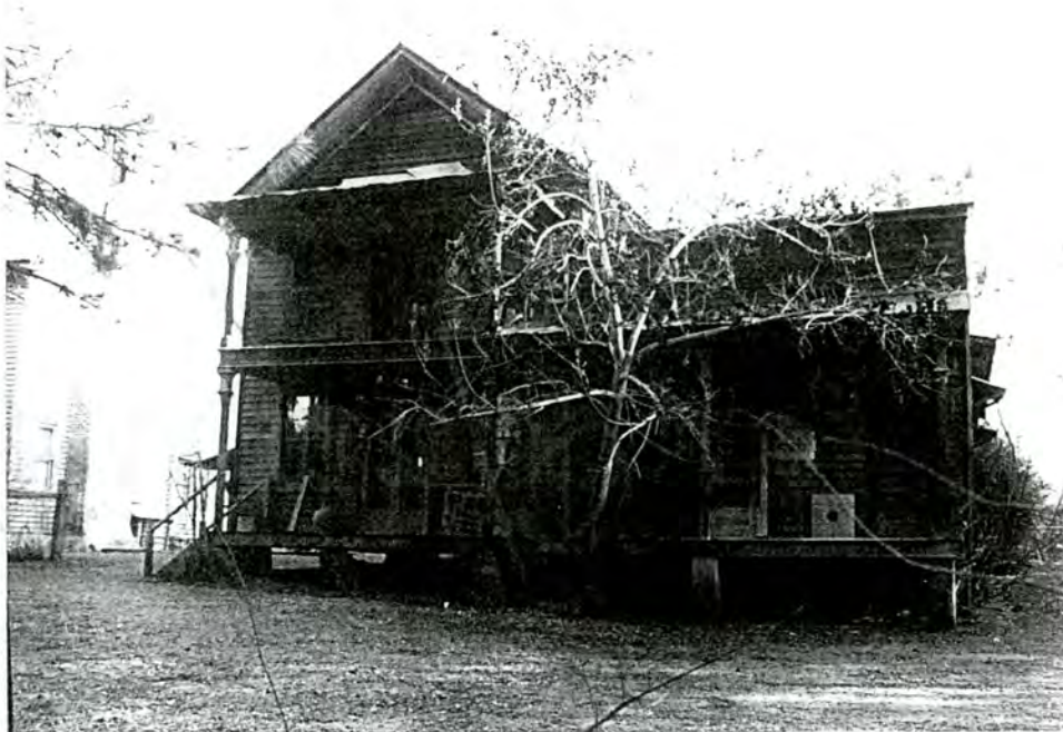
71-I. Merry Oaks Historic District, Yates Store, view to SE
