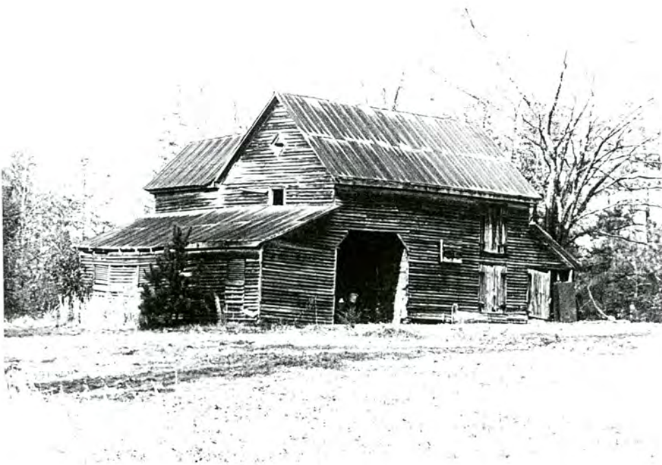
16-B. Thomas Fred Cross House, barn, view to W
