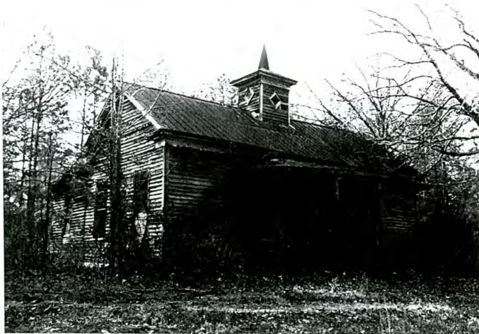
17-B. Lawrence School, overall view to SW
