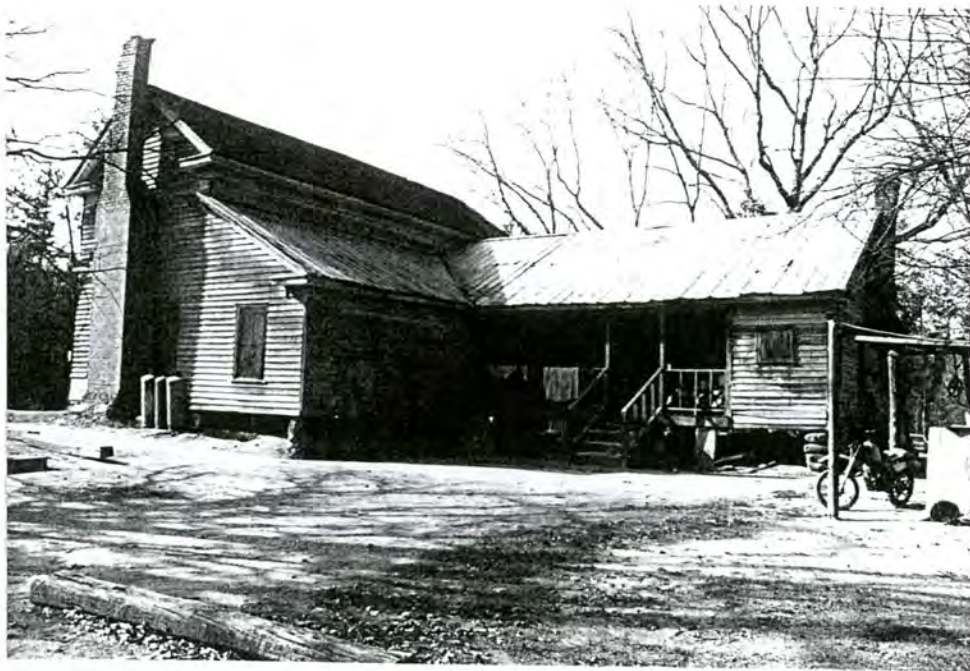
2-B. Thomas A. Ausley House, rear view to W
