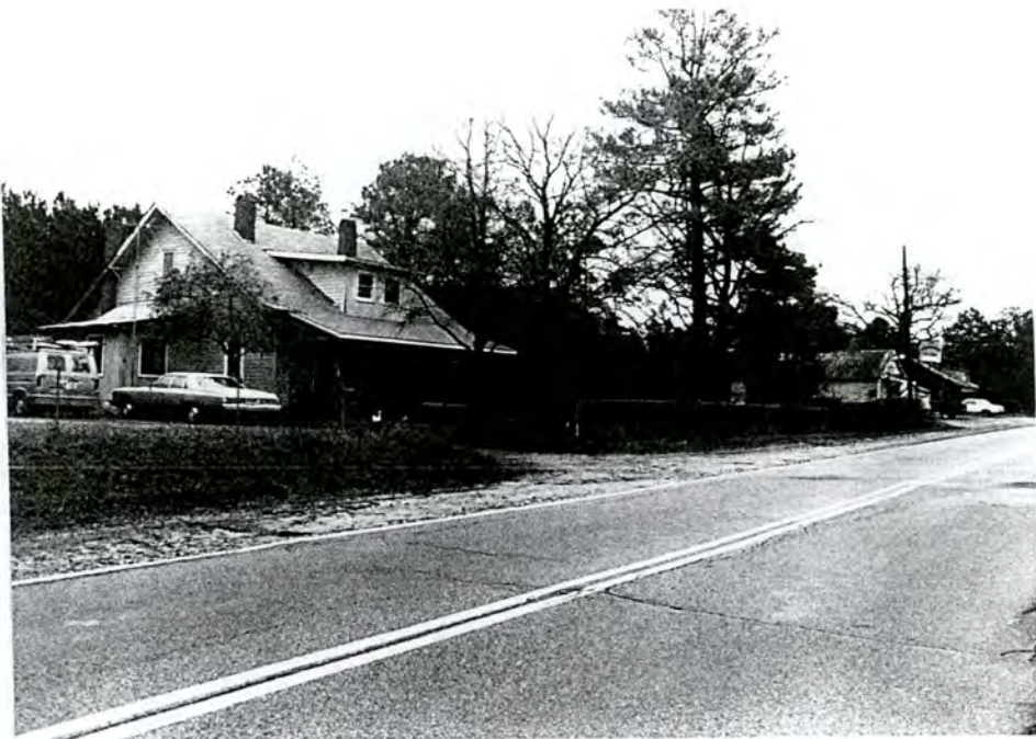
69-B. Bonsal Stores and Houses, view to NE
