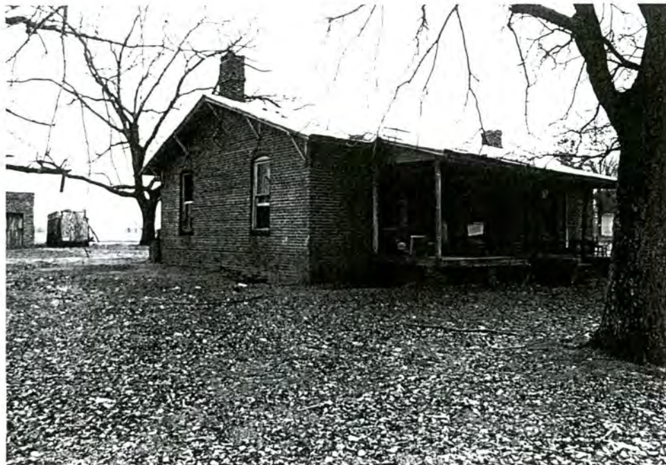
31-32-B. Cherokee Brick Company Tenant Houses, house #31, overall view to SE
