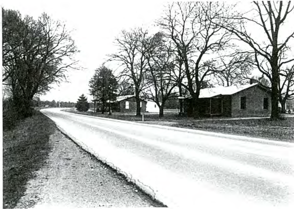
31-32-A. Cherokee Brick Company Tenant Houses, overall view to N
