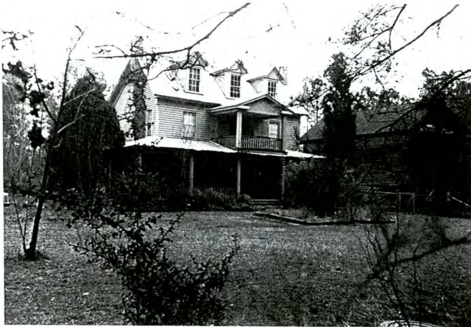
71-H. Merry Oaks Historic District, Edwards House, view to S
