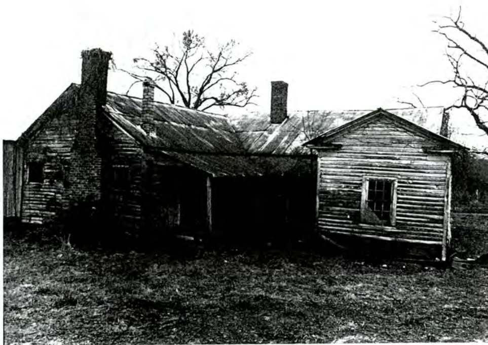
20-B. James Rufus Marks House, rear view to SW
