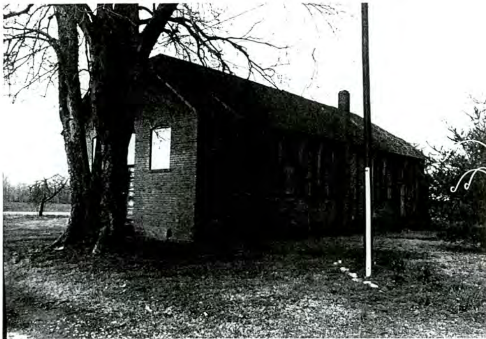
33-C. Brickhaven School, rear view to NW
