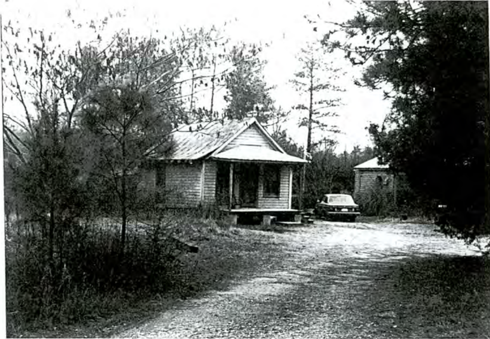
71-G. Merry Oaks Historic District, Merry Oaks Post Office, view to S
