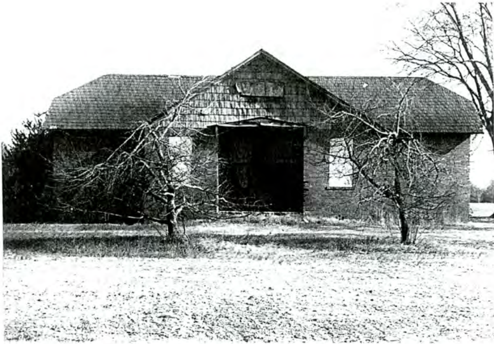
33-B. Brickhaven School, facade, view to E
