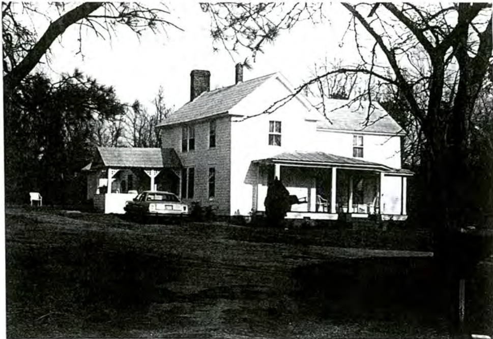
16-A. Thomas Fred Cross House, overall view to N
