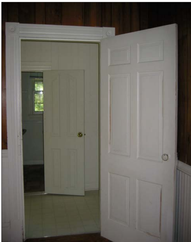
Armfield McLean House figure 25, above: center hall, facing north towards kitchen and bathroom
