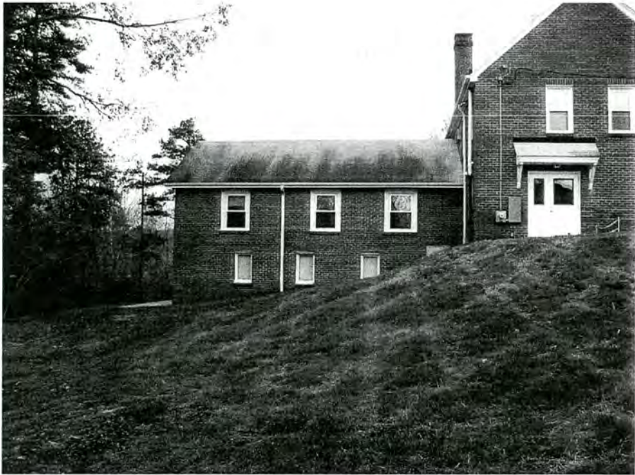
Plate 3. Oakdale United Methodist Church, Side (South) Elevations of Church and Rear Education Wing, Looking North.
