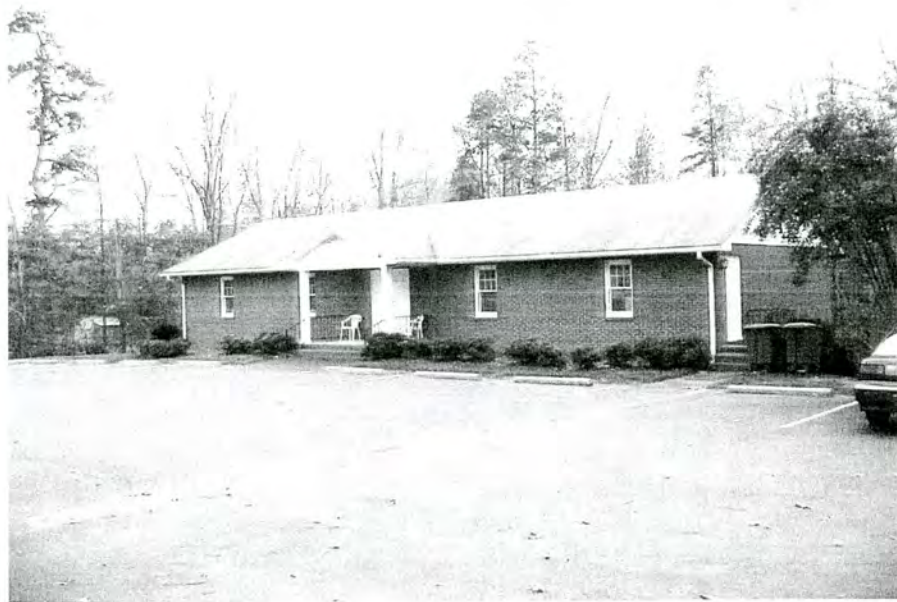
Plate 8. Oakdale United Methodist Church, Parish Hall Building, Looking Southwest.
