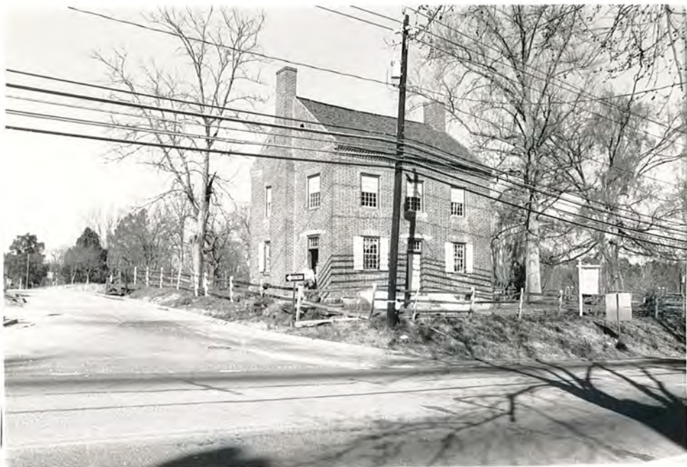
18. (D) Jamestown Historic District, Mendenhall Store, view to NE
