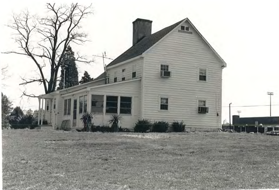
105. (B) Mark Iddings House, side and rear view to SE
