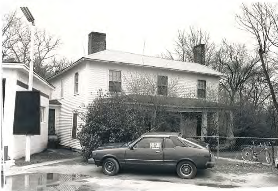
110. Wharton House, overall view to S
