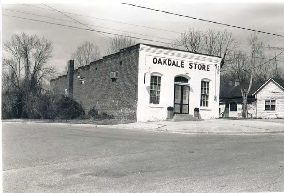
30. (B) Oakdale Cotton Mill Village Historic District, Oakdale Store, view to N
