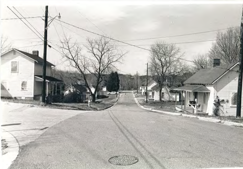
31. (C) Oakdale Cotton Mill Village Historic District, Oak Street, view to NW
