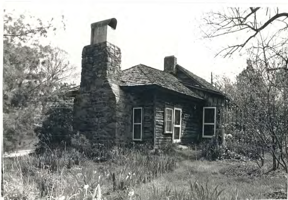
28. (B) Potter House, west side and rear, view to NE
