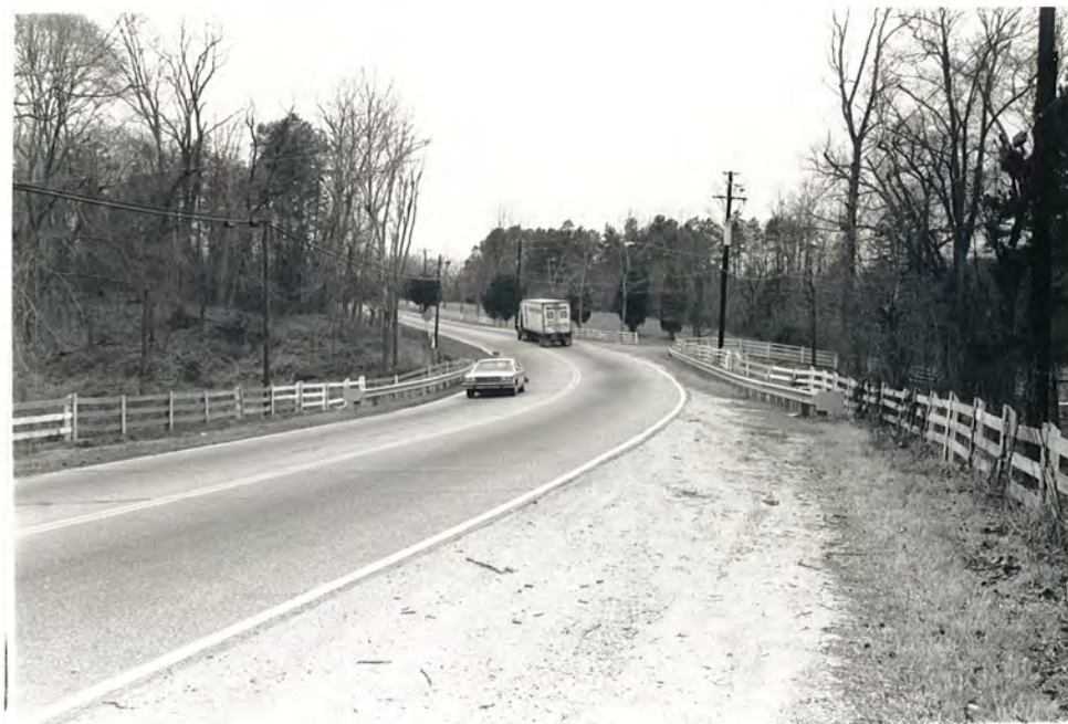
4. High Point Rd. just W of RR overpass, view to NW
