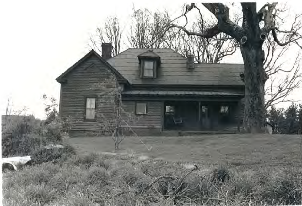
101. (A) House, facade, view to S
