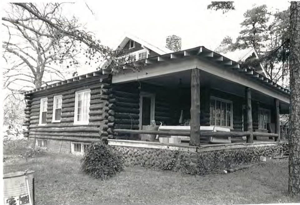
47. (C) Jamison-Ward House, side and facade, view to N
