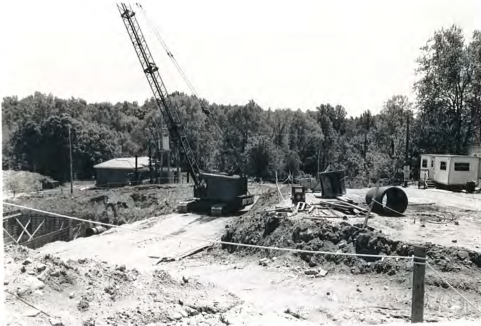
97. (A) High Point Waterworks, new construction, view to S
