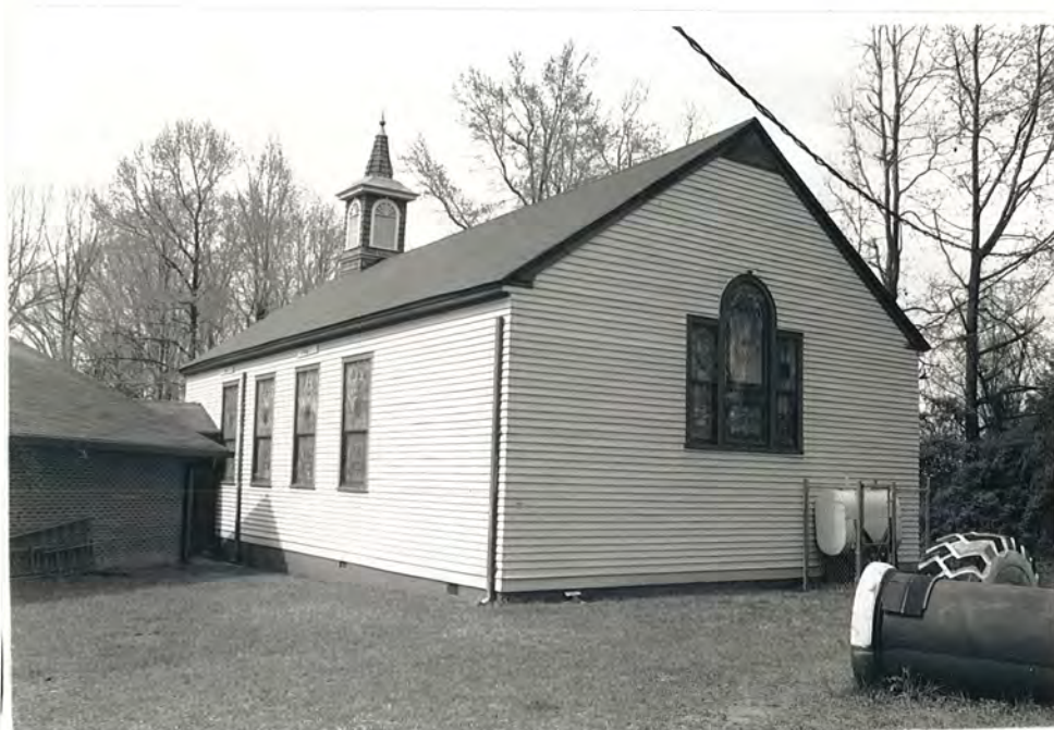
55. (C) Celia Phelps Methodist Episcopal Church, rear and side, view to NW
