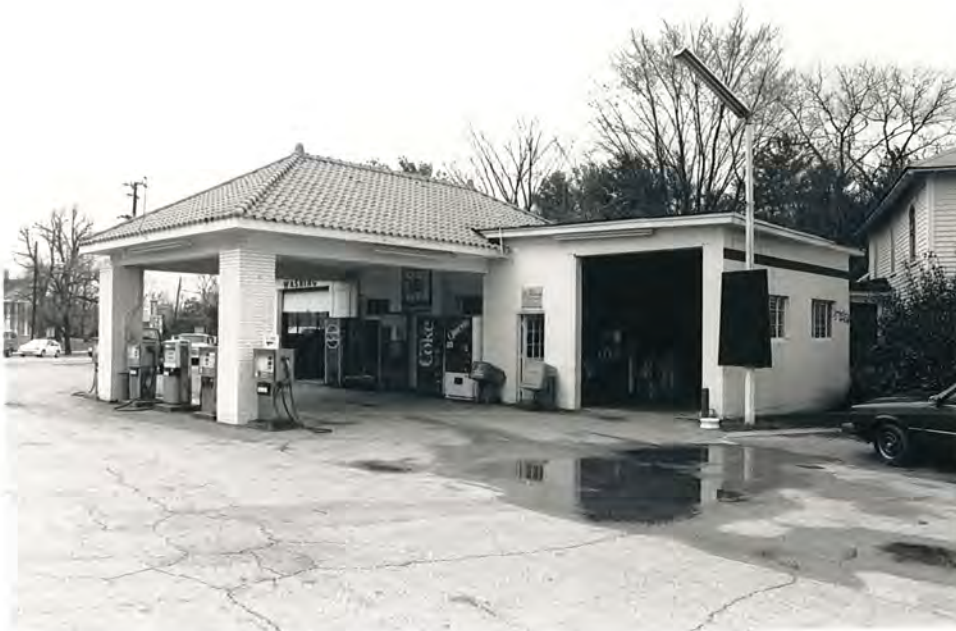
96. (A) Gas Station, overall view to E
