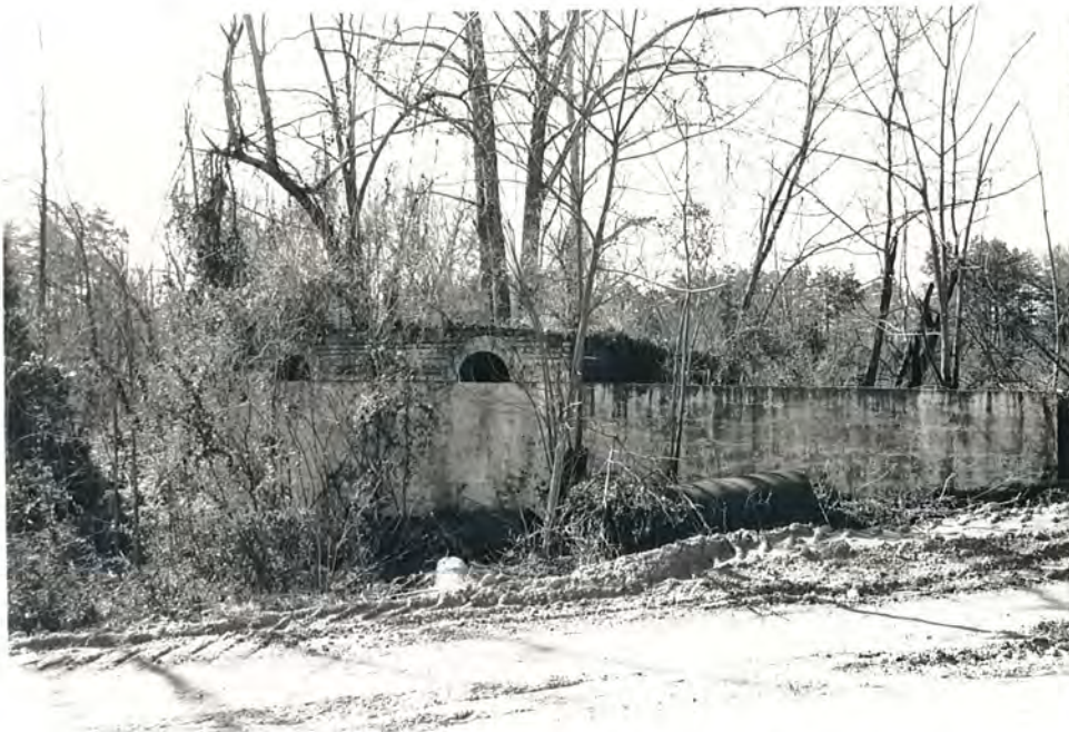
98. (B) High Point Waterworks, remains of steam-powered pumping station, view to SW
