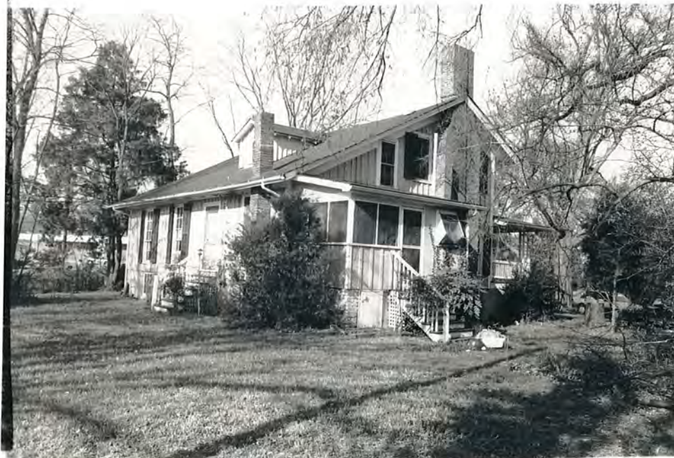
23. (C) Shubal Coffin House II, rear and south elevations, view to NE
