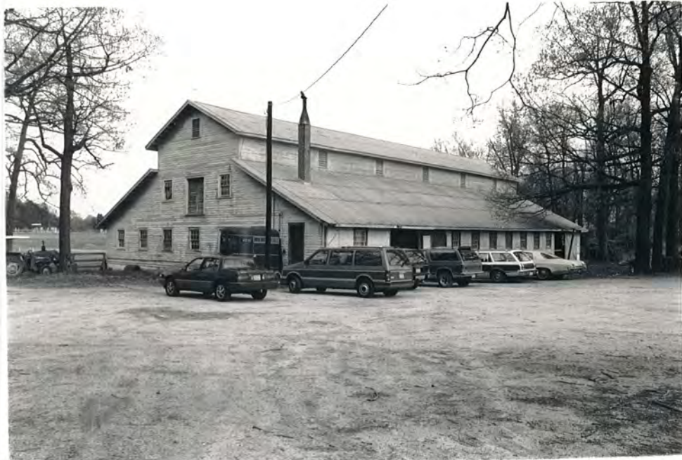
76. (A) Sedgefield Stables, main stable, view to SE
