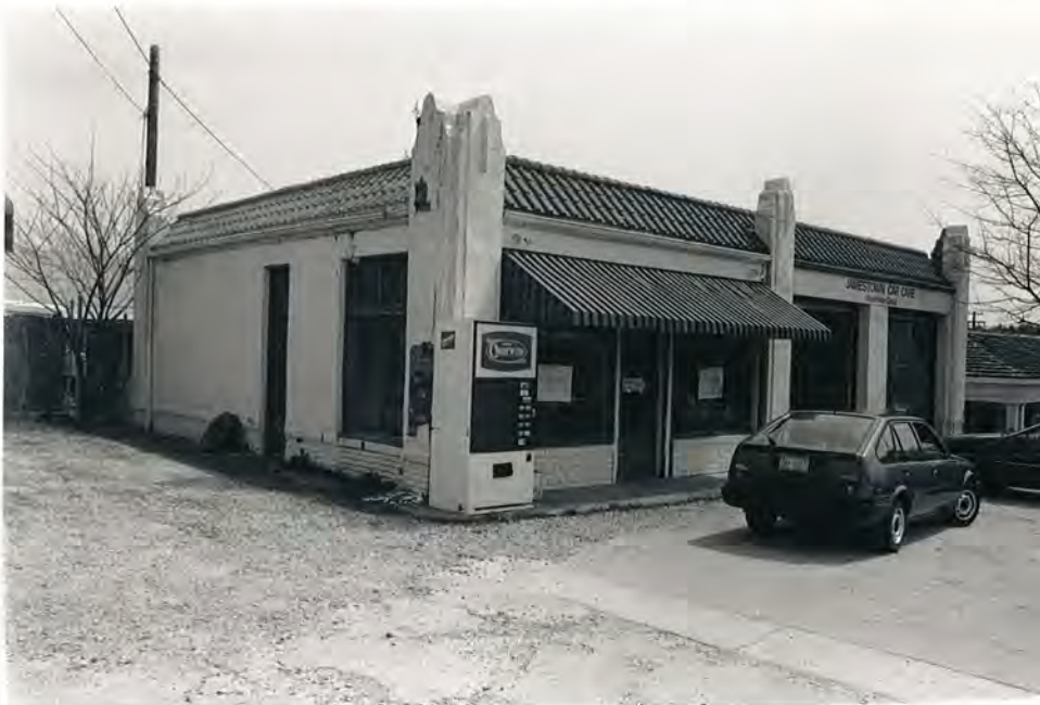
80. (A) Standard Oil Station, overall view to SE
