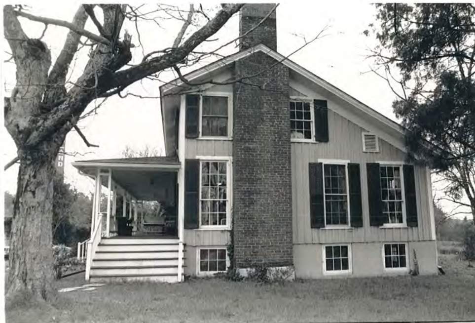
22. (B) Shubal Coffin House II, north elevation, view to S
