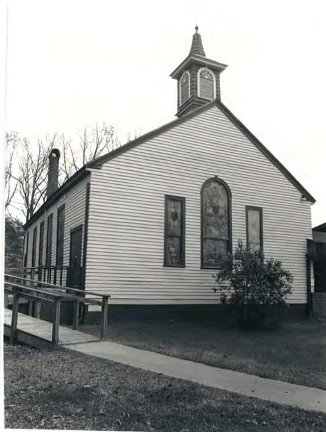
54. (B) Celia Phelps Methodist Episcopal Church, facade and side view to SE
