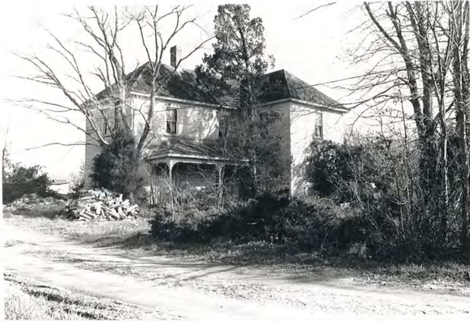
94. (A) Garrett-Moore House, overall view to SE
