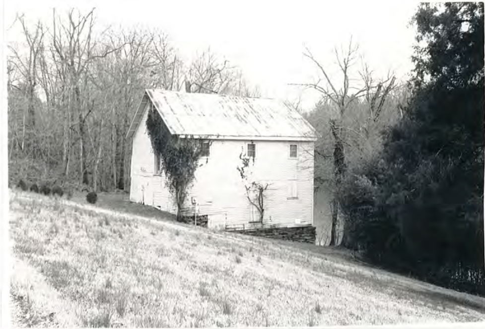
49. (A) Mill and Miller's House, mill, view to SE
