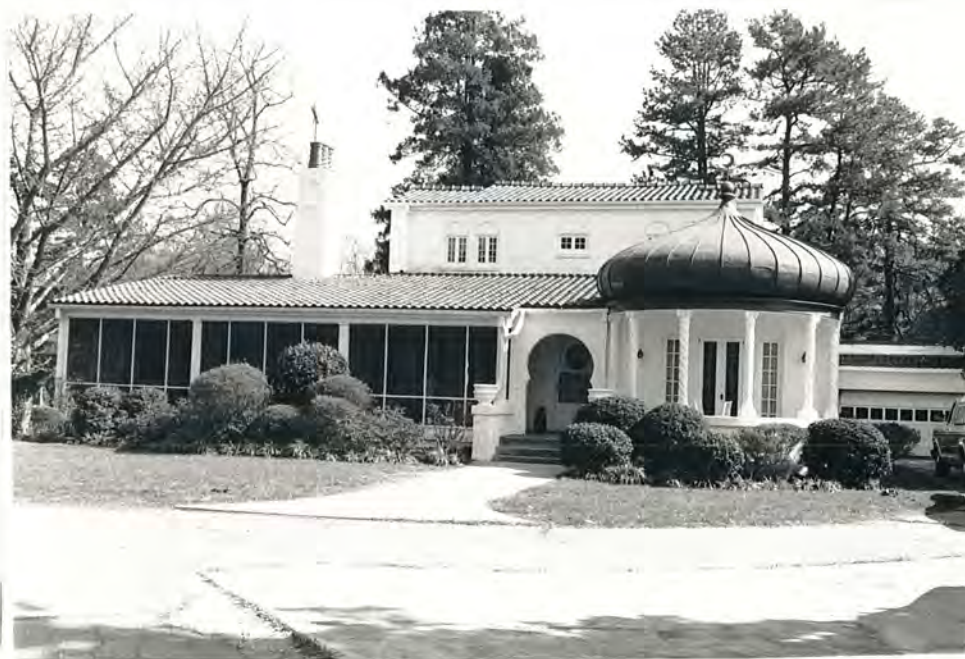
40. (A) Terry Harper House, facade, view to SE
