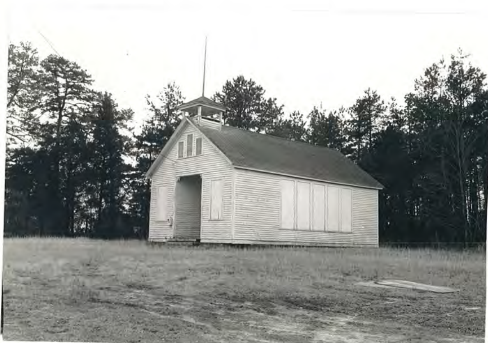
33. (E) Oakdale Cotton Mill Village Historic District, Oakdale School, view to S
