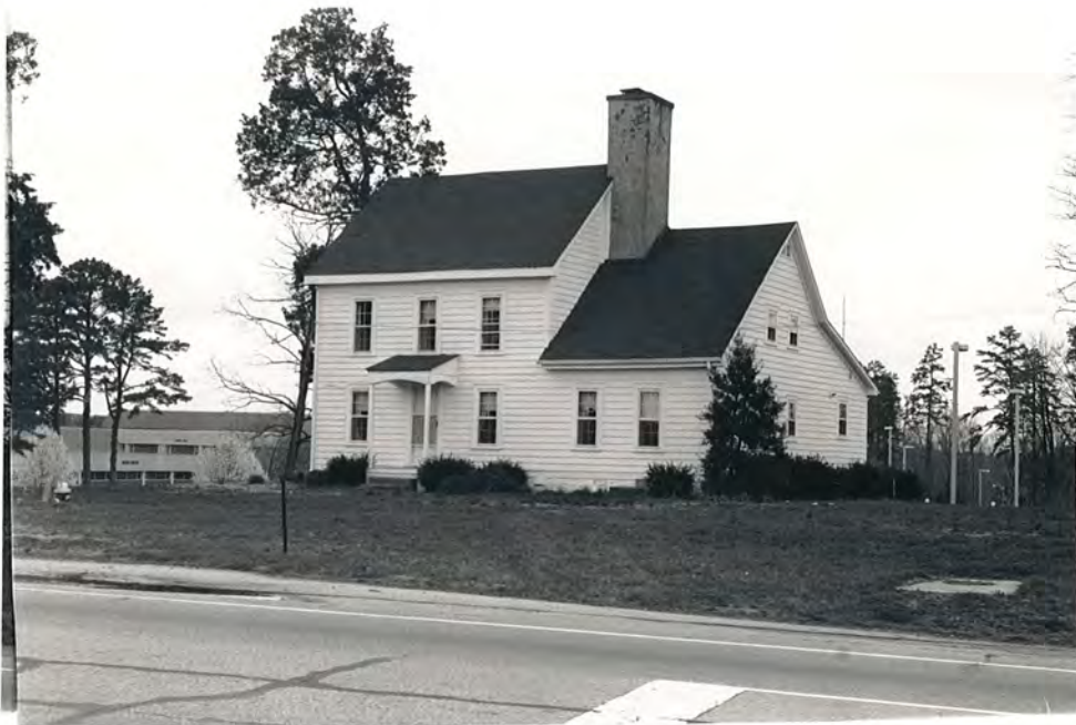
104. (A) Mark Iddings House, overall view to NW
