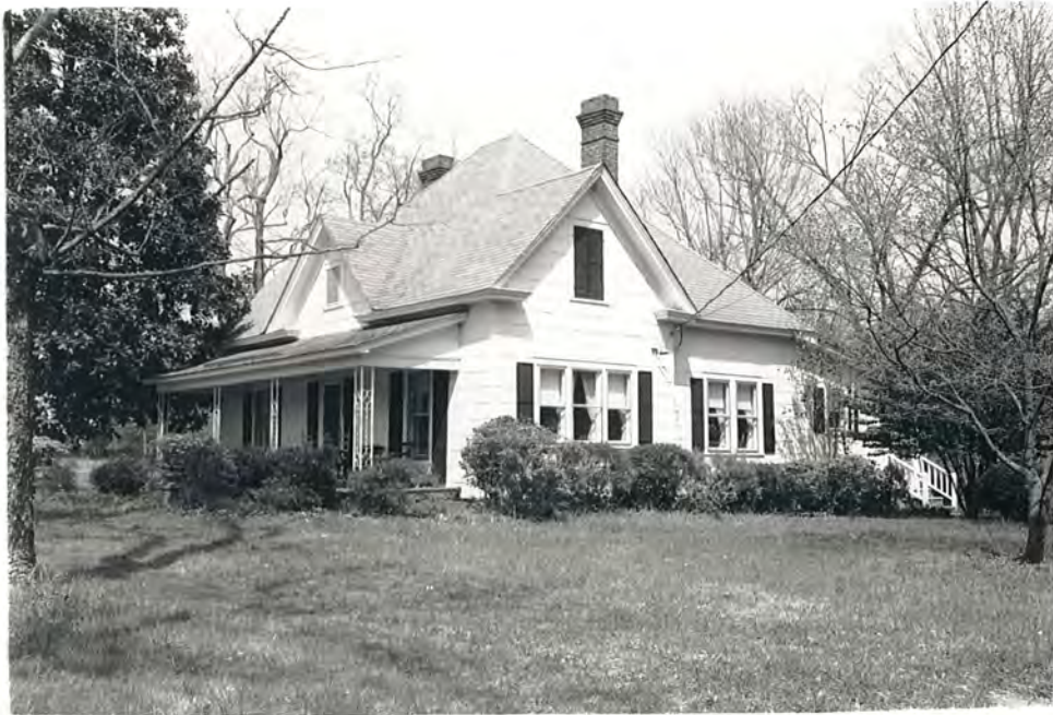
89. (A) Armfield-McLean House, overall view to N
