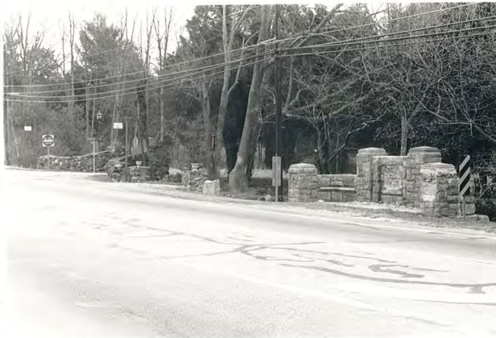
68. (G) Sedgefield Historic District, gate and stone seating, entrance to E. Sedgefield Dr., view to SE
