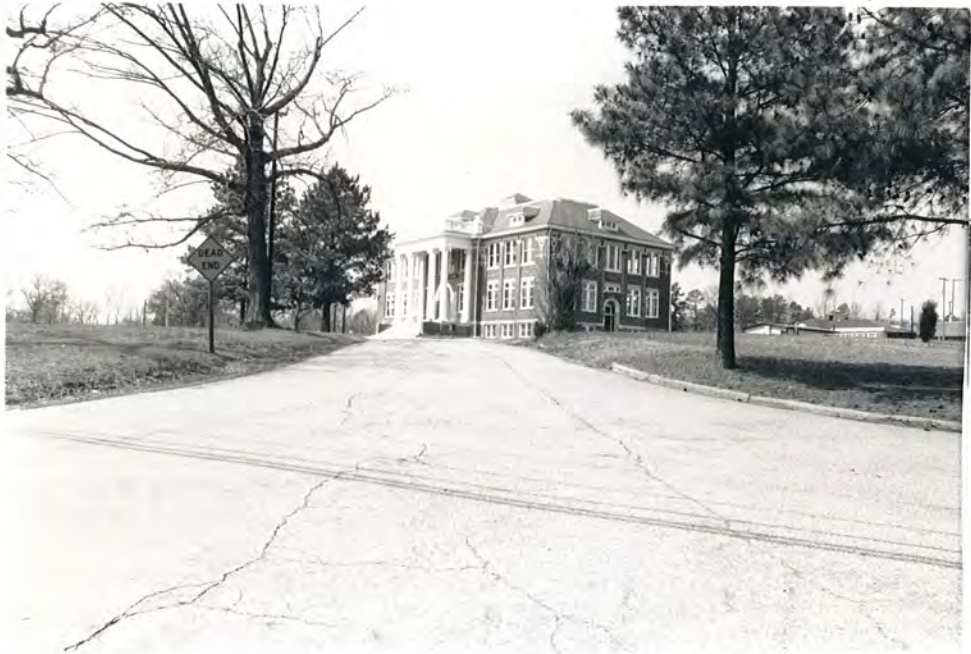
24. (A) Jamestown Public School, view with setting, to NW
