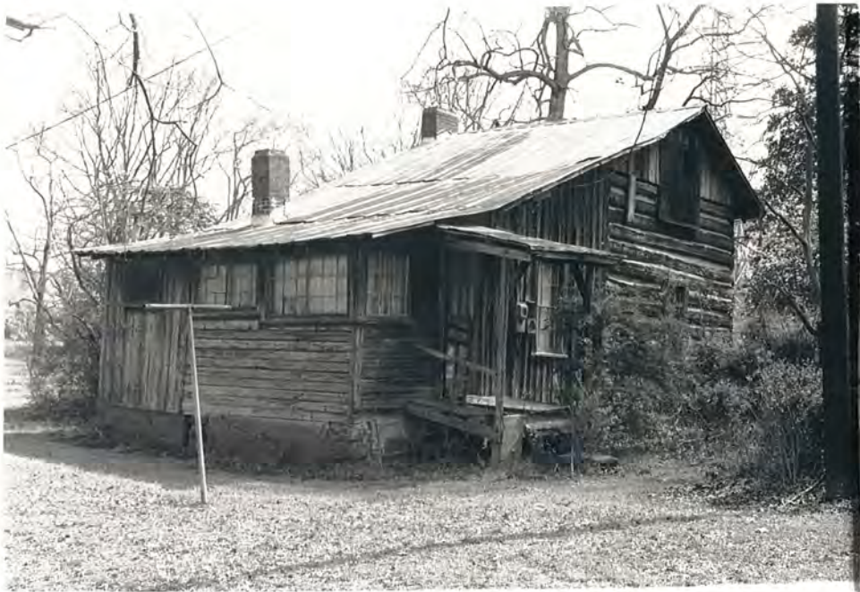
109. (B) Suits House, rear and southwest side, view to E
