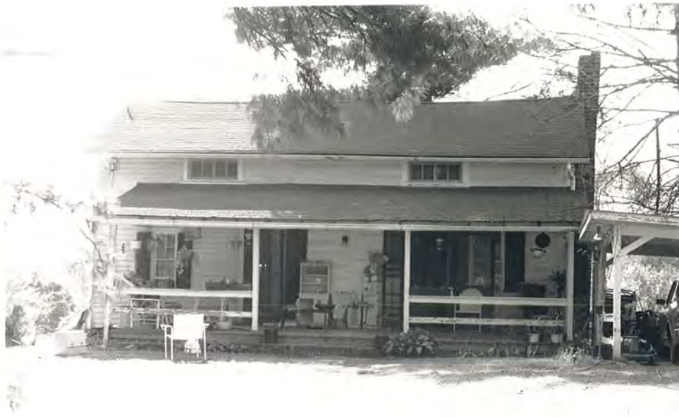
60. (E) Ragsdale Farm, tenant house, view to W
