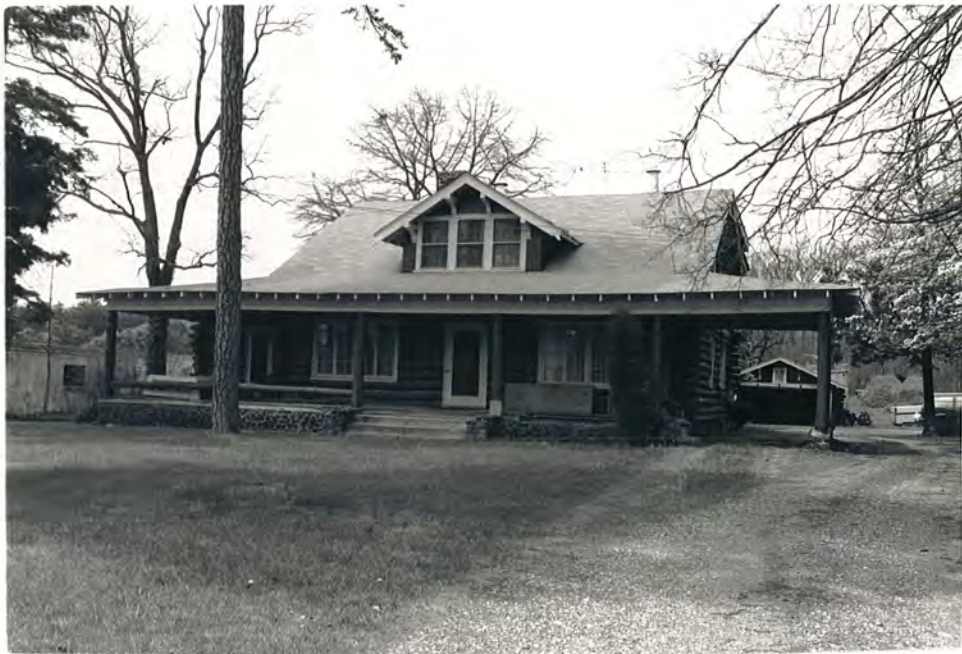
46. (B) Jamison-Ward House, overall view to W
