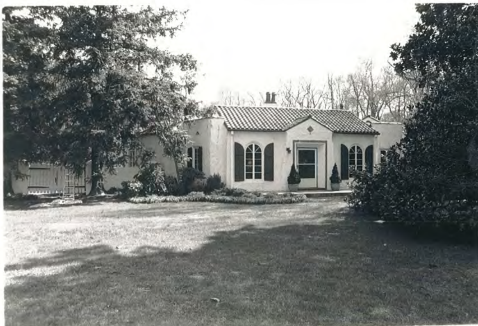
42. (C) J. C. Welch House, overall view to S
