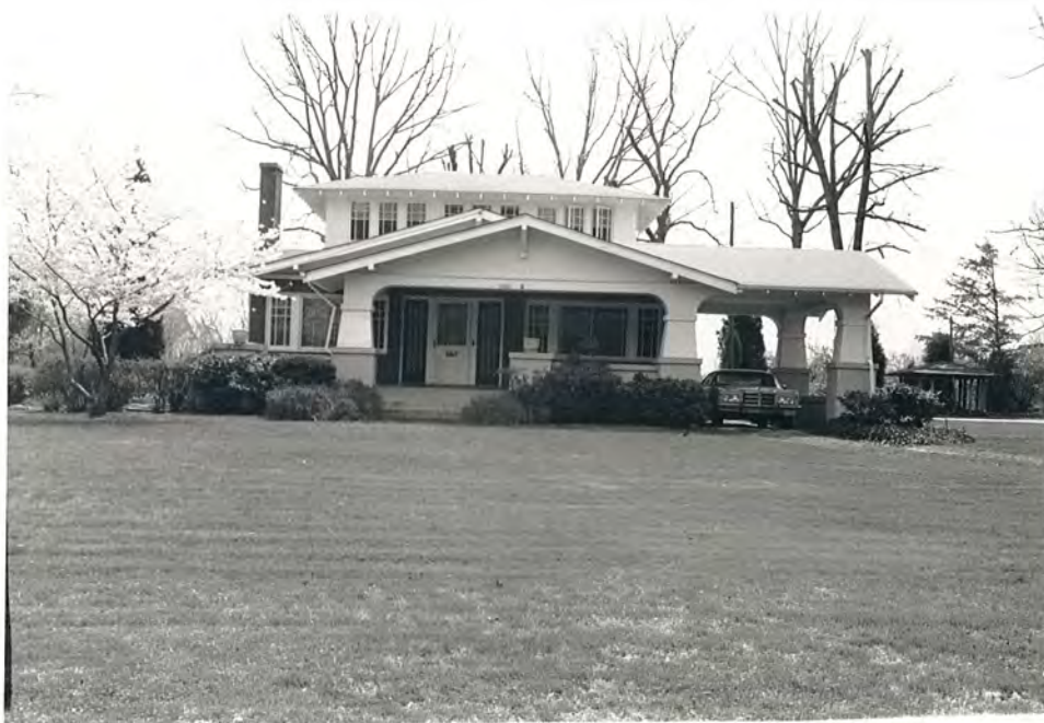
86. (B) Orville Williard House, facade, view to S
