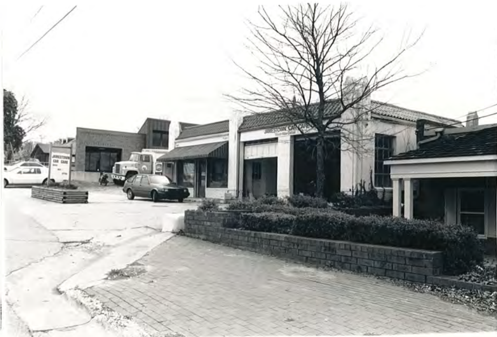
81. (B) Standard Oil Station, setting, view to NE
