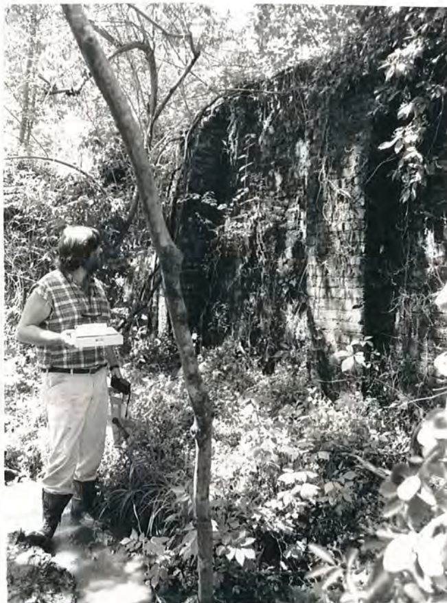
100. (D) High Point Waterworks, basin wall, view to N
