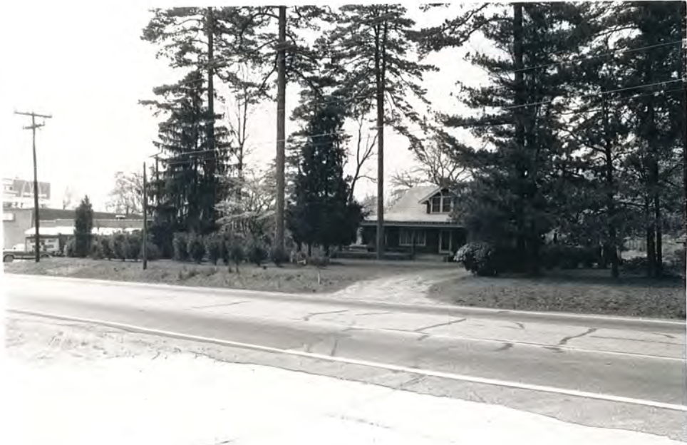
45. (A) Jamison-Ward House, setting, view to NW
