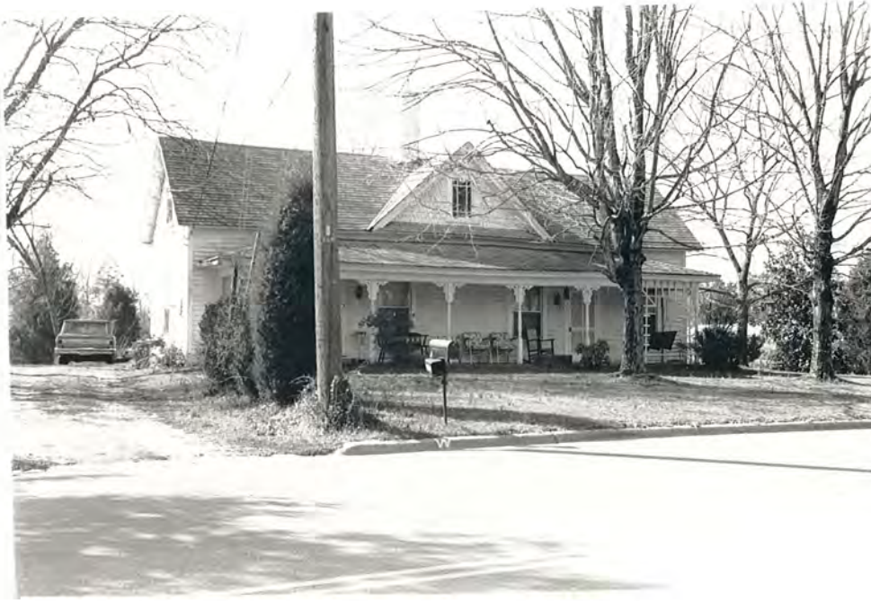
103. (A) House, overall view to NW
