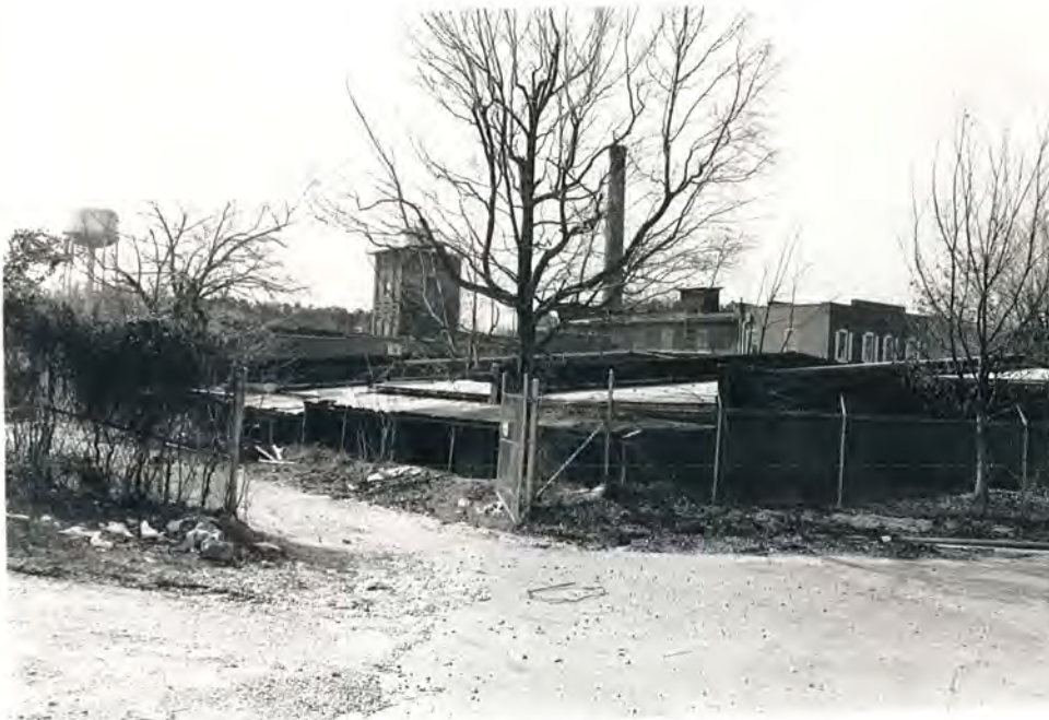
29. (A) Oakdale Cotton Mill Village Historic District, overall view of Mill to SW
