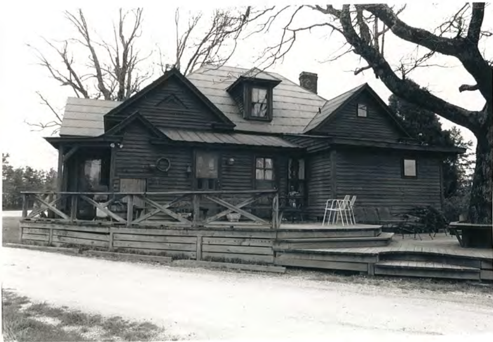
102. (B) House, rear, view to N
