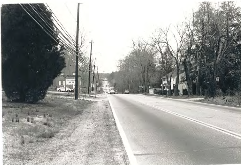
6. Main St. at City Lake Park, view to E
