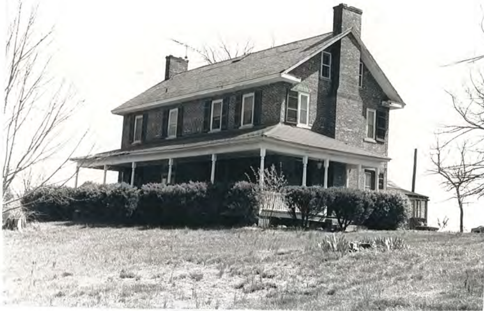
13. (B) Stephen Gardner House and Gardner Hill Gold Mine Site, house, view to SE
