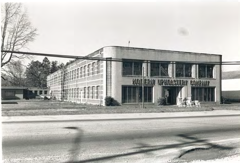
107. (A) Modern Upholstery Company, overall view to N
