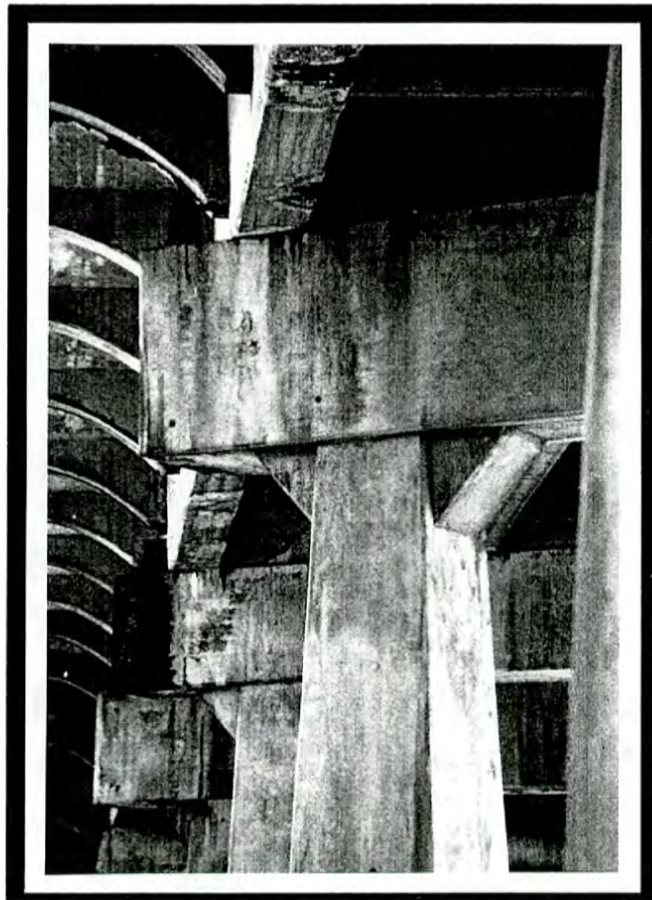
Plate VII.44 McDowell Street Viaduct (# 1) Structure of Bridge
