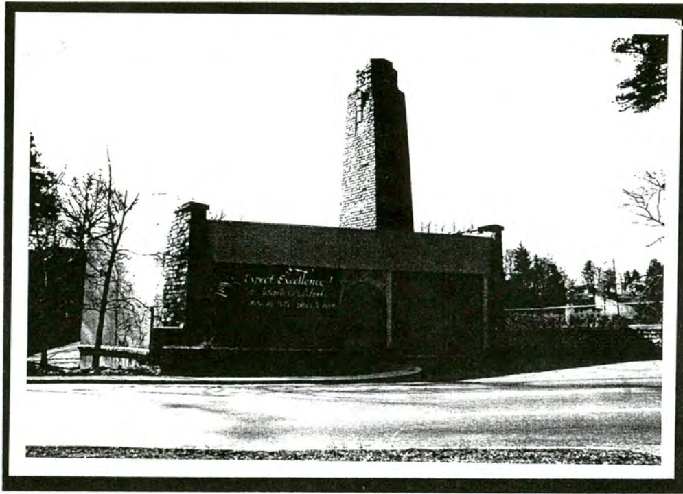
Plate VII.40 Asheville High School Power House (# 4)
