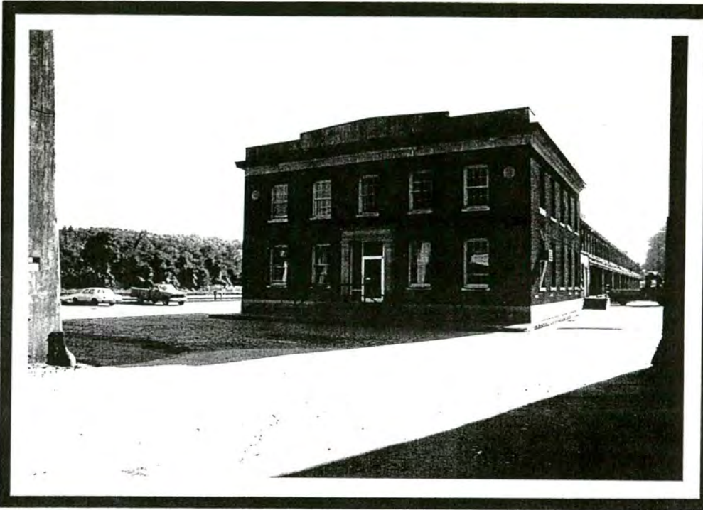
Plate VII.48 Southern Railway Freight Depot (# 41), 33 Meadow Road
