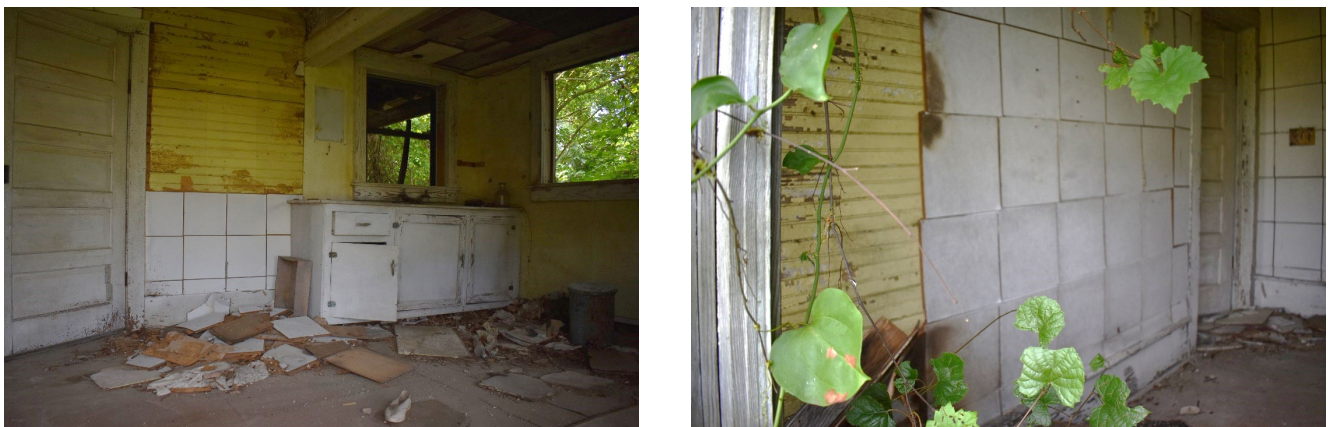
Figure 33: Left and right, interior views through rear ell windows of the house, facing southeast.
