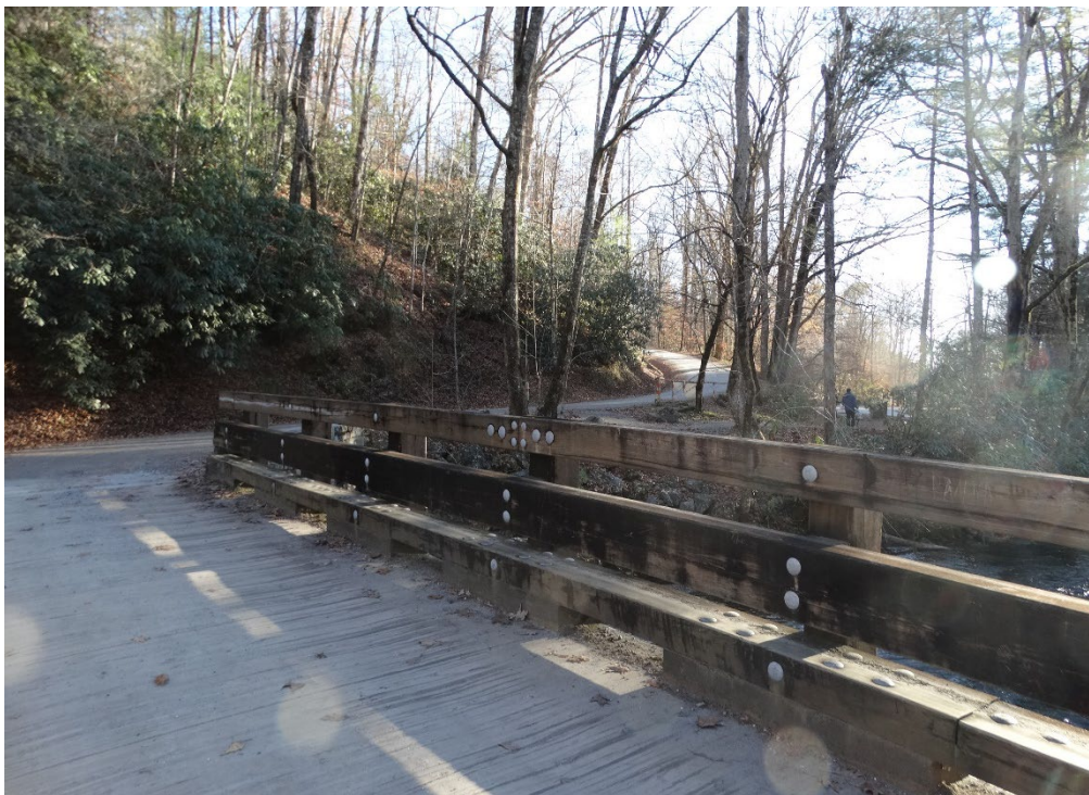
Figure 33: Toms Branch Bridge deck and rail, facing southeast (QE 2020).
