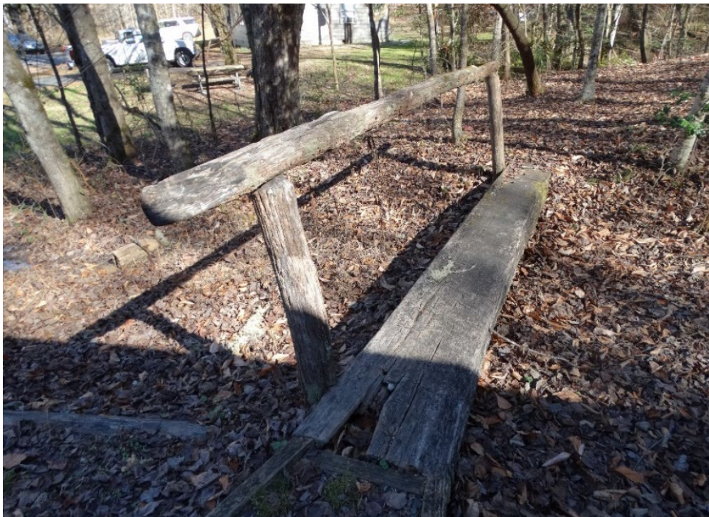
Figure 17: Split log bridge (QE 2020).
