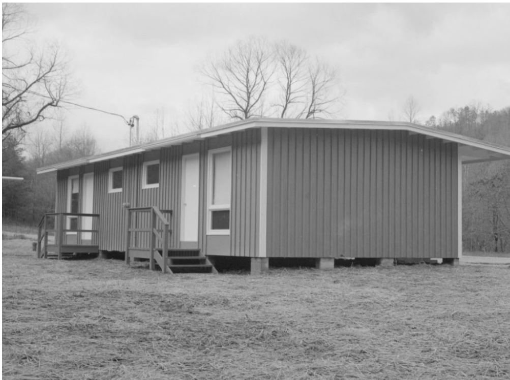
Figure 47: Photograph of the multiple dwelling at the Deep Creek Campground, 1961 (demolished) (Open Parks Network, 1961).
