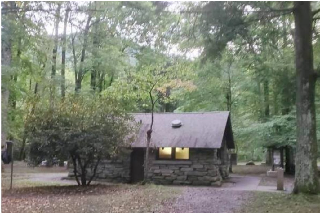
Figure 40: Comparable Example, Smokemont Campground, comfort station (https://www.flashpackingamerica.com/north-carolina-travel/smokemont-campground-smoky-mountains/) .
