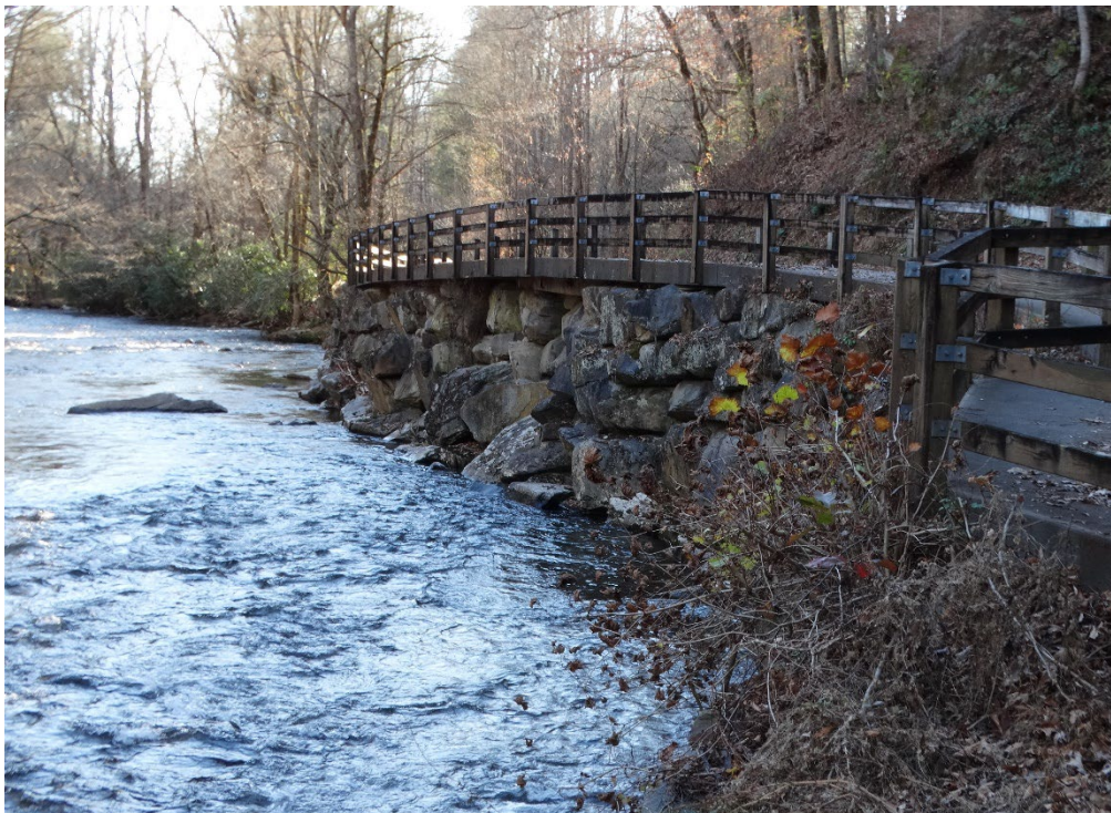
Figure 37: Stone retaining wall at West Deep Creek Road (QE 2020).
