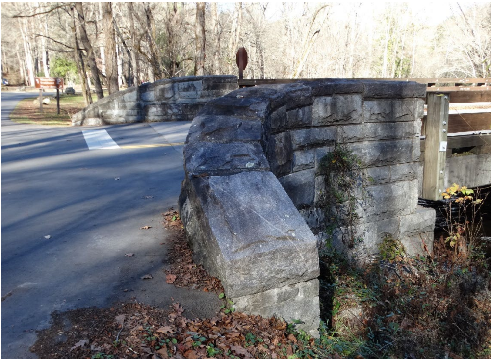
Figure 35: Deep Creek Campground Entrance Bridge (QE 2020).
