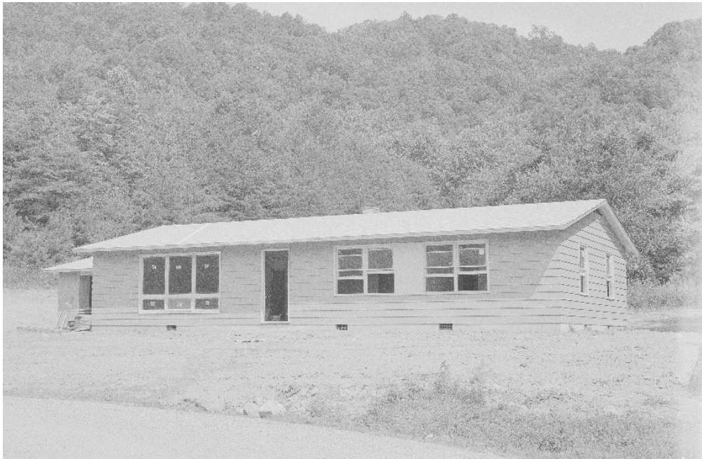
Figure 48: Photograph of the employee residence, 1961 (Open Parks Network, 1961).
