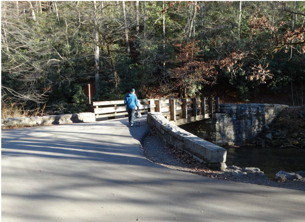
Figure 30: Toms Branch Bridge west abutments, facing northeast (QE 2020).
