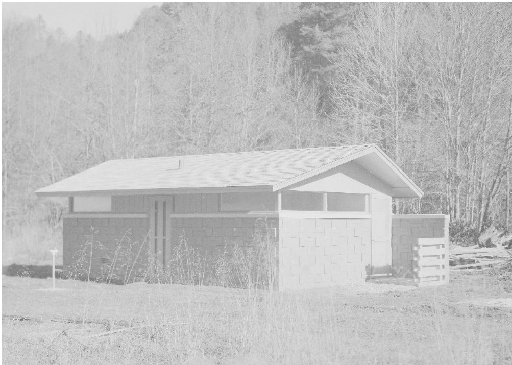
Figure 46: Photograph of the campground comfort station, 1960 (Open Parks Network, 1960).
