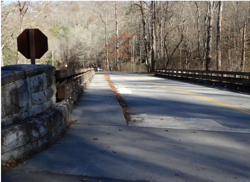
Figure 36: Deep Creek Campground Entrance Bridge, facing east (QE 2020).
