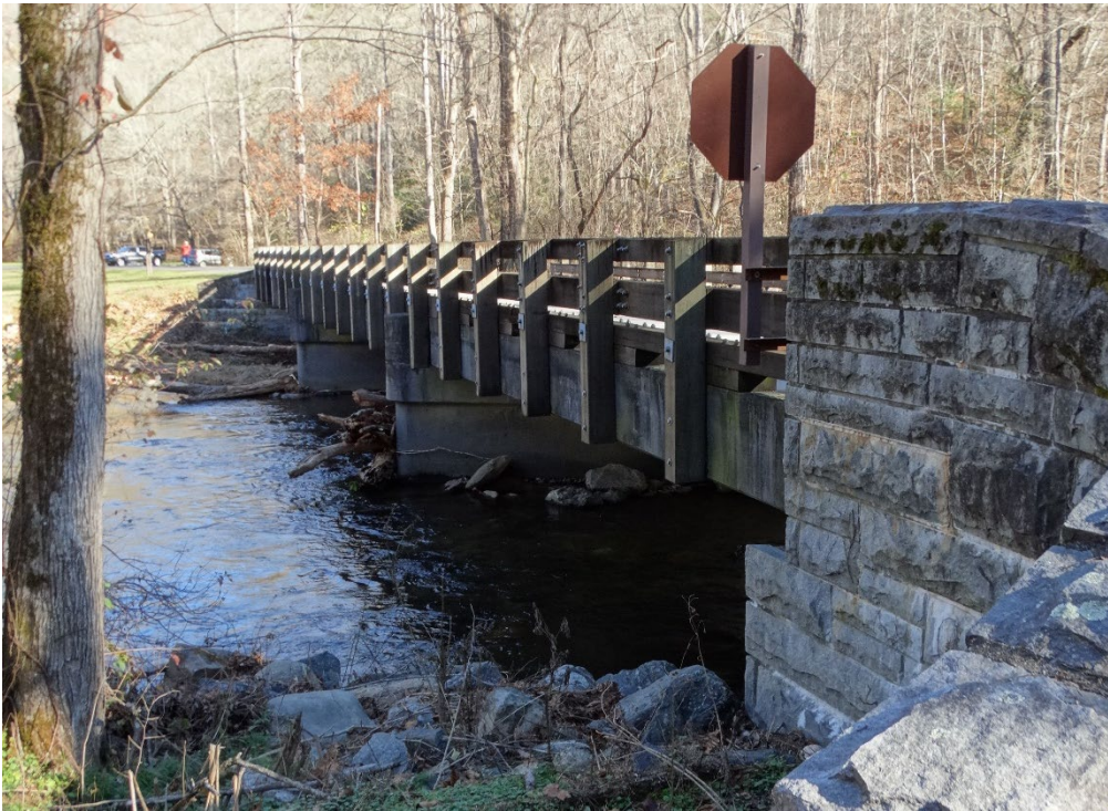
Figure 34: Deep Creek Campground Entrance Bridge (QE 2020).
