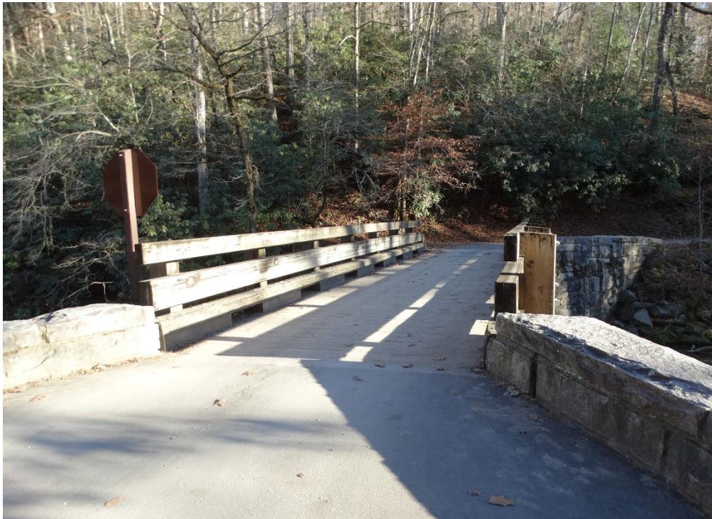
Figure 32: Toms Branch Bridge facing east (QE 2020).
