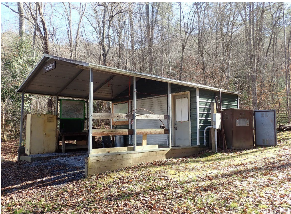
Figure 29: Maintenance Trail Building, looking east (QE 2020).
