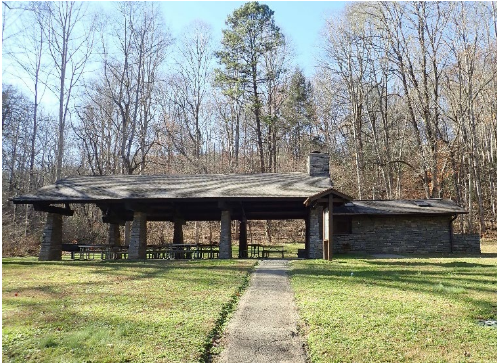
Figure 24: Picnic Pavilion 349/63524, looking west (QE 2020).
