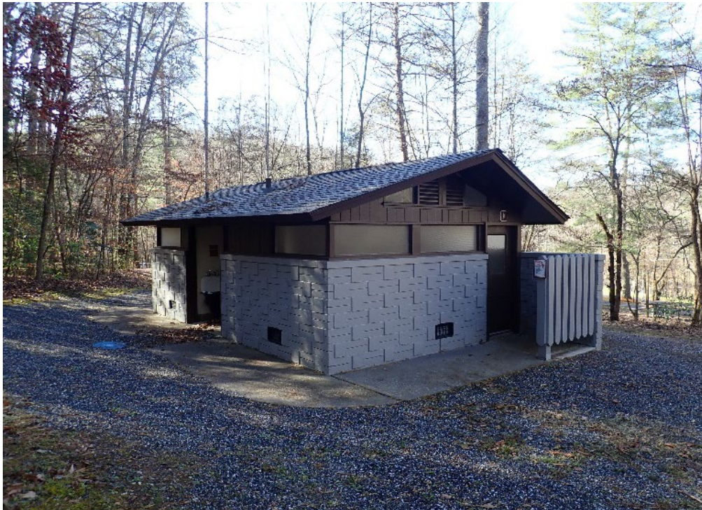
Figure 22: Comfort Station 559/63530, looking southwest (QE 2020).
