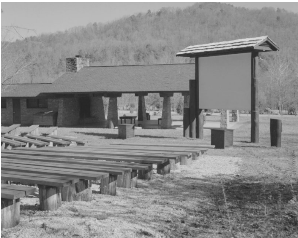
Figure 49: Photograph of the amphitheater and projection screen (demolished), ca. 1963. The 1954 Picnic Pavilion is in the background (Open Parks Network, 1954).
