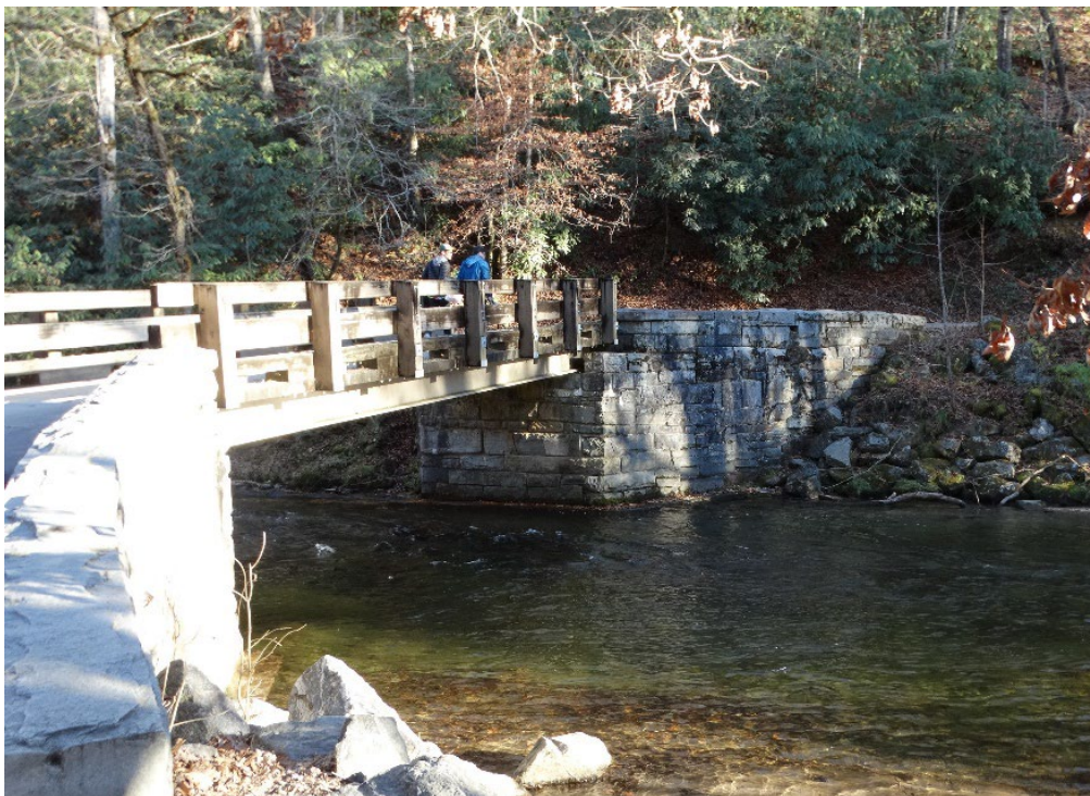
Figure 31: Toms Branch Bridge facing northeast (QE 2020).
