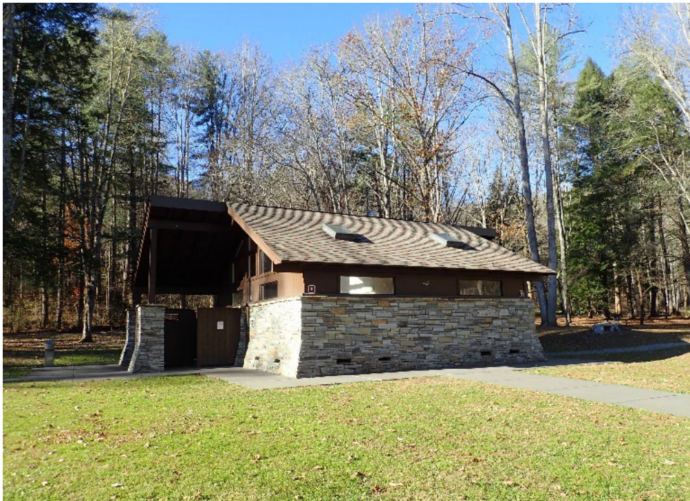
Figure 23: Comfort Station 462/63527, looking northwest (QE 2020).
