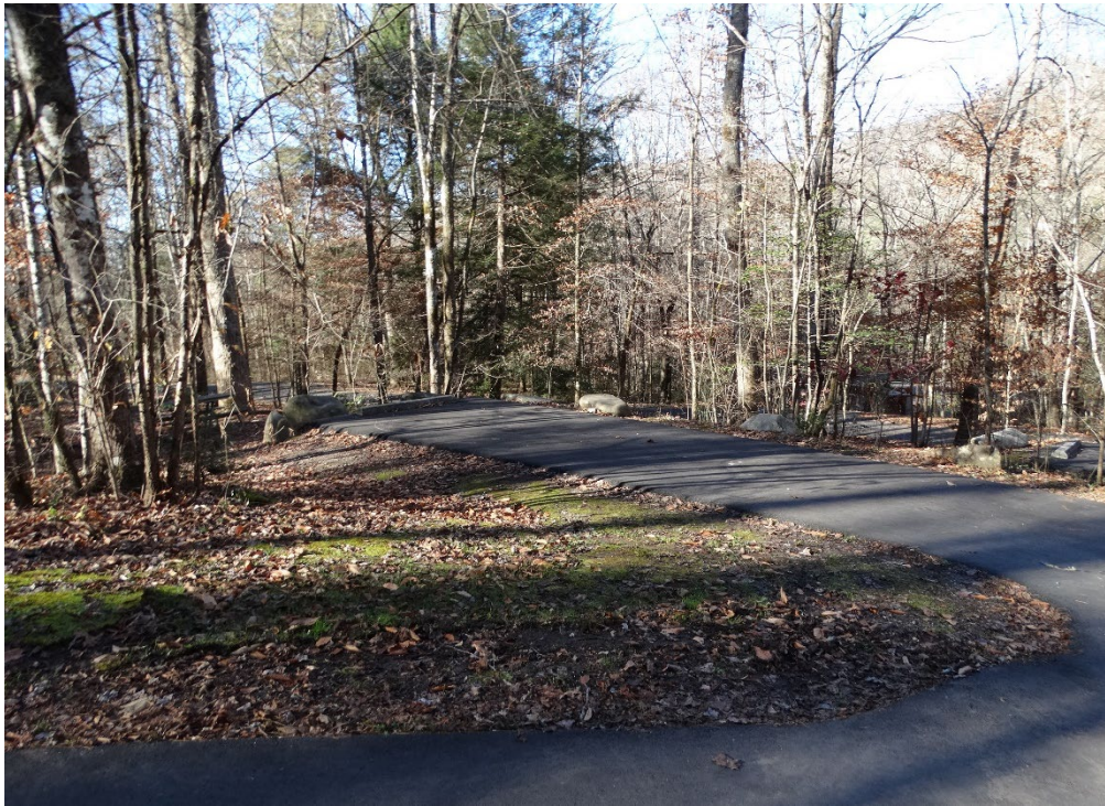
Figure 10: Primary campground campsite with angled single-spur parking with rocks at edge of paving (QE 2020).
