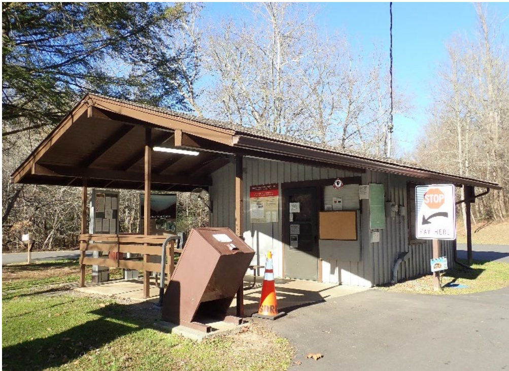
Figure 25: Campground Kiosk 648/63522, looking northeast (QE 2020).
