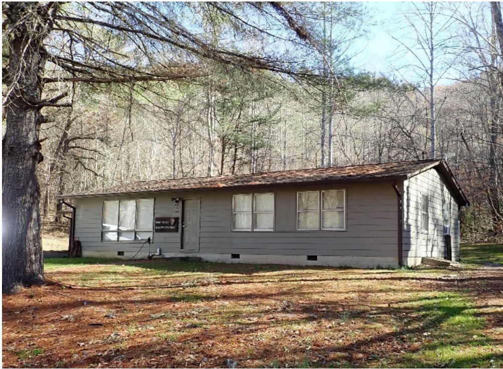
Figure 26: Ranger and Maintenance Office 437/63491, looking east (QE 2020).
