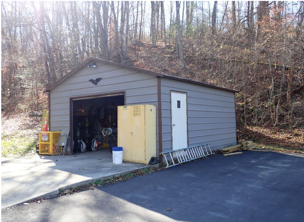
Figure 28: Maintenance Storage Building 316/63523, looking south (QE 2020).
