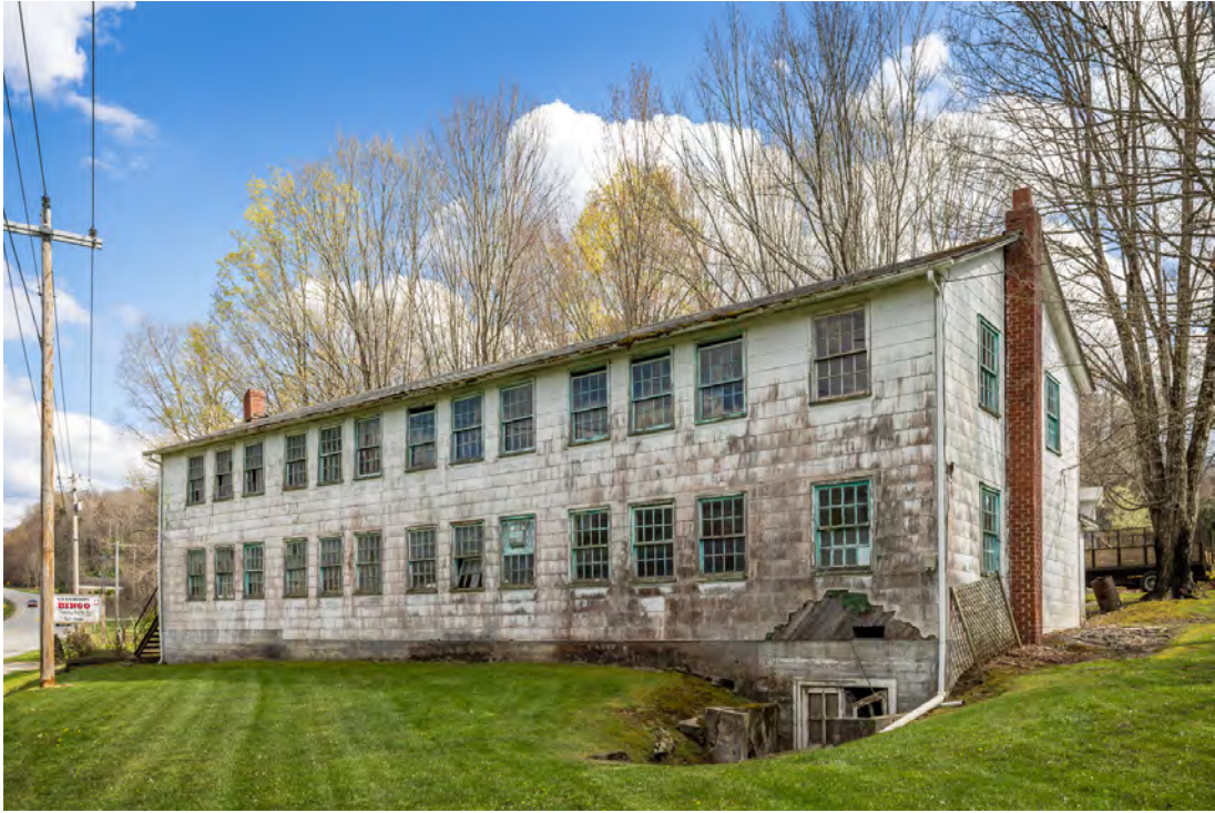
Agriculture building, view to the southeast
