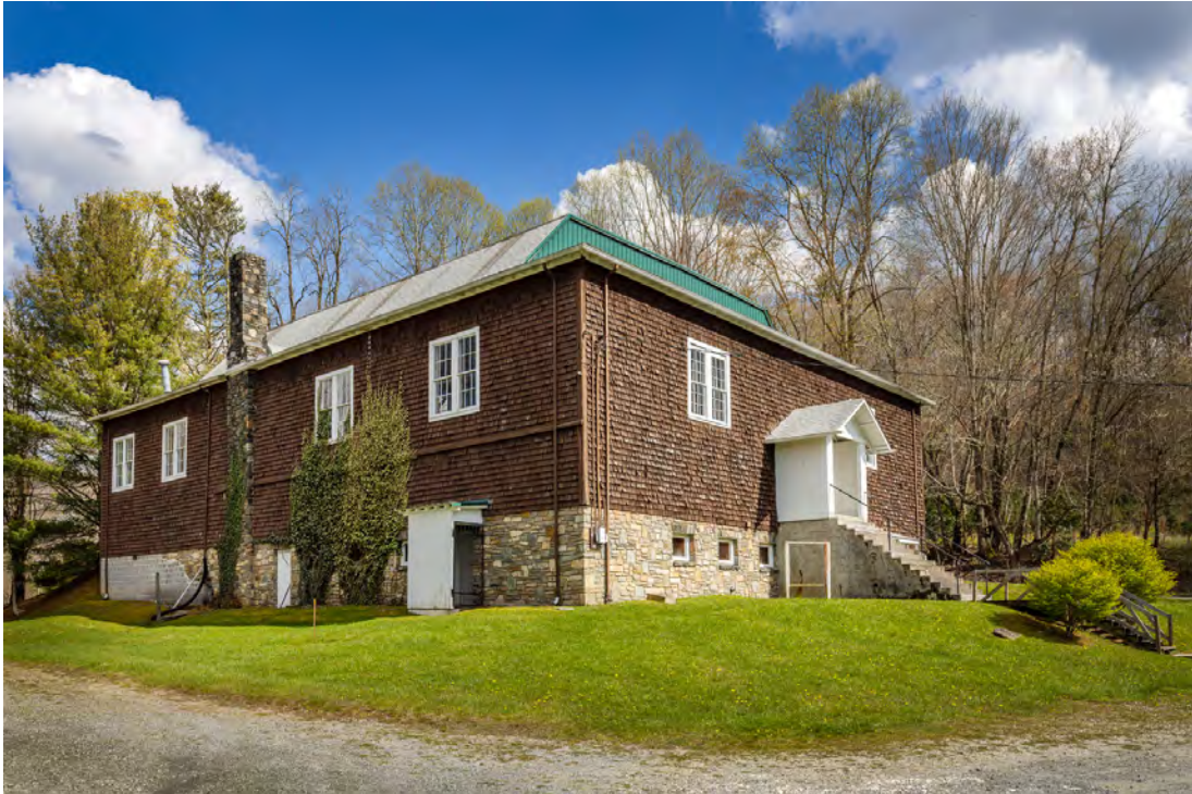
Gymnasium, view to the south-southeast
