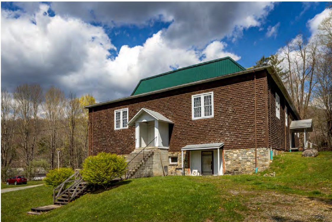
1937 gymnasium, view to the northeast
