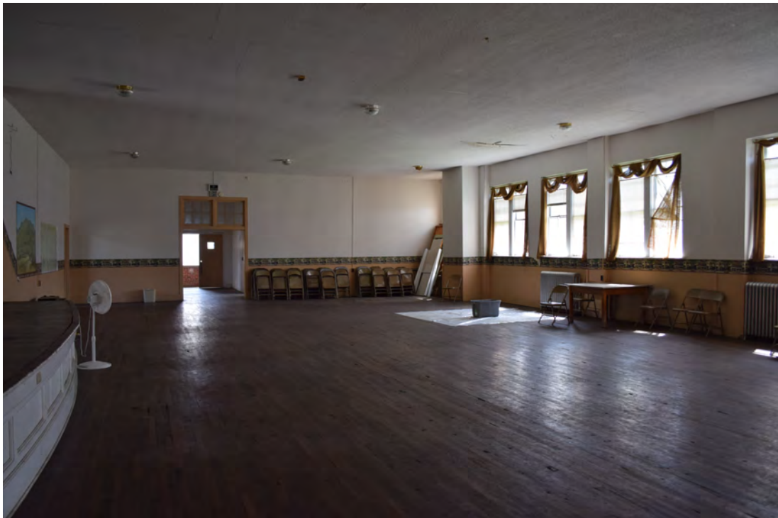
Upper story auditorium with stage to the left, view to the south-southwest
