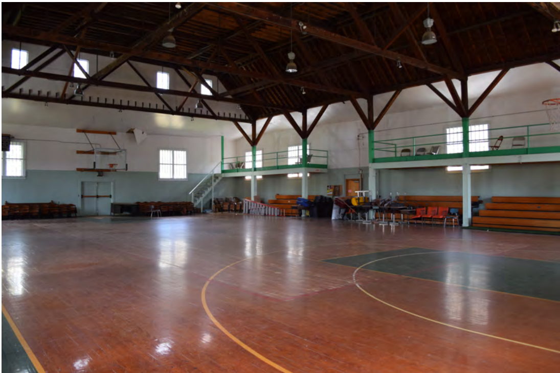
Gymnasium interior, view to the southeast
