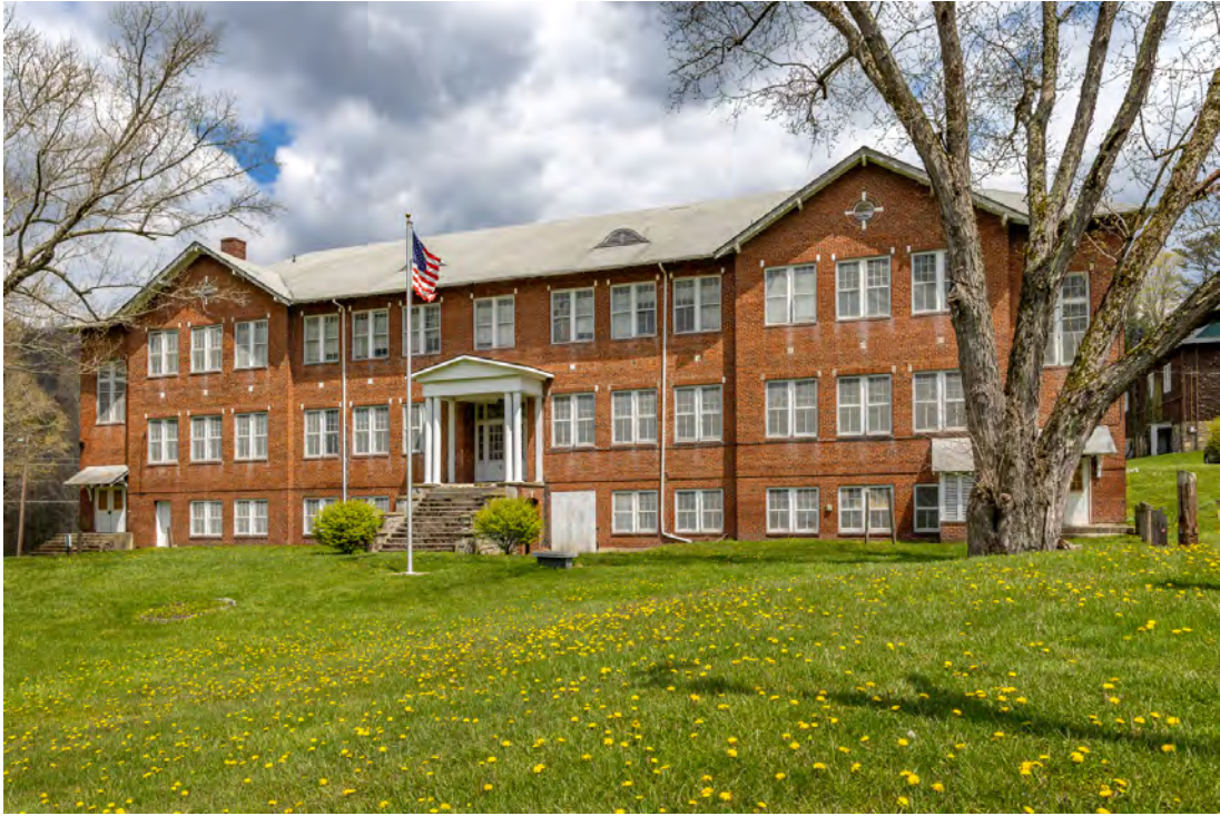
Classroom building facade, view to the east-northeast
