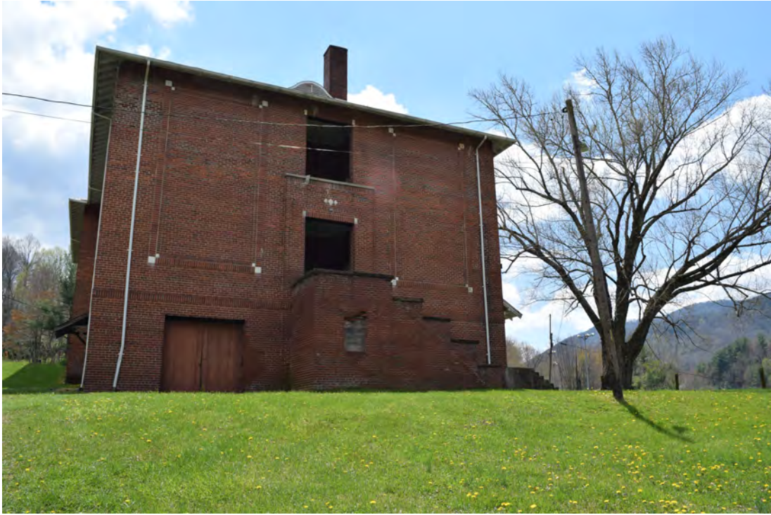
Classroom building's north end, view to the south-southwest
