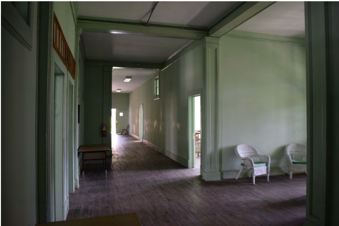
Classroom building main level, main entrance to the right looking down north-south corridor, view to the south
