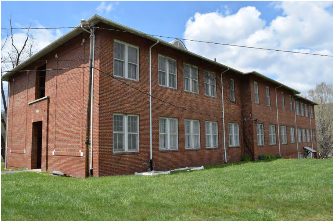
Classroom building rear elevation (east elevation) and south end, view to the northwest
