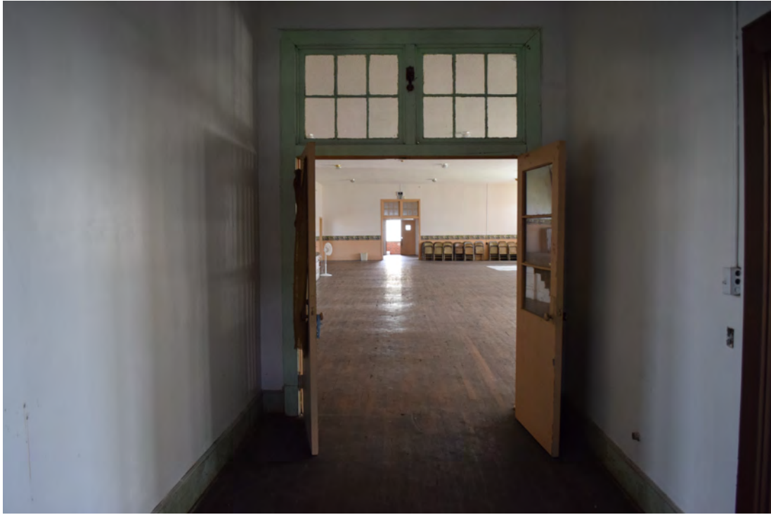
Upper story corridor looking into auditorium, view to the south
