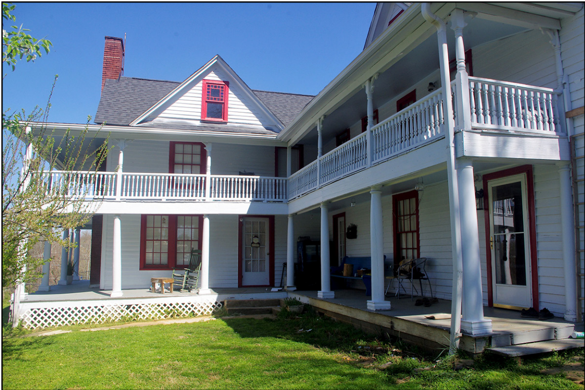
PLATE 2: Burch-Mathis House (YD0617), South Elevation of Main Block and West Elevation of Rear Ell, Yadkin County, North Carolina
