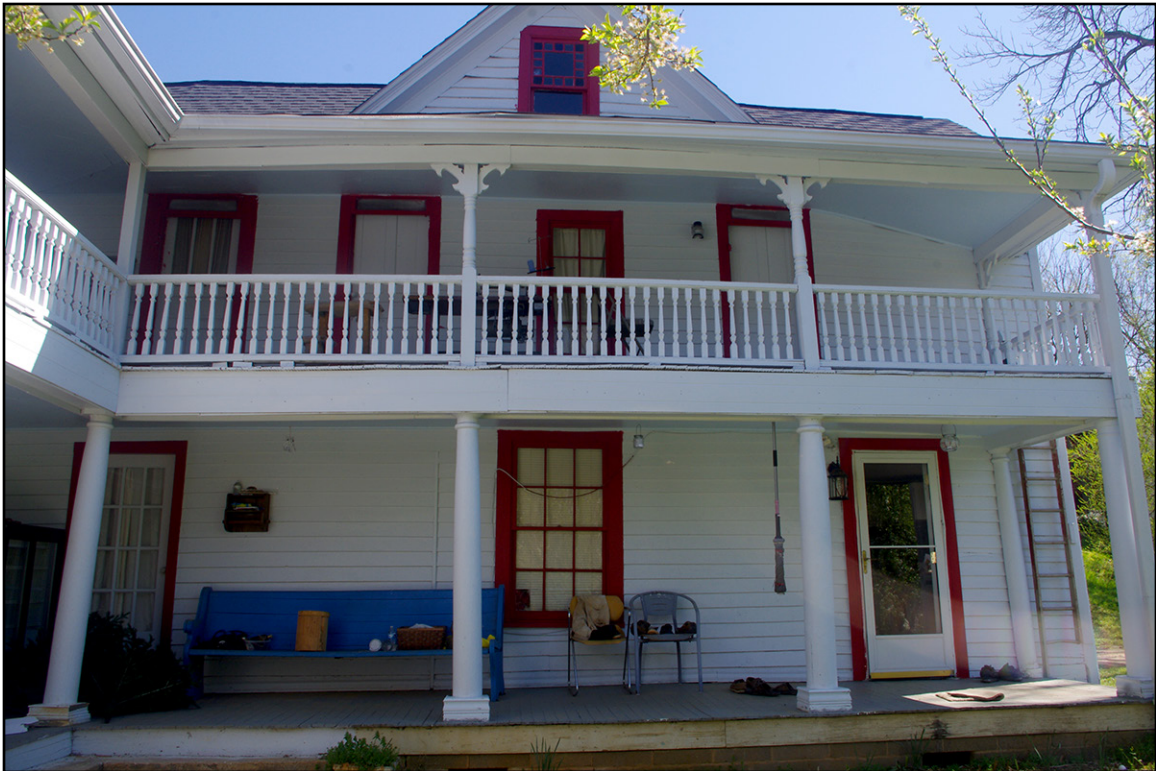
PLATE 5: Burch-Mathis House (YD0617), West Elevation of Rear Ell, Yadkin County, North Carolina
