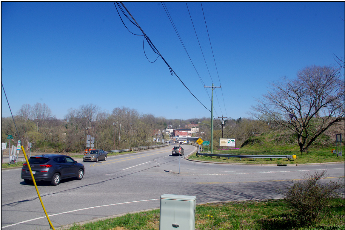
PLATE 20: Gwyn-McNeill Bridge at W. Main Street from Burch-Mathis House Property, Facing North, Yadkin County, North Carolina
