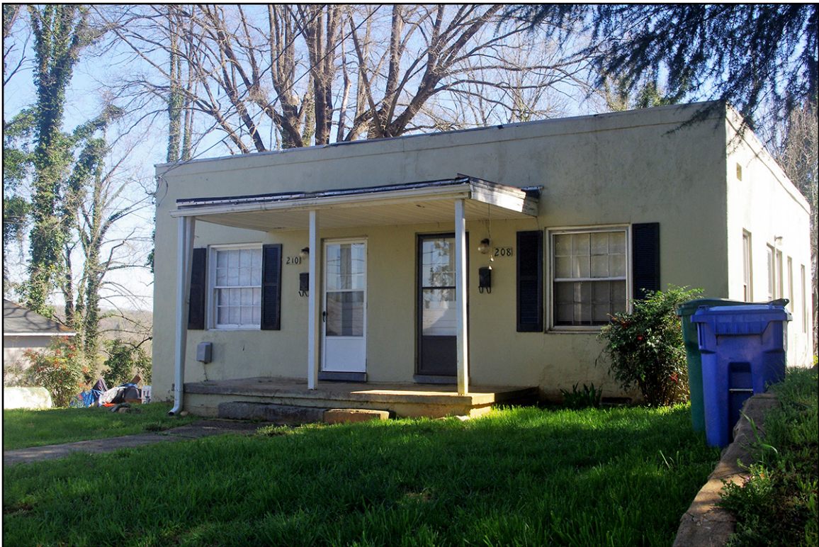
PLATE 28: Duplex at 210-208 Cherry Street (YD0723), West Elevation, Yadkin County, North Carolina
