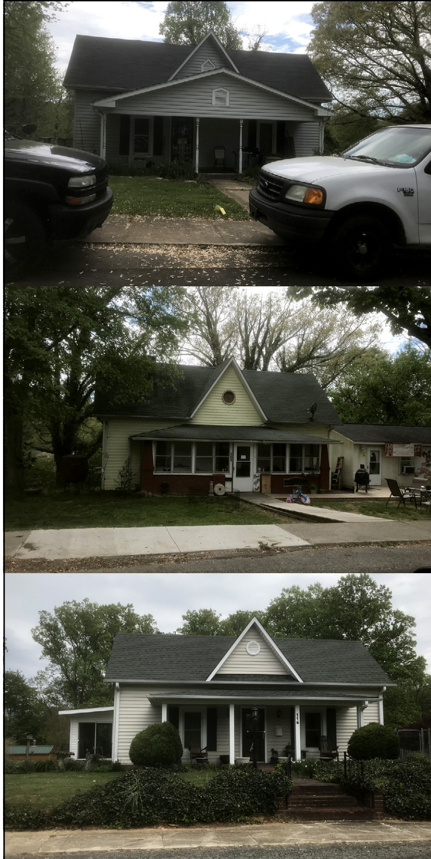
PLATE 36: Typical One-story Frame Cottages Built Along Cherry Street Potentially for Working-class Families, ca. 1915-1930
