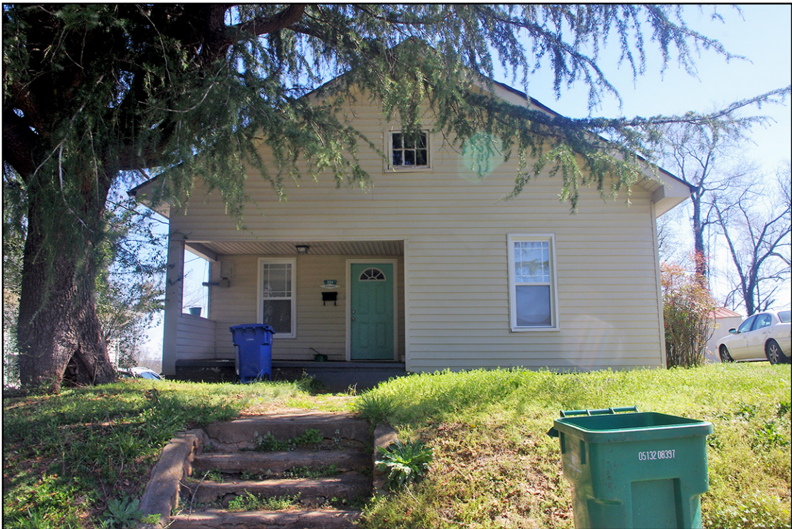
PLATE 30: House at 204 Cherry Street (YD0725), West Elevation, Yadkin County, North Carolina
