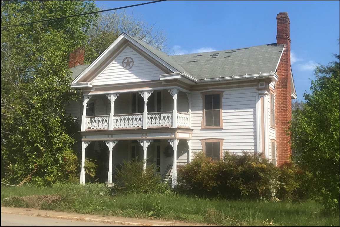
PLATE 17: James A. Smitherman House (YD0339), South Elevation, East Bend, Yadkin County, North Carolina
