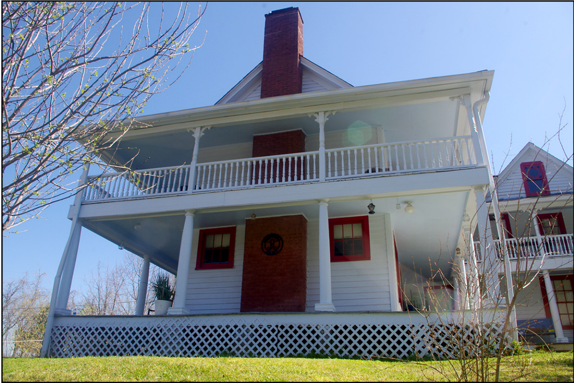
PLATE 3: Burch-Mathis House (YD0617), West Elevation, Yadkin County, North Carolina
