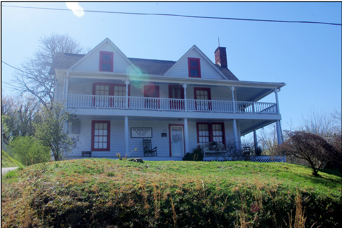
PLATE 4: Burch-Mathis House (YD0617), North Elevation (façade), Yadkin County, North Carolina
