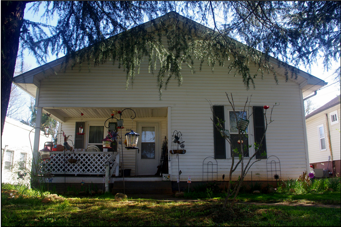
PLATE 29: House at 206 Cherry Street (YD0724), West Elevation, Yadkin County, North Carolina
