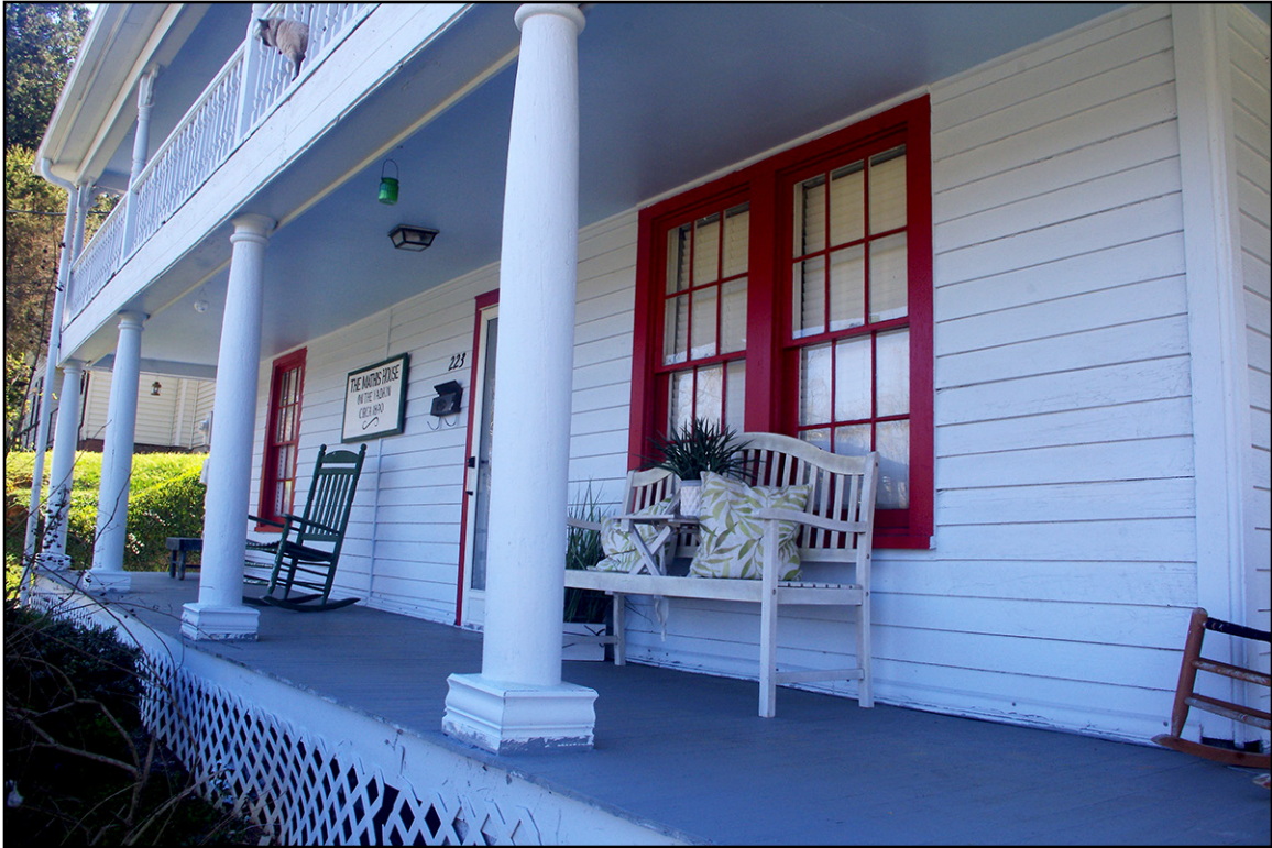
PLATE 19: Burch-Mathis House (YD0617), Detail of First-story Replacement Porch Columns, North Elevation, Yadkin County, North Carolina
