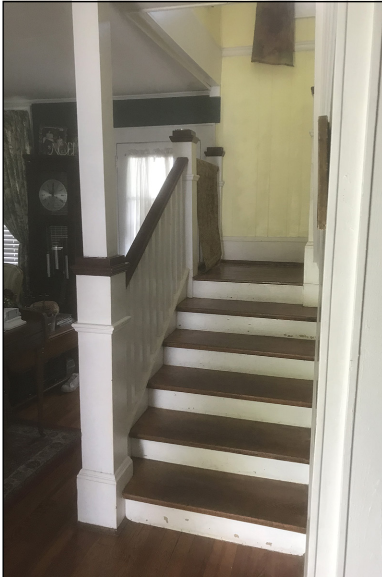
PLATE 9: Burch-Mathis House (YD0617), Interior Entryway from South Elevation, Facing North, Yadkin County, North Carolina
