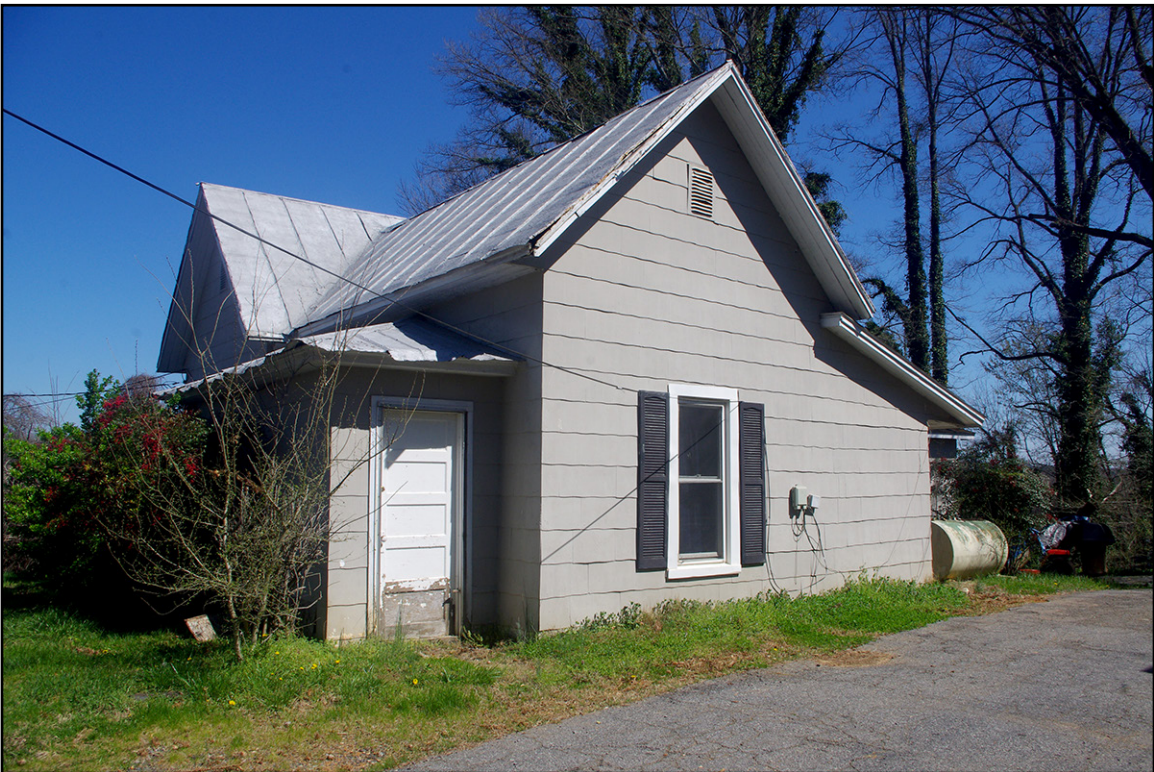
PLATE 26: House at 212 Cherry Street (YD0678), South Elevation, Yadkin County, North Carolina
