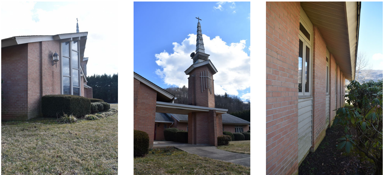
Figure 88: Left, detail of stain glass windows and projecting eaves on front elevation, looking south; middle, detail view of belltower, looking south; right, detail view of overhanging eaves and brick pilasters along north elevation of sanctuary block, looking west.
