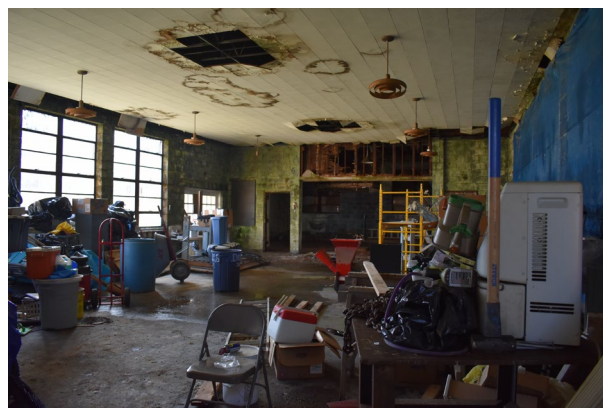
Figure 75: Interior view of cafeteria addition from northern door, looking south.
