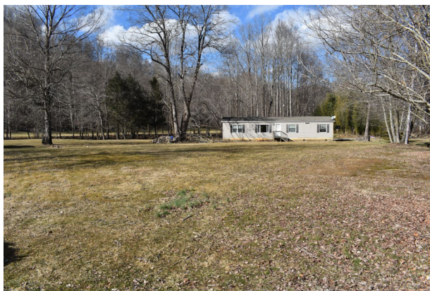
Figure 27: Above, south elevation of Resource J at 181 Jonathan Creek Road, looking north.
