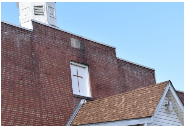
Figure 69: View of decorative brick detailing on front parapet and wall.
