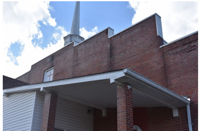
Figure 77: Left, detail view of covered walkway at southwest corner of building connecting original school and cafeteria addition; right, detail view of original brick parapet wall and modern steeple.
