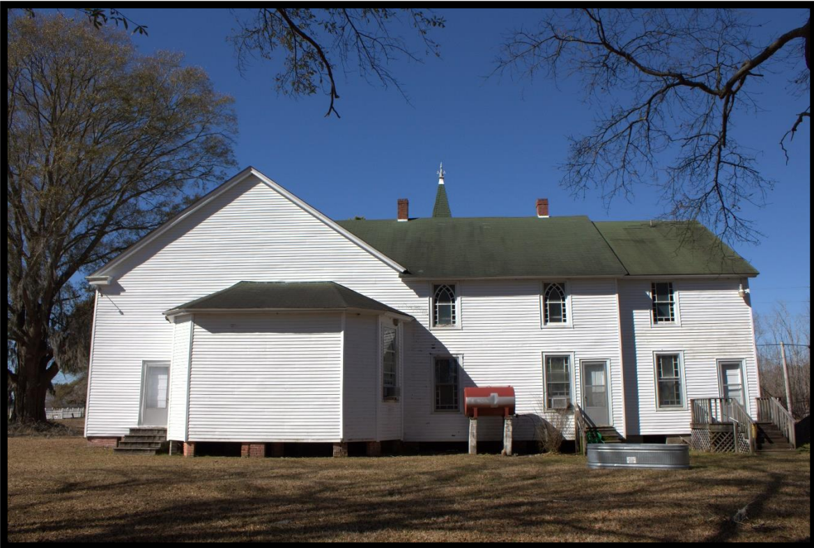
Figure 10: Union United Methodist Church, Looking West.
