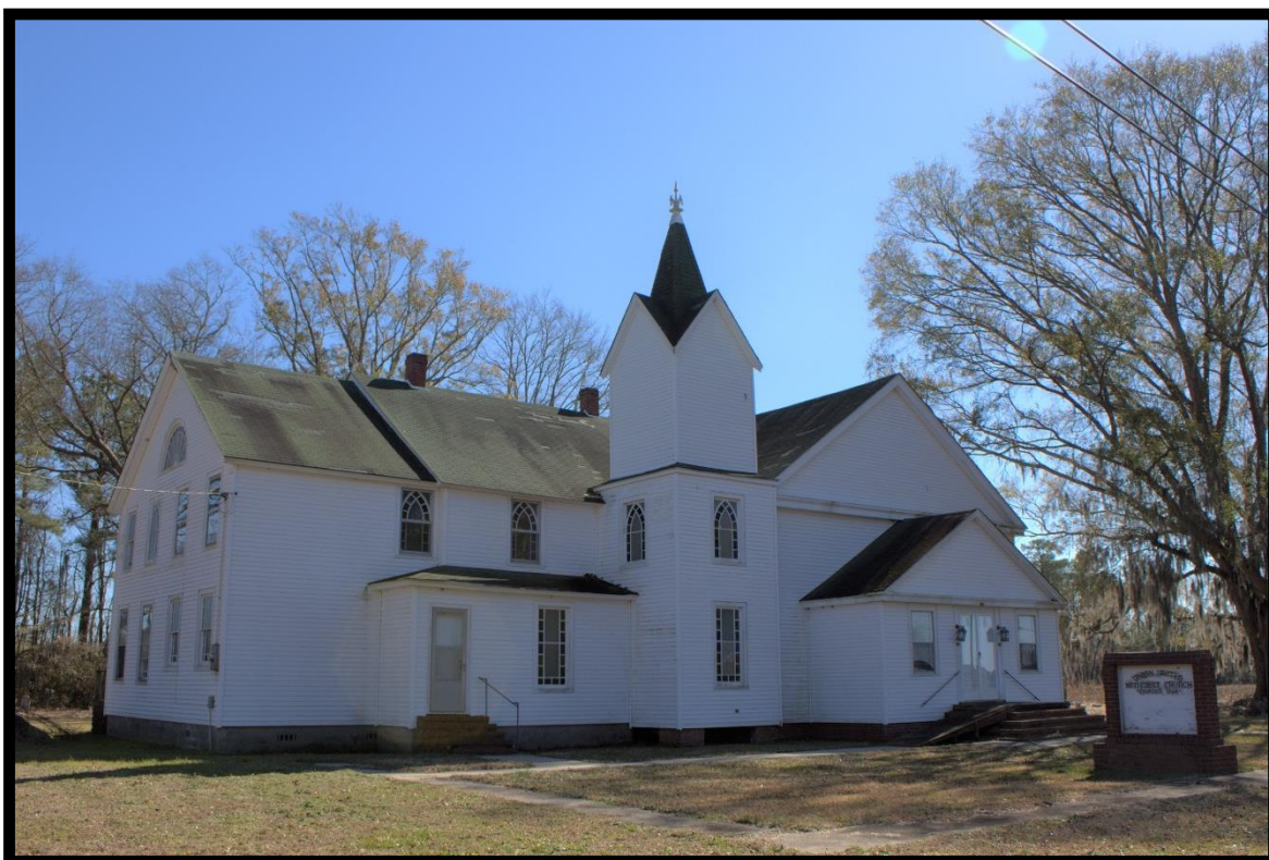
Figure 7: Union United Methodist Church, Looking Southeast.
