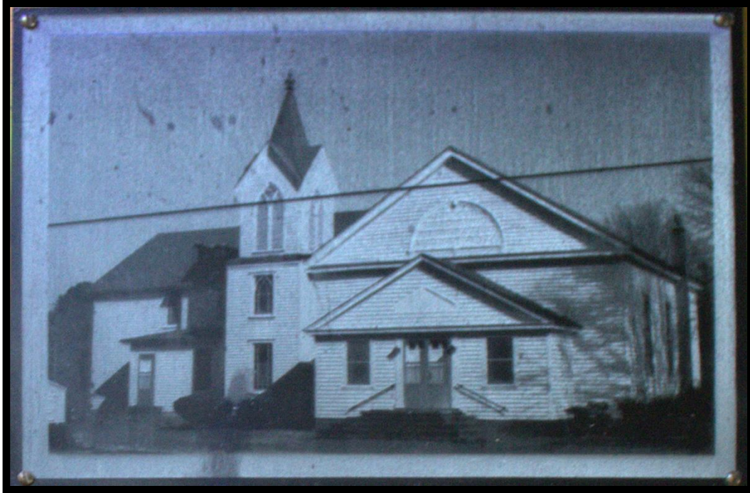
Figure 43: Union United Methodist Church (“Carpet Given By” Plaque at Church, Ca. 1975). Note location of original fanlight and vents on belfry.
