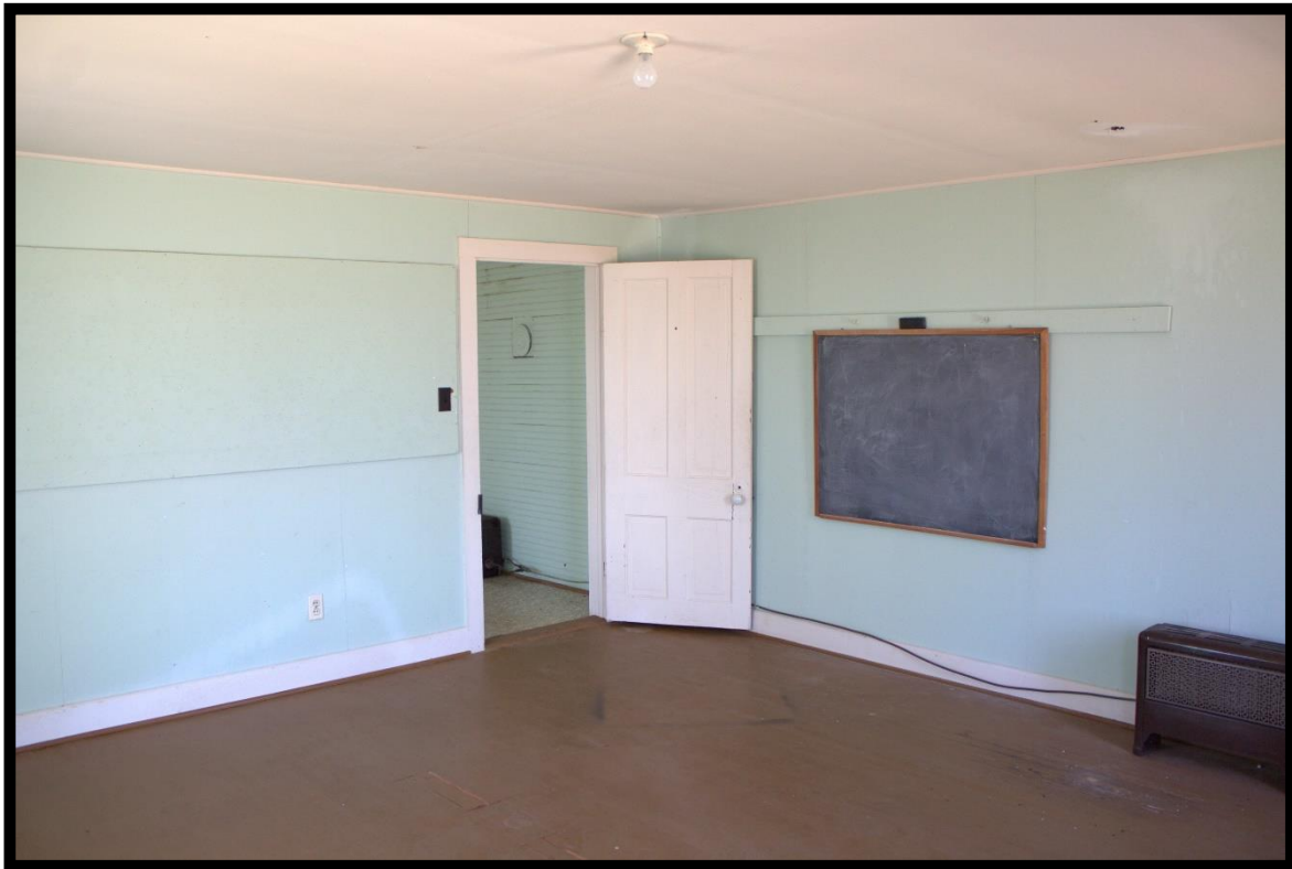
Figure 25: Union United Methodist Church, Interior, Second Floor, 1958 Classroom, Looking Southwest.
