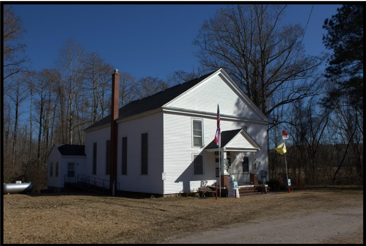
Figure 46: Former Halls Creek United Methodist Church (PK0677), Looking East.
