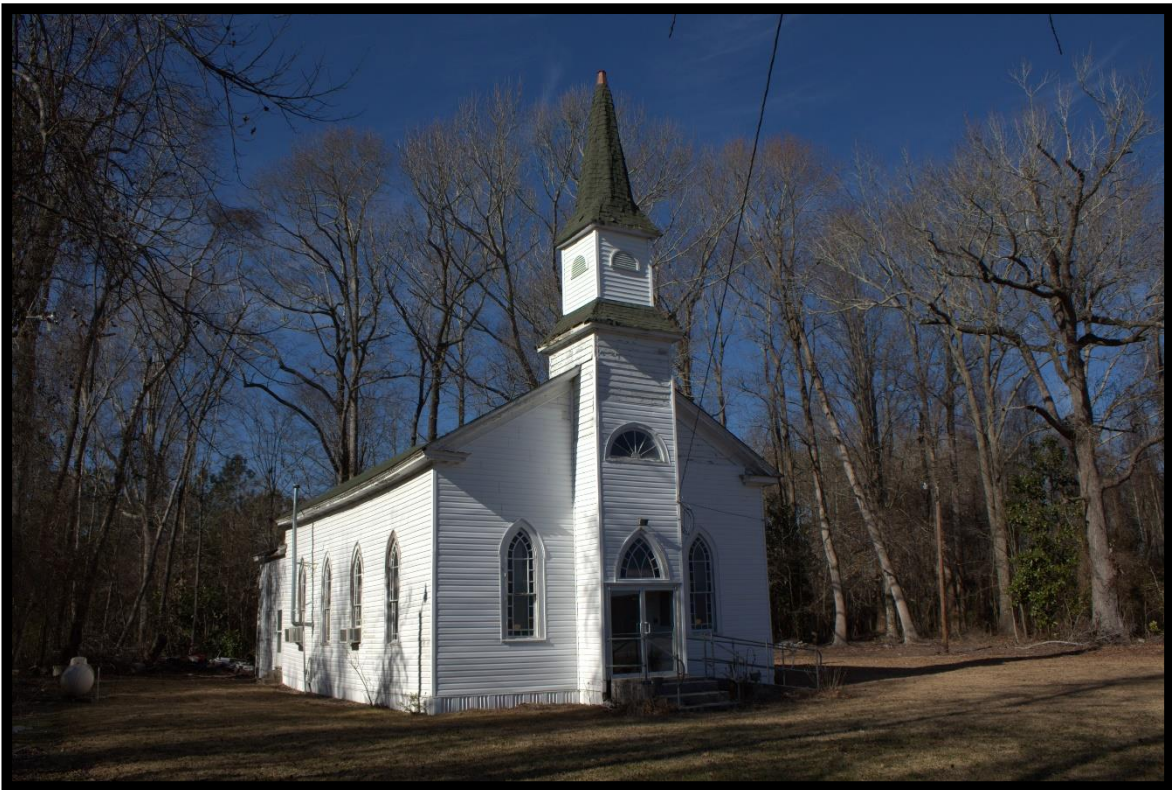
Figure 66: Pitts Chapel A.M.E. Zion Church (PK0760), Looking North.
