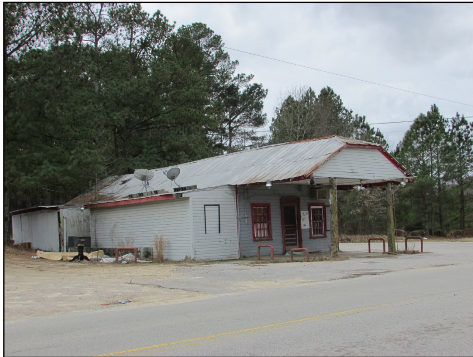
Figure 46. Martin's Store, north and east elevations, looking southwest.
