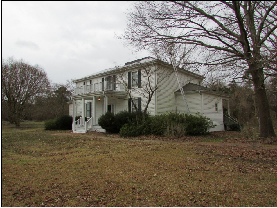
Figure 14. Captain Bailey Williamson House, east and north elevations, looking southwest.
