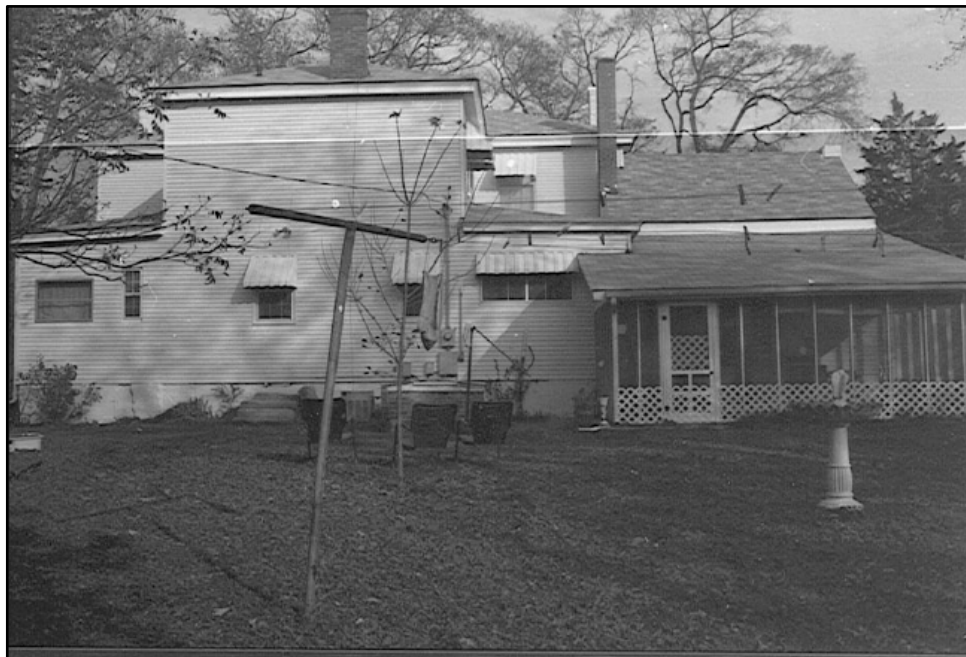
Figure 12. Captain Bailey Williamson House, west (rear) elevation, 1988 photograph showing the original two-story house with the enclosed rear porches flanking the kitchen ell and the one-story dining room and porch addition (now enclosed) to the right (Lally 1988, WA0264).
