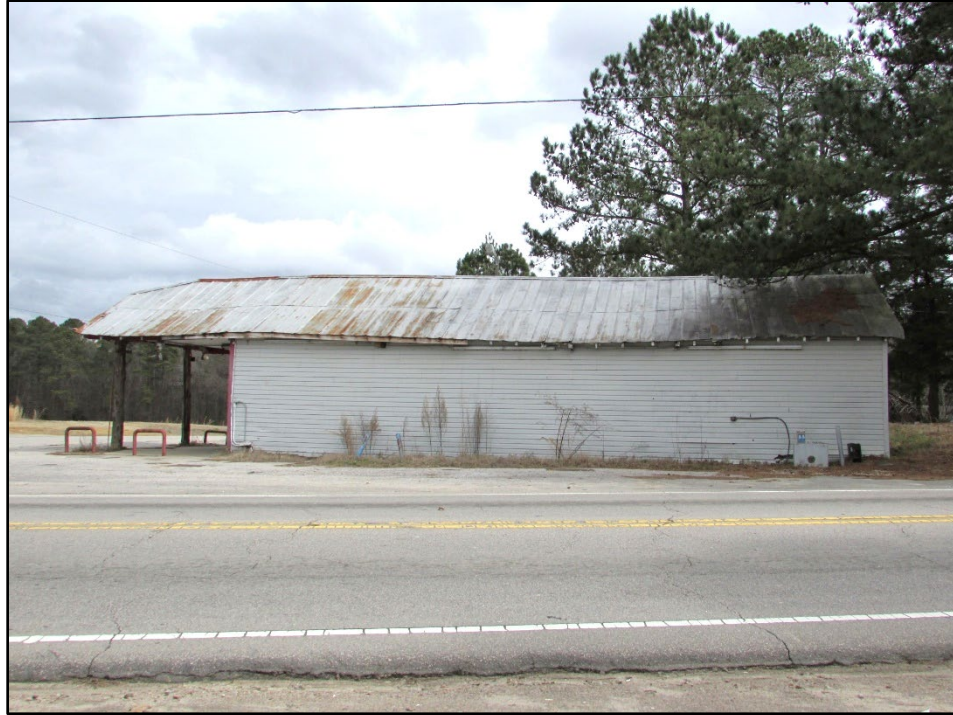
Figure 49. Martin's Store, west elevation, looking east.
