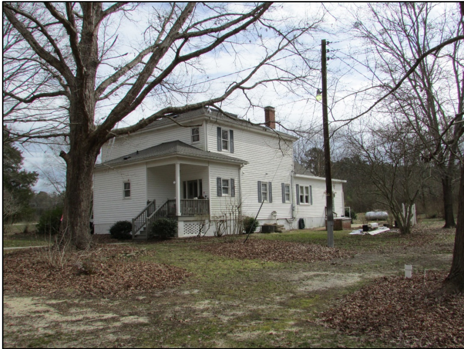
Figure 15. Captain Bailey Williamson House, north and west elevations, looking southeast.
