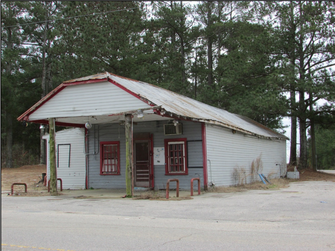
Figure 41. Martin's Store, front (north) and west elevations, looking southeast.
