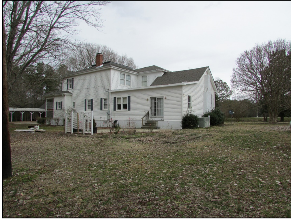
Figure 16. Captain Bailey Williamson House, west and south elevations, looking northeast.
