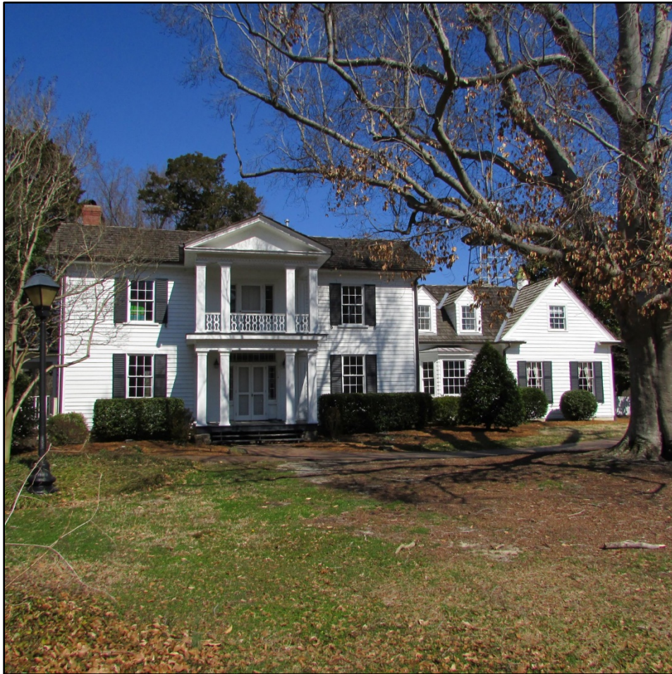
Figure 37. Oak View Plantation (WA1502), looking northeast.
