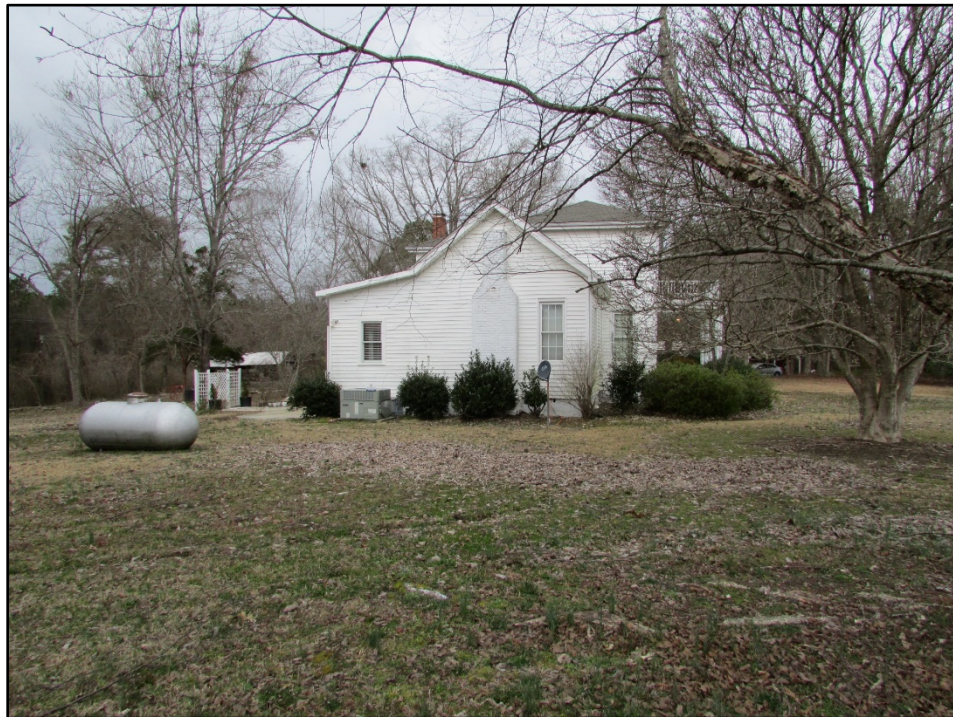
Figure 17. Captain Bailey Williamson House, south elevation, looking north.
