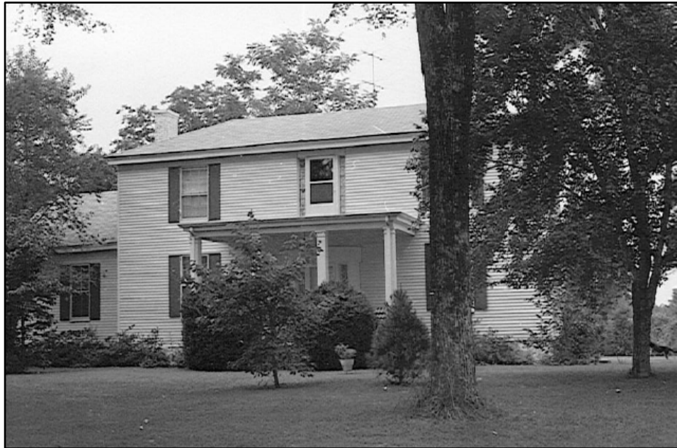
Figure 11. Captain Bailey Williamson House, east (front) elevation, photograph from 1973 survey (WA0264) showing the original two-story mass of the house with the one-story dining room addition to the left (south; Lally, 1988, WA0264).
