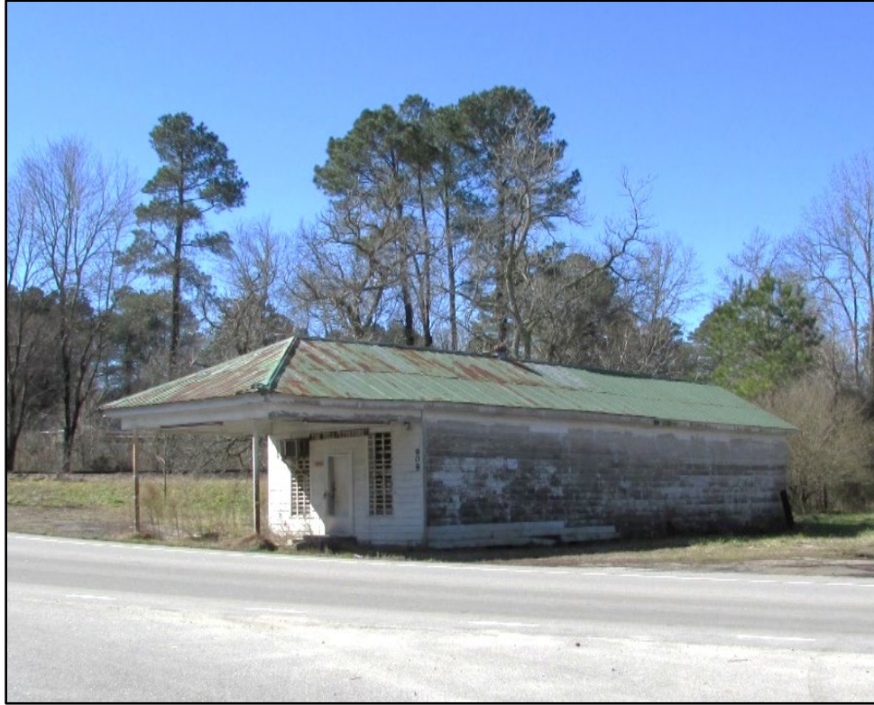
Figure 56. Eagle Rock Store (WA7707), looking southwest.
