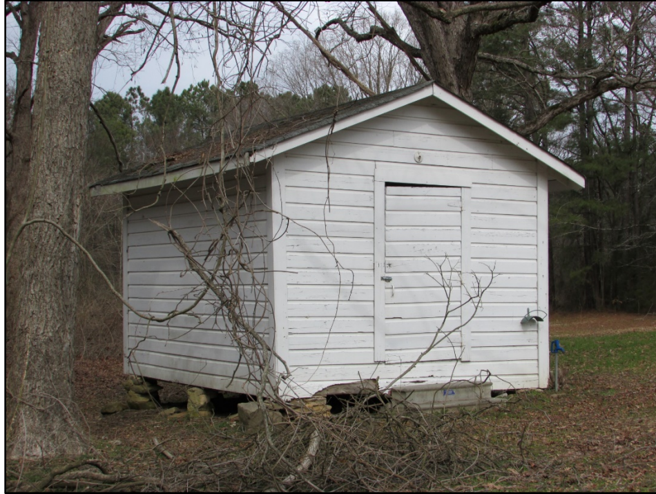
Figure 26. Captain Bailey Williamson House, Granary, west and south elevations, looking northeast.
