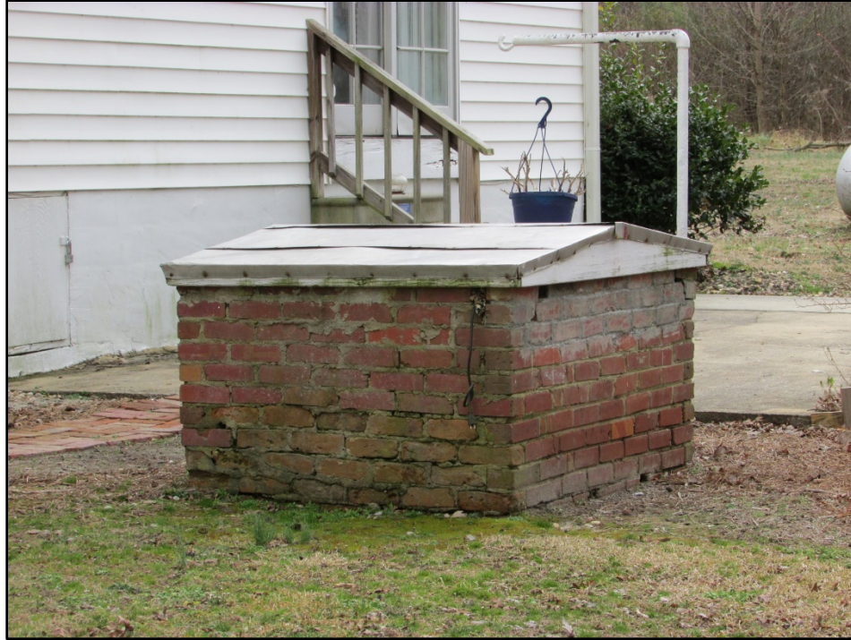
Figure 29. Captain Bailey Williamson House, Pump house, north and west elevations, looking southeast.
