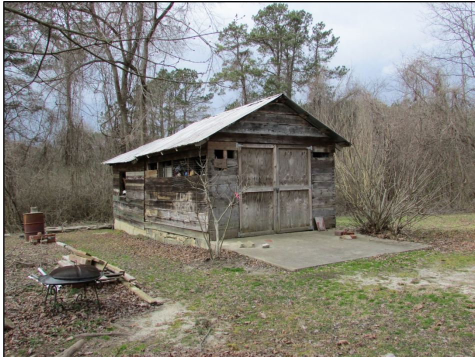
Figure 28. Captain Bailey Williamson House, Garage/Carriage House, east and south elevations, looking northwest.
