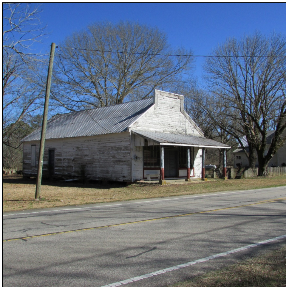
Figure 54. Davis Adcock Store (WA548), looking southeast.
