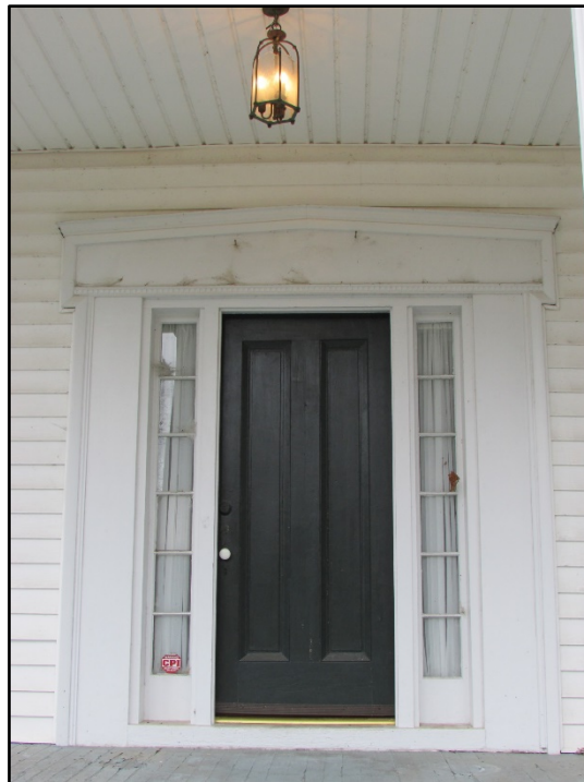
Figure 18. Captain Bailey Williamson House, detail of primary entrance, east façade.
