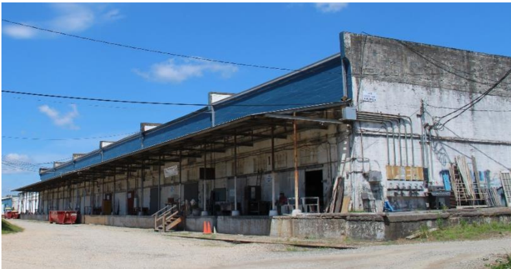
Figure 69. The Raleigh Bonded Warehouse (WA2675) at 1505 Capital Boulevard in Raleigh.
