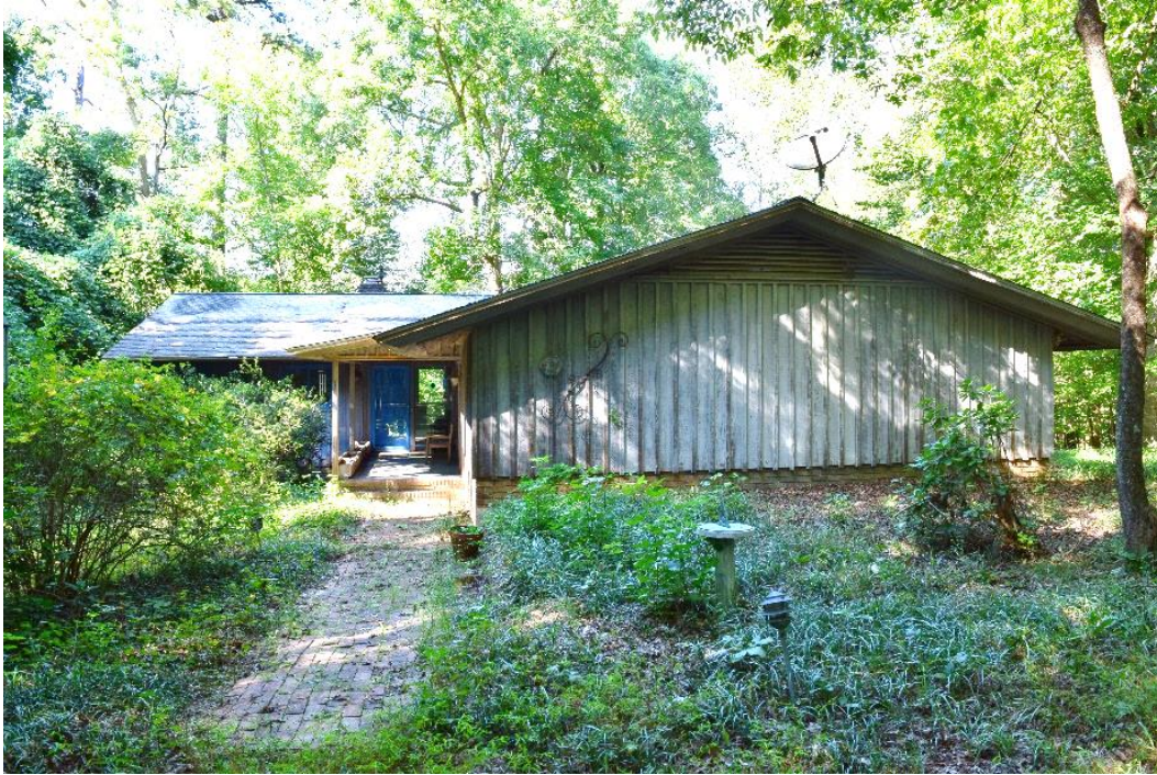
Figure 14. 1967 house, south-facing facade, view facing north..
