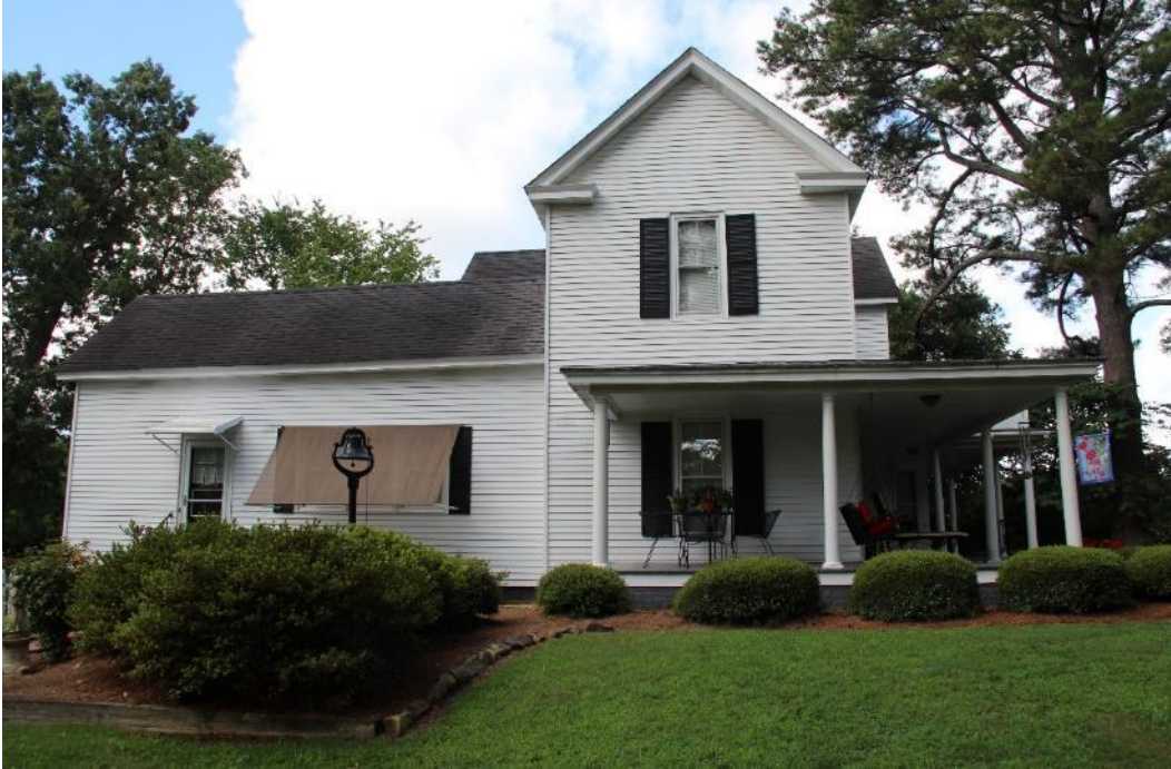
Figure 25. The 1900 Sexton House, northeast elevation, view facing southwest.
