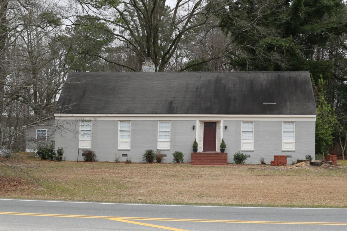
18. House, 7424 Sunset Lake Road, 1960, PIN 0667712621, view facing east.
