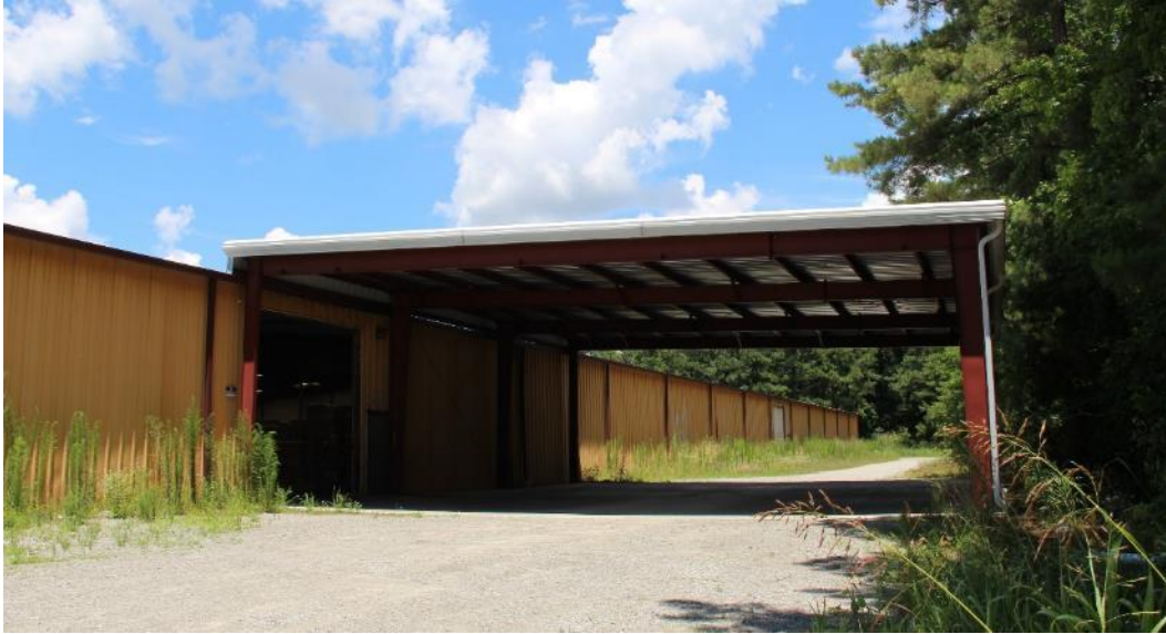
Figure 61. Powell Brothers Warehouse rear (east) elevation, view facing northwest.
