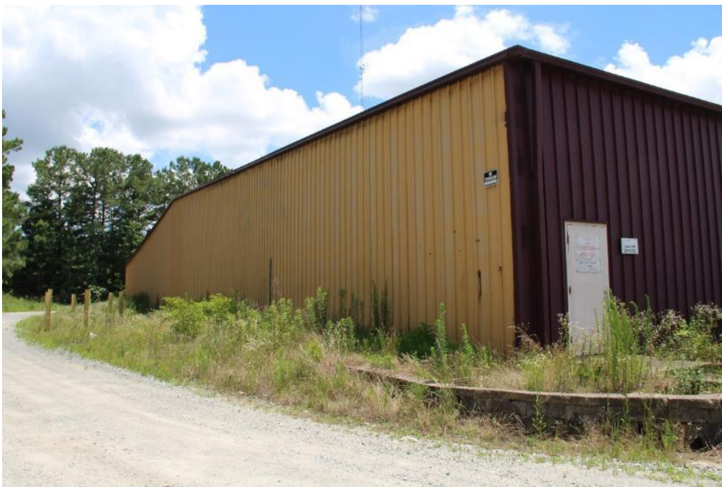
Figure 60. Powell Brothers Warehouse side (north) elevation, view facing southeast.
