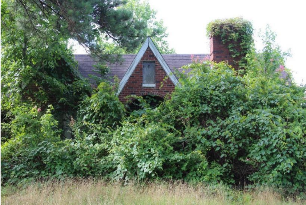
Figure 51. The 1953 Tudor Revival House, north-facing facade, view facing south.
