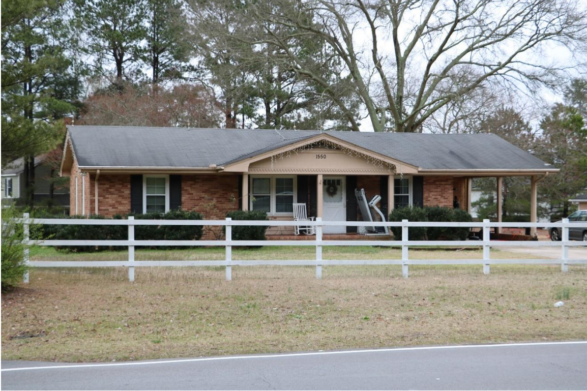
7. House, 1550 N Stewart Street, 1970, PIN 0667249821, view facing east.
