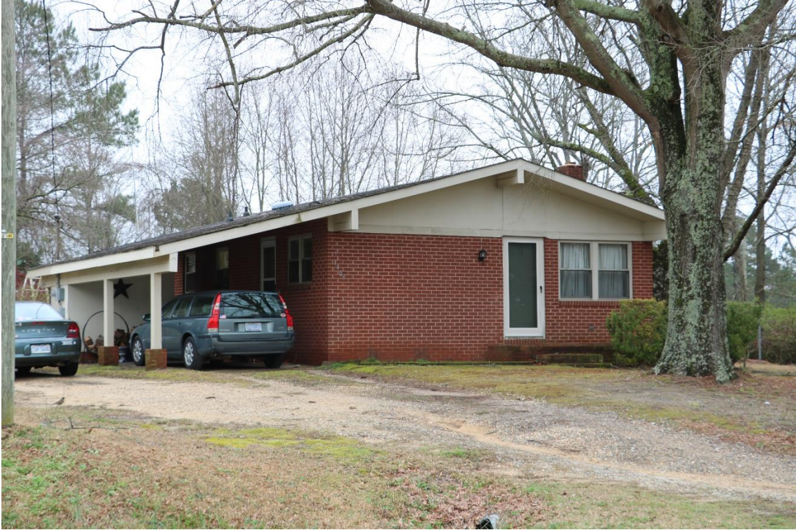
33. House, 1403 Wilbur Jones Road, 1961, PIN 0677024019, view facing east.
