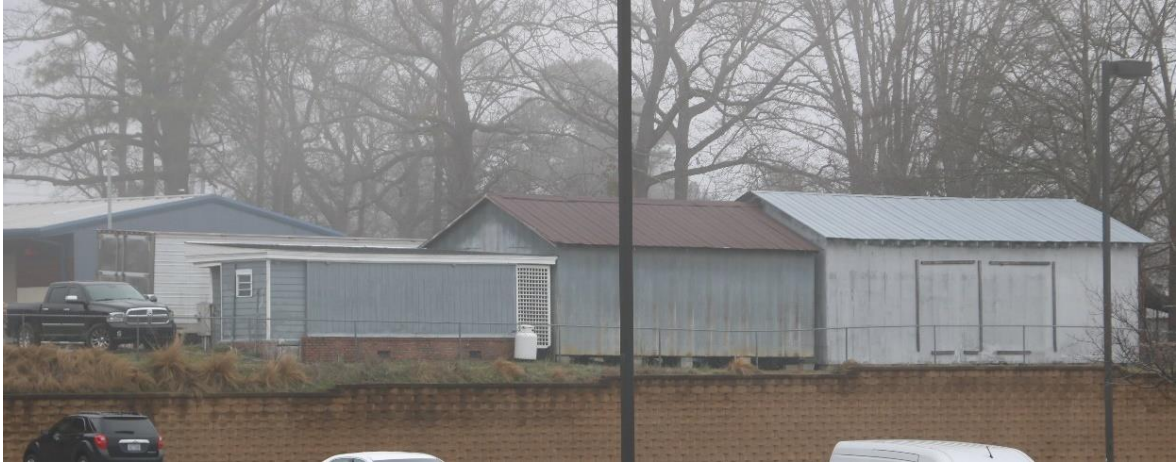
28. Commercial Sheds, 0 N. Main Street, c.1970, PIN 0667915383, view facing northeast.
