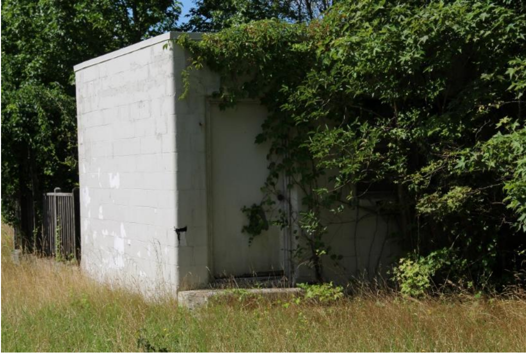
Figure 53. Tudor Revival House, c.1950 concrete-block addition along east elevation, view facing southwest.
