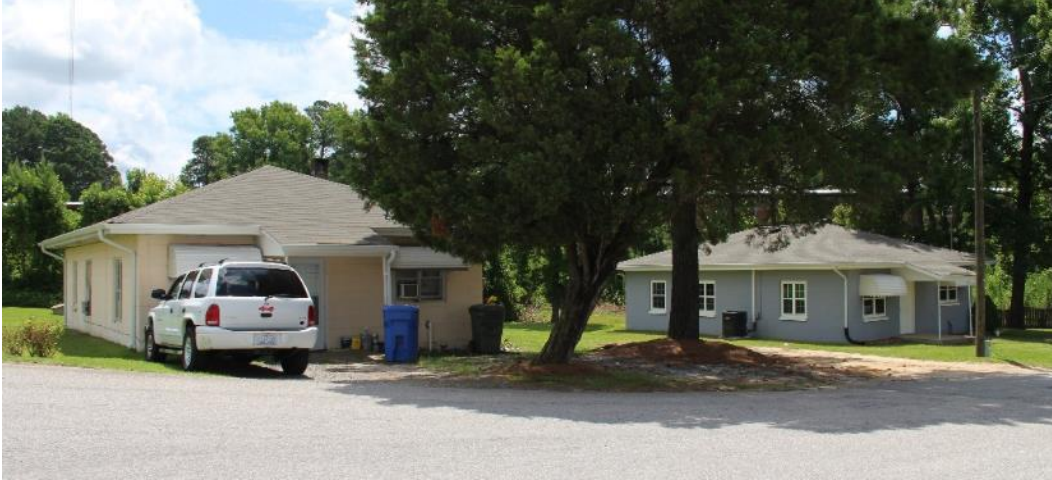
Figure 49. Concrete-block houses at 1830 (left) and 1828 Eakes Street (right), view facing southeast.
