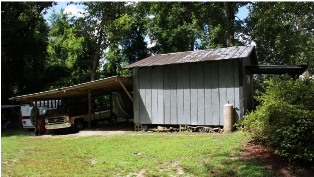
Figure 29. c.1945 shed with shed-roof extension to the rear, view facing southwest.
