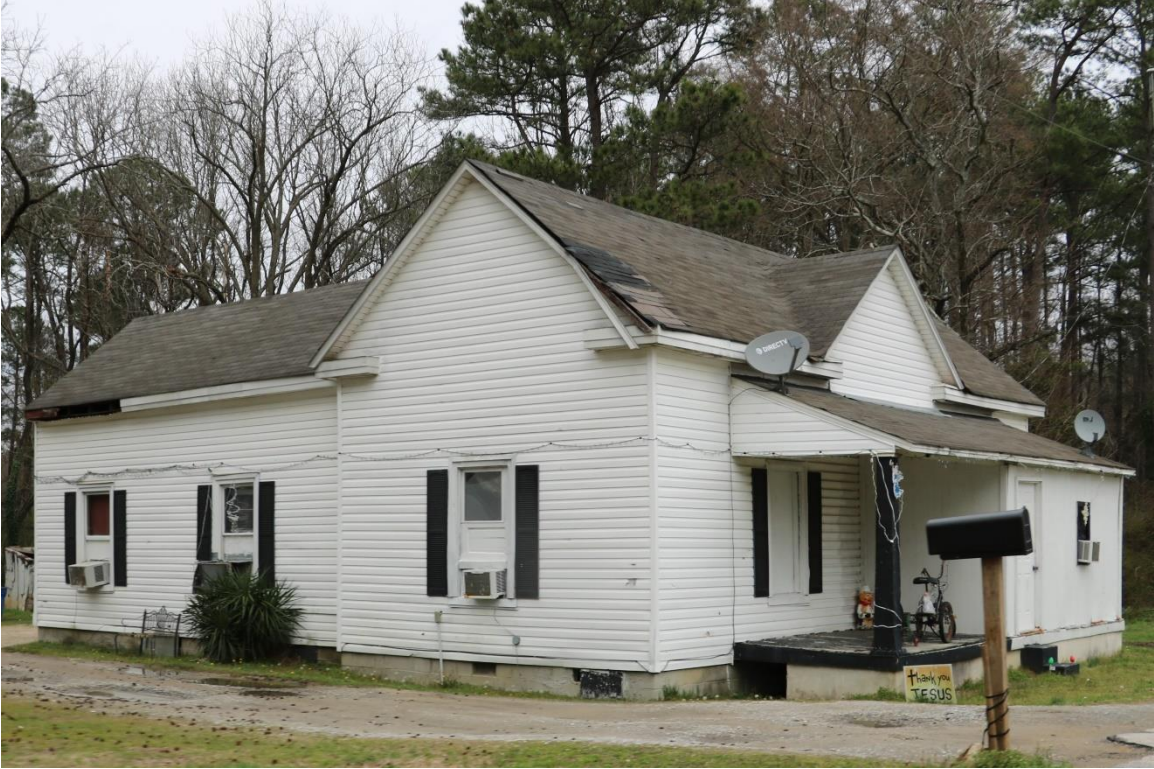
49. House, 7002 Johnson Pond Road, 1920, PIN 0677124893, view facing northeast.
