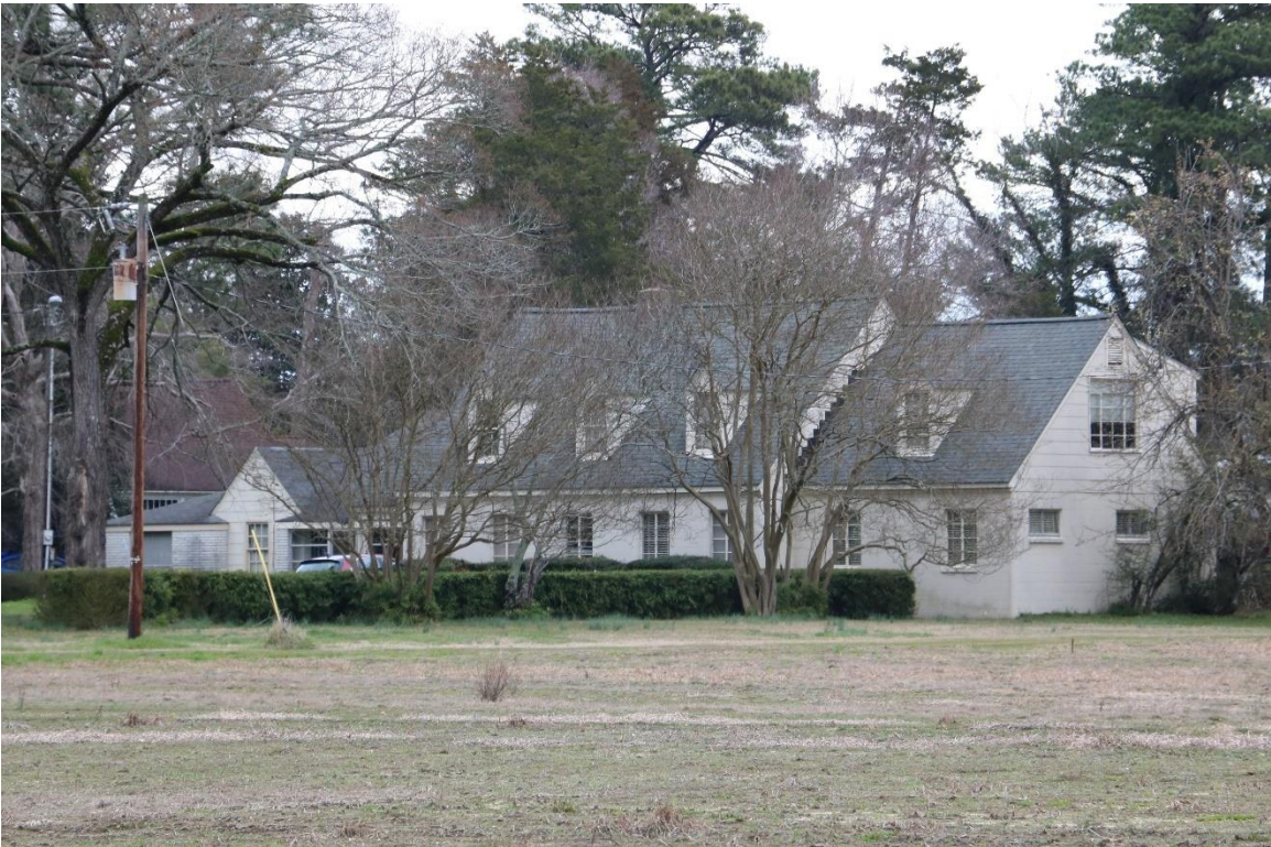
11.c House, 7116 Sunset Lake Road, 1967, PIN 0667758185, view facing northeast.
