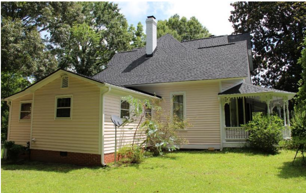
Figure 42. The c.1895 Kemp B. Johnson House, side (southwest) elevation, view facing northeast.
