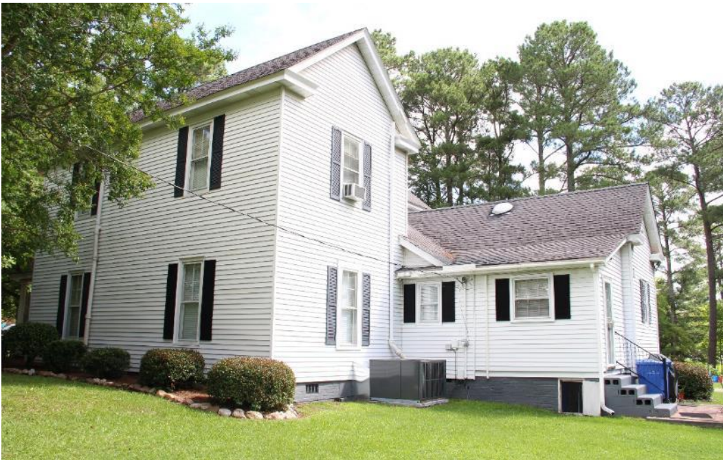
Figure 26. The 1900 Sexton House, southwest elevation, view facing northeast.
