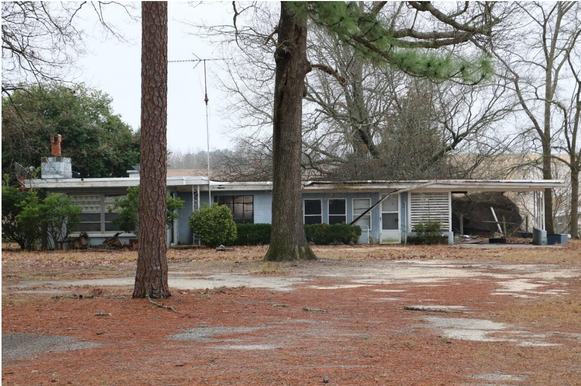
29. House, 1528 N. Main Street, c.1960, PIN 0677010464, view facing southeast.
