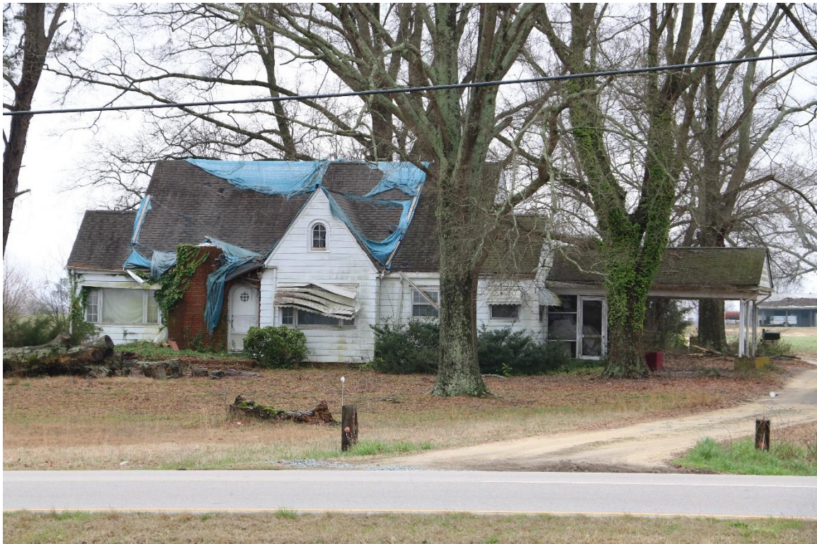
53. House, 1912 N. Main Street, 1949, PIN 0677338829, view facing southeast.
