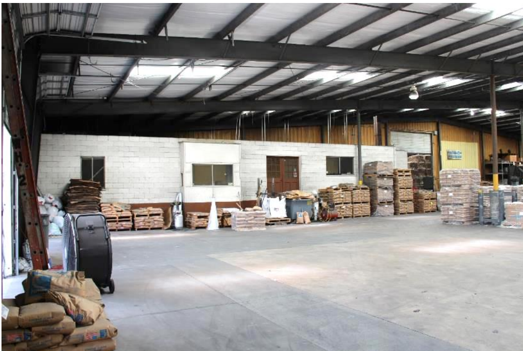
Figure 66. Powell Brothers Warehouse office located in the northwest corner of the 1973 portion. Note the standing seam metal wall and oversized garage door between the two portions of the building.
