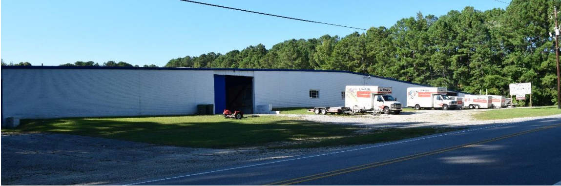
Figure 71. c.1960 New Deal Warehouse (WA7557), view facing north.
