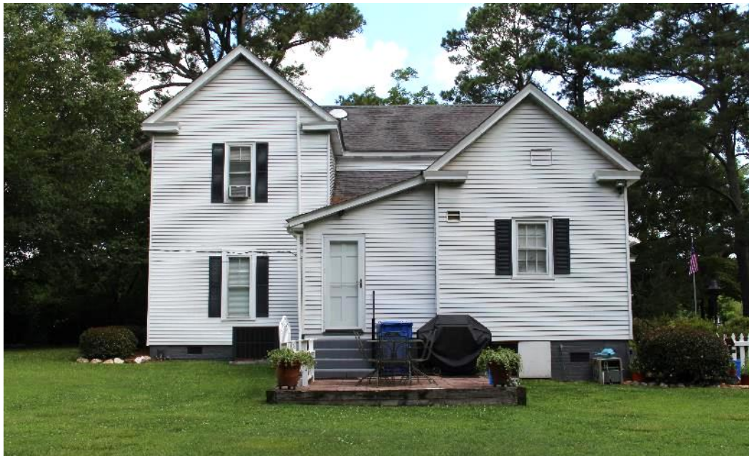
Figure 27. The 1900 Sexton House, southeast elevation, view facing northwest.
