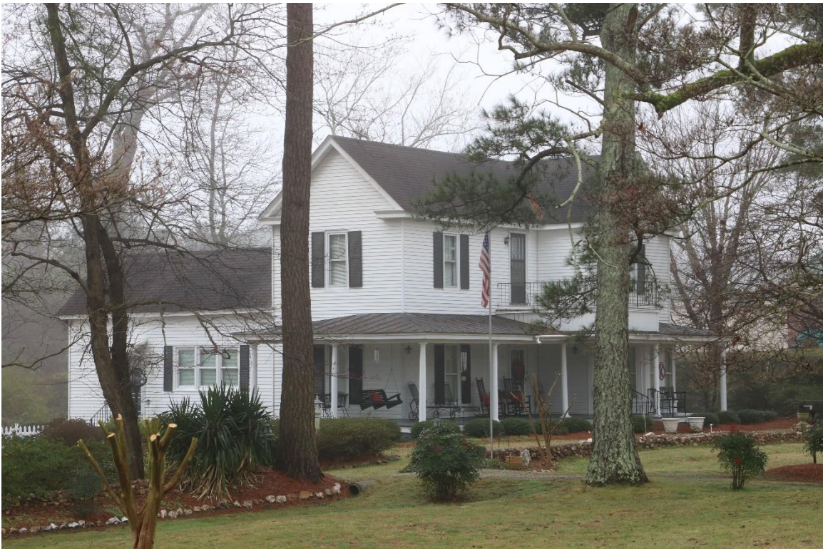
21. Edward Sexton House (WA0573), 1440 N. Main Street, c.1920, PIN 0667805946, view facing south.
