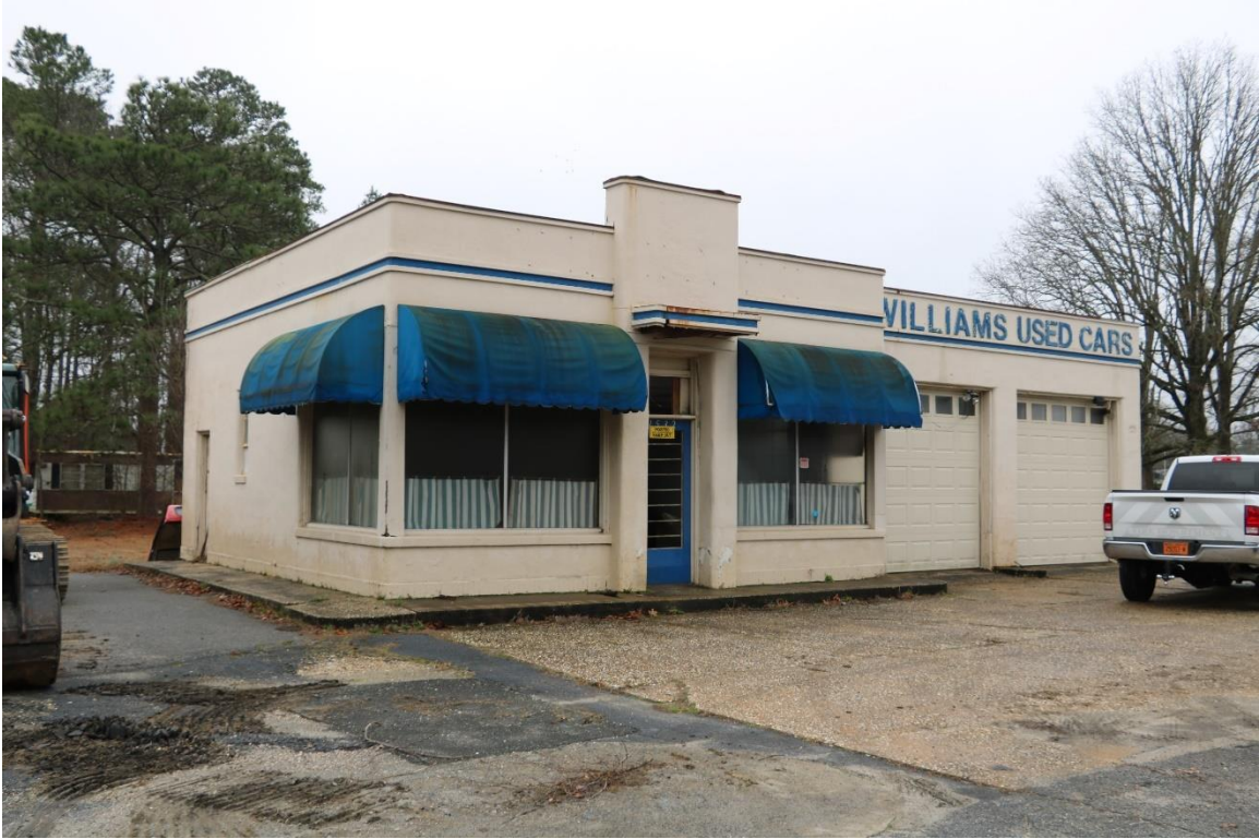
30.a Service station, 1532 N. Main Street, c.1930, PIN 0677012466, view facing south.
