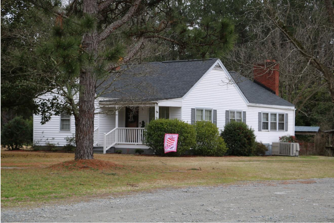
60. House, 1490 NC 42, 1940, PIN 0676795802, view facing southeast.
