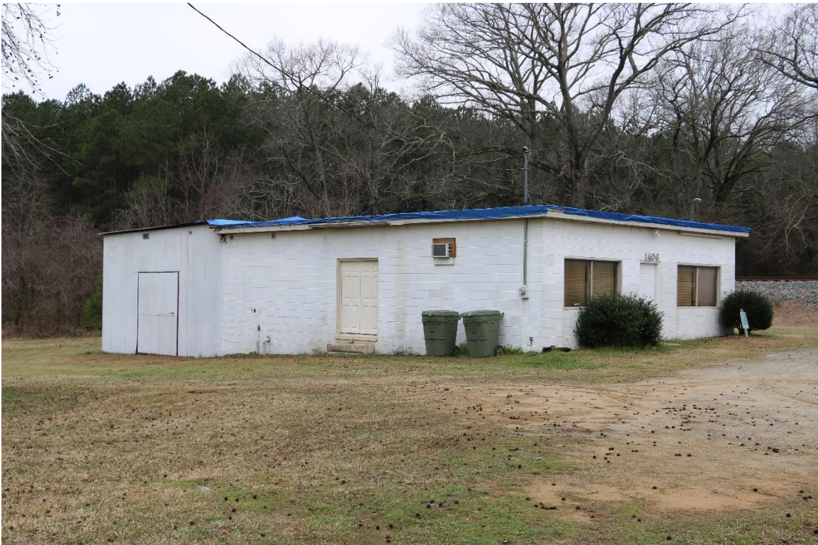
32.b Commercial Building, 1406 Wilbur Jones Road, 1964, PIN 0677012888, view facing northwest.
