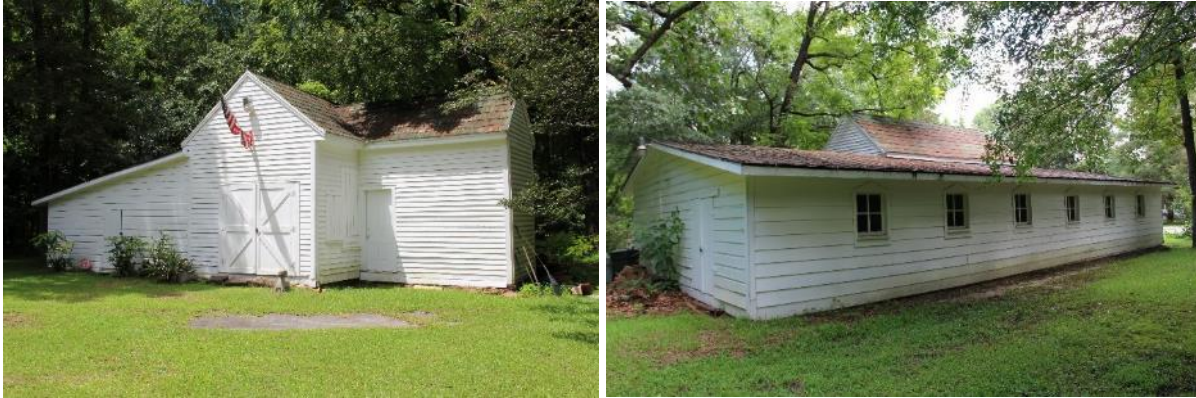
Figure 44. c.1900 carriage house, views facing southwest and northeast.
