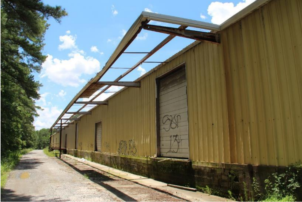
Figure 63. Powell Brothers Warehouse rear (east) elevation, view facing south.
