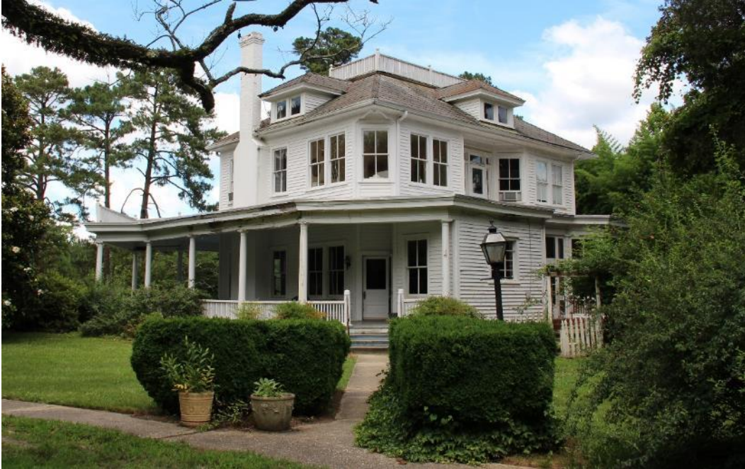
Figure 6. The c.1860 Johnson House, side (west) and rear (south) elevations, view facing northeast.
