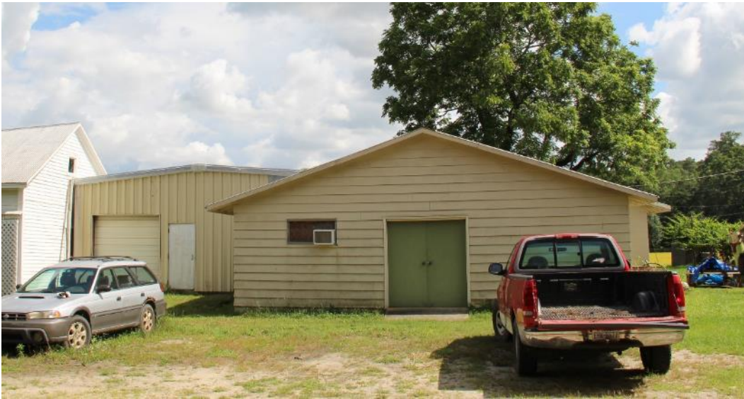
Figure 18. c.1970 storage buildings, view facing south.
