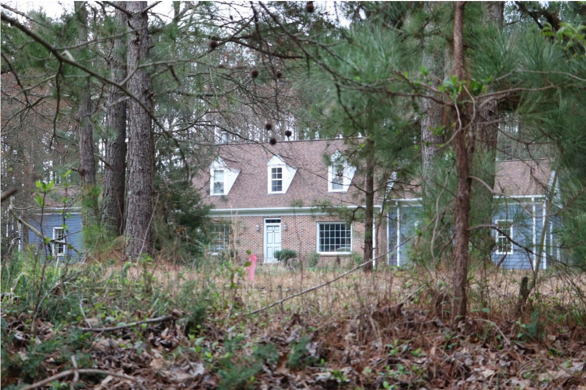
61. 1580 NC 42, 1950, PIN 0676891717, view facing south.
