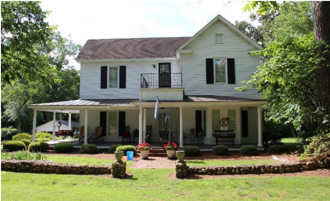
Figure 24. The 1900 Sexton House, northwest-facing facade, view facing southeast.
