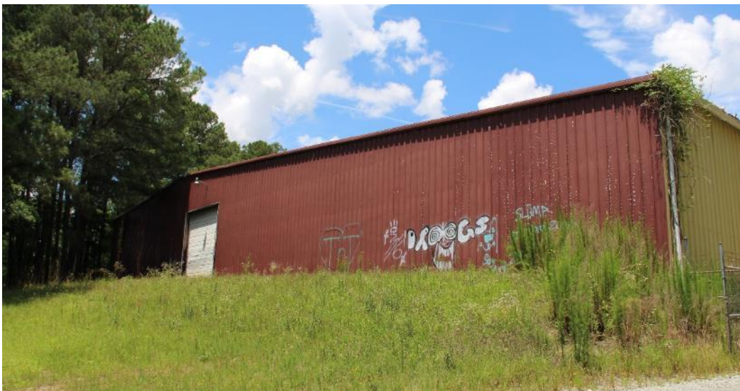
Figure 62. Powell Brothers Warehouse side (south) elevation, view facing northwest.
