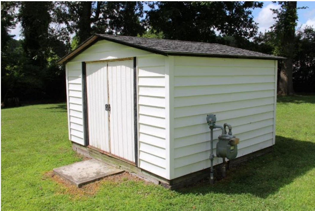
Figure 31. c.1945 pump house, view facing south.
