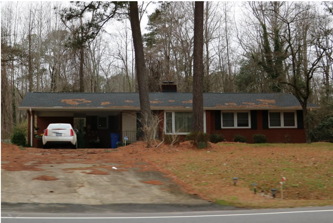
38. House, manufactured single-wide, 6304 South NC 55, 1962, PIN 0676290005, view facing west.
