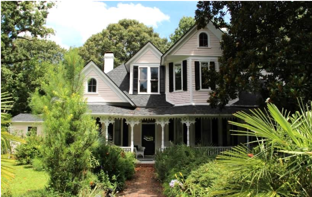
Figure 40. The c.1895 Kemp B. Johnson House, southeast-facing facade, view facing northwest.
