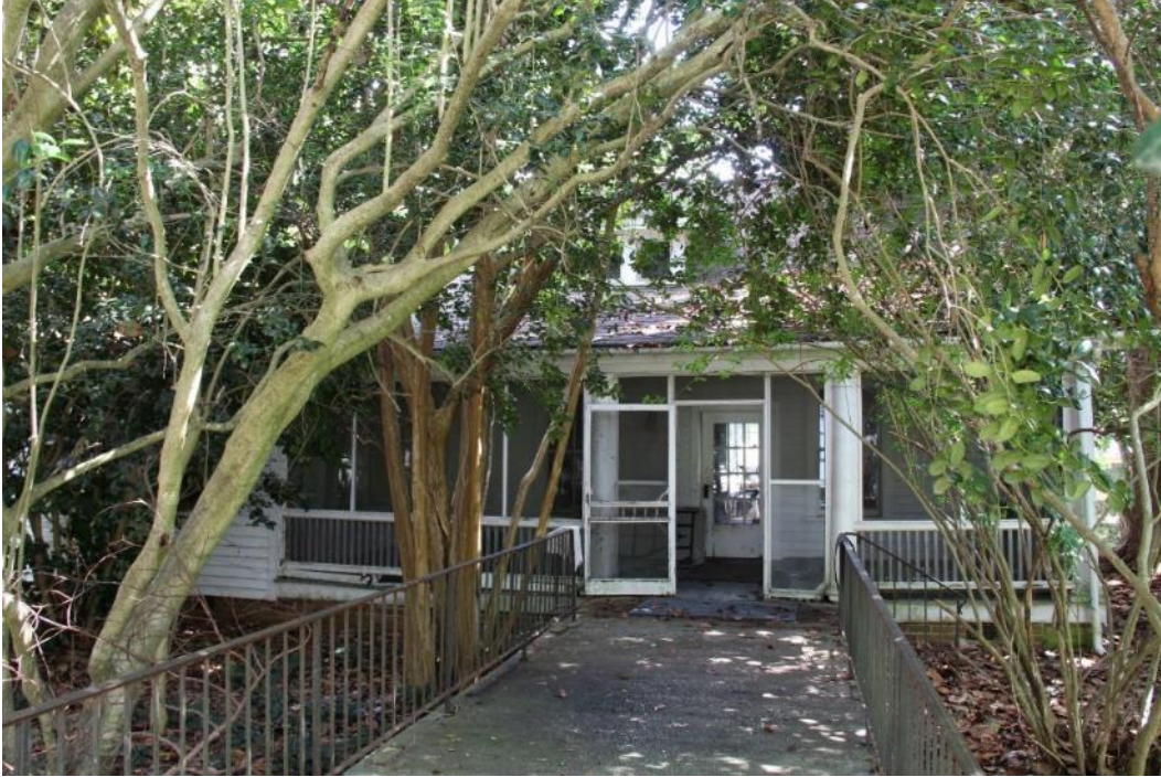
Figure 11. The c.1800 Jones House, view facing south from the Johnson House with the walkway in the foreground.
