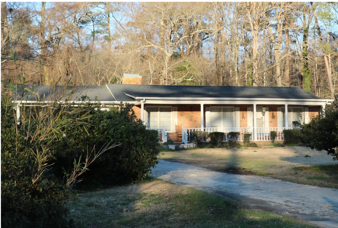
39. House, 6316 South NC 55, 1961, PIN 0676280719, view facing west.
