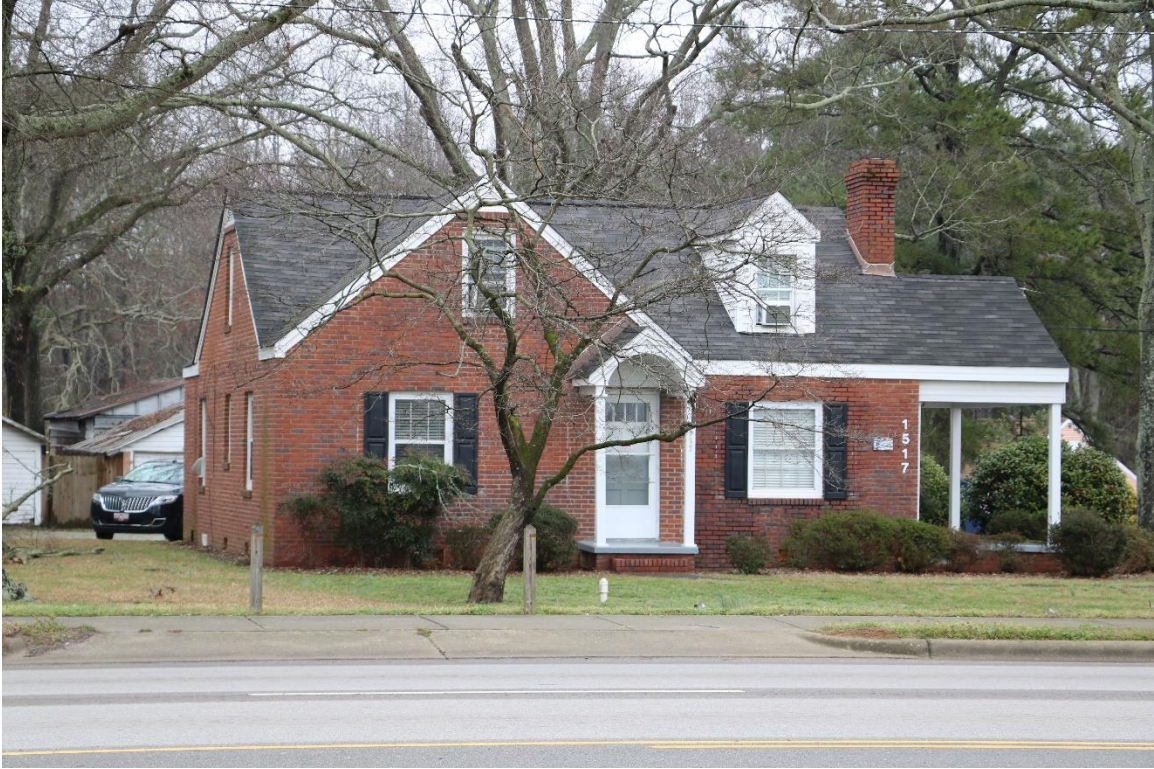
26. 1517 N. Main Street, 1945, PIN 0667917607, view facing north.
