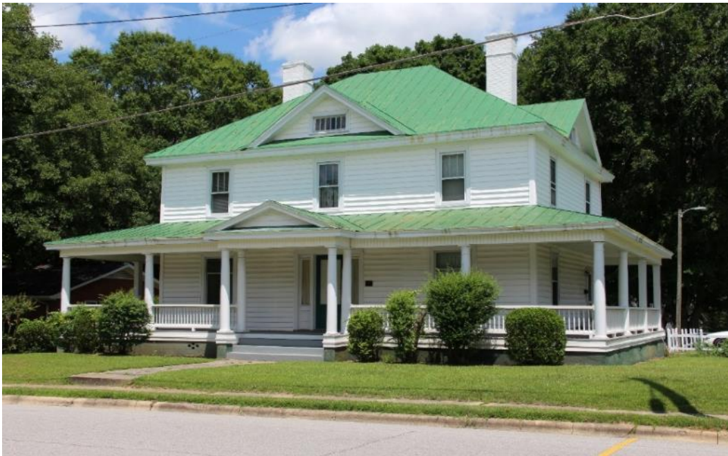
Figure 35. The c.1915 T.H. Stephenson House (WA0481) at 501 N. Ennis Street.
