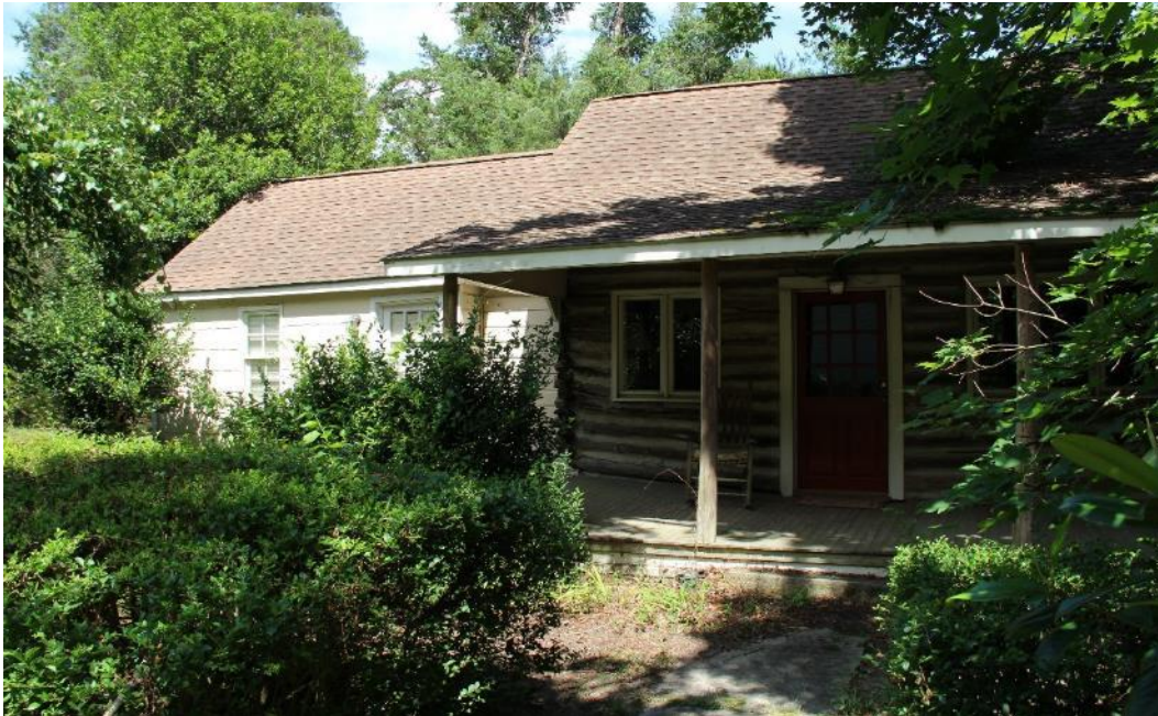
Figure 9. c. 1780 log cabin, view facing east.
