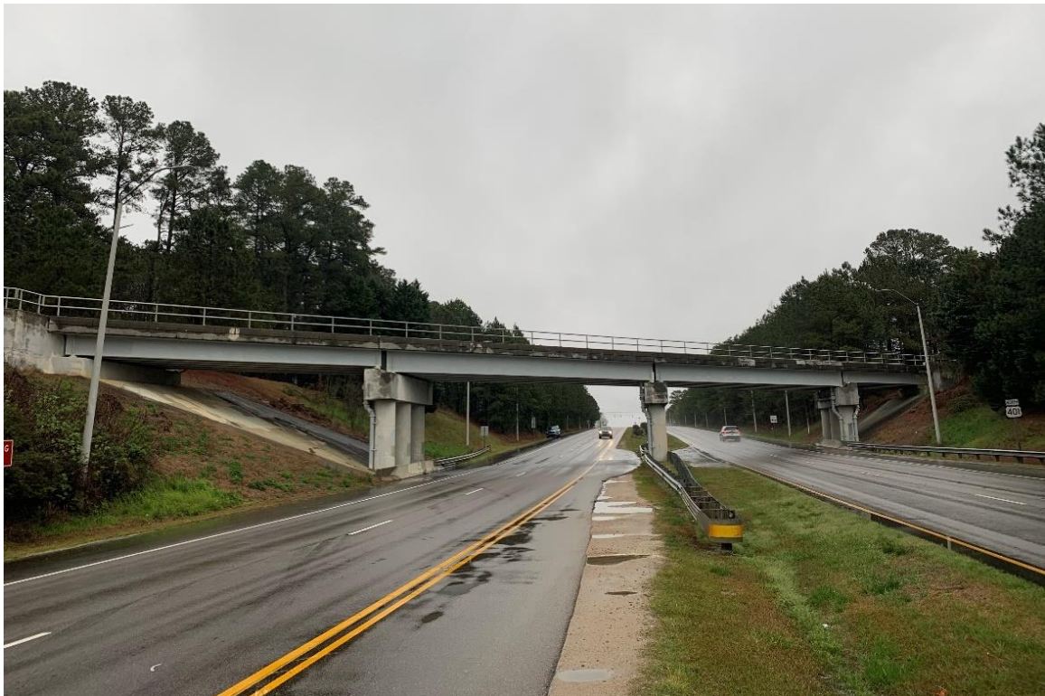
63. Norfolk Southern Railway Bridge over US 401, view facing northeast.
