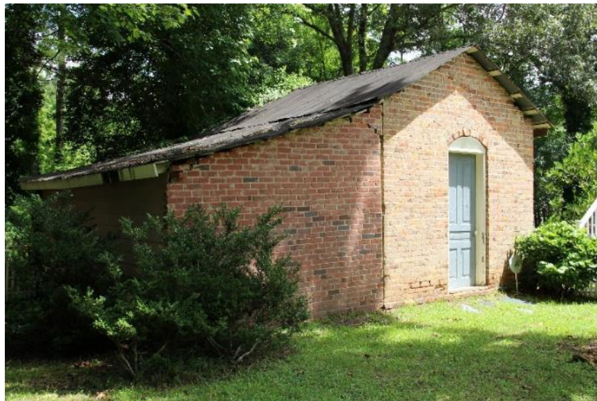
Figure 45. c.1895 storage building, view facing northeast.
