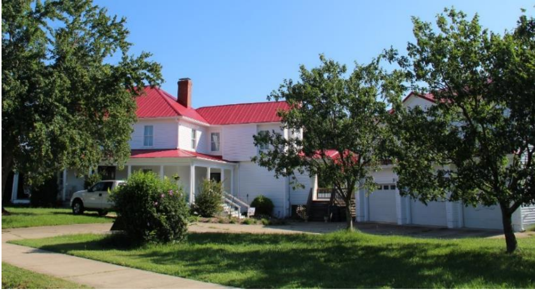
Figure 36. The c.1900 Bryant Brewer House (WA0650) at 201 Grigsby Avenue.
