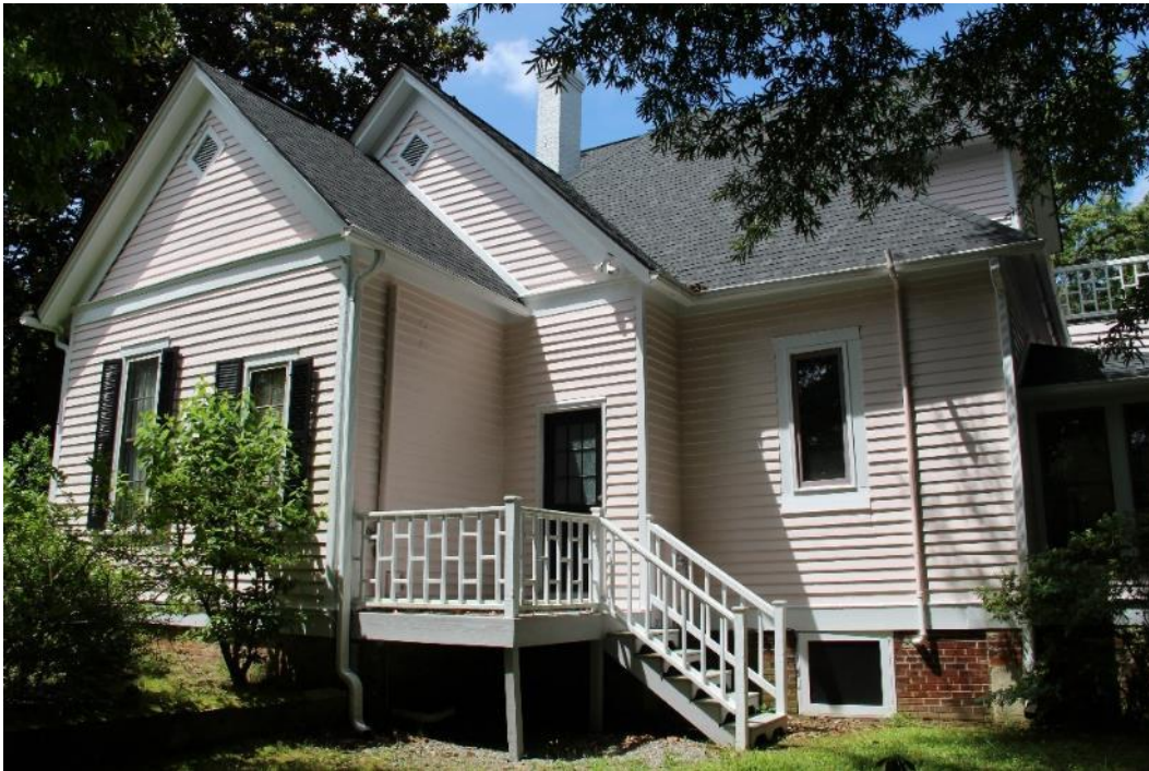
Figure 41. The c.1895 Kemp B. Johnson House, side (northeast) elevation, view facing southwest.
