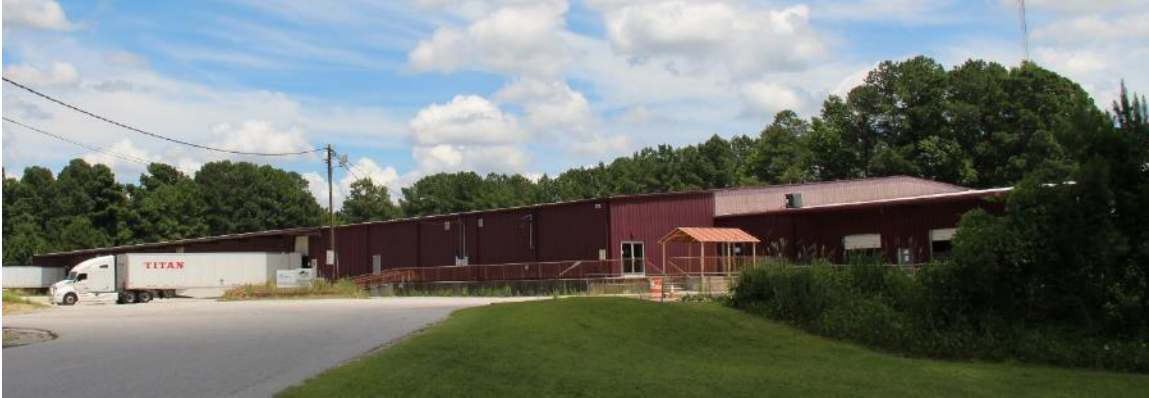
Figure 58. The 1971 and 1973 Powell Brothers Warehouse, west-facing facade, view facing east.
