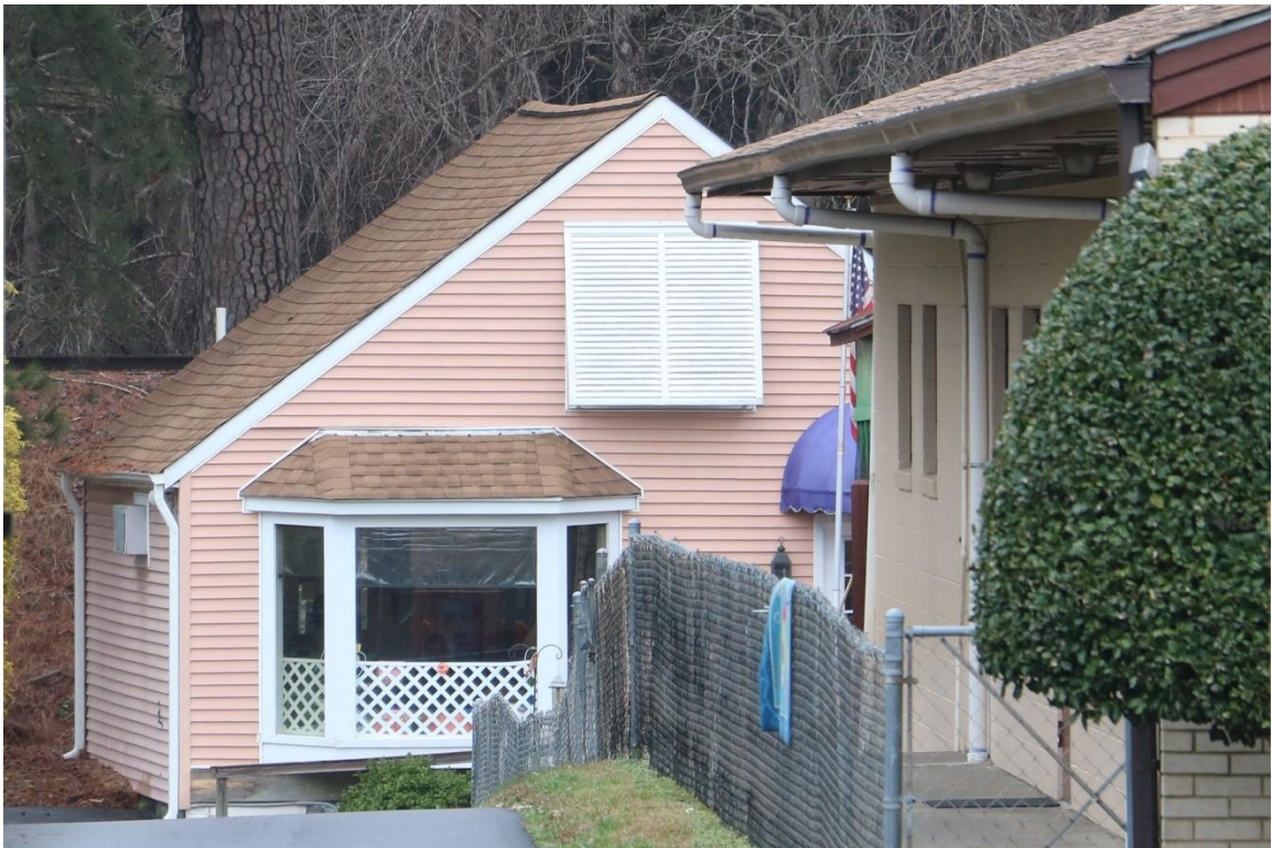
27. 1521 N. Main Street, c.1940, PIN 0667918629, view facing north.
