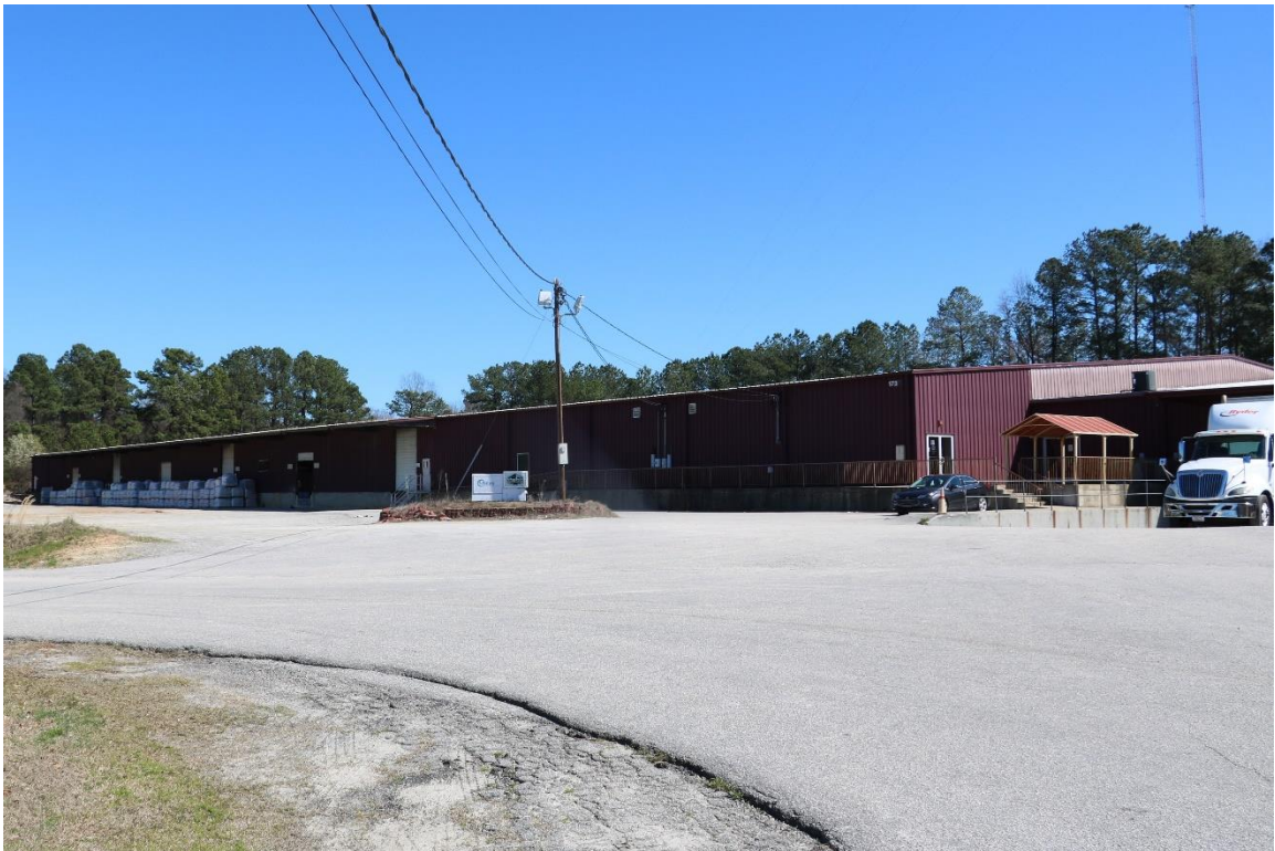
48. Powell Brothers Warehouse, 1730 Five Points Lane, c.1971, PIN 0677225246, view facing east.
