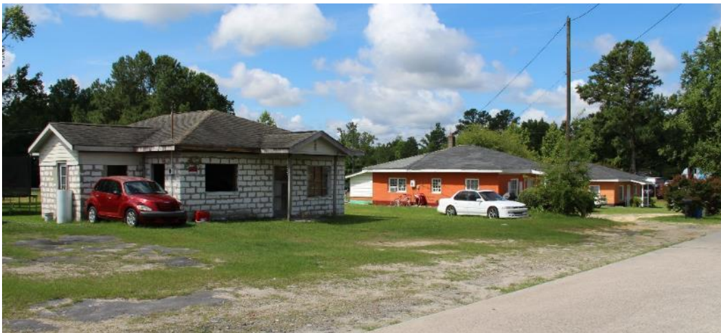
Figure 48. Concrete-block houses at 1718, 1712, and 1708 Five Points Lane (left to right), view facing southwest.
