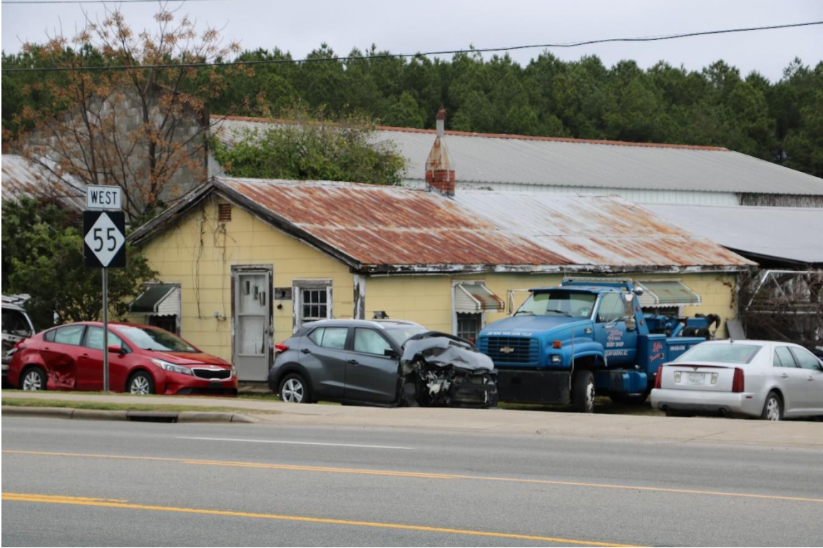
2.b Converted house, 1200 N. Broad Street, c. 1930, PIN 0657931229, view facing northeast.
