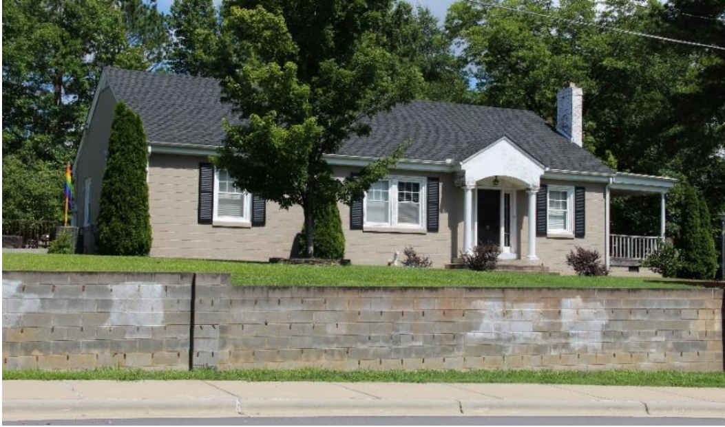
Figure 55. Concrete-block house with Colonial Revival features and concrete-block retaining wall at 313 Spring Avenue in Fuquay-Varina, view facing southeast.
