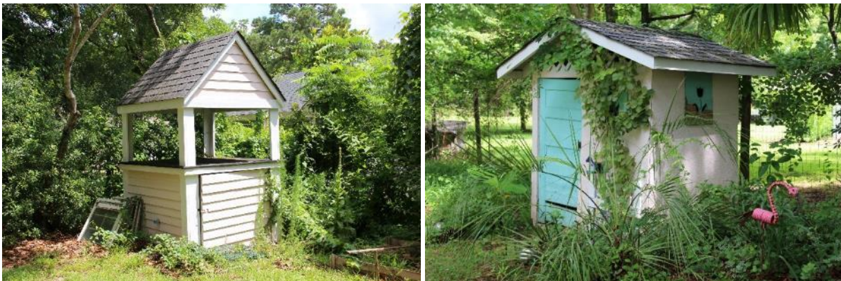
Figure 46. c.1950 well, view facing northeast, and c.2010 shed, view facing northwest.
