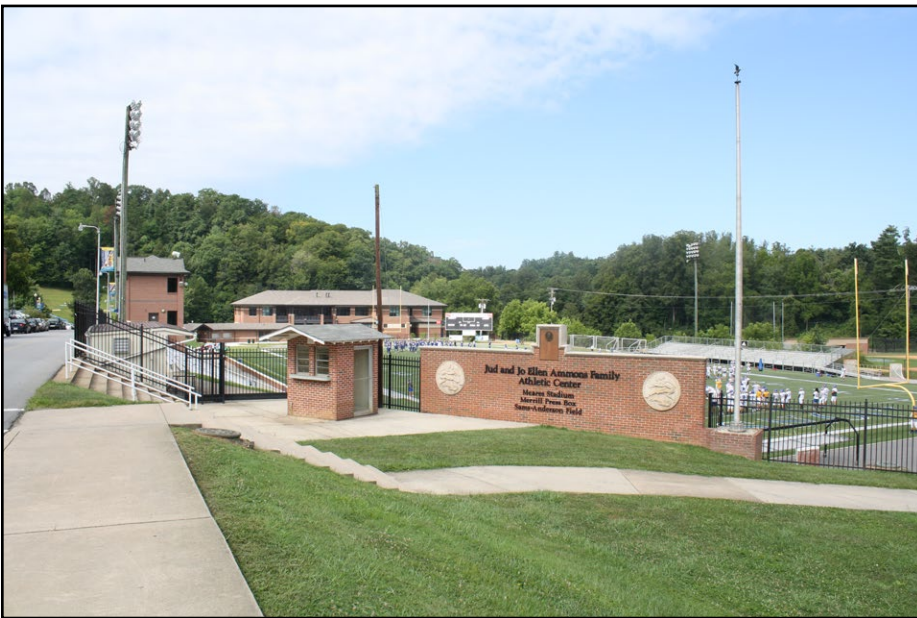
Plate 4.5 View from Athletic Street to the Ammons Family Athletic Center, which is located southwest of the Chambers Gymnasium and Harrell Pool.
