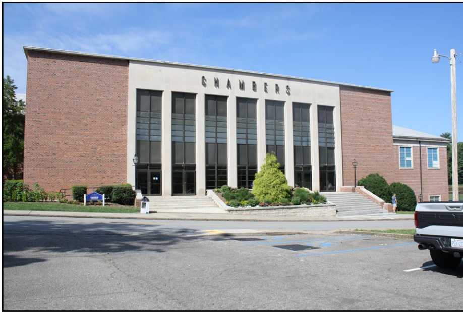
Plate 4.10 View of the northeast elevation of the Chambers Gymnasium and Harrell Pool showing the entry pavilion.
