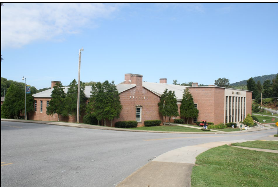
Plate 4.16 View of the northeast elevation of the Chambers Gymnasium and Harrell Pool at the intersection of Bailey Street and Athletic Street.
