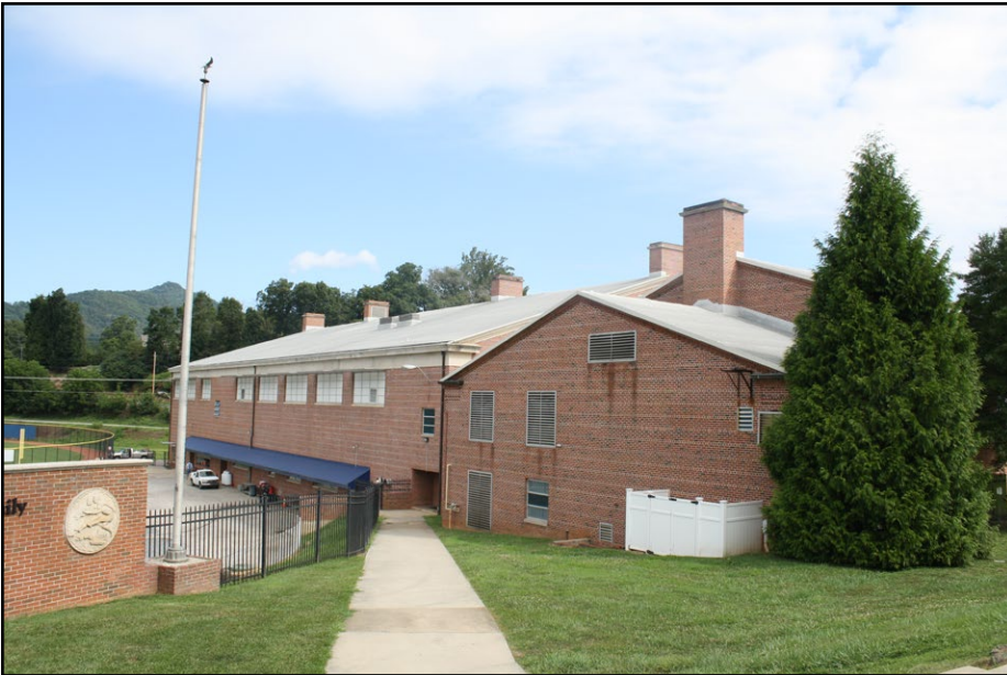
Plate 4.14 View of the southwest elevation of the Chambers Gymnasium and Harrell Pool showing a paved walkway from Athletic Street.
