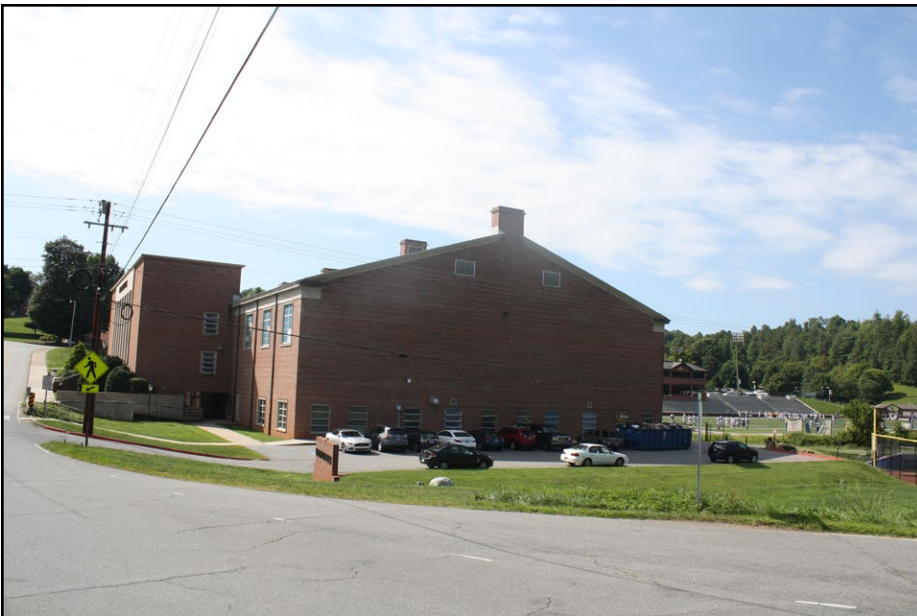
Plate 4.12 View of the parking lot and an unnamed driveway at the northeast corner of the Chambers Gymnasium and Harrell Pool, showing the intersection of Hickory Street and Bailey Street and Bridge No. 184 at the center-far left of the photograph.
