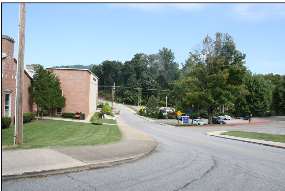
Plate 4.3 View of northeast elevation of the Chambers Gymnasium and Harrell Pool along Bailey Street.
