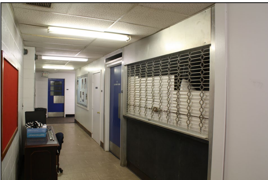
Plate 4.27 View of the equipment room and classrooms in the basement of the Chambers Gymnasium and Harrell Pool.
