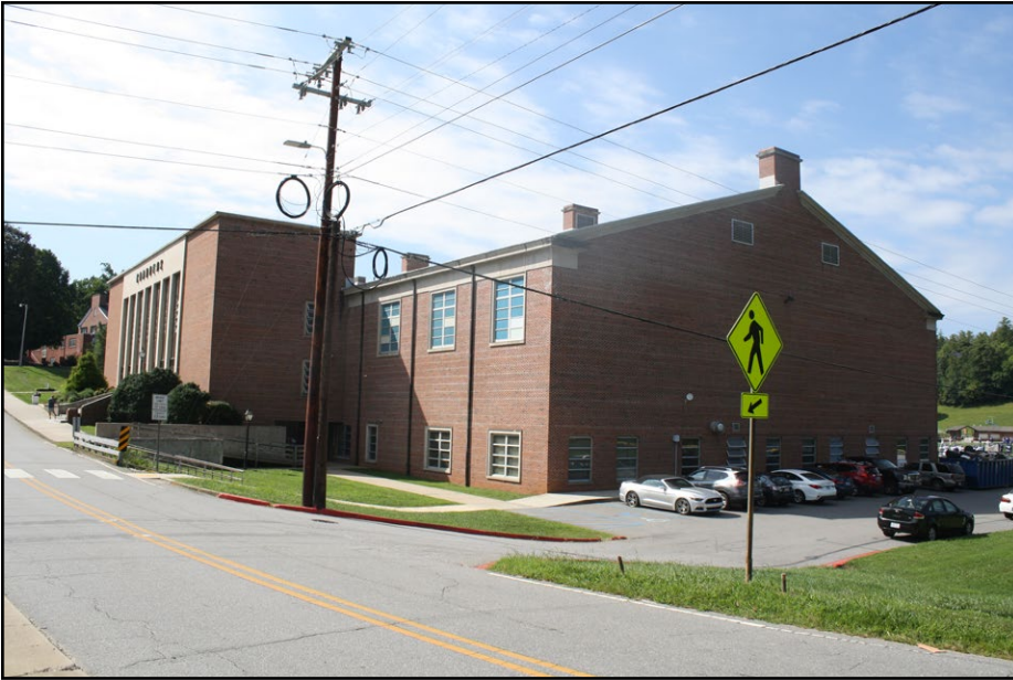
Plate 4.11 View of the northwest elevation of the Chambers Gymnasium and Harrell Pool.
