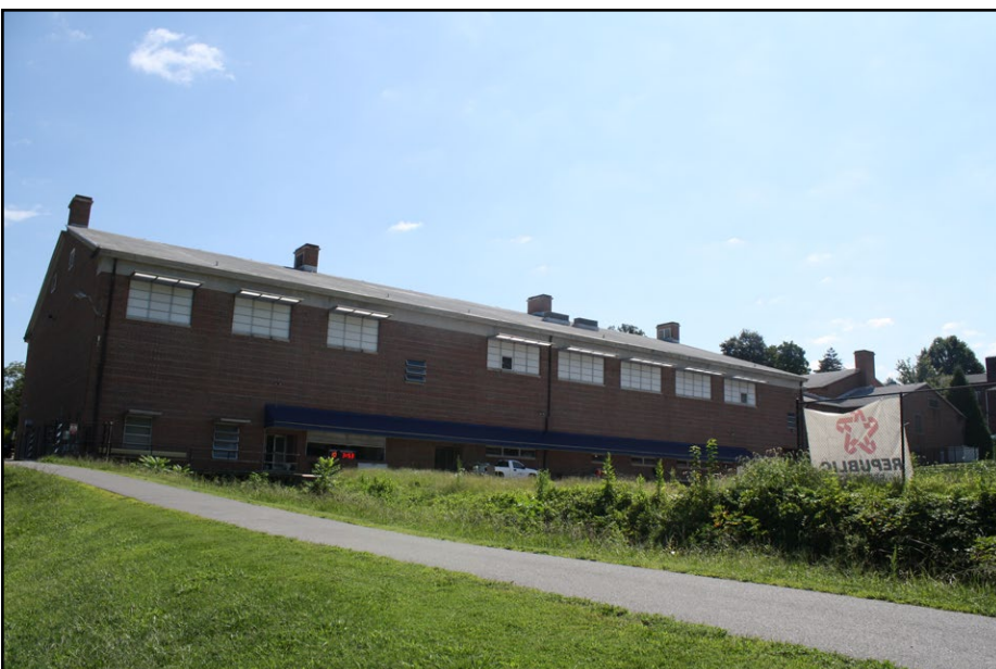
Plate 4.13 View of the southwest elevation of the Chambers Gymnasium and Harrell Pool.
