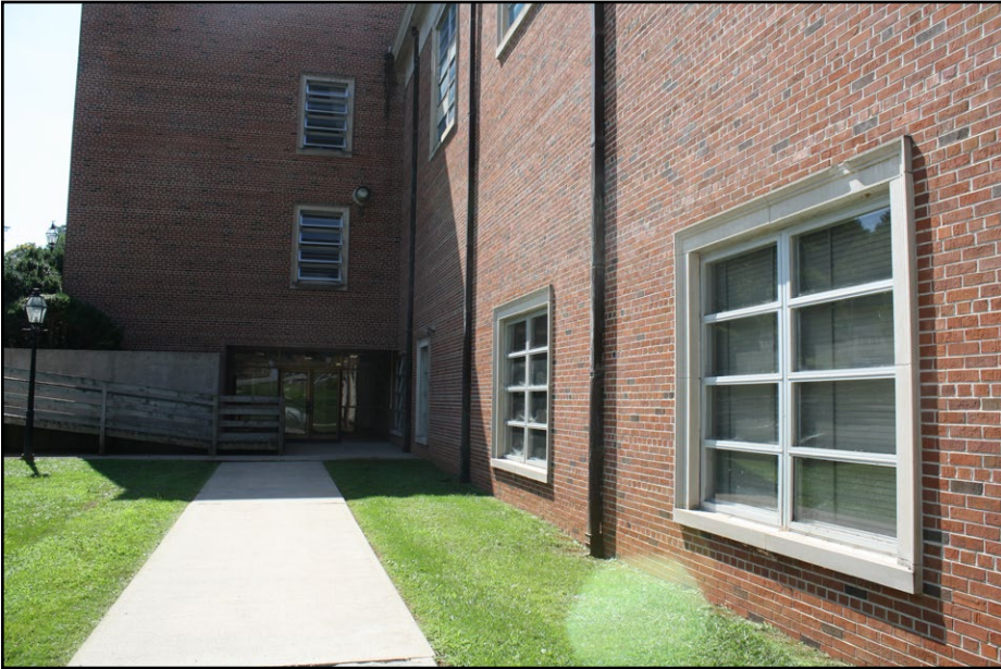
Plate 4.18 View of a paved walkway from the parking lot at the northeast corner of the Chambers Gymnasium and Harrell Pool showing an entryway to the building's basement.
