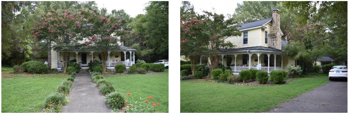
Figure 3. Left, view of façade, looking south; right view of northeast corner, looking southwest
