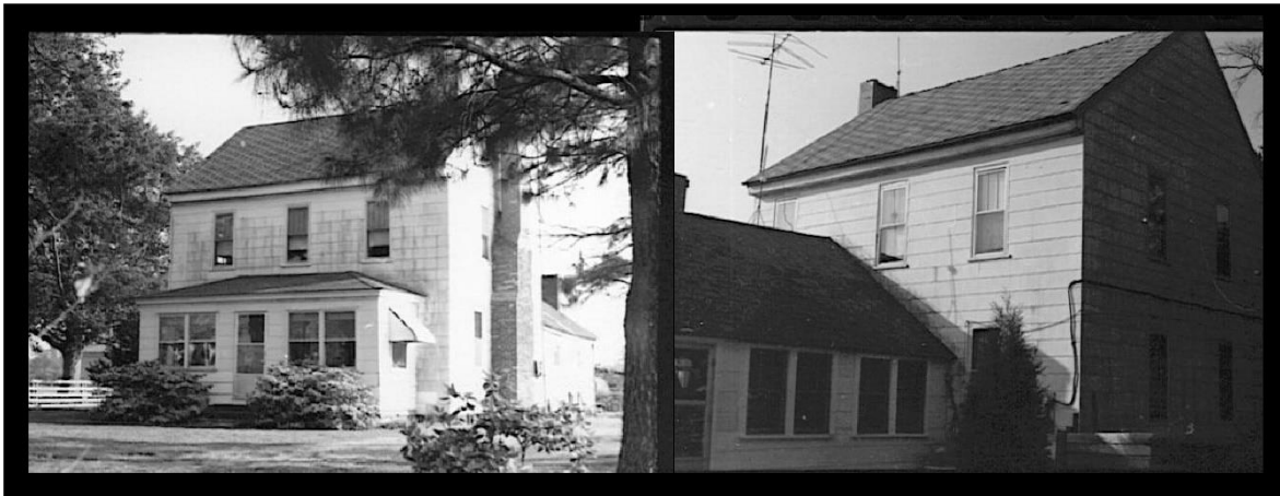
Figure 24: G. M. Bray House (HPO Survey File, CM0046).
