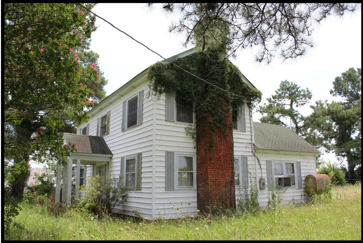
Figure 6: Gregory House, Looking Southeast.
