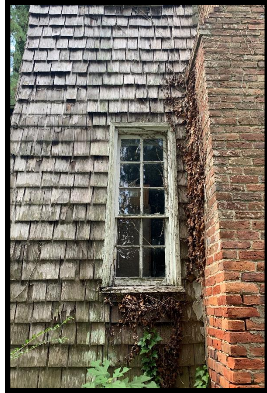
Figure 91: Morrisette House, Window Detail.
