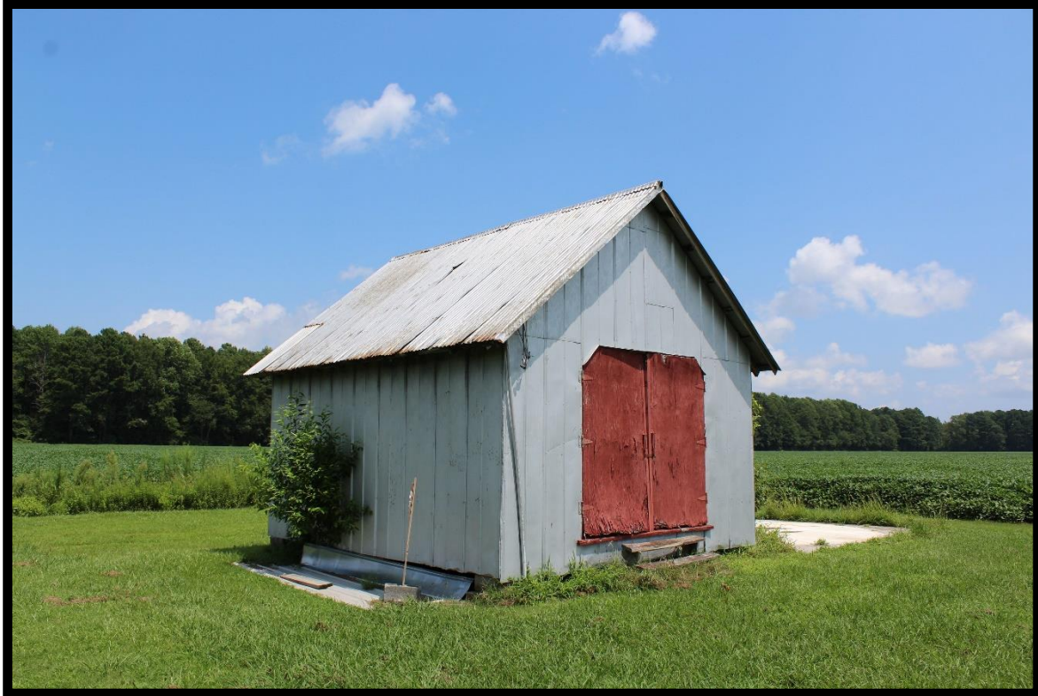
Figure 77: Nash Place, Shed, Looking Northeast.
