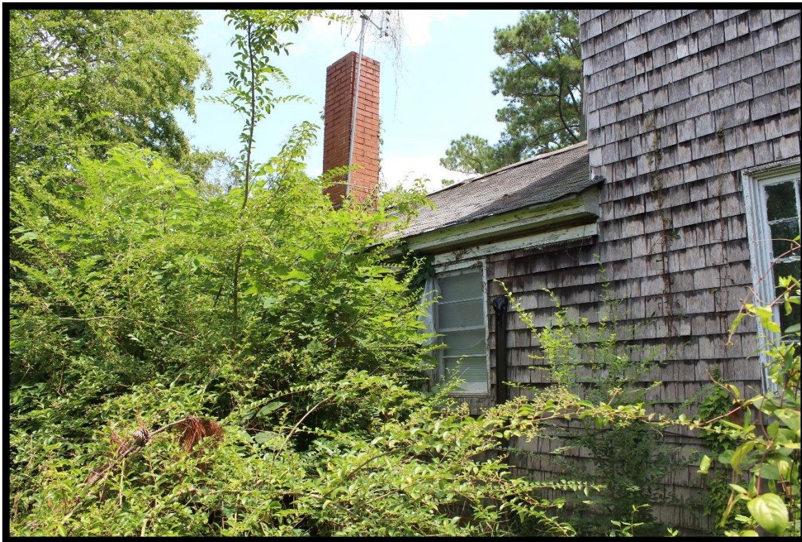
Figure 95: Morrisette House, Looking South.
