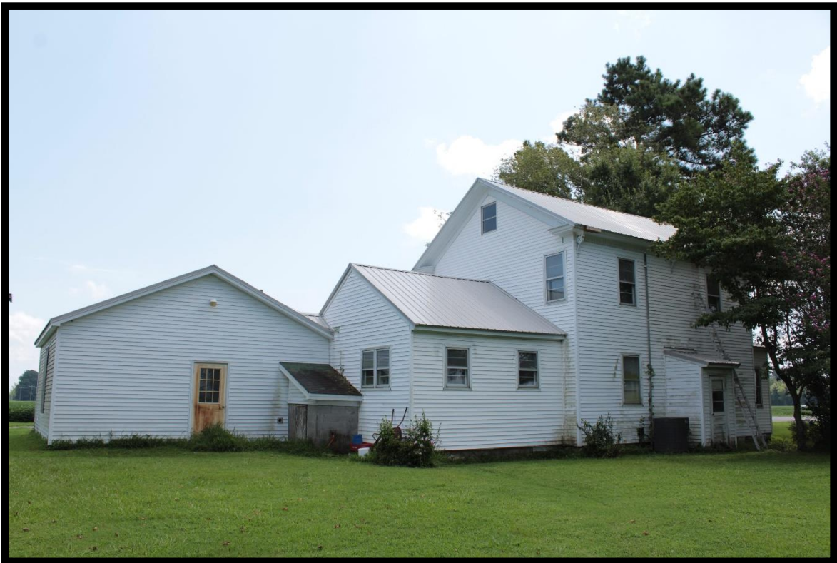
Figure 70: Nash Place, Looking Southeast.
