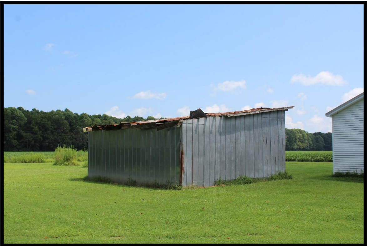
Figure 76: Nash Place, Shed, Looking Northeast.
