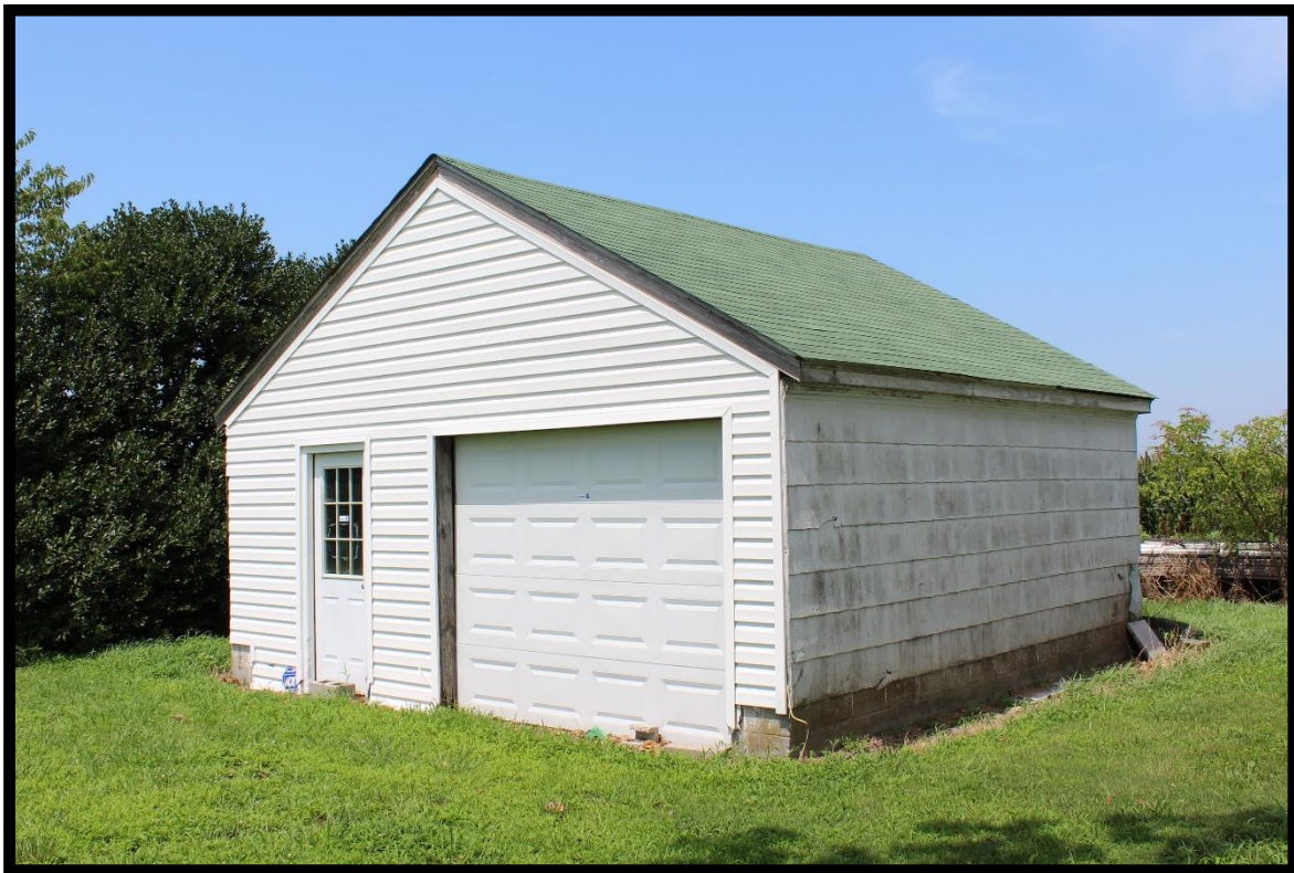
Figure 57: Berry House, Garage, Looking North.
