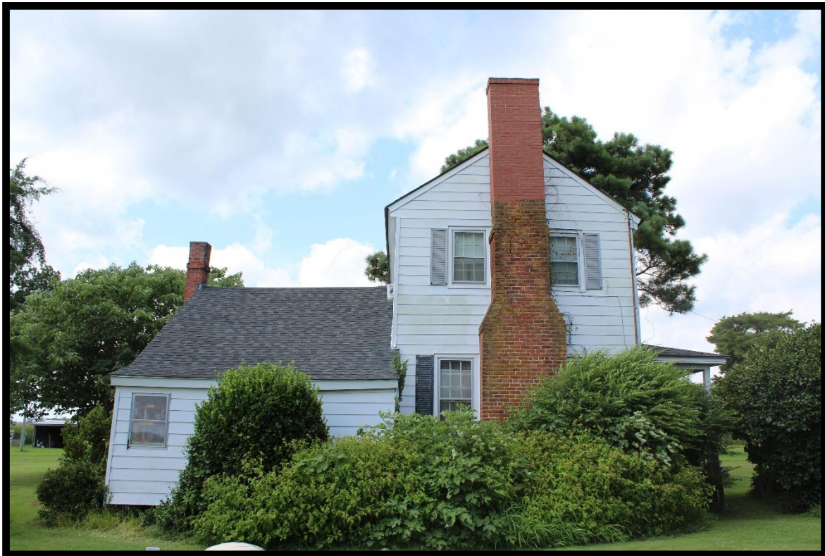
Figure 112: Hughes-Williams House, Looking Northwest.
