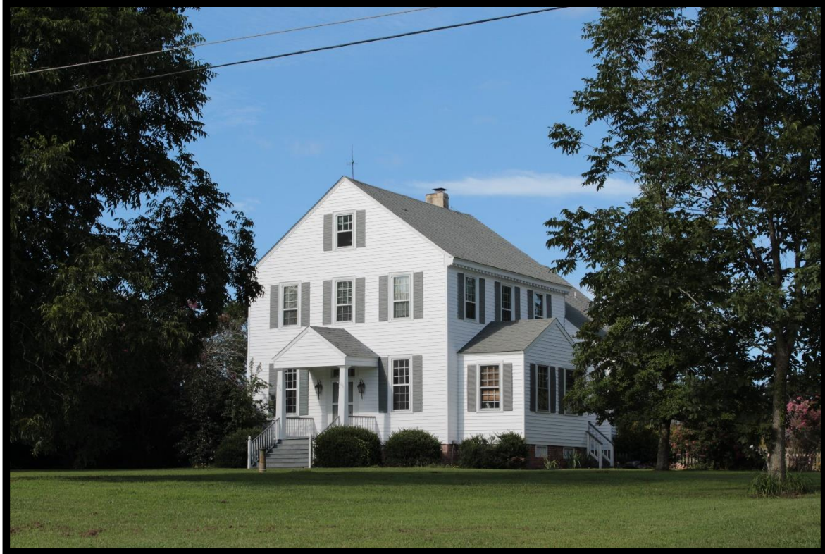
Figure 84: Culong (CK0006), Looking North.
