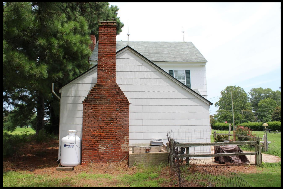
Figure 18: G. M. Bray House, Looking North.
