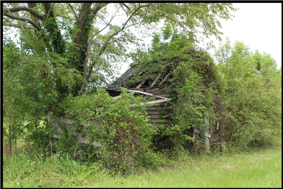
Figure 41: Stevens House, Shed, Looking North.
