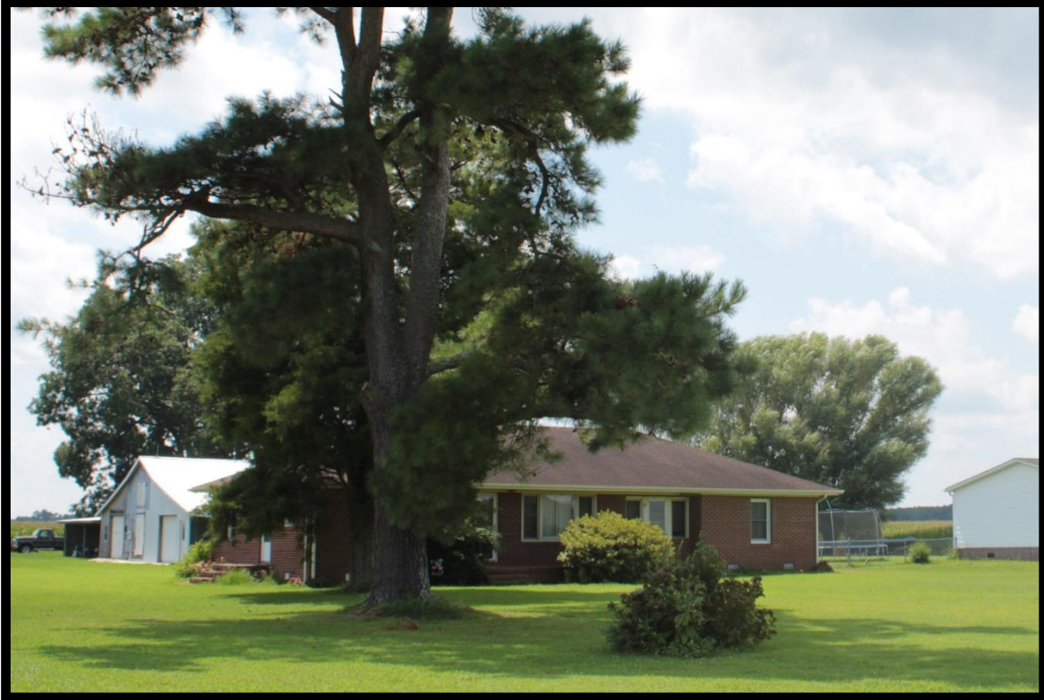
Figure 116: Hughes-Williams House, 1964 Dwelling, Looking East.
