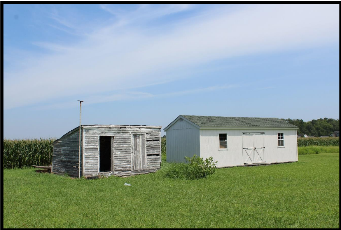
Figure 59: Berry House, Sheds, Looking East.
