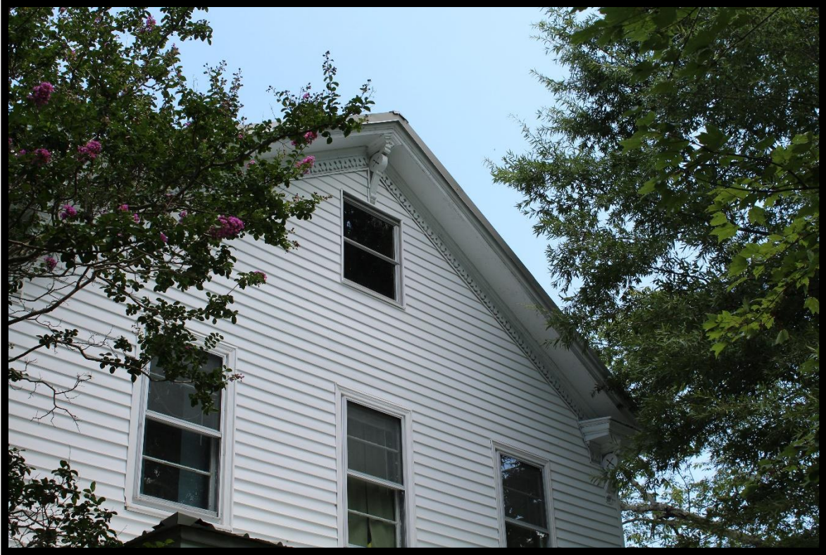
Figure 69: Nash Place, Façade, Detail of Eave.
