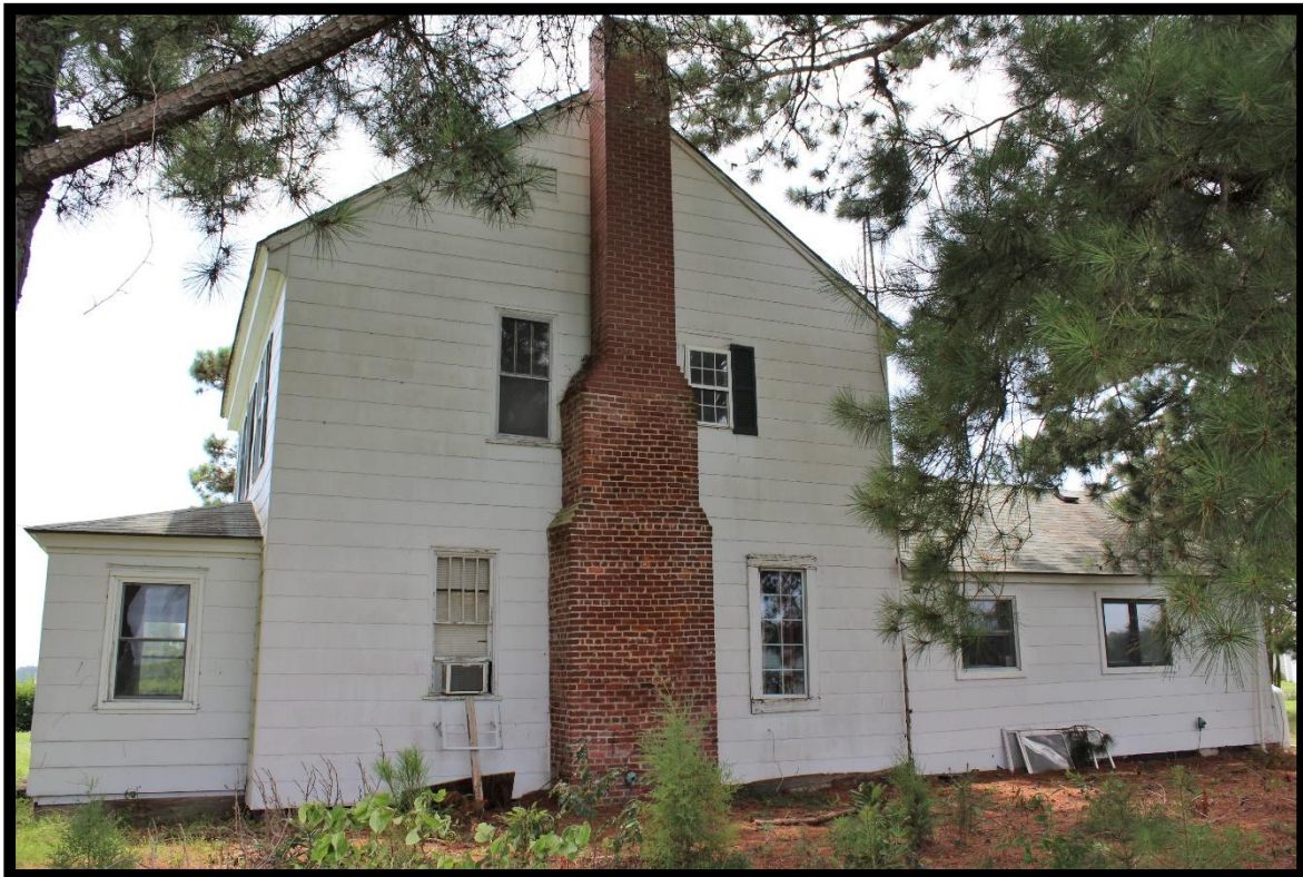
Figure 16: G. M. Bray House, Looking Southeast.
