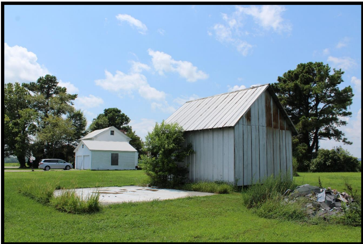
Figure 78: Nash Place, Shed and Concrete Slab, Looking Southwest.
