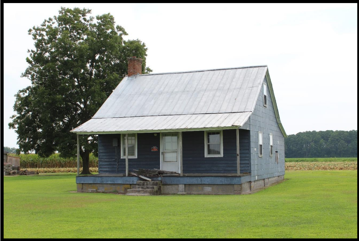
Figure 45: Charles Whitehurst House (CM0167), Looking Southwest.
