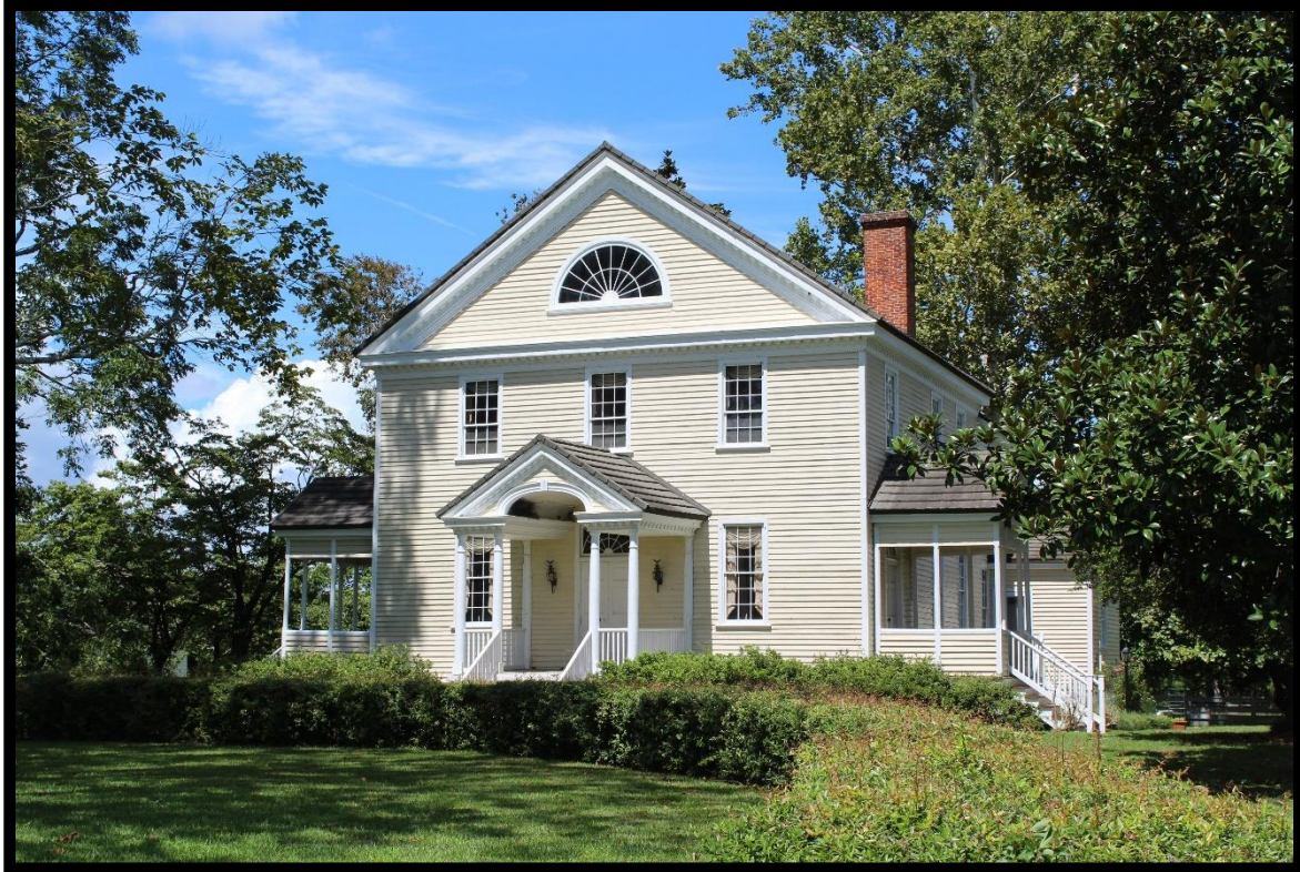
Figure 65: Morgan House, Looking North.
