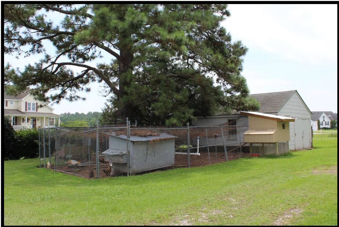
Figure 21: G. M. Bray House, Chicken Houses, Looking Southeast.
