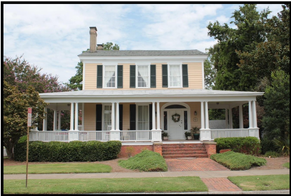
Figure 103: Hinton-Pailin House (PK0038), Looking North.
