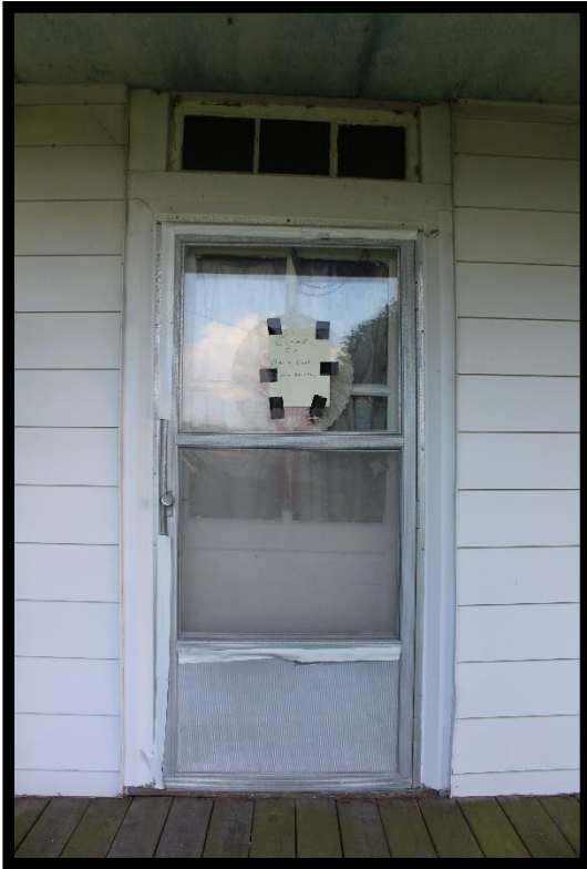
Figure 108: Hughes-Williams House, Front Door.
