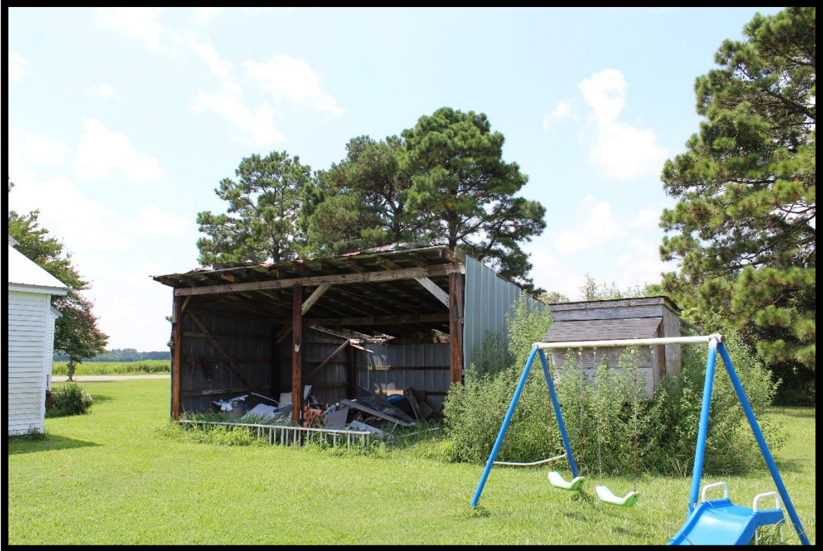
Figure 75: Nash Place, Shed, Looking Southwest.
