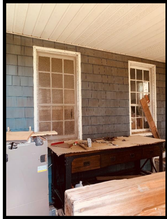
Figure 89: Morrisette House, Front Windows.
