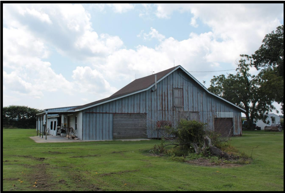
Figure 117: Hughes-Williams House, Barn, Looking West.
