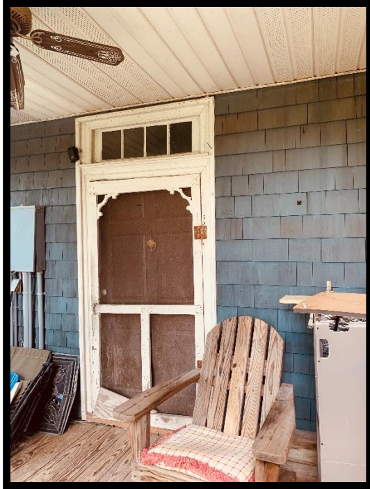
Figure 88: Morrisette House, Front Door.
