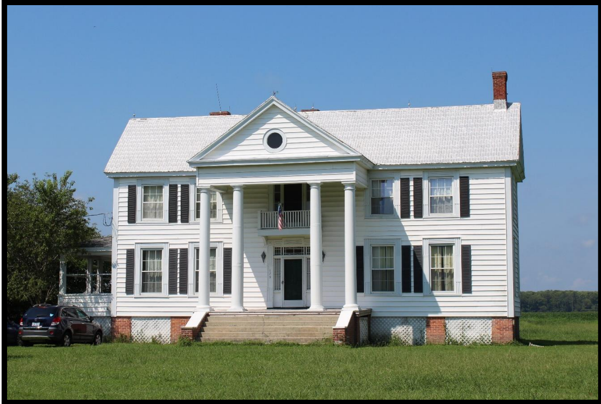
Figure 12: William Riley Abbott House (CM0003), Looking Southwest.
